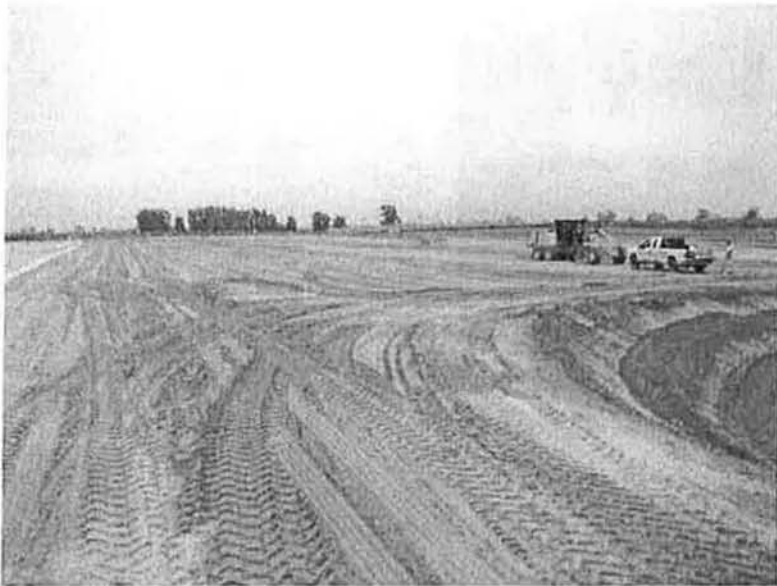
Sludge drying bed subgrade compacted and ready for aggregate base
