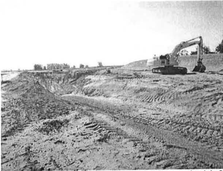
Continued excavation for Clarifiers No. 1 & 2, approximately 65% complete
