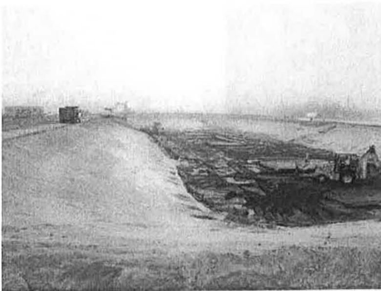
Liner removed and continued removal of sludge from Pond No. 1
