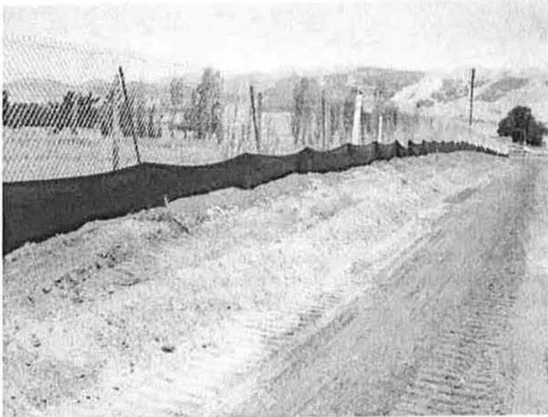
New entrance road and temporarily relocated fence
