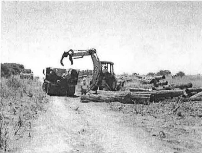
Removing eucalyptus logs and debris from the site
