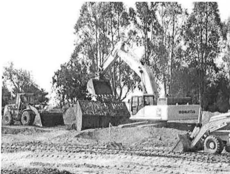
Separating debris from sand with Grizzly
