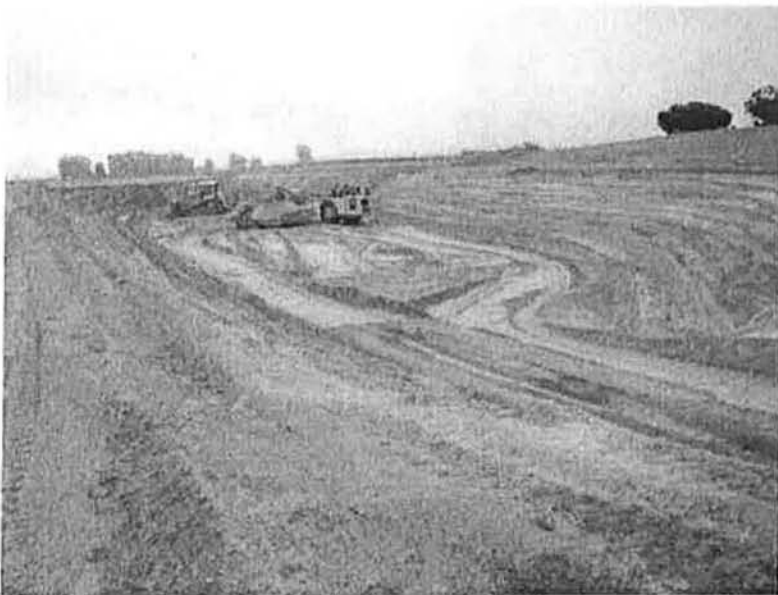
Continued excavation of Clarifiers No 1 & 2
