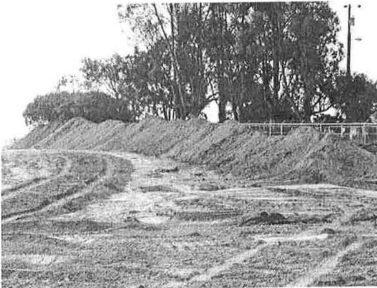
Remaining sand material after buried debris was separated out
