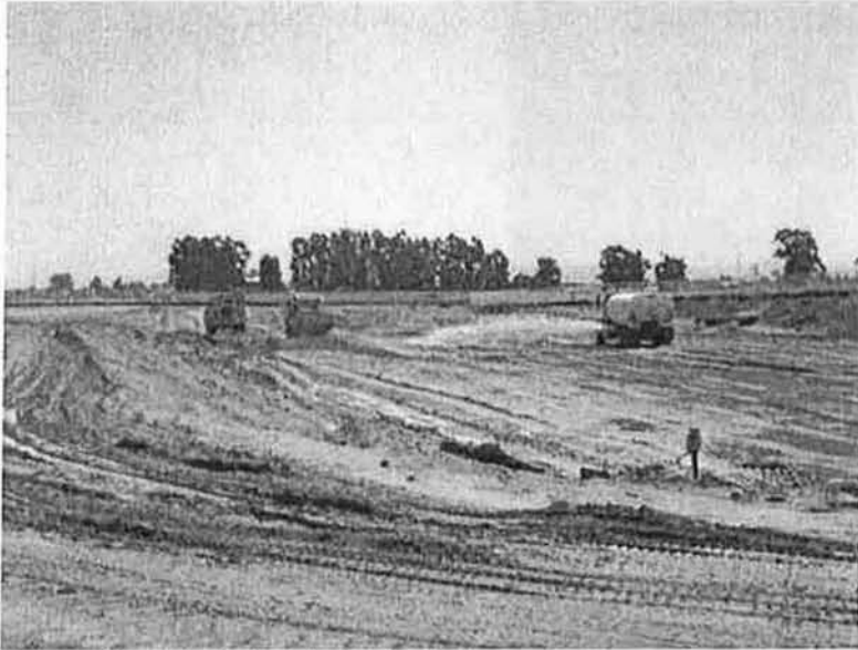
Excavation of sludge drying beds
