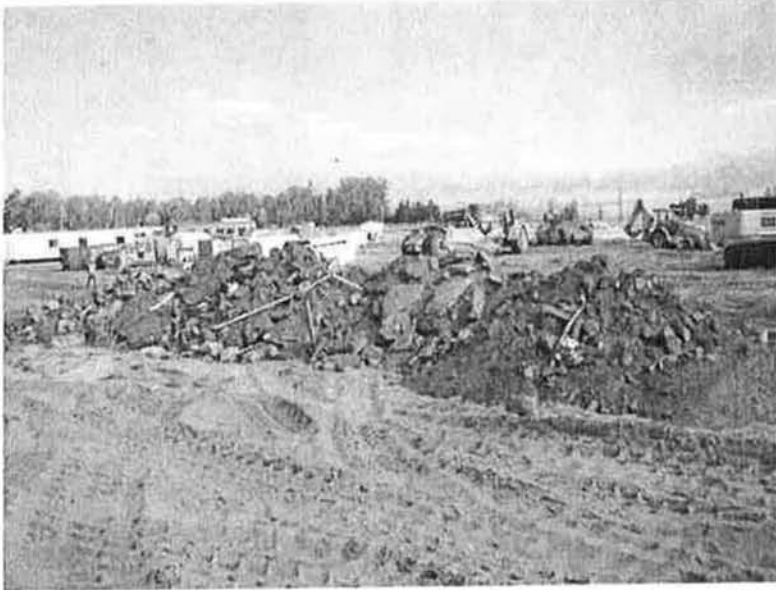
Debris to be hauled from site
