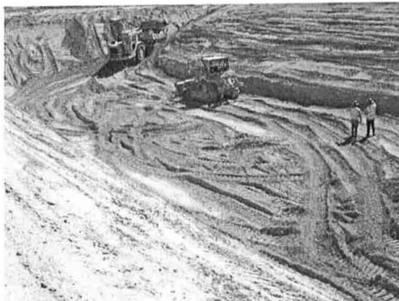
Excavation approximately 75% complete
