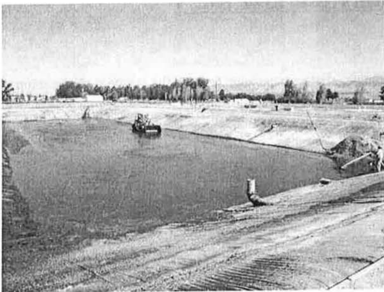
Removing sludge from Pond No. 1
