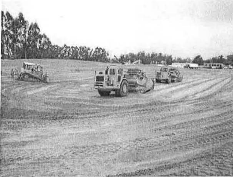
Starting excavation for Clarifiers No. 1 & 2
