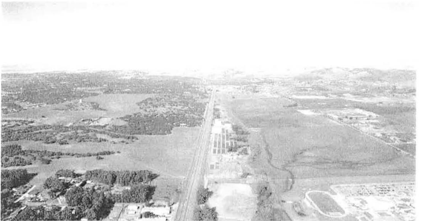
Before Looking North
