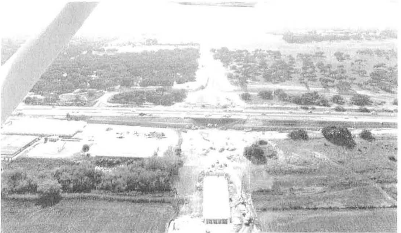
Construction Looking West
