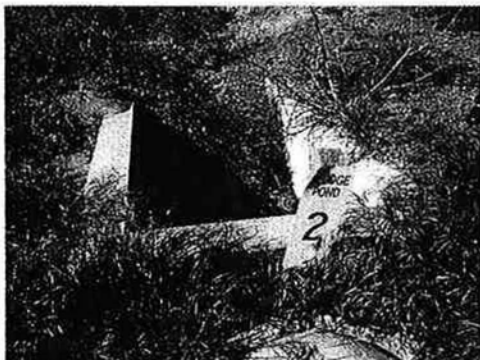
Sludge Drying Bed No. 1 and No. 2: Sludge drying beds are unlined and have no facilities to decant water. Sludge management will be a focus of the Facility Master Plan (optional task).
