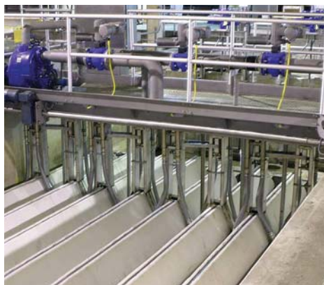
AquaDiamond® backwash assembly and laterals.
