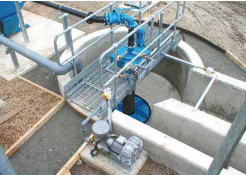
The completed Jetair installation.
