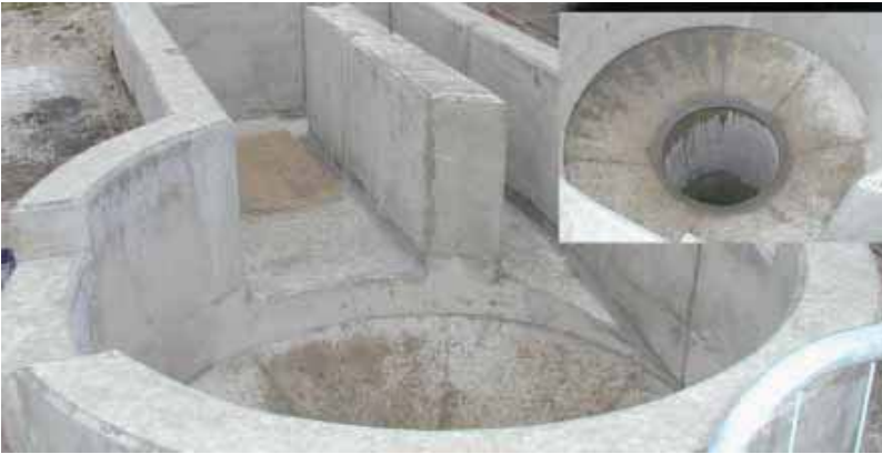
Civil construction and installation.
