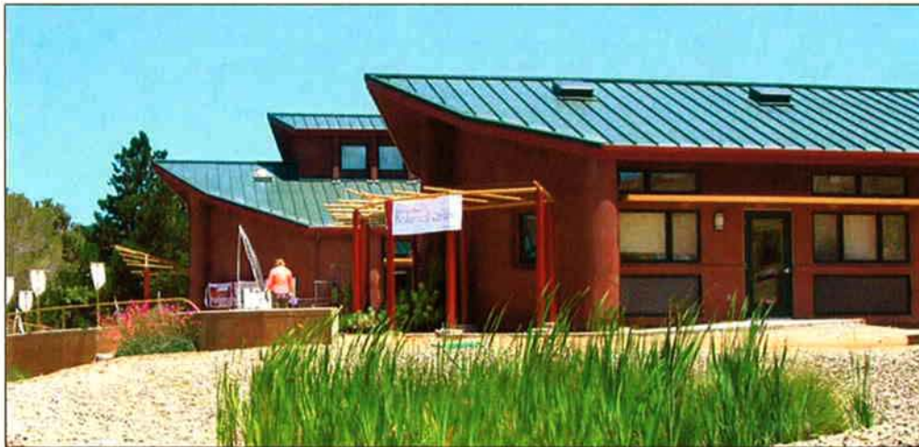
SLO Botanic Garden building uses a constructed wetland water reclamation system creating riparian habitat page, 21-22.
