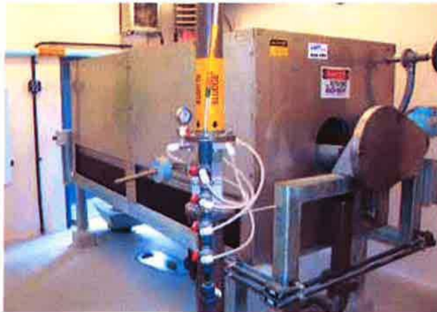
Figure 3 Rotary Drum Thickener (BDP)
