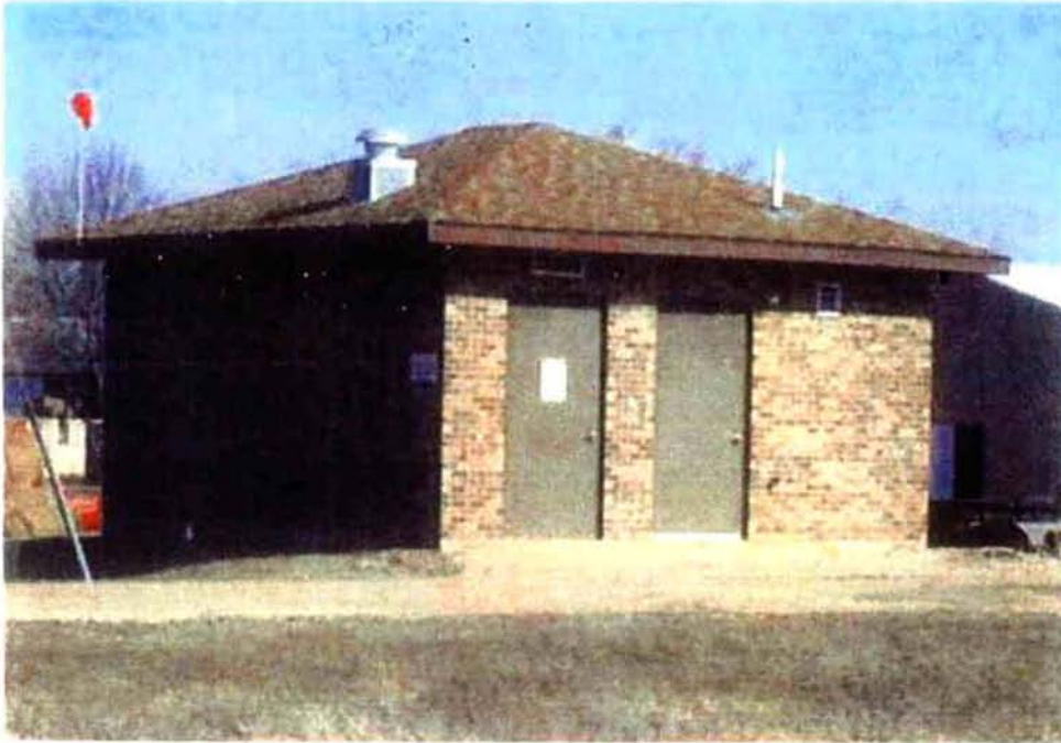
FIGURE 14 Typical Booster Station
