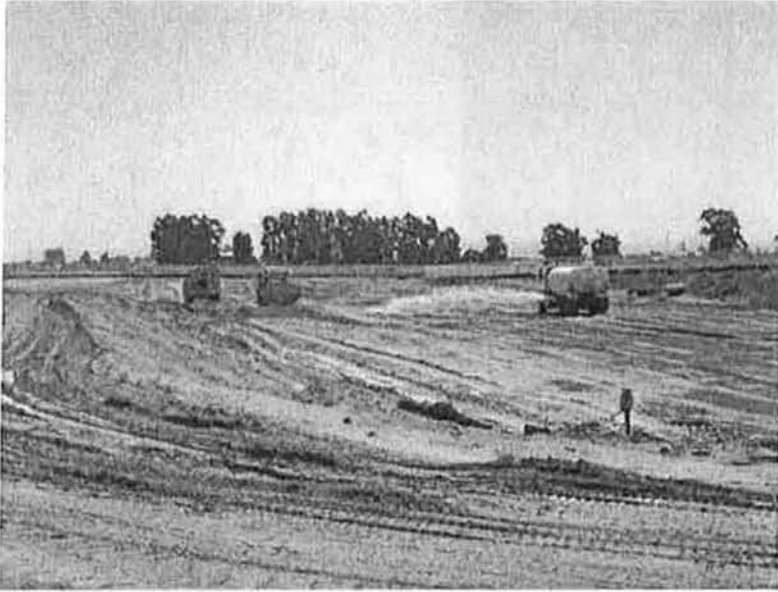
Excavation of sludge drying beds
