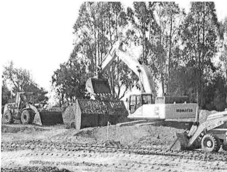
Separating debris from sand with Grizzly
