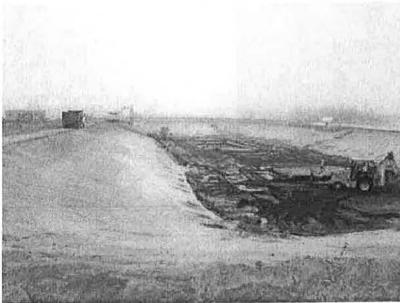
Liner removed and continued removal of sludge from Pond No. 1
