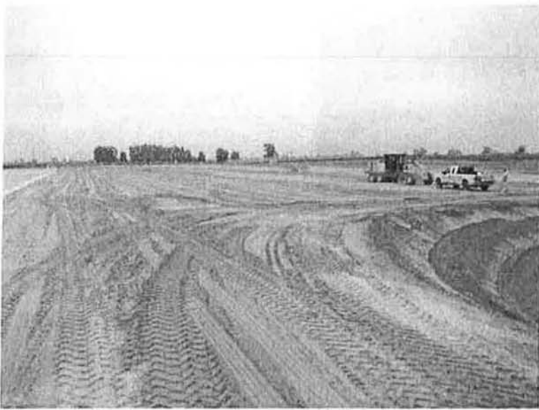
Sludge drying bed subgrade compacted and ready for aggregate base
