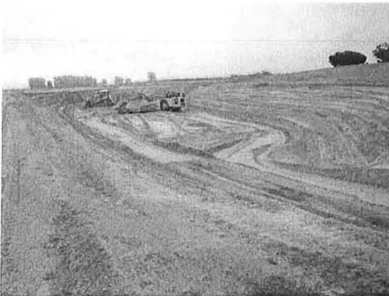
Continued excavation of Clarifiers No 1 & 2
