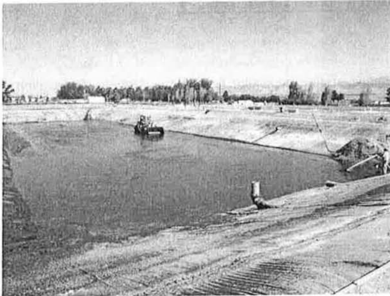
Removing sludge from Pond No. 1
