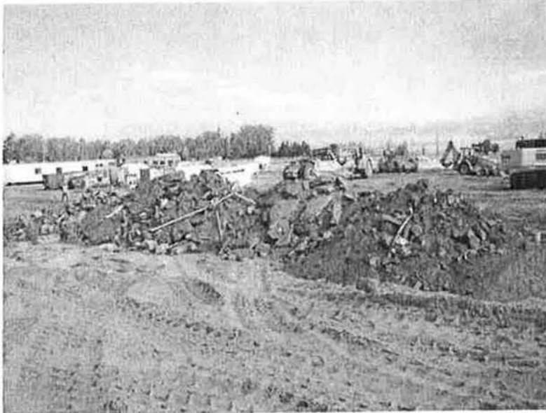
Debris to be hauled from site
