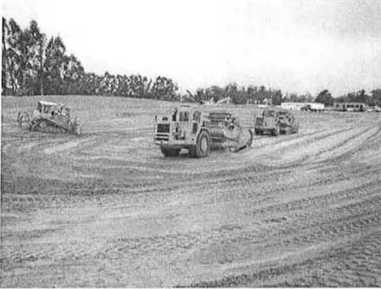
Starting excavation for Clarifiers No. 1 & 2
