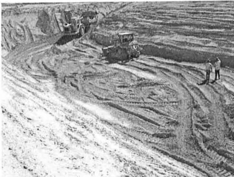
Excavation approximately 75% complete
