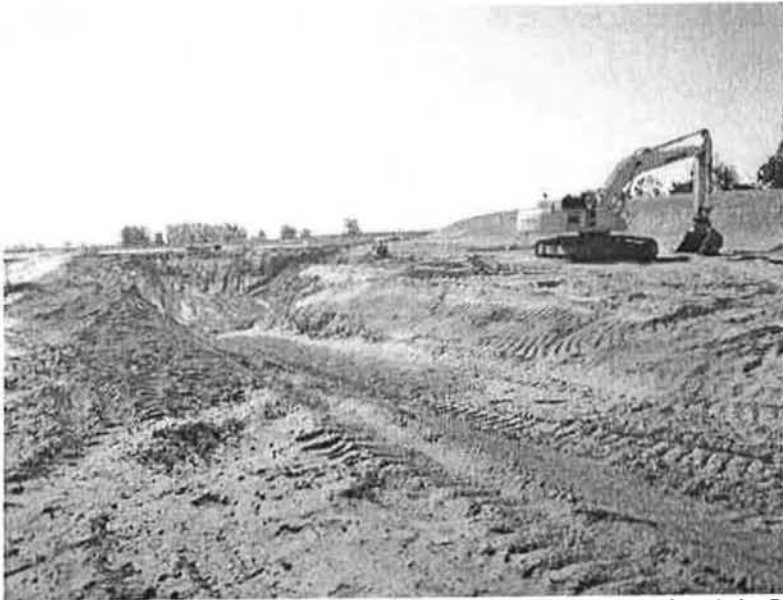
Continued excavation for Clarifiers No. 1 & 2, approximately 65% complete
