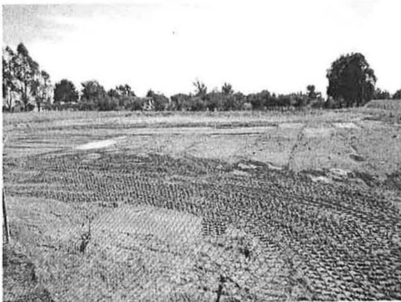
Prepping staging area for trailers, parking and equipment
