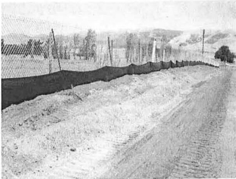
New entrance road and temporarily relocated fence
