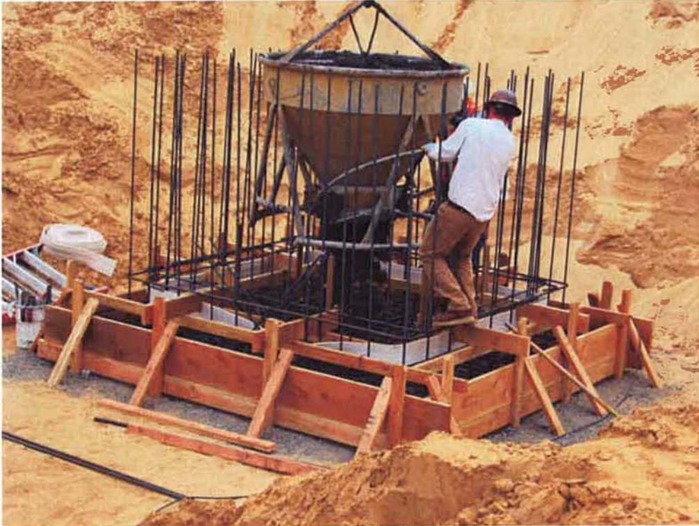
Pouring slab and foundation for the RAS/WAS pump station.
