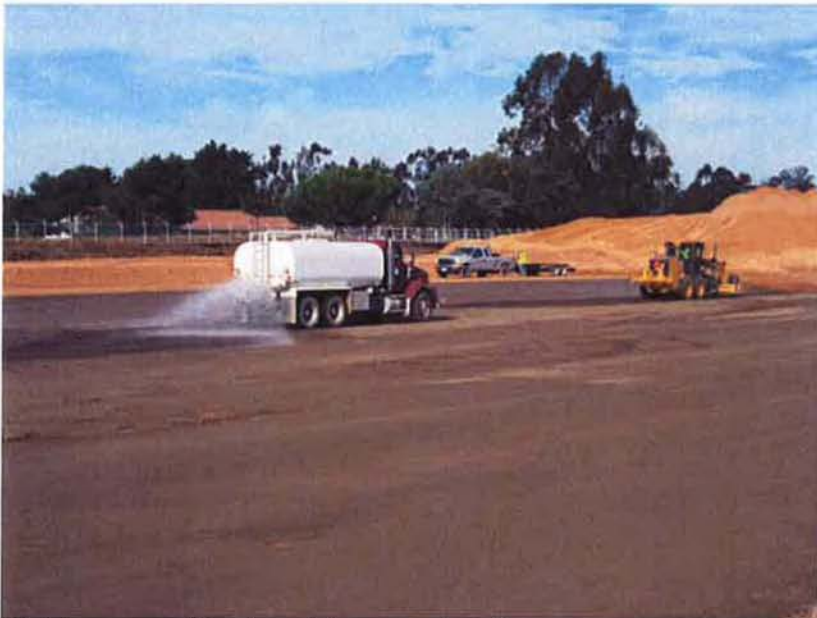
Moisture conditioning of base material.
