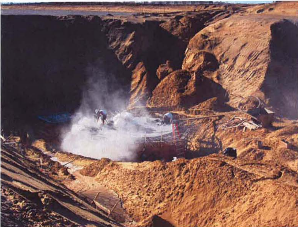
Stripping forms at Clarifier #1 center base structure.
