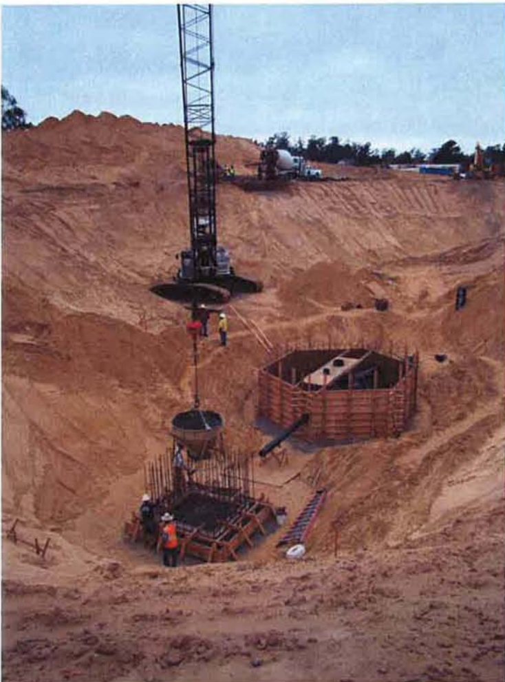
First concrete pour for Clarifier #1 and the RAS/WAS pump station.
