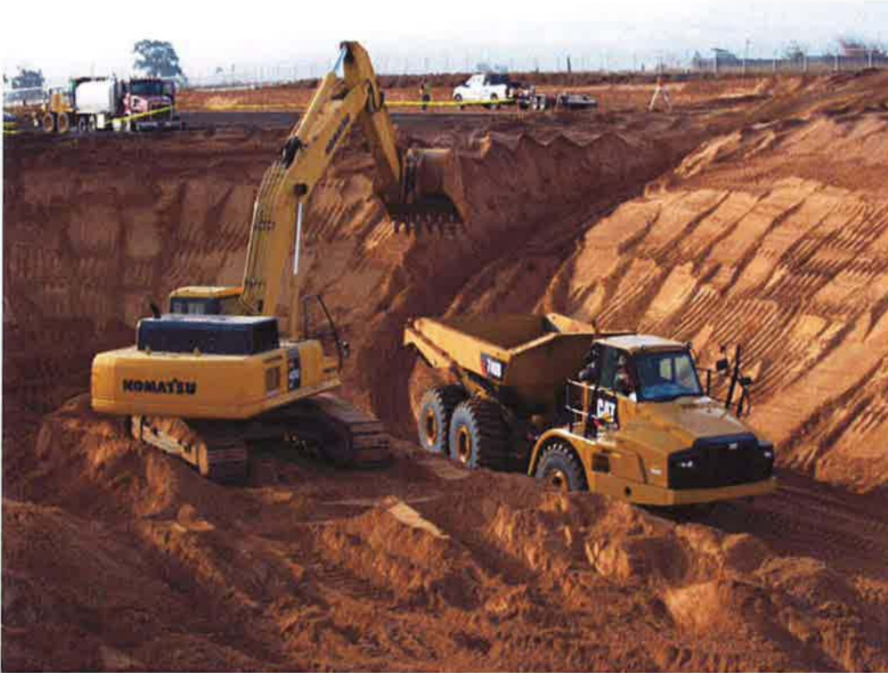
Completing clarifier excavation.
