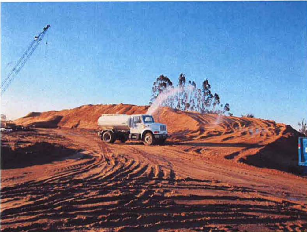
Dust control on stockpile.
