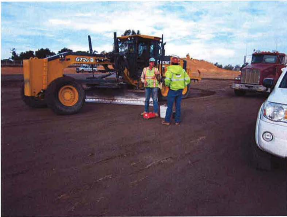
Checking compaction of base material at sludge drying beds.
