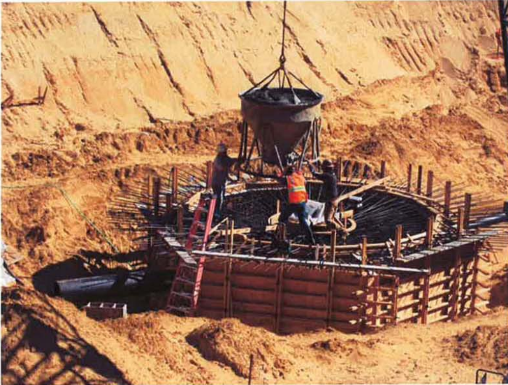
Second concrete pour at Clarifier #1 center base structure.
