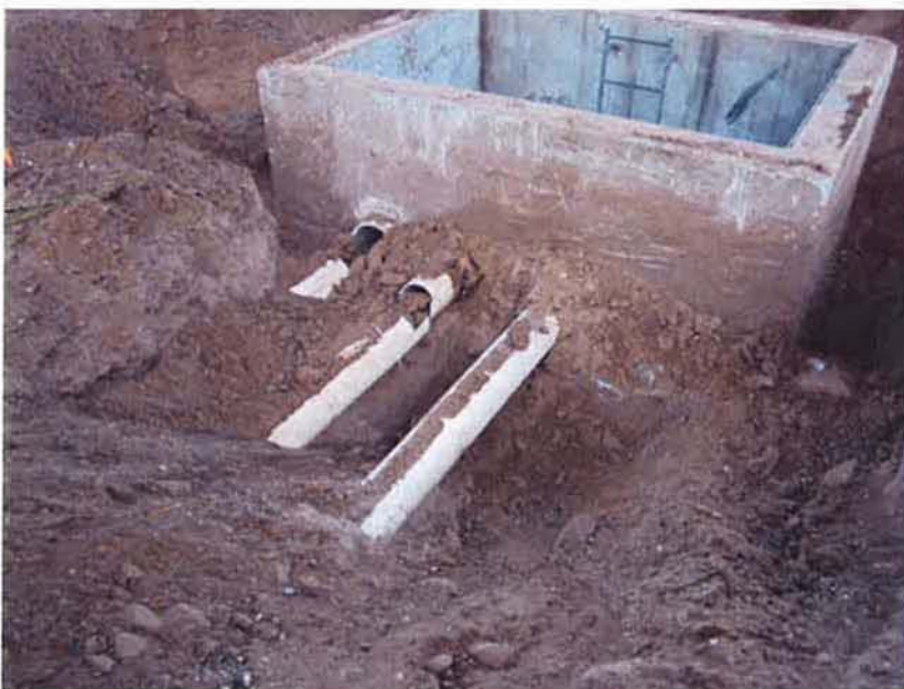
Demo of 8" influent piping and distribution vault.
