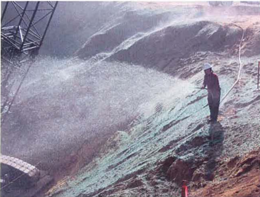
Applying mulch erosion control to slopes around clarifier excavation.
