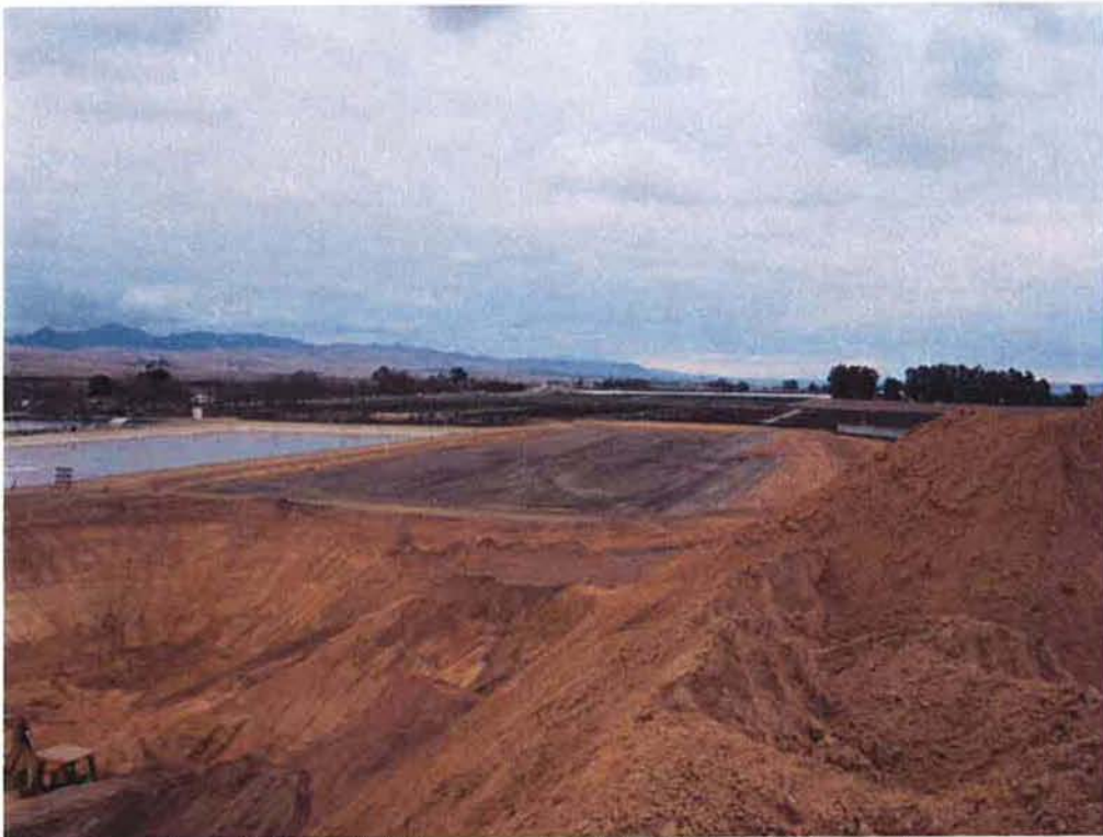
Completed installation of 4" base material in sludge drying beds.
