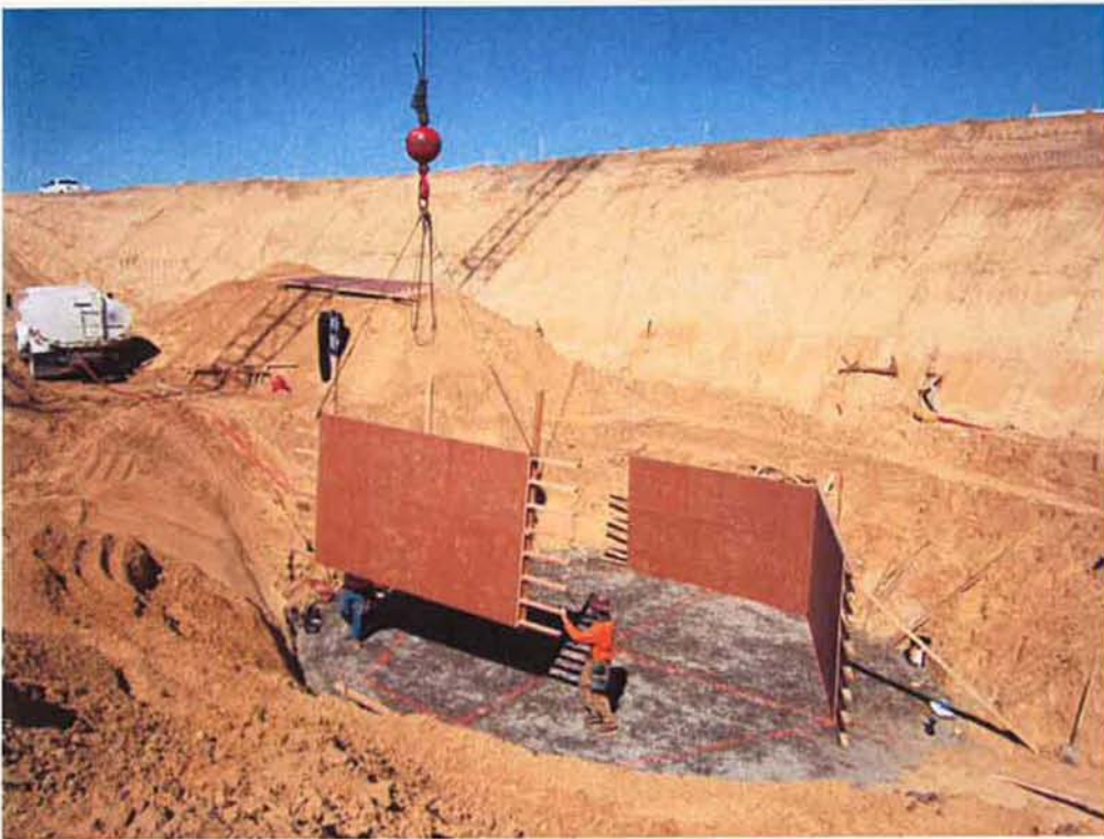
Setting forms for Clarifier #1 center sump structure.
