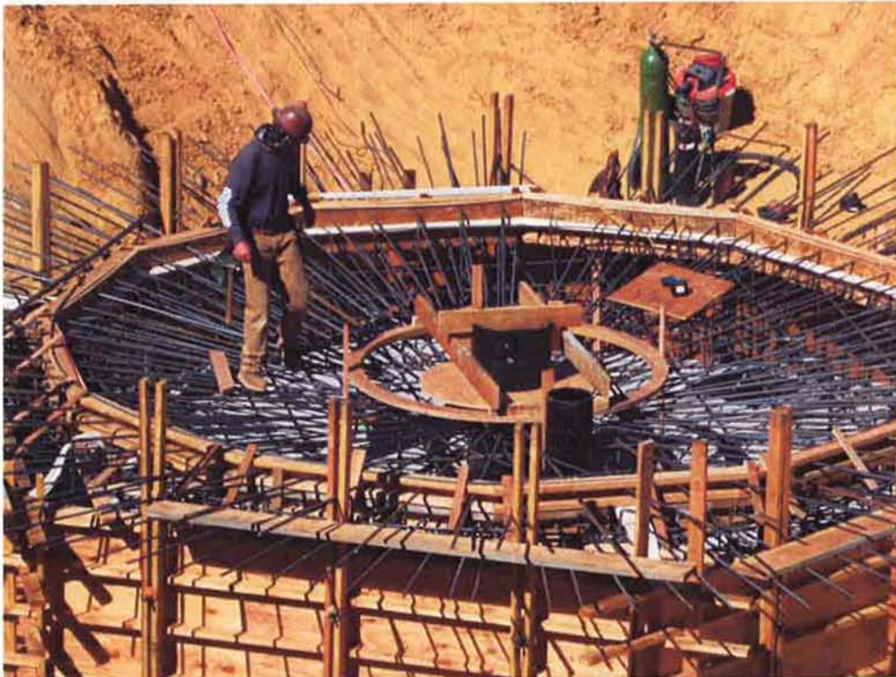
Installing second layer of rebar for Clarifier #1 center structure.
