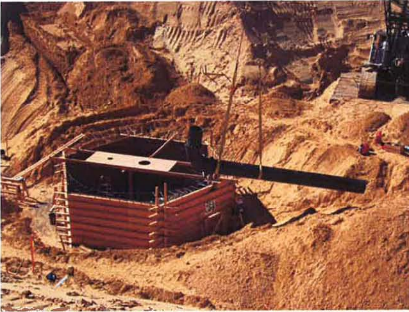
Using crane to install under structure piping 18" ML
