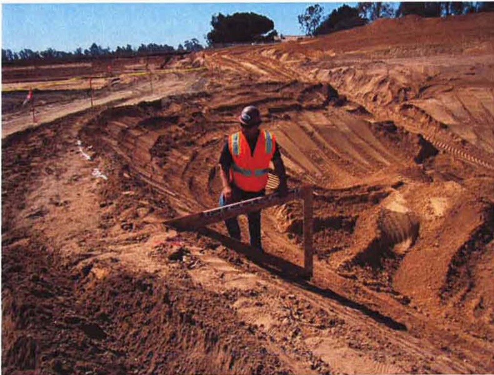
Checking slope of clarifier excavation.
