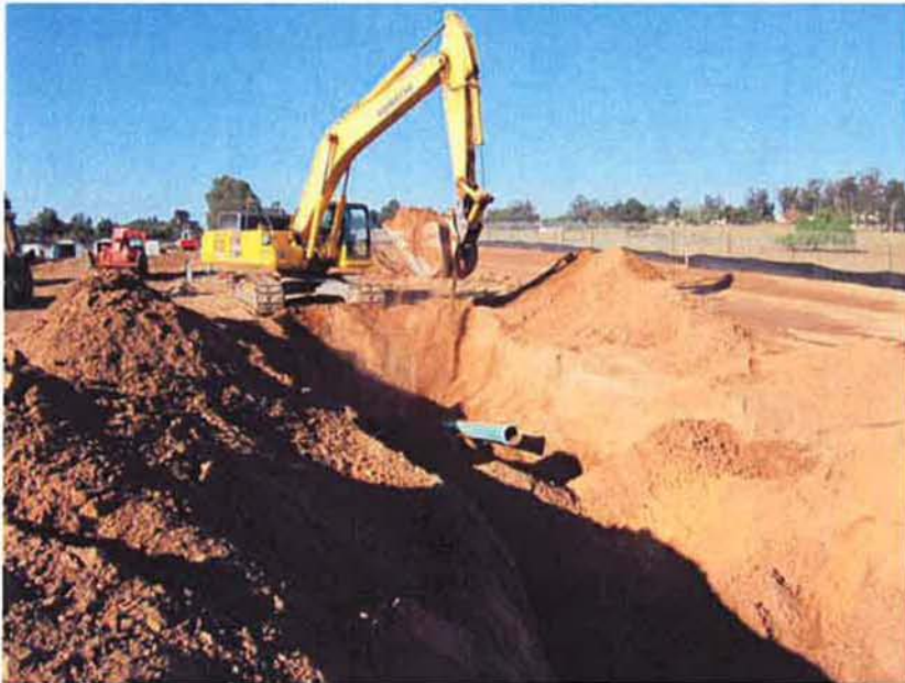
Demo of existing 10" Influent piping.
