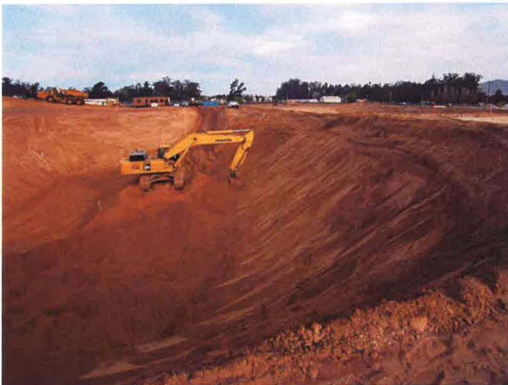
Widening and cutting slope of open cut excavation.
