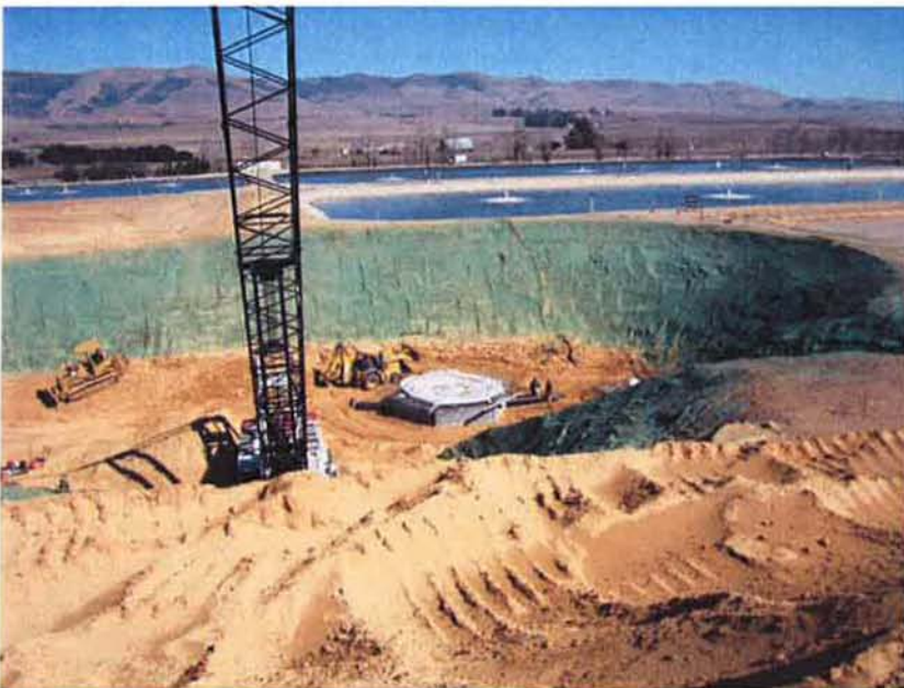
Mulch erosion control on clarifier excavation slopes.
