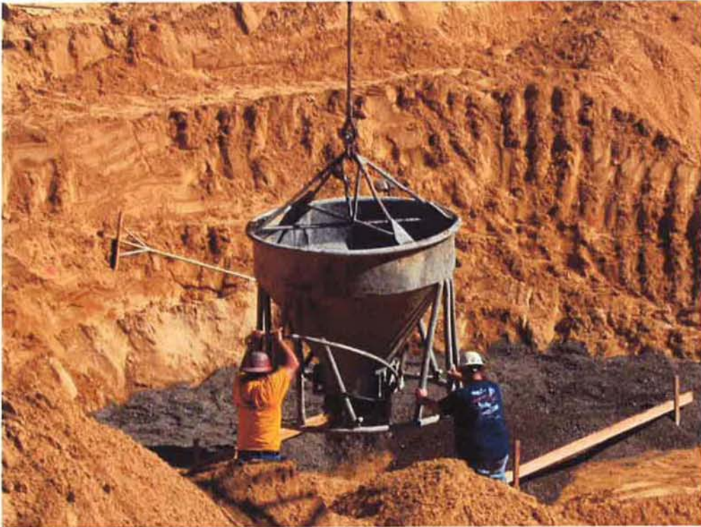
Placing base material with crane for Clarifier #1
