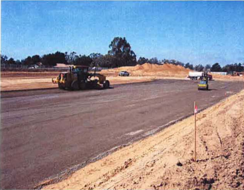
Placing, grading and compacting 4" recycled base material at sludge drying beds.
