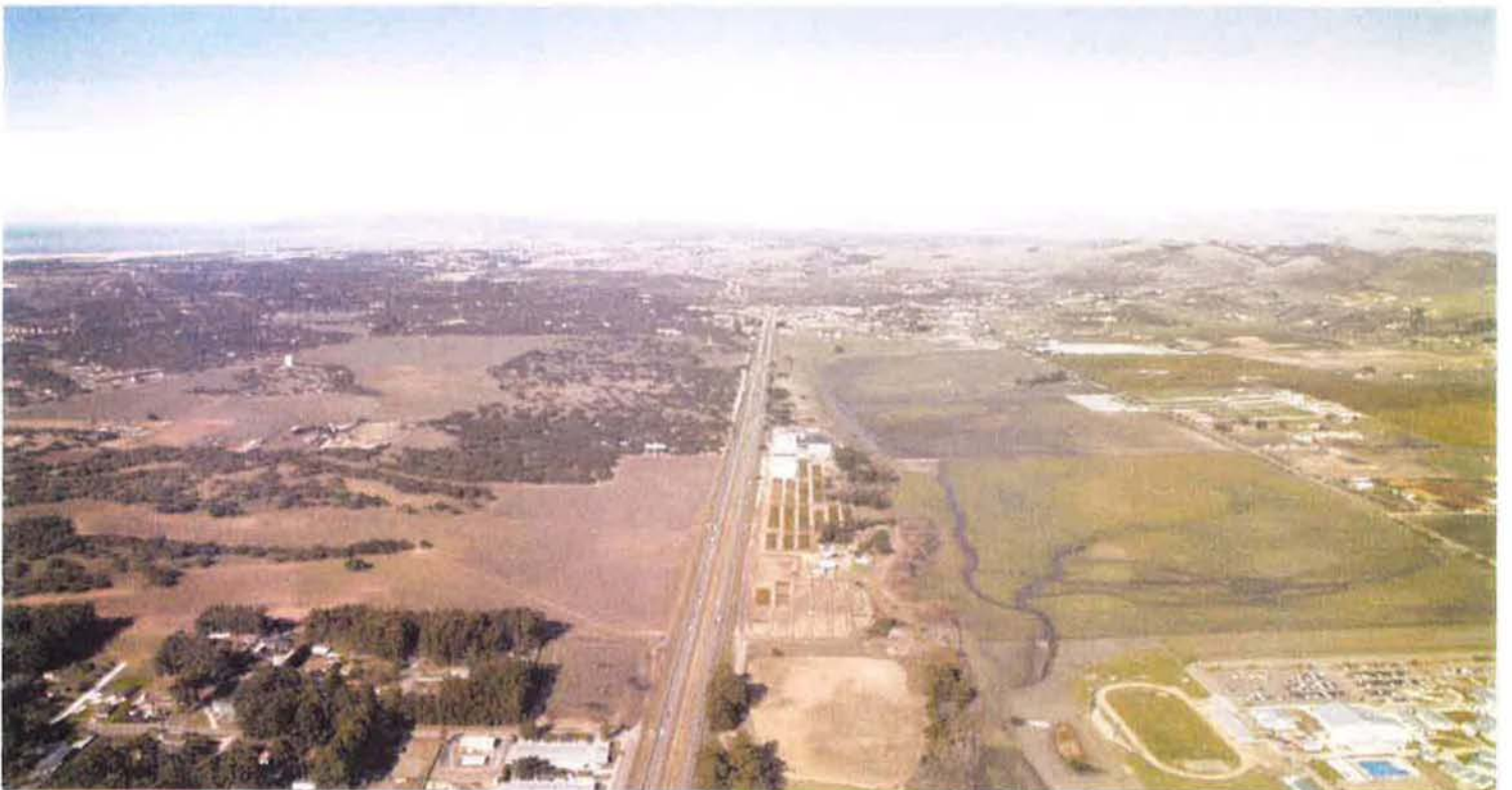
Before Looking North
