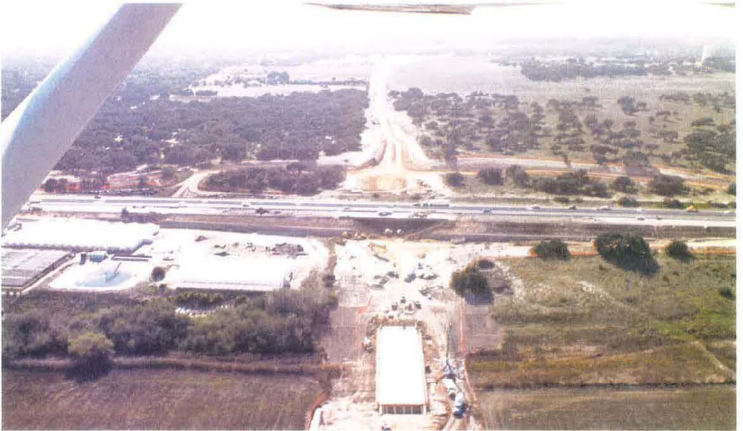
Construction Looking West
