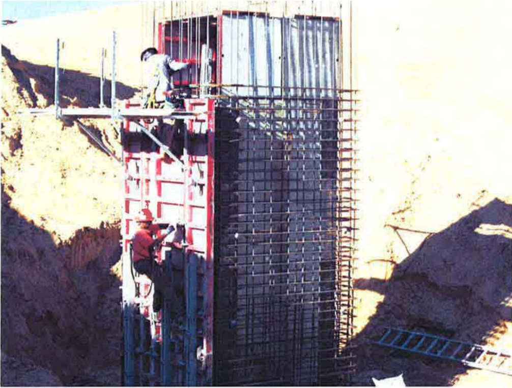
Installing forms on RAS/WAS pump station walls.
