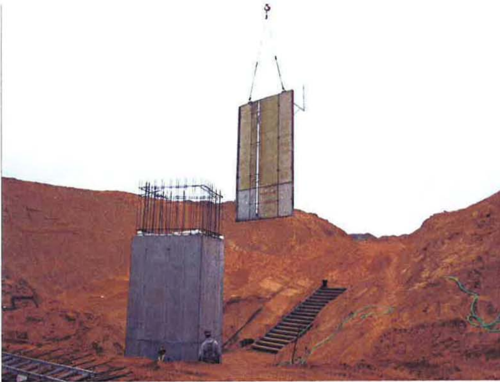
Stripping forms from RAS/WAS Pump Station #2.
