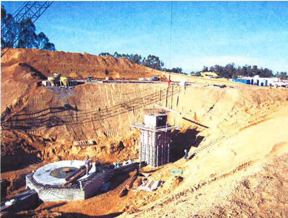
Finalizing forms on RAS/WAS Pump Station #2 walls.
