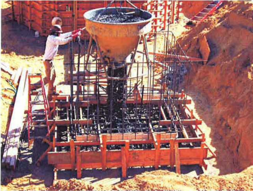
Placing concrete at RAS/WAS Pump Station # 2 foundation.
