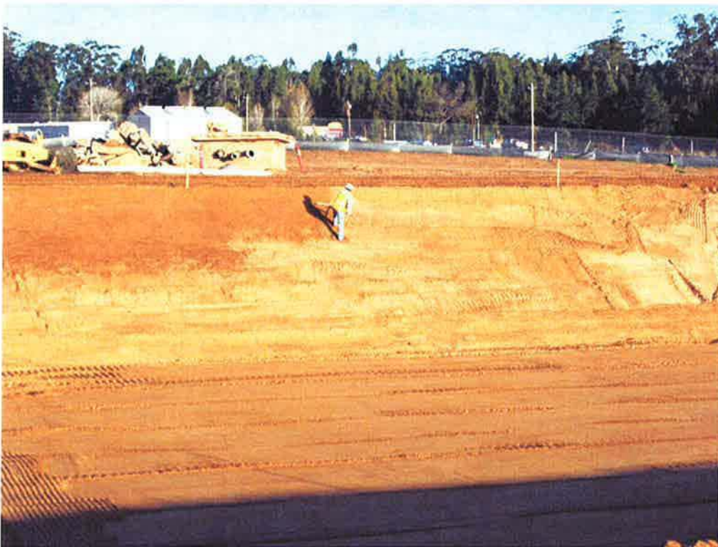
Finish grading by hand at Aeration Basin #1.
