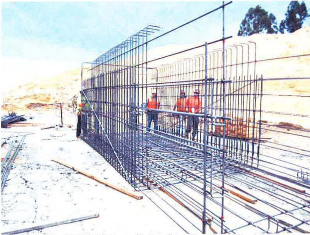
Tying rebar for RAS/WAS Pump Station #2 walls before lifting into place.
