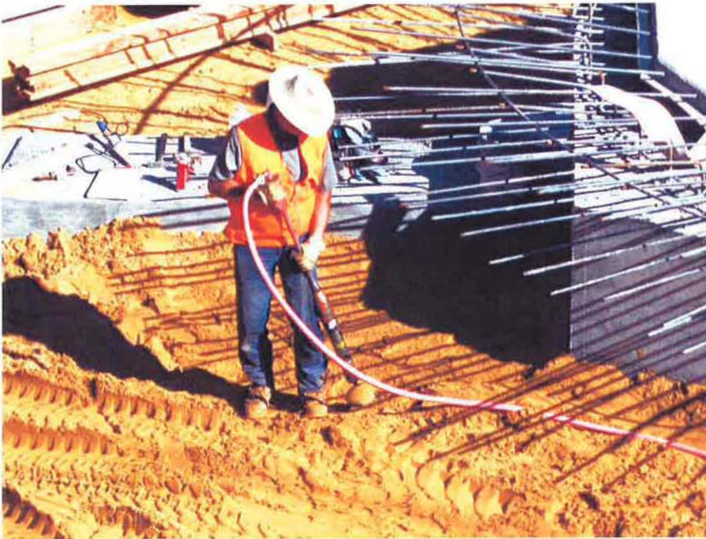
Compacting around Clarifier #2 center base with a "powder puff".
