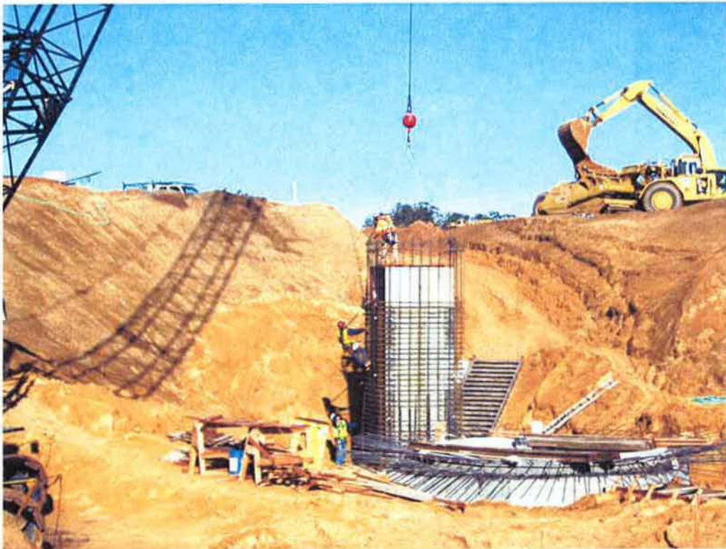
Installing reinforcing for RAS/WAS Pump Station #2.
