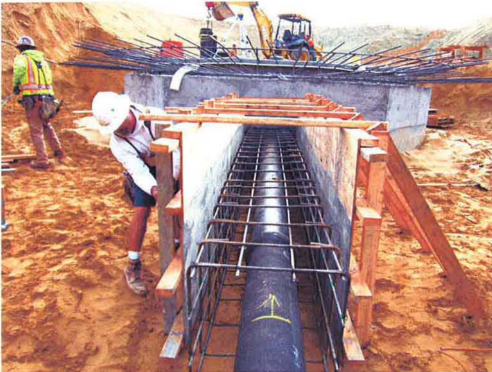
Installed reinforcing and forming pipe encasement.
