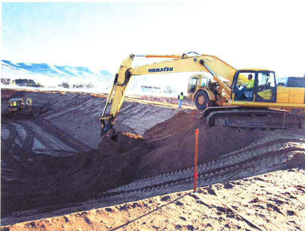
Completing grading at separation embankment (from Aeration Basin side).
