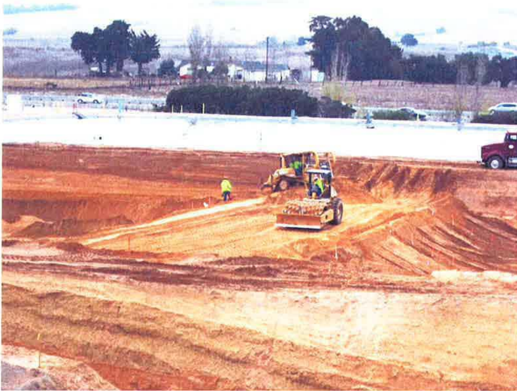
Grading and compacting separation embankment.
