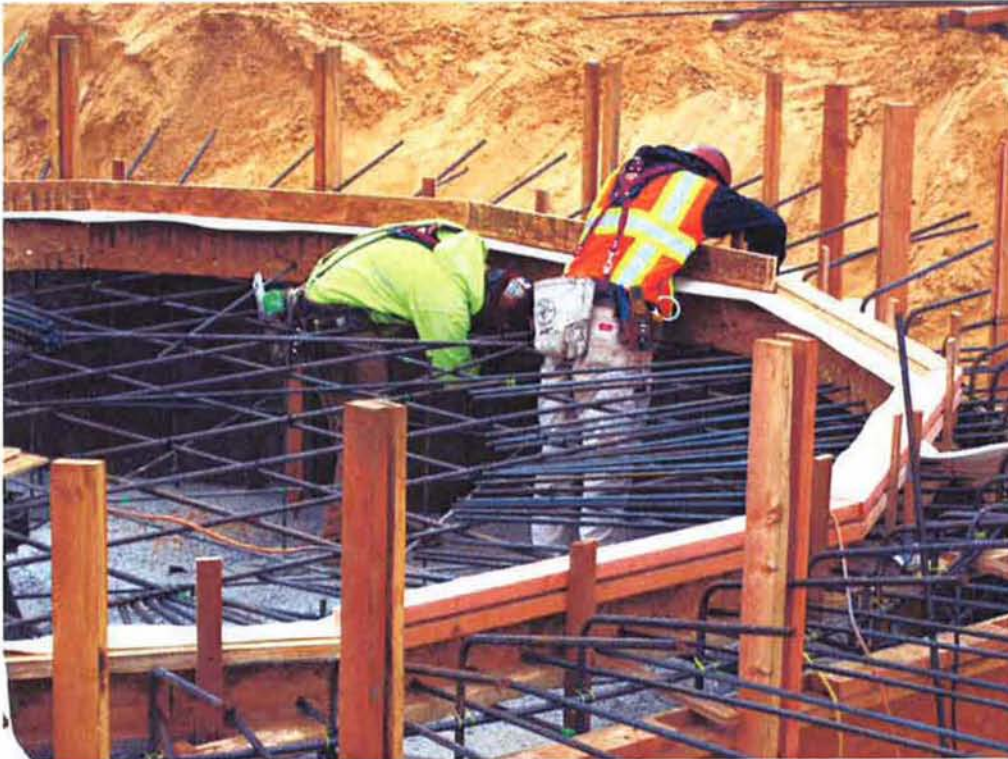
Forming construction joint with waterstop at Clarifier #2.
