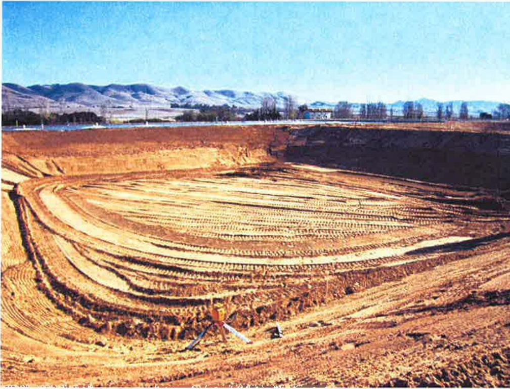
Grading almost completed on Aeration Basin #1.
