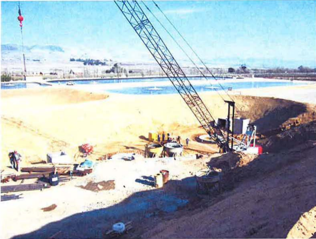
Overview of clarifier excavation.
