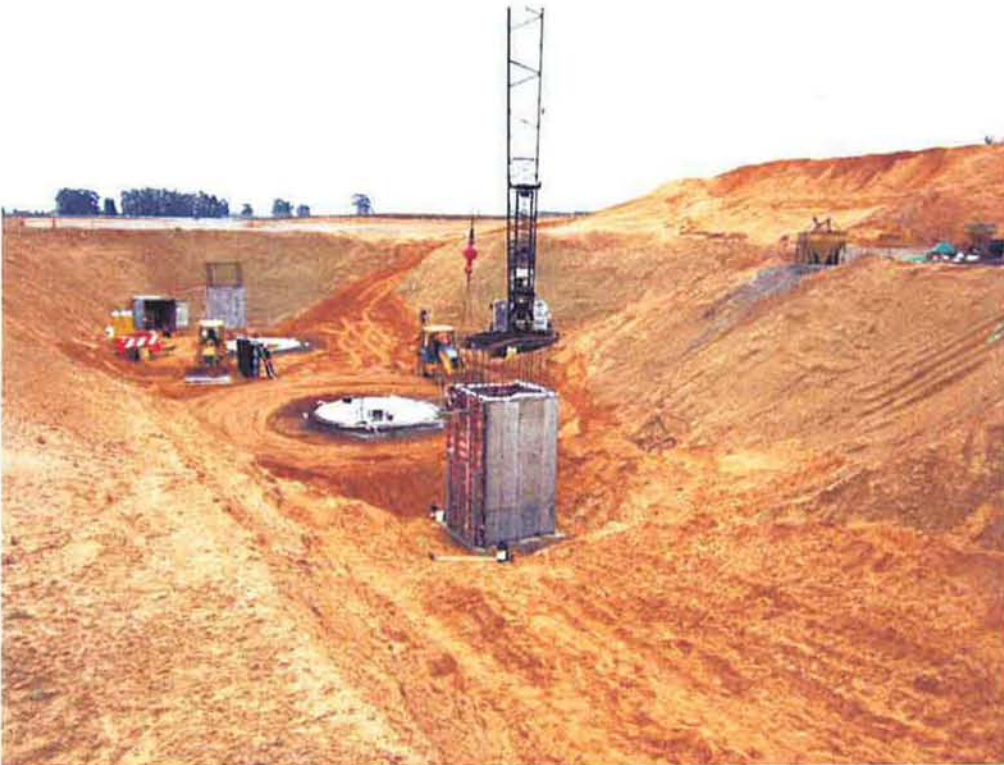
Stripping wall forms from RAS/WAS Pump Station #2.
