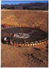
Construction of Southland Wastewater Treatment Facility
