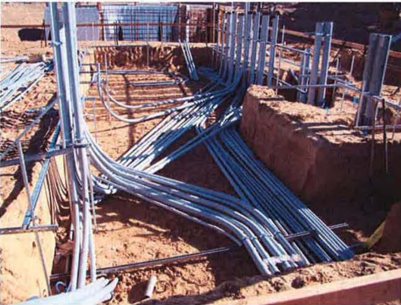
Conduit being installed under foundation of Electrical/Blower Building.
