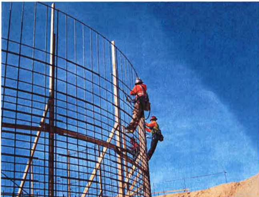
CMC Steel finishing rebar for clarifier walls.
