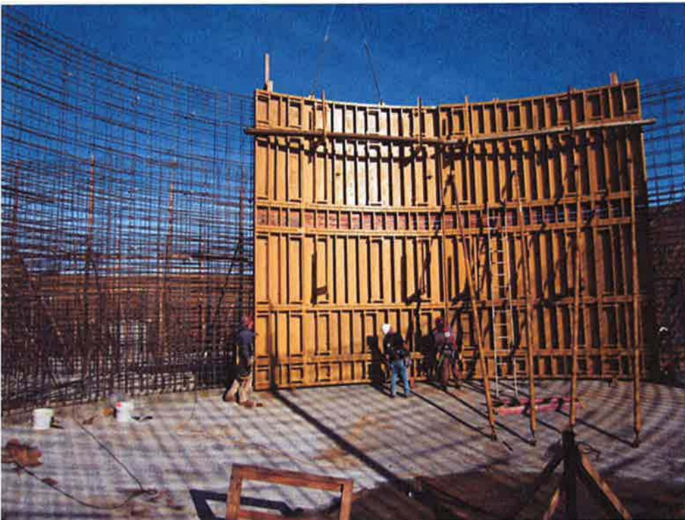
Cushman positioning and bracing inside wall forms at Clarifier #1.
