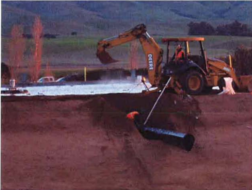
Installing 18" SI pipe at Aeration Basin.
