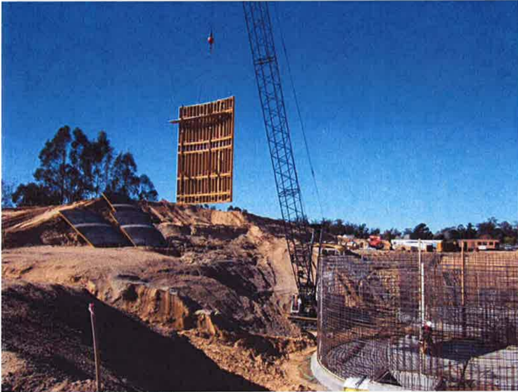
Swinging outside form into place.
