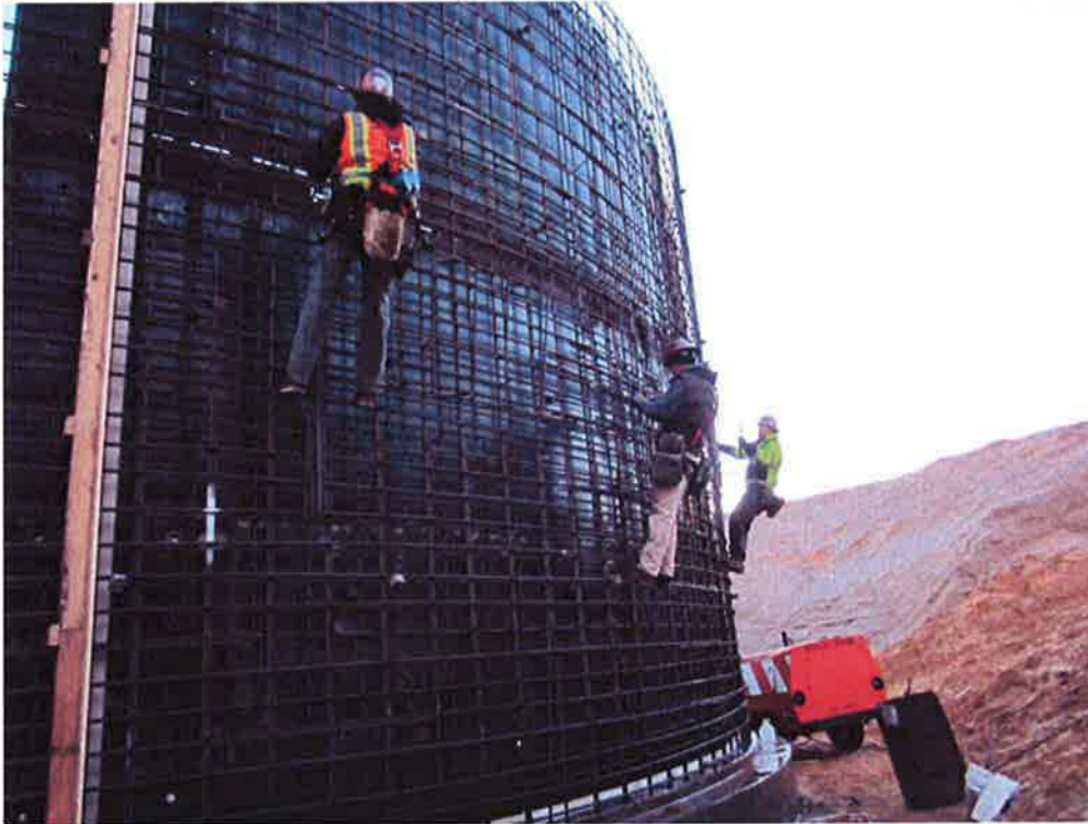
Finalizing rebar and clearances with inside form in place at Clarifier #1.
