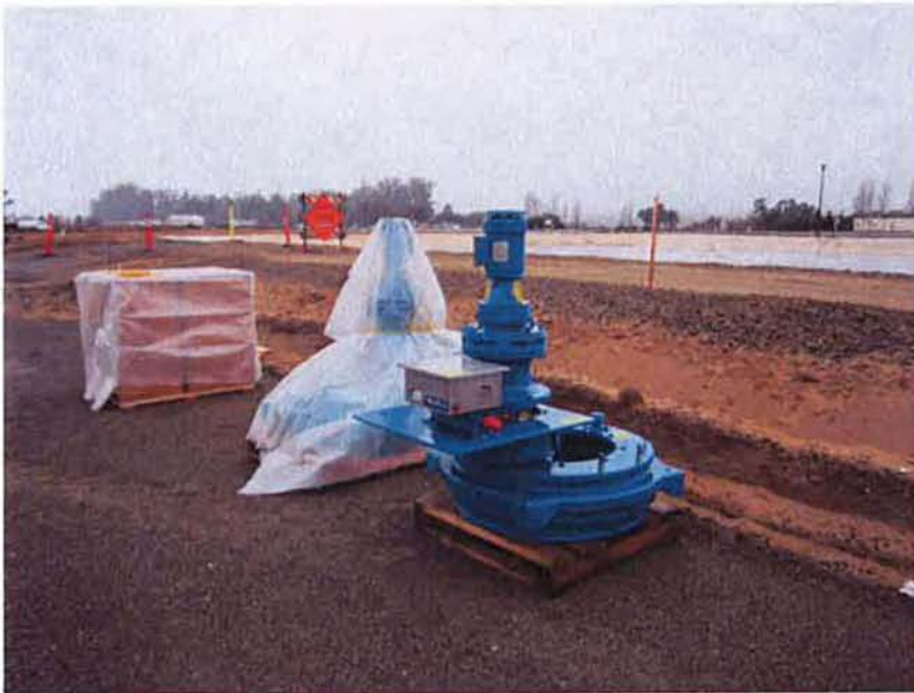
Motors for clarifier mechanisms delivered to site.
