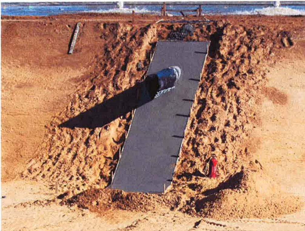
Pour of splash pad completed in Aeration Basin.
