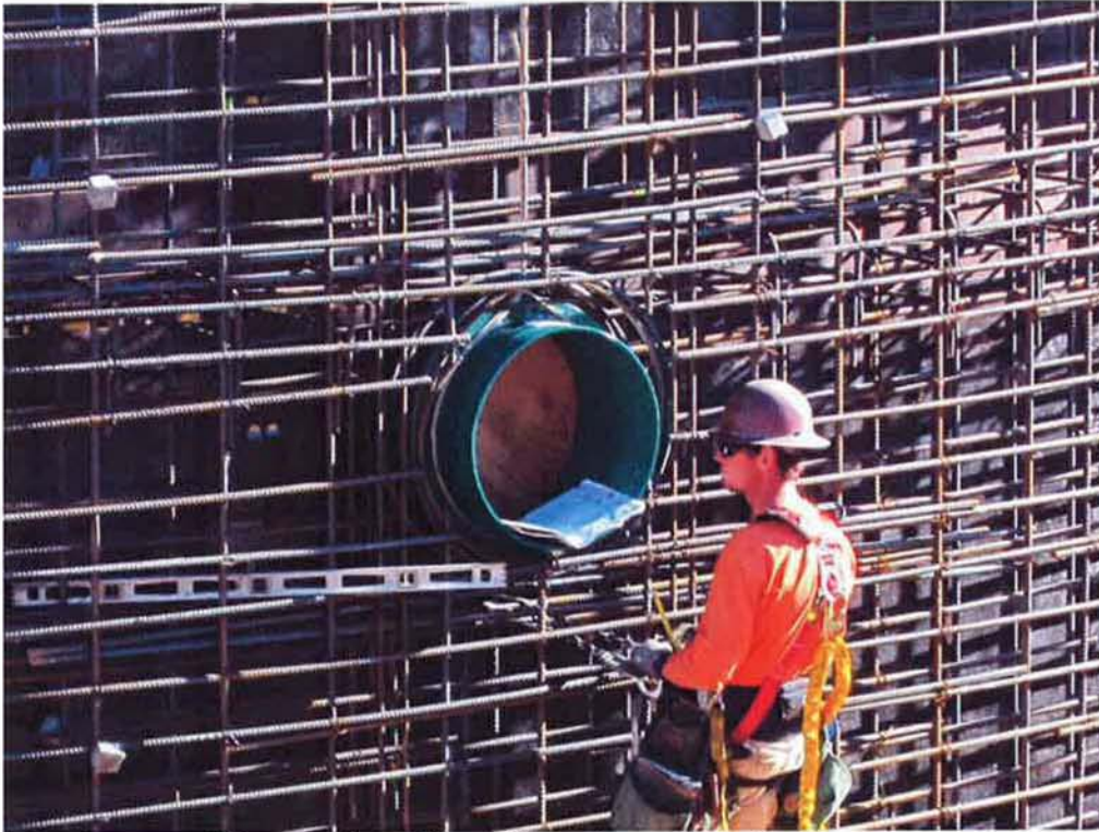
Installing spool for a wall section with a pipe penetration.
