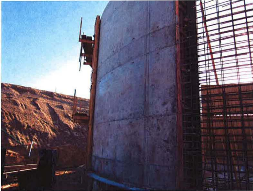
First section of outside wall form removed on Clarifier #1.
