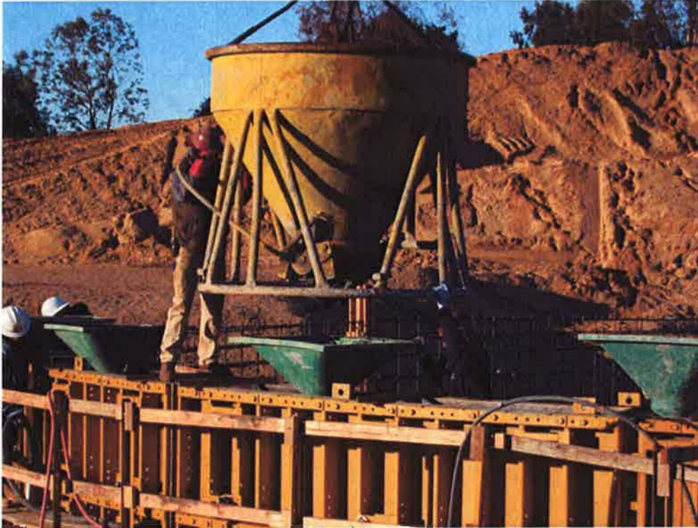
Pouring concrete in a wall section using the funnels and tremmies.
