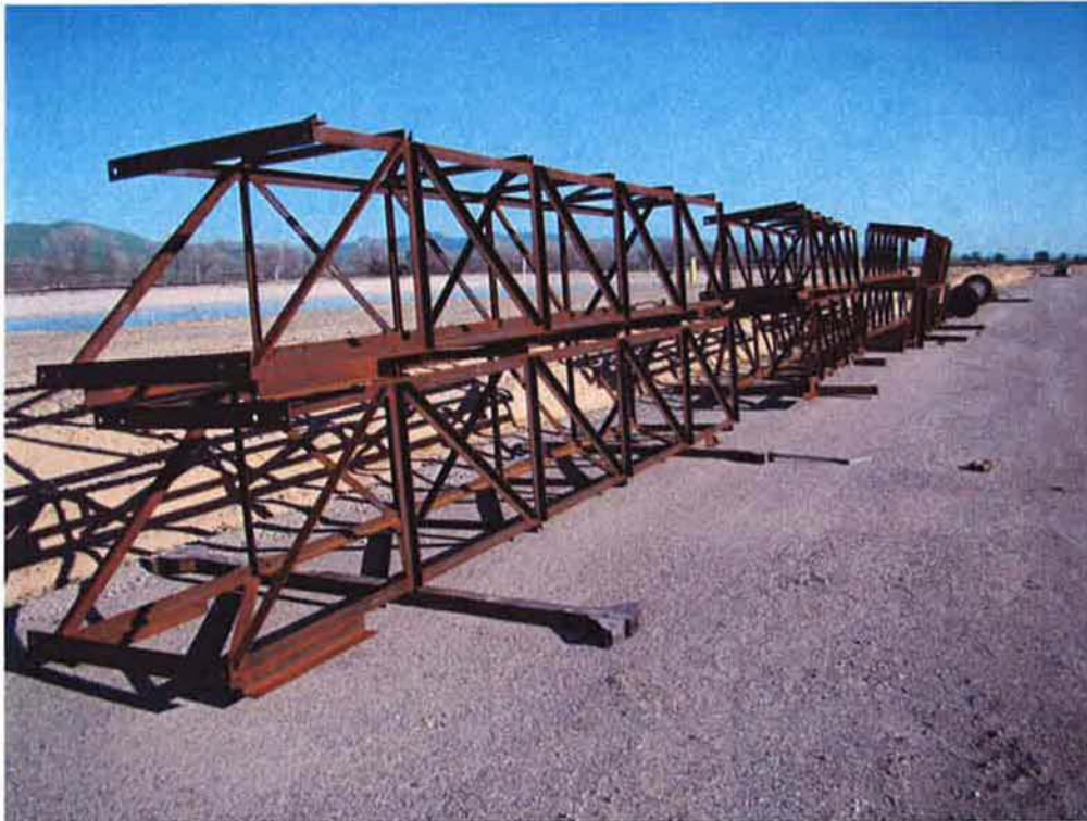
Clarifier mechanism delivered to site.
