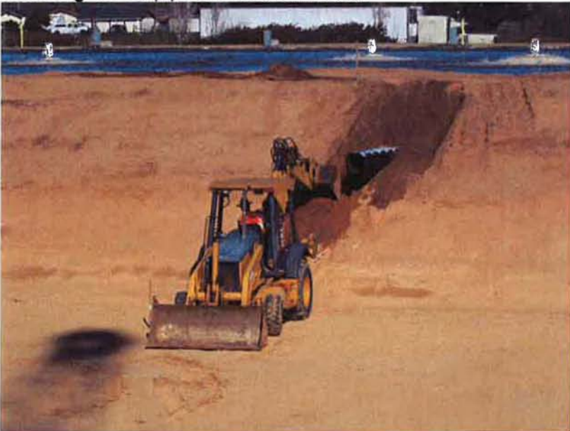
Excavating for 18" SI pipe splash pad in Aeration Basin.
