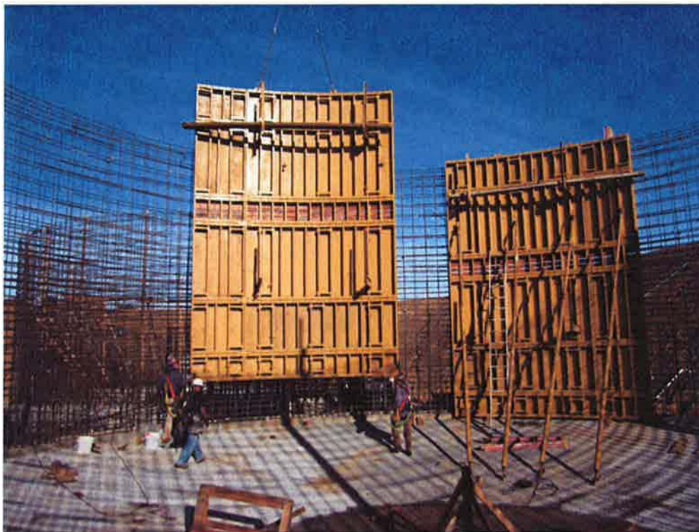
Installing and supporting inside wall form at Clarifier #1.
