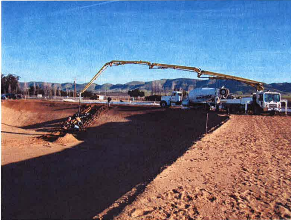
Pouring influent pipe splash pad in the Aeration Basin.
