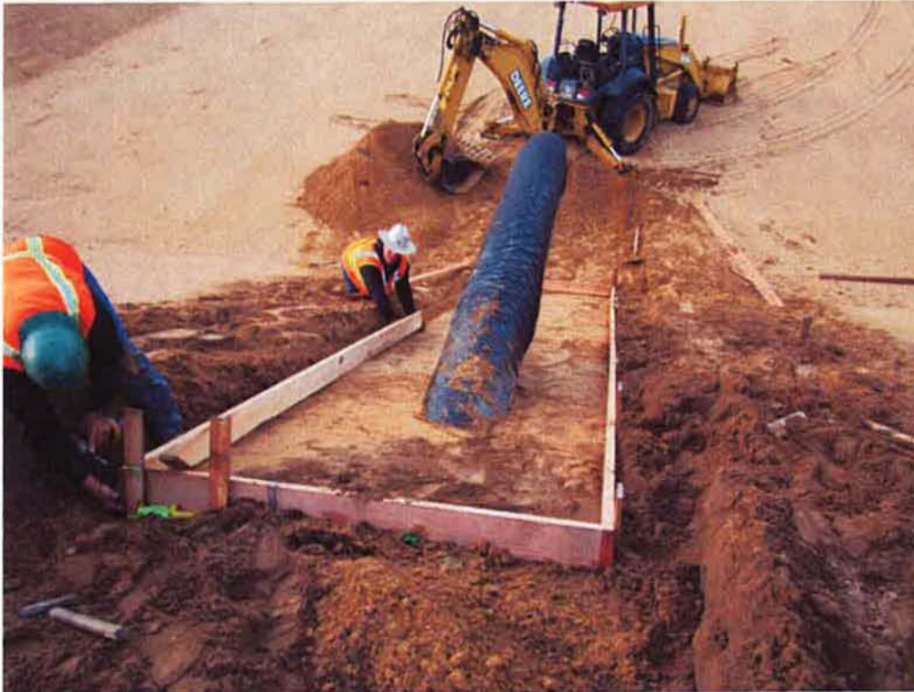
Setting forms for splash pad in Aeration Basin.
