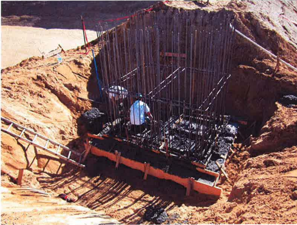
Pouring foundation for effluent weir box for Emergency Basin.
