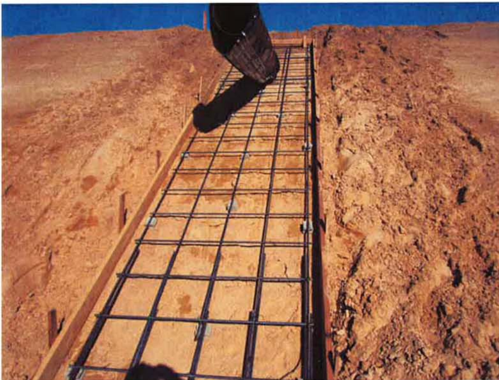
Installing rebar at splash pad in Aeration Basin.
