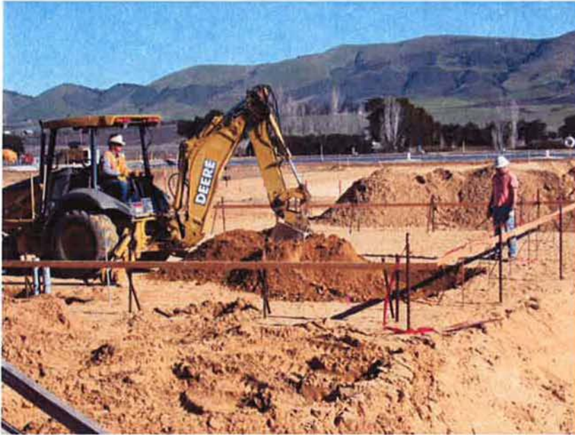
Excavating electrical duct banks in layout for new Electrical/Blower Building.
