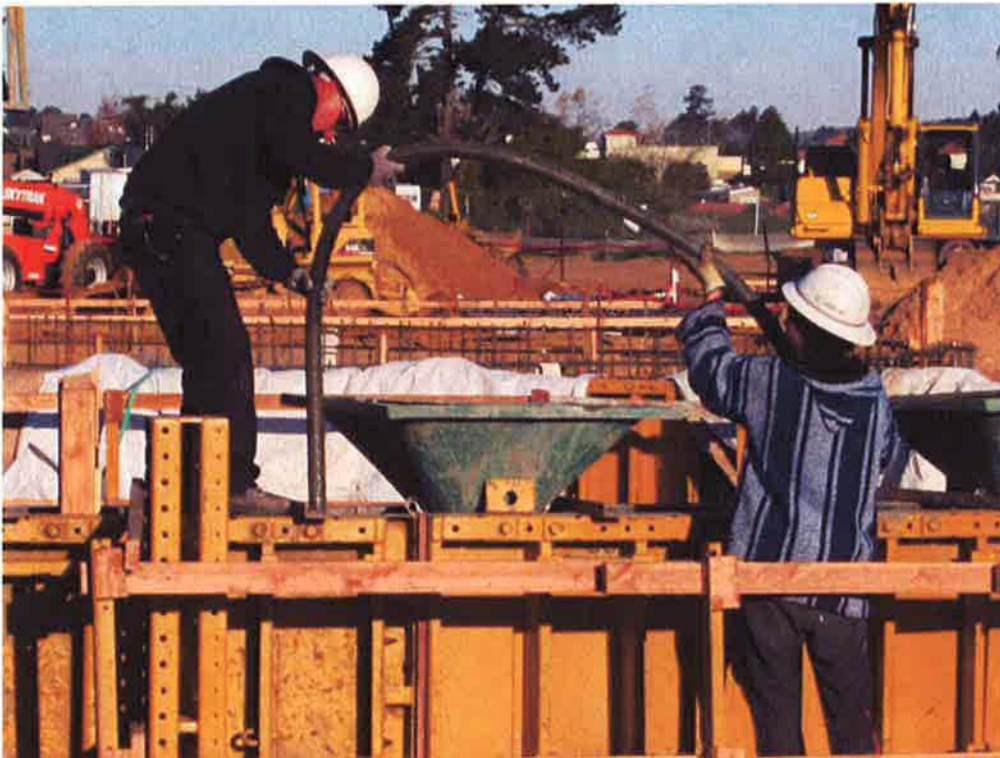
Vibrating the concrete during a wall pour.
