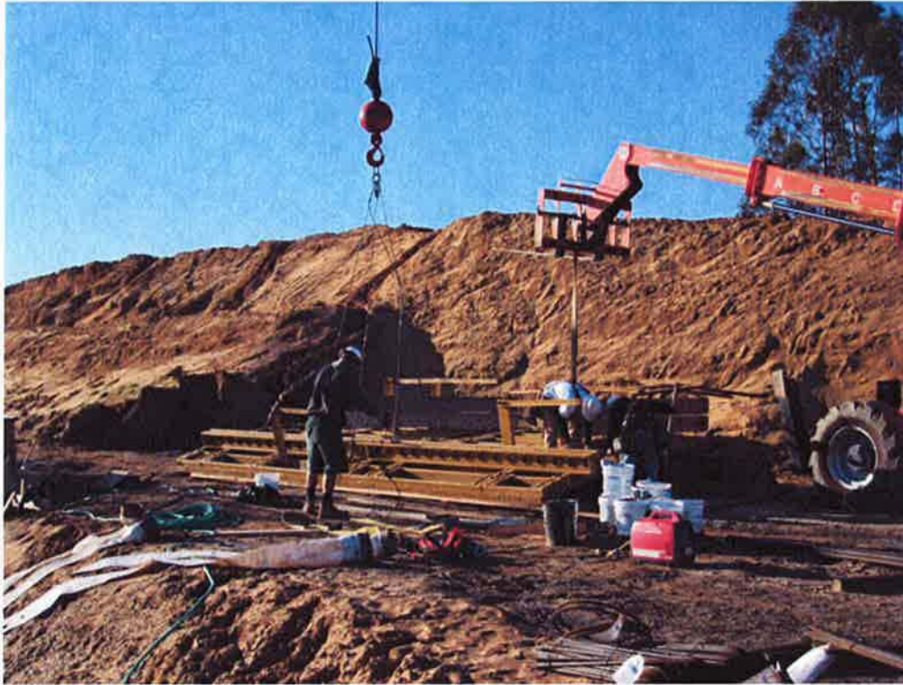
Cushman assembling wall forms and preparing to lift into place.
