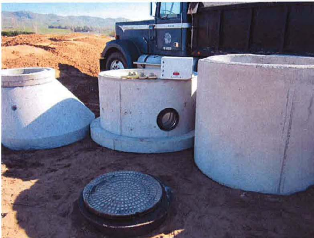
Manholes delivered to site.
