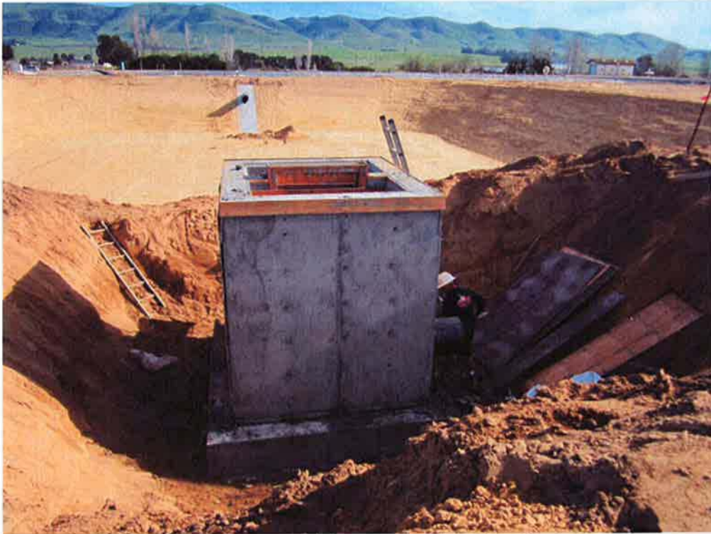
Removing forms from effluent weir box at the Aeration Basin.
