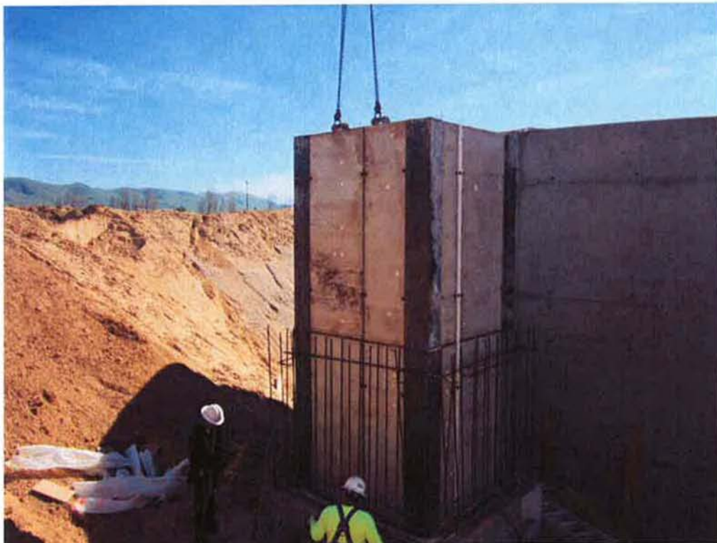
Setting inside forms for RAS/WAS Pump Station #2.
