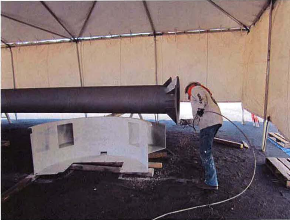
Applying primer to clarifier mechanisms.
