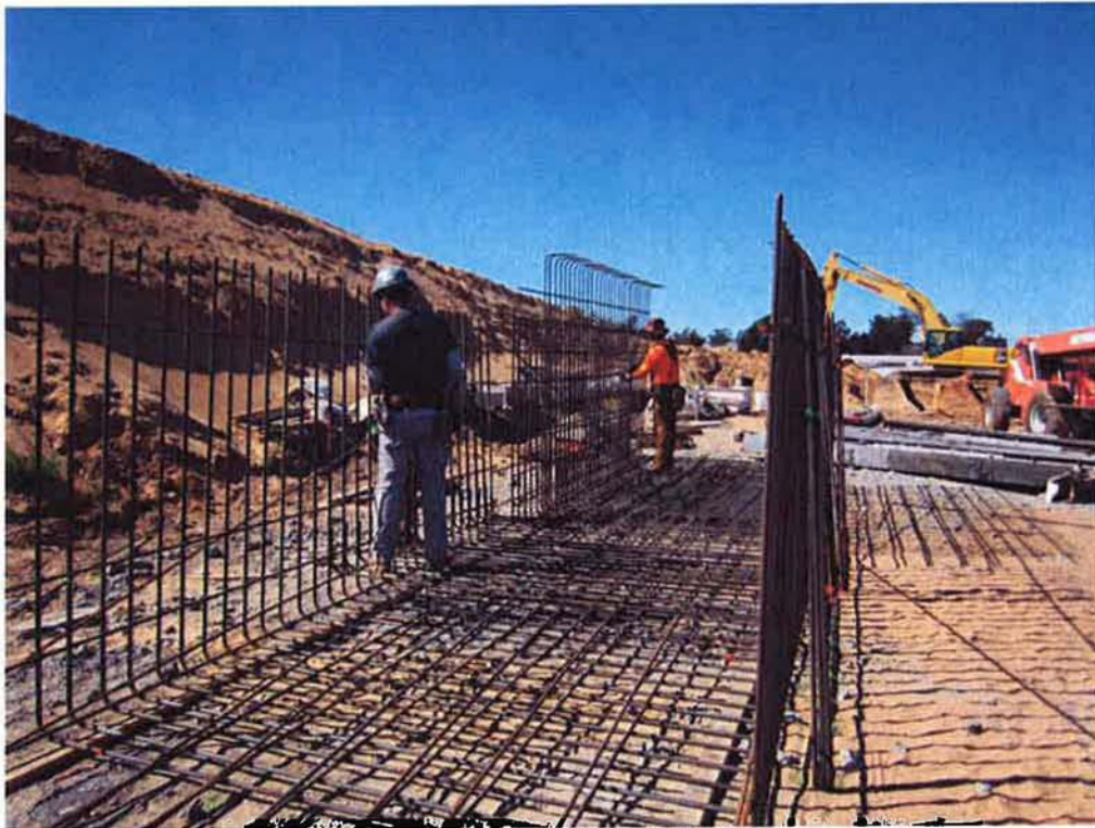
Reinforcement steel for the top half of the RAS/WAS pump stations.
