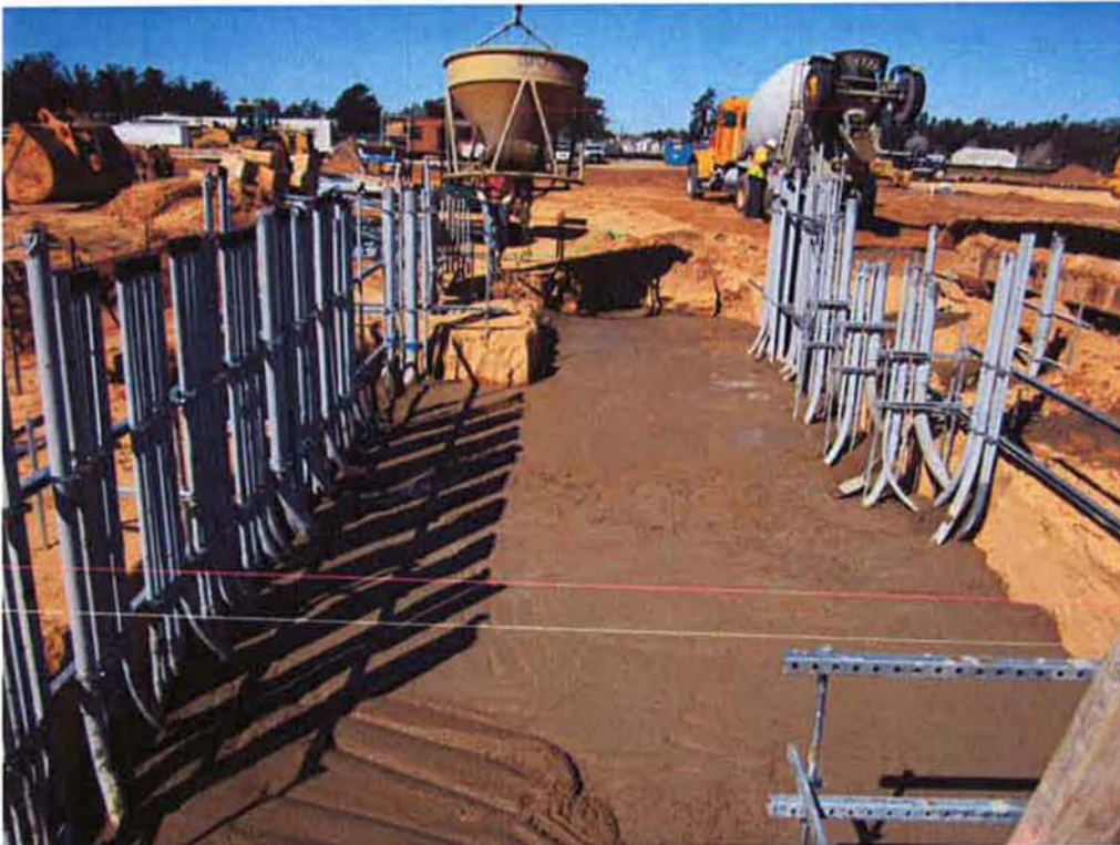
Completed slurry placement at Electrical/Blower Building.
