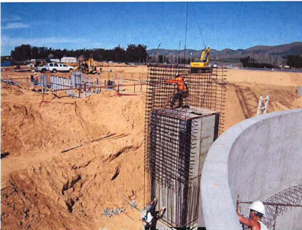
Setting reinforcing steel at RAS/WAS Pump Station #2.
