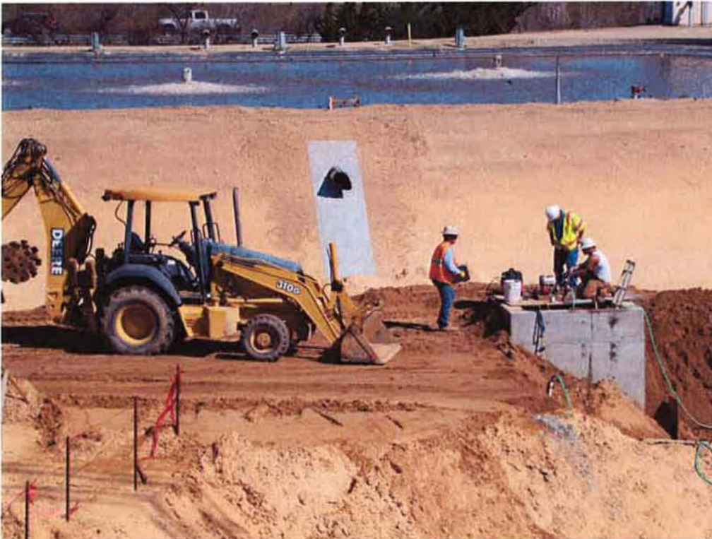
Water testing the weir box at the Aeration Basin.
