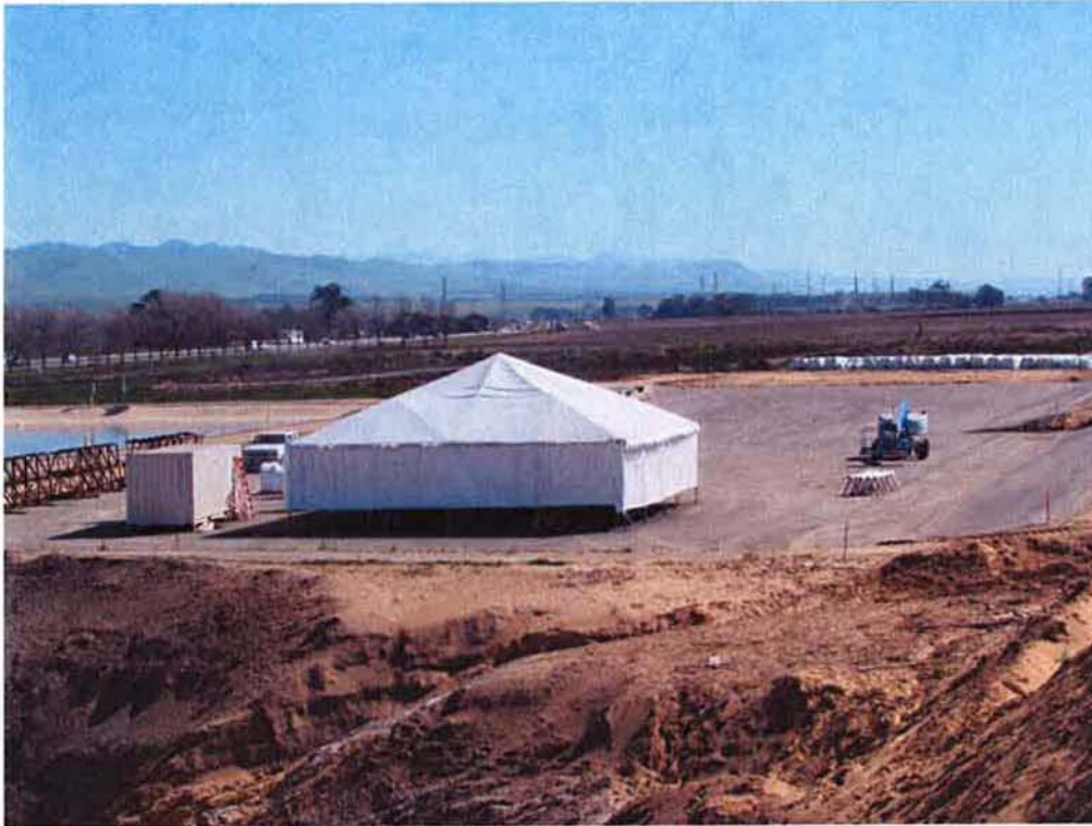
Coating tent for clarifier mechanisms.
