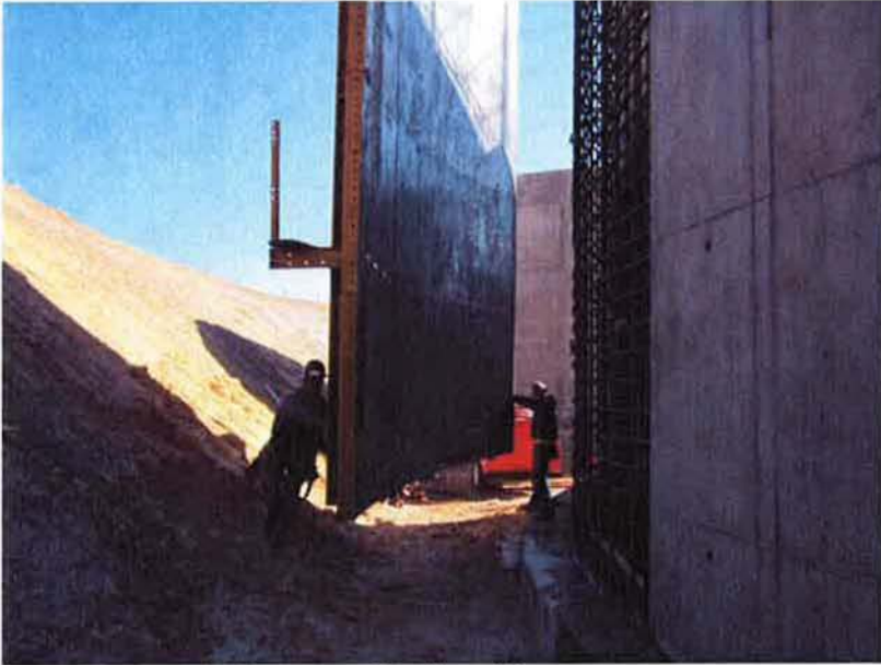
Closing outside forms at Clarifier #2.
