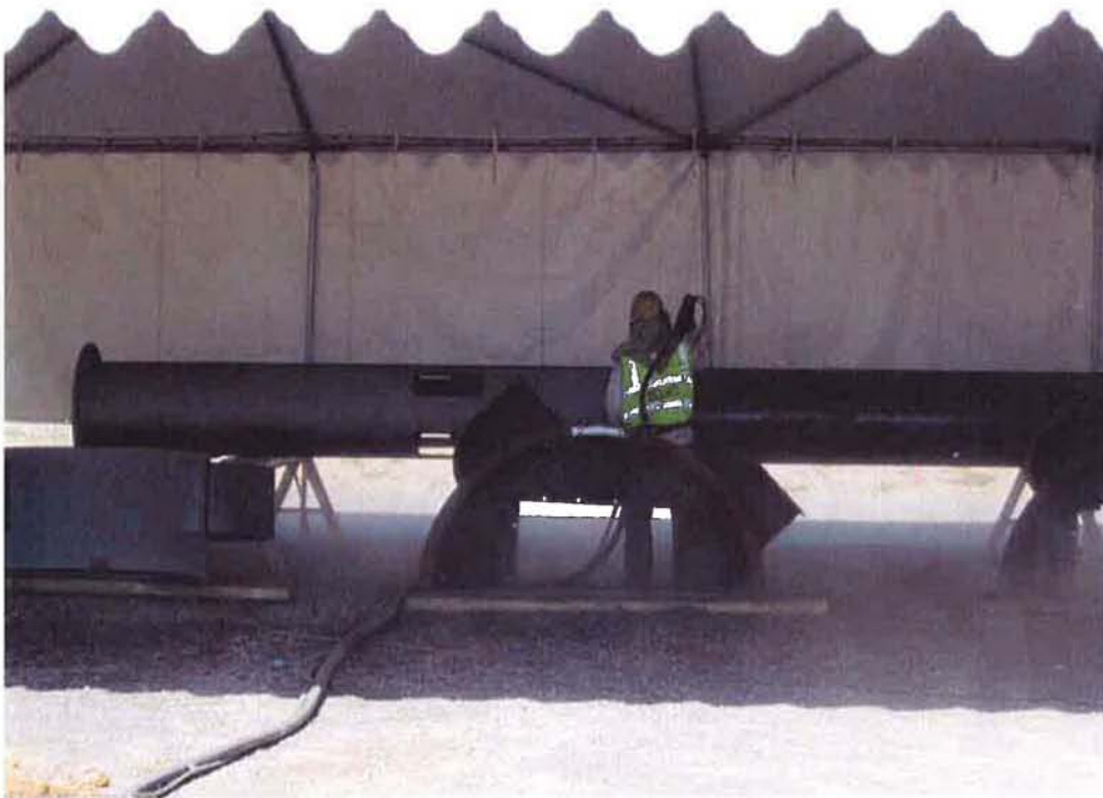
Blasting corrosion off clarifier mechanisms to prepare for primer.
