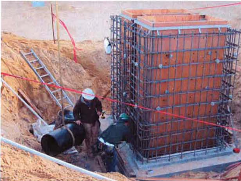
Finishing forms and installing pipe spoils for the effluent weir boxes.
