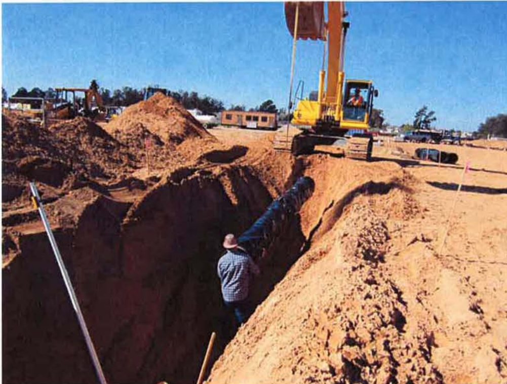
Installing 18" ML pipe between weir boxes.
