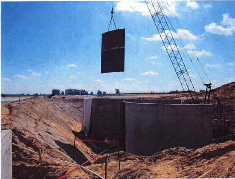
Swinging wall forms into place at Clarifier #2.
