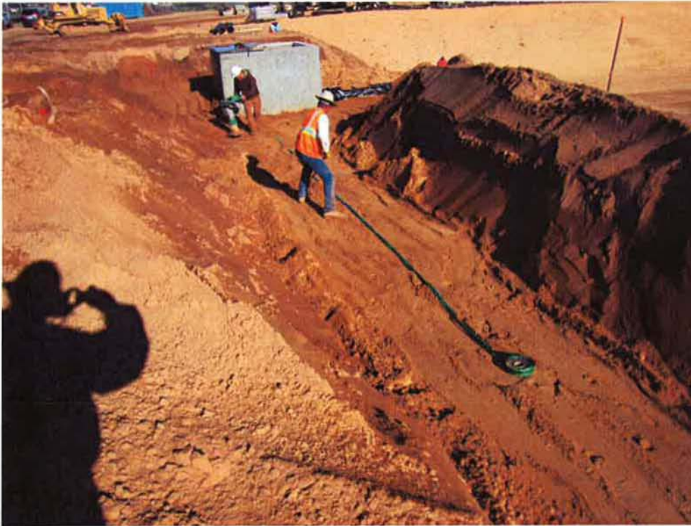
Backfilling over 18" ML pipe between weir boxes and placing warning tape.
