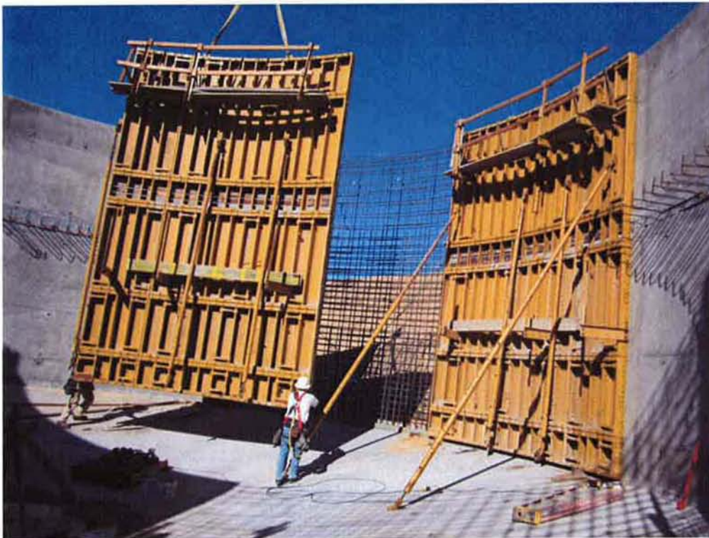
Setting inside forms at Clarifier #2.
