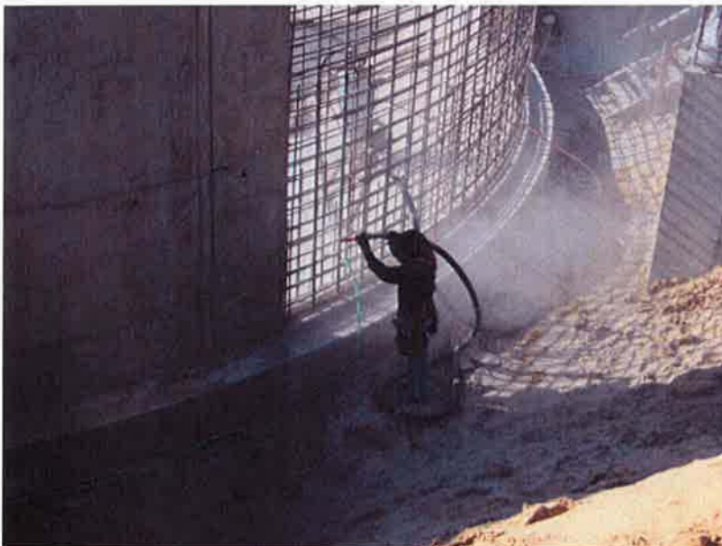
Sand blasting construction joints.
