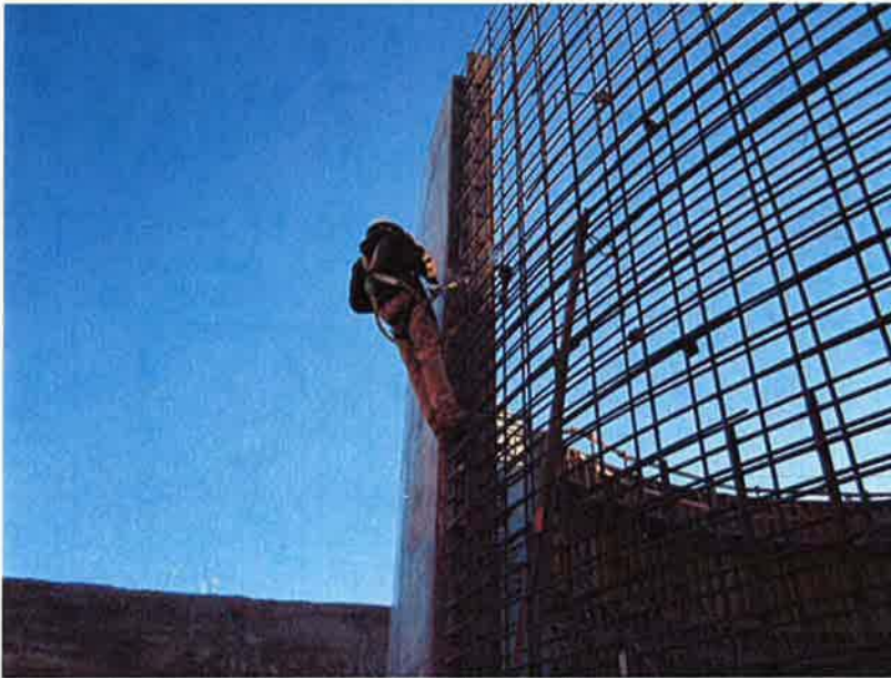
Removing forms from construction joints.
