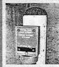
photos of typical cathodic testing stations and rectifier
