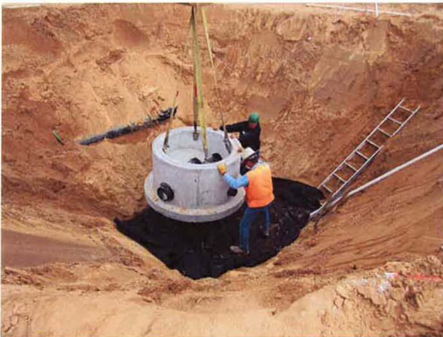
Setting base for Manhole #5.
