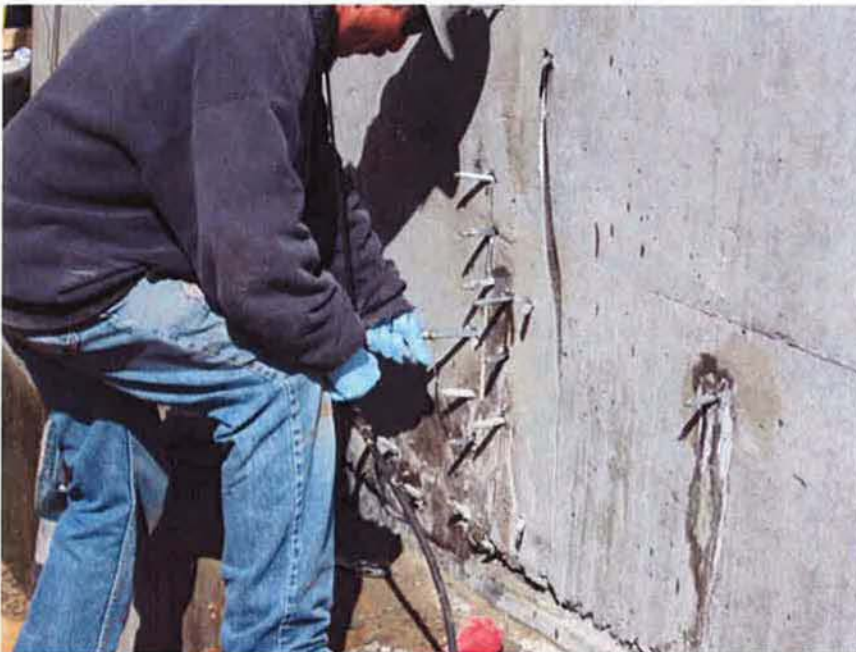
Patching leaks after leak test in Clarifier #1.
