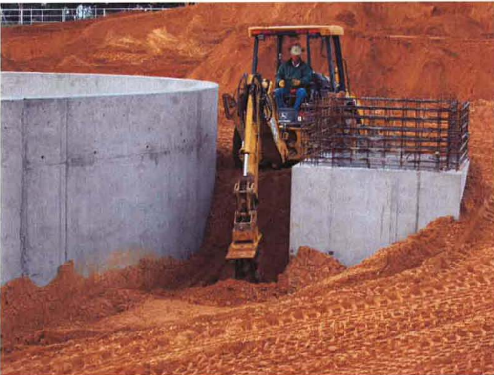
Backfilling and compacting between Clarifier #2 and RAS/WAS Pump Station #2.
