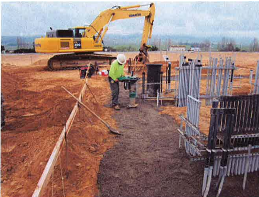
Backfilling and compacting at Electrical/Blower Building footing.
