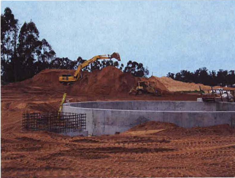
Backfilling and compacting almost complete around clarifiers.
