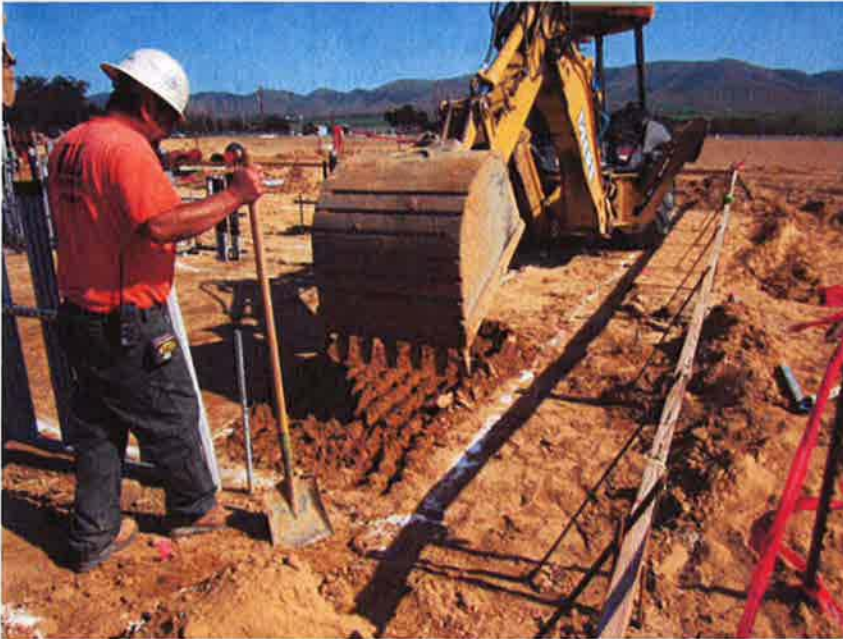
Excavating for Electrical/Blower Building foundation footing.
