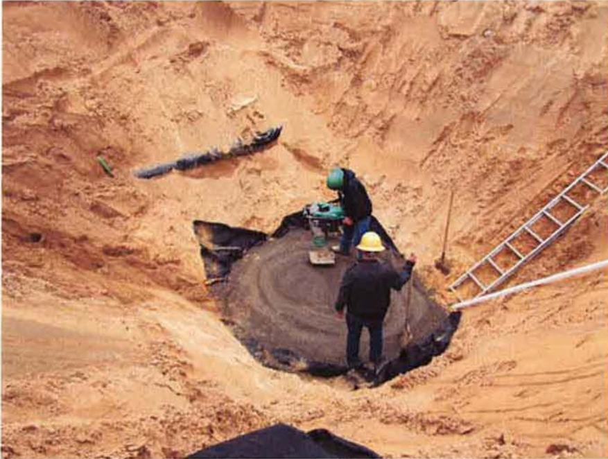
Compacting aggregate base wrapped in fabric for Manhole #5.
