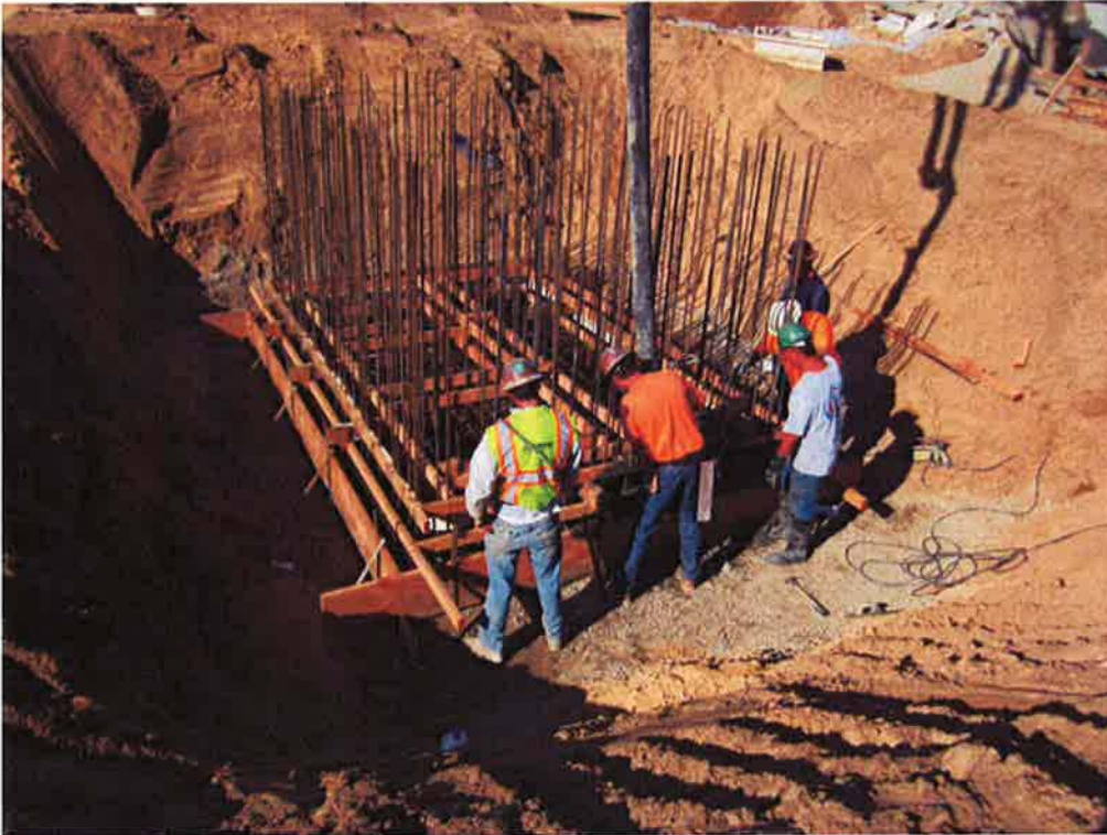
Pouring base of Distribution Box #1.
