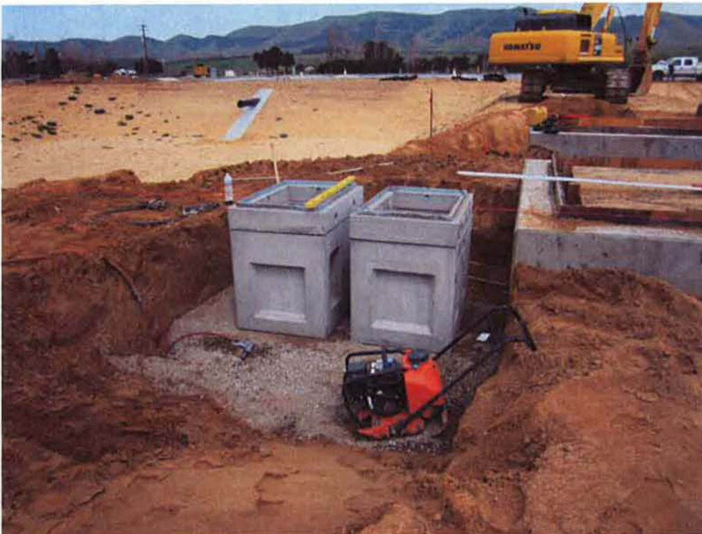
Pull box PBO5 (2 boxes) installed next to the Air Vault.
