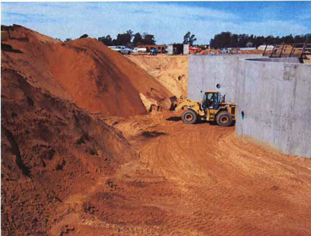
Backfilling and compacting around the clarifiers.
