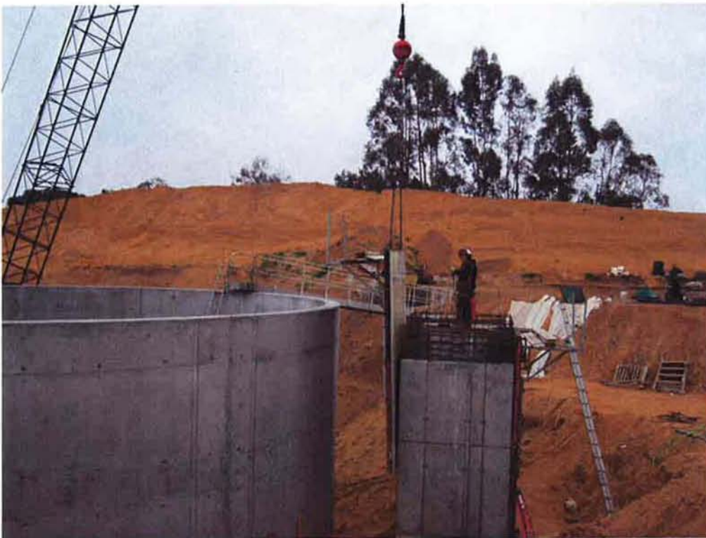
Removing forms after second pour of walls for RAS/WAS Pump Station #2.
