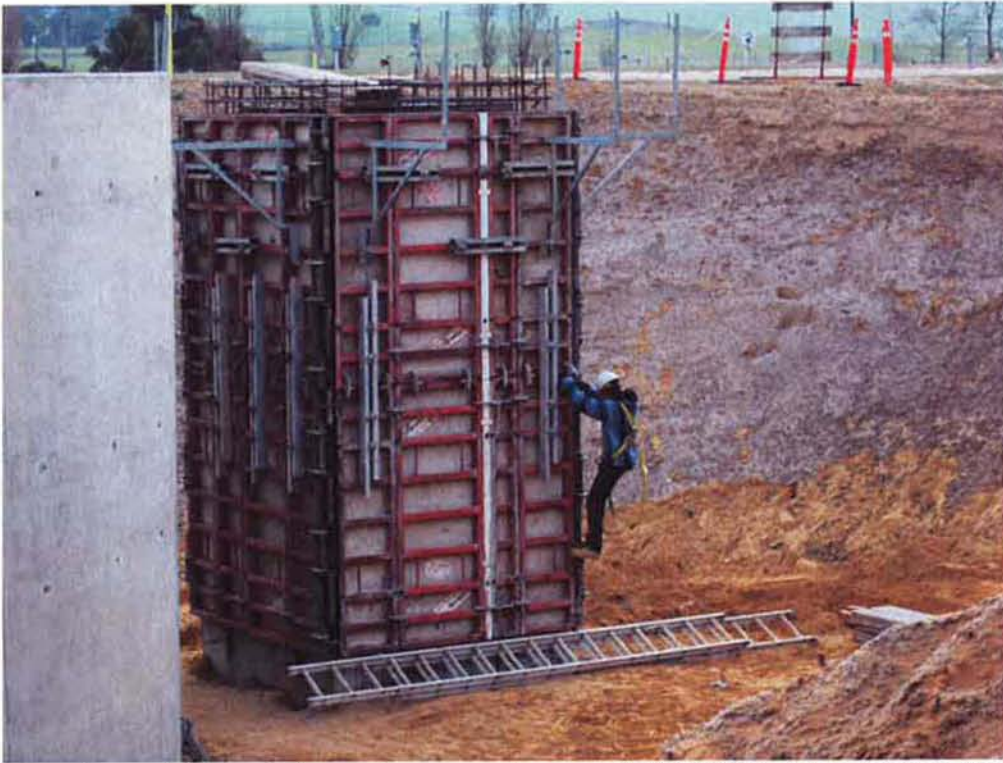
Securing outside wall forms for second pour of RAS/WAS Pump Station #2.
