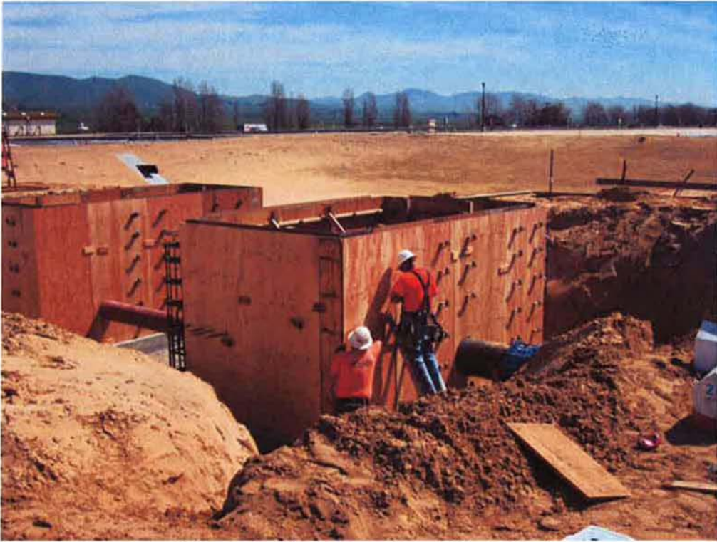
Completing the wall forms for the Air Vault and Meter Vault.
