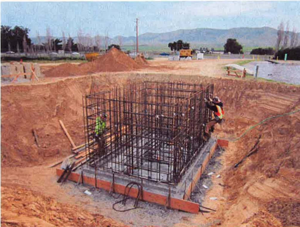
Installing rebar in walls for Distribution Box #1.
