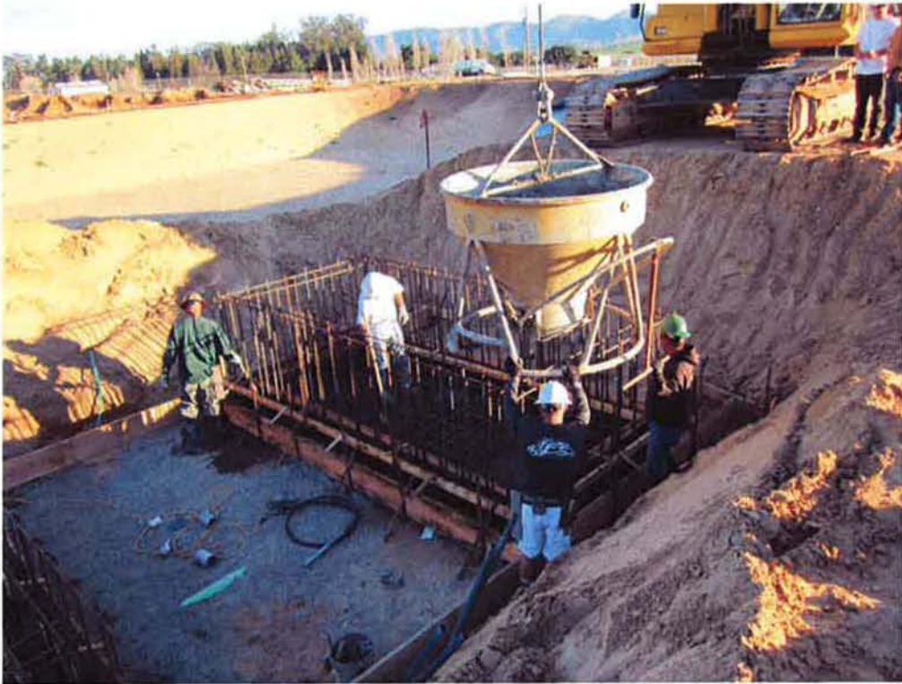
Pouring the foundations of the Air Vault and Meter Vault.
