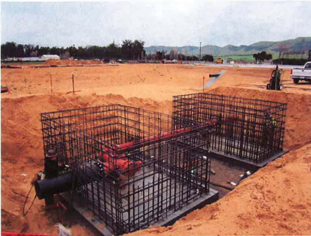
Installing the wall reinforcing for the Air Vault and Meter Vault.
