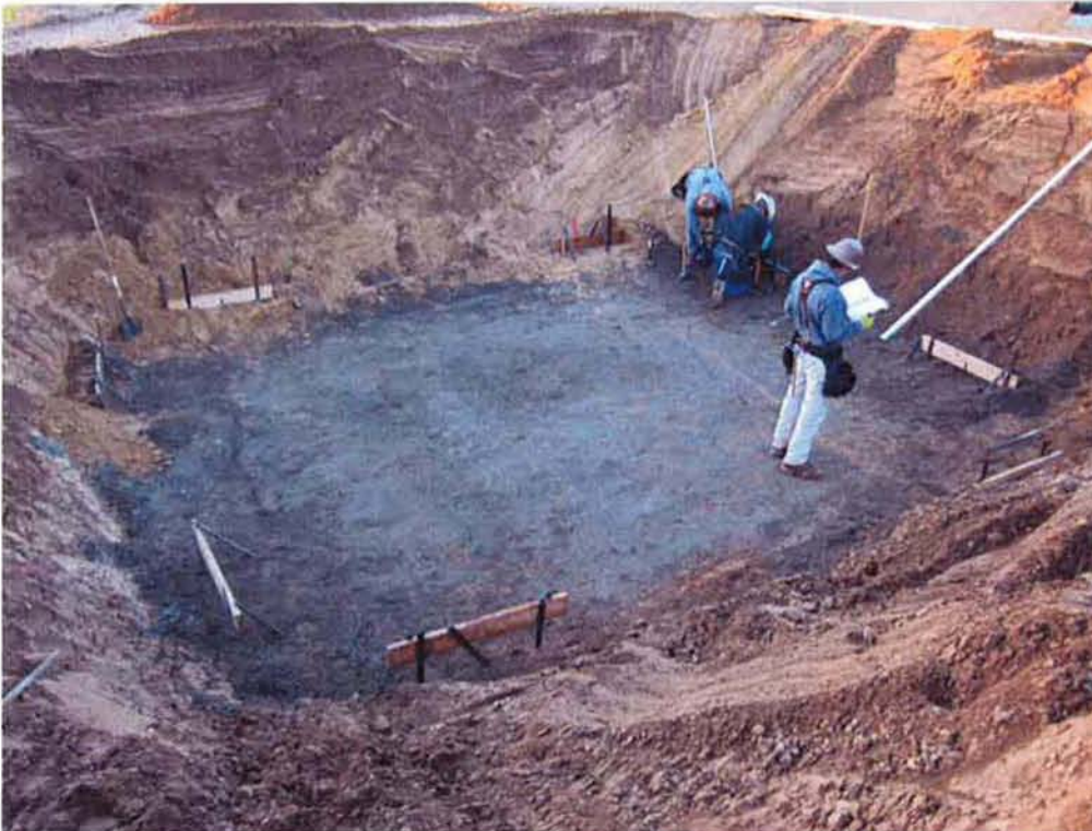
Excavation and base for Distribution Box #1.
