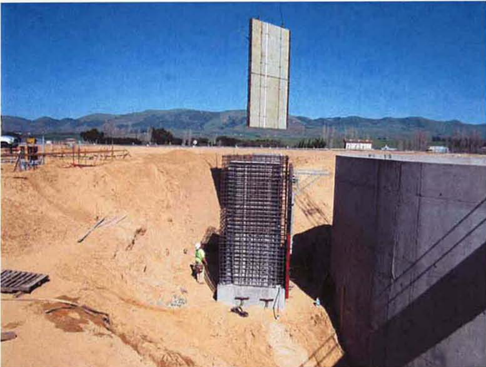
Setting wall forms for RAS/WAS Pump Station #2 second wall pour.
