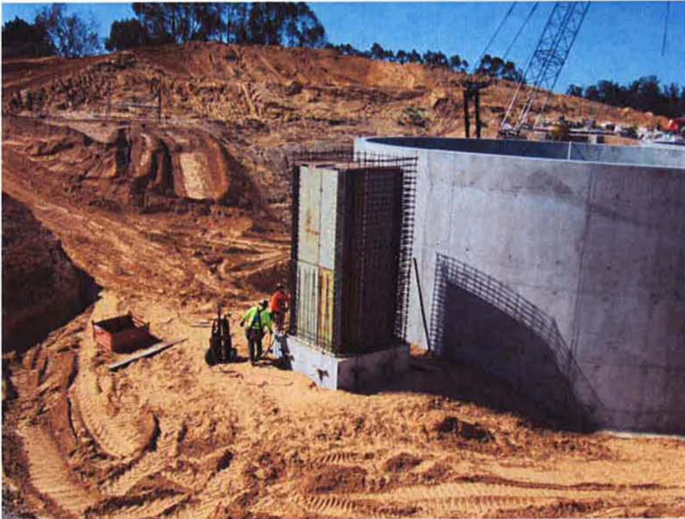
Preparing for second wall pour at RAS/WAS Pump Station #1.
