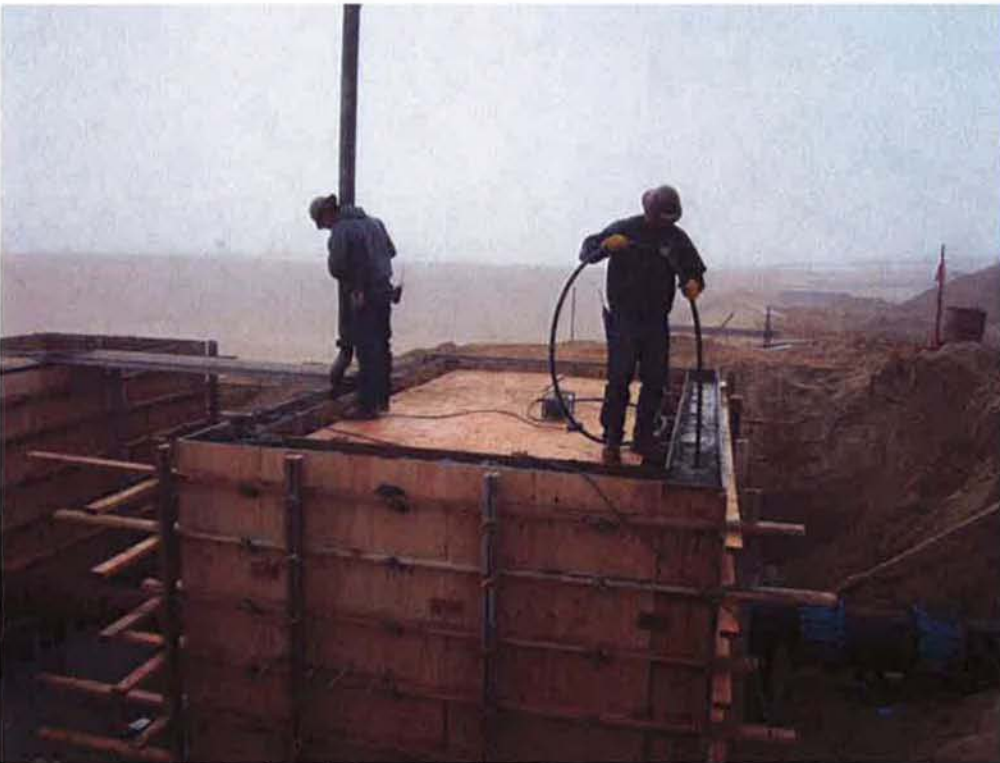
Pouring the Air Vault and Meter Vault walls.
