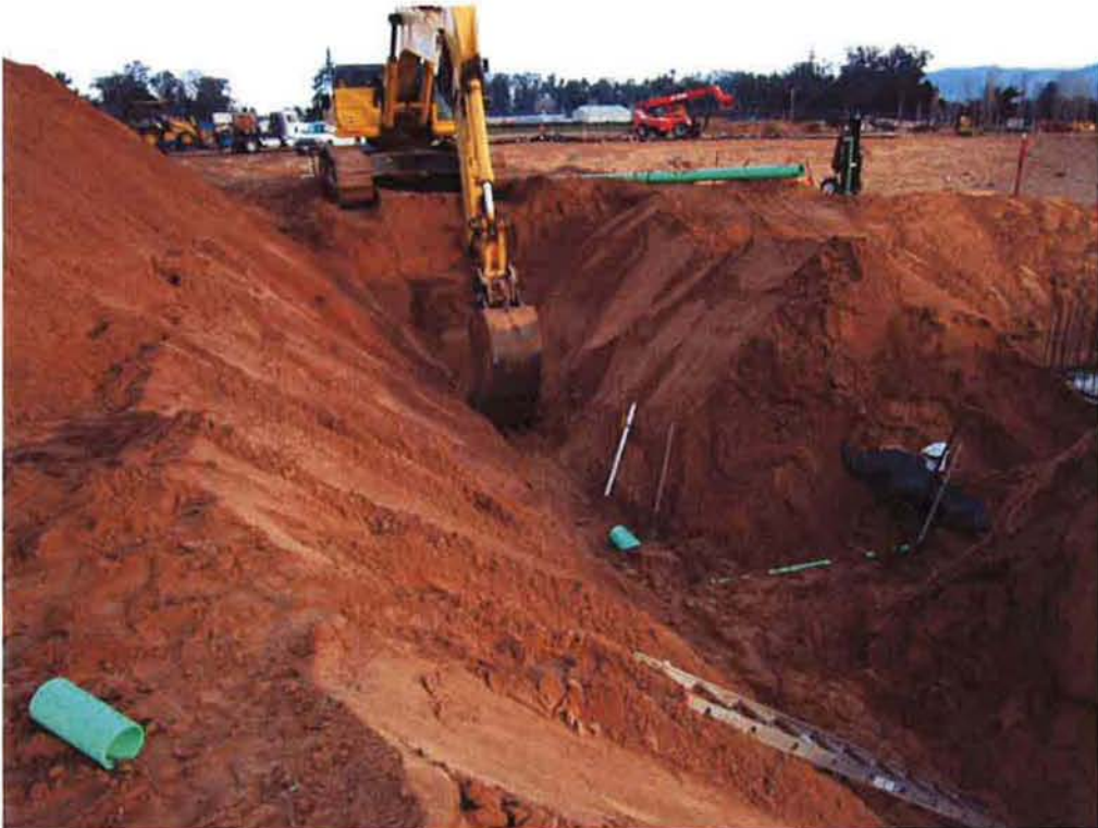
Installing 8" DR piping from Manhole #5 to Manhole #4.
