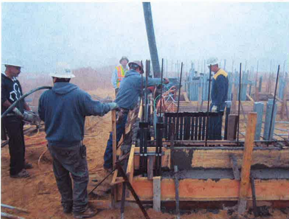
Pouring Electrical/Blower Building footing.
