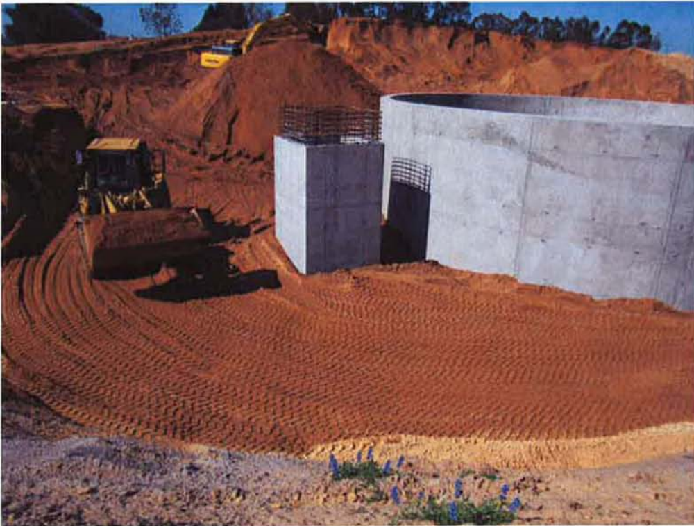
Backfilling and compacting around RAS/WAS Pump Station #1 and Clarifier #1.
