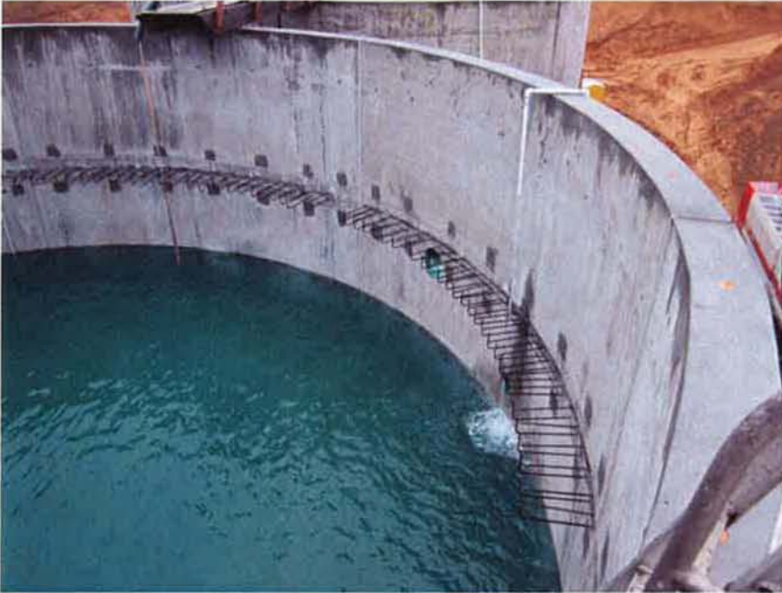
Leak testing inside Clarifier #2.
