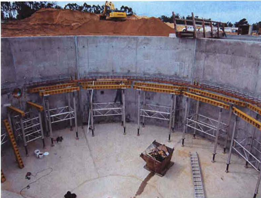
Setting forms for pouring launder inside Clarifier #1.
