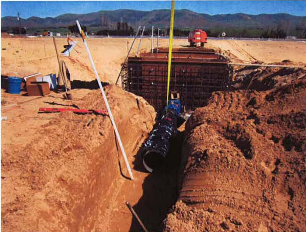
Installing the 18" AR piping to the Air Vault and Meter Vaults.
