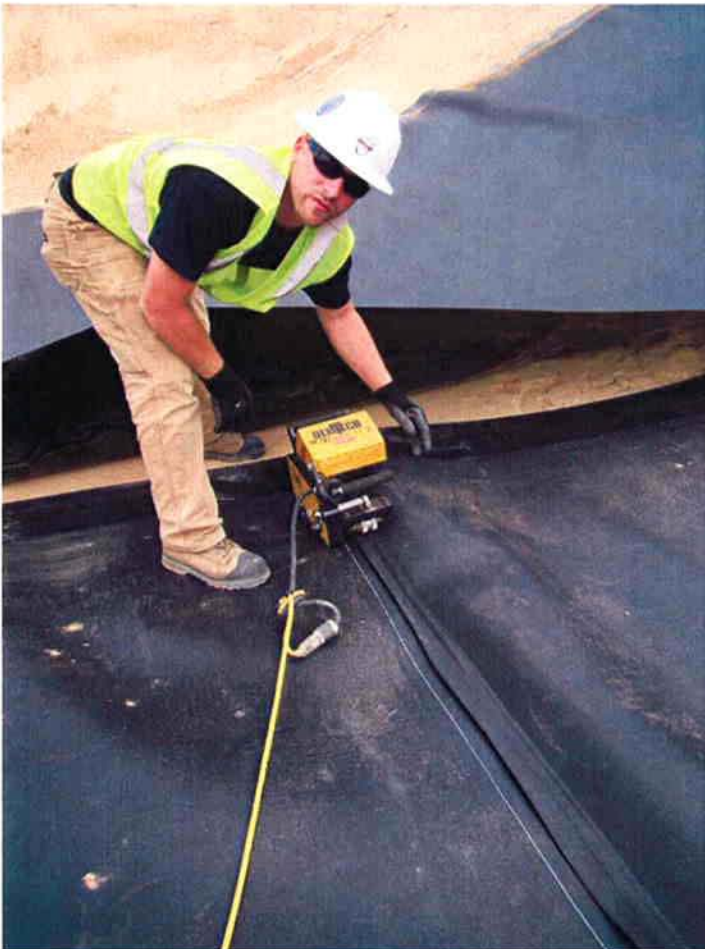
Barber-Webb double fusion welding the liner at 800 degrees.
