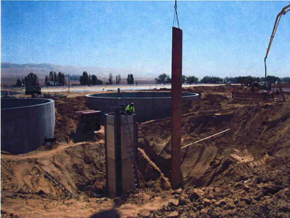
Cushman setting forms for the Scum Well walls.
