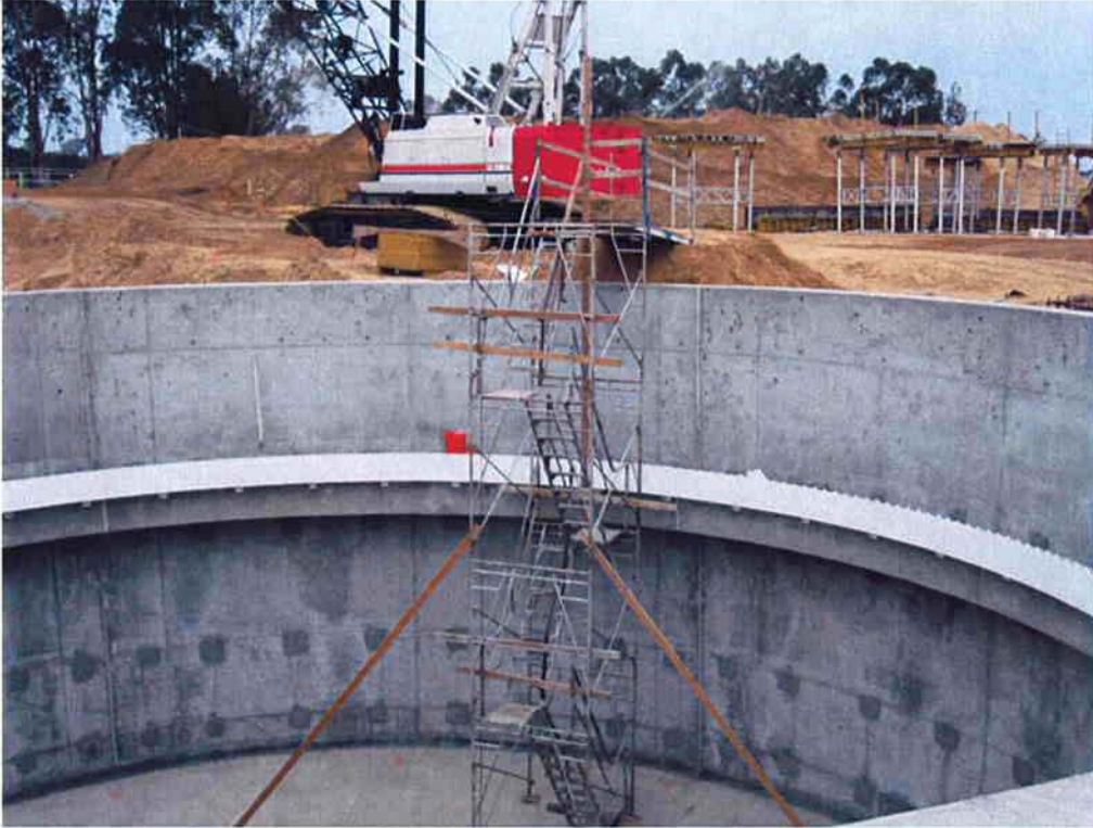
Cushman building scaffolding for access into Clarifier #2.
