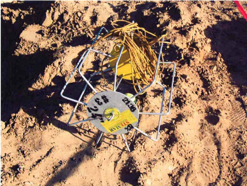
Mandrel used for testing the 24" SE2 pipe.
