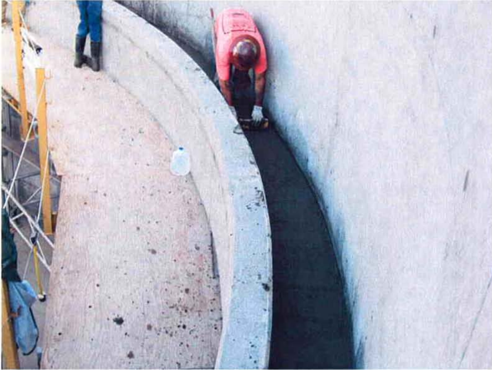
Finishing concrete floor of launder in Clarifier #2.
