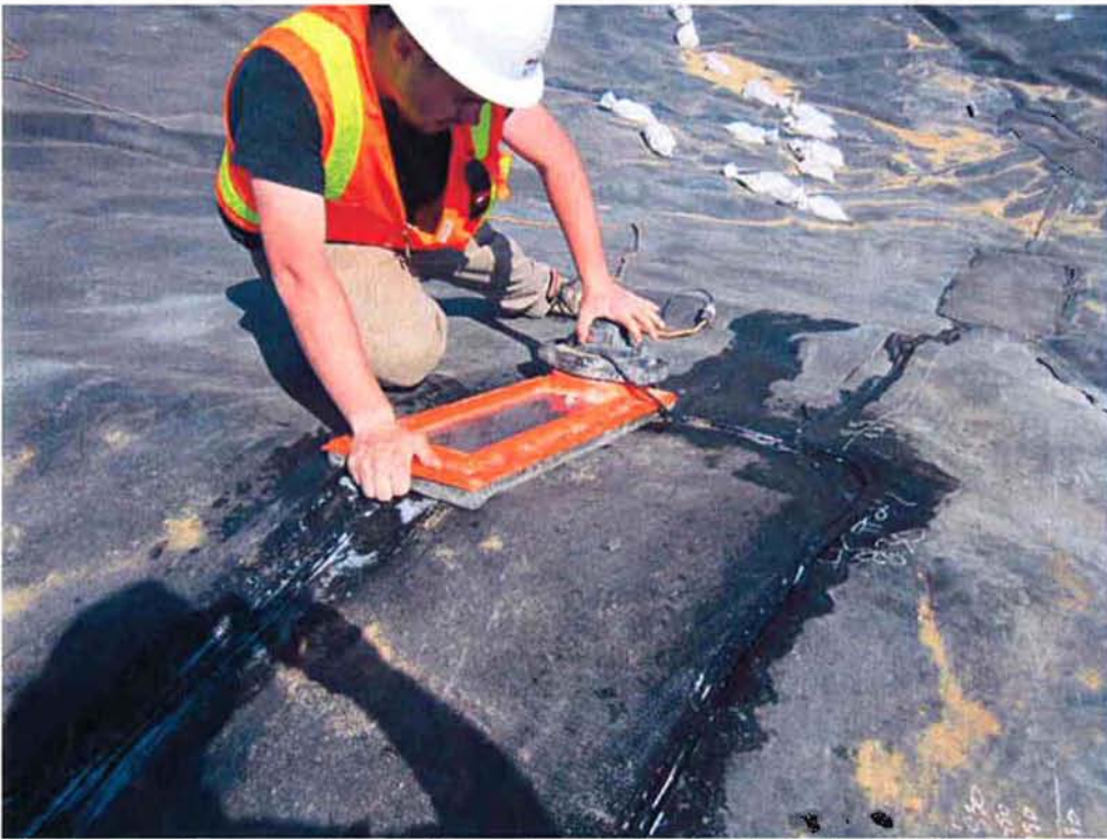
Vacuum testing extrusion welds at destructive double fusion weld test location.
