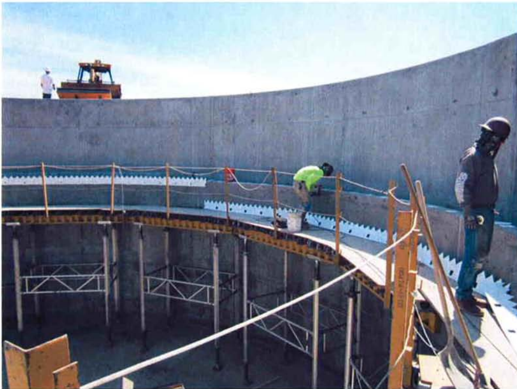
Installing toothed weir plate in Clarifier #2.
