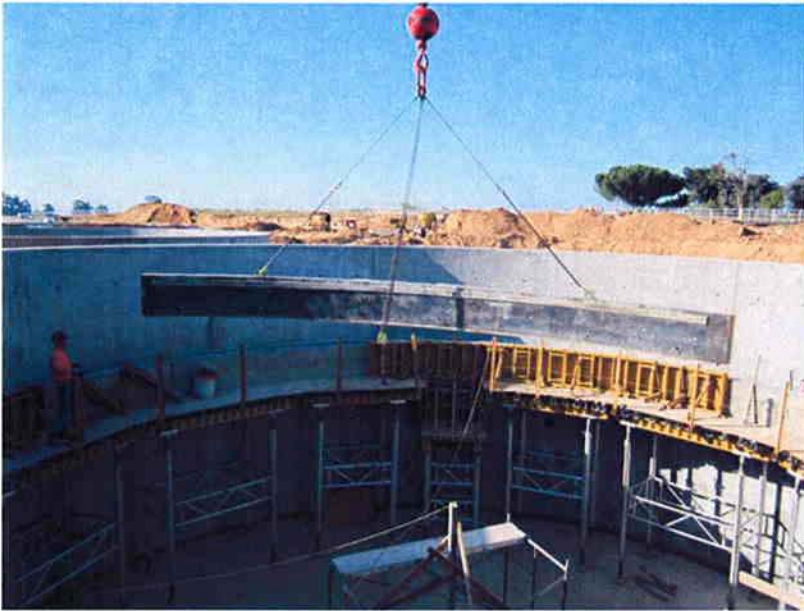
Setting forms in Clarifier #2 for last launder pour.
