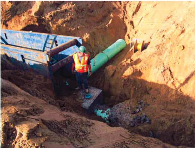
Thrust block installed on 24" SE2 pipe.
