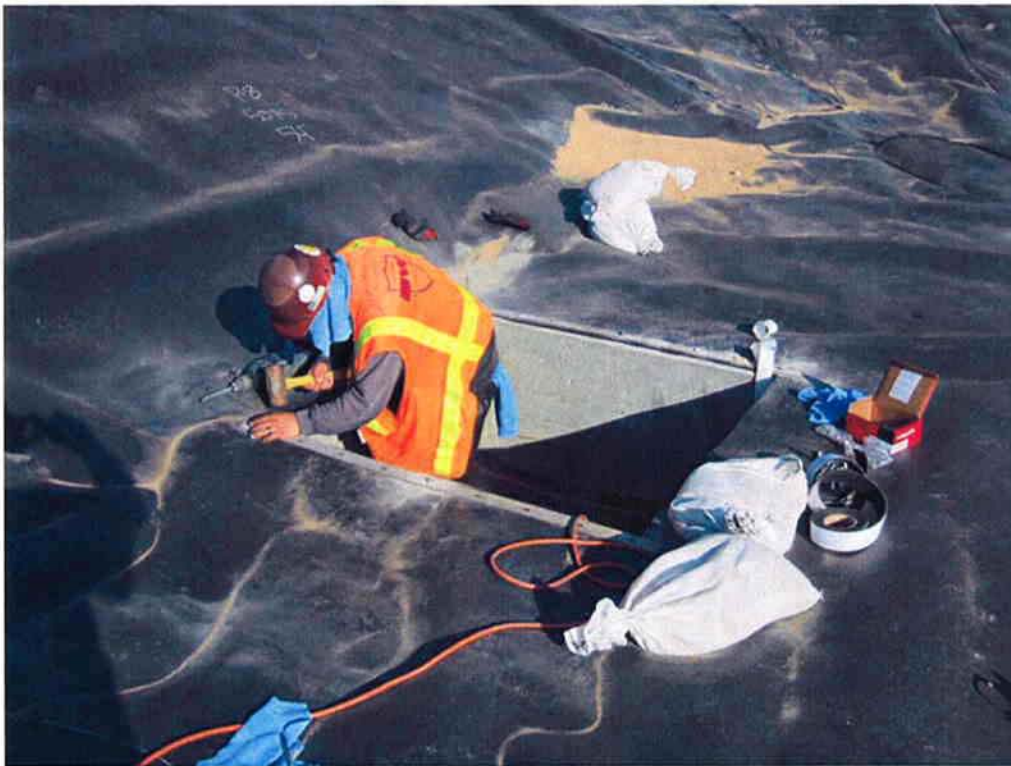
Installing liner around catch basin at the bottom of Aeration Basin #1.
