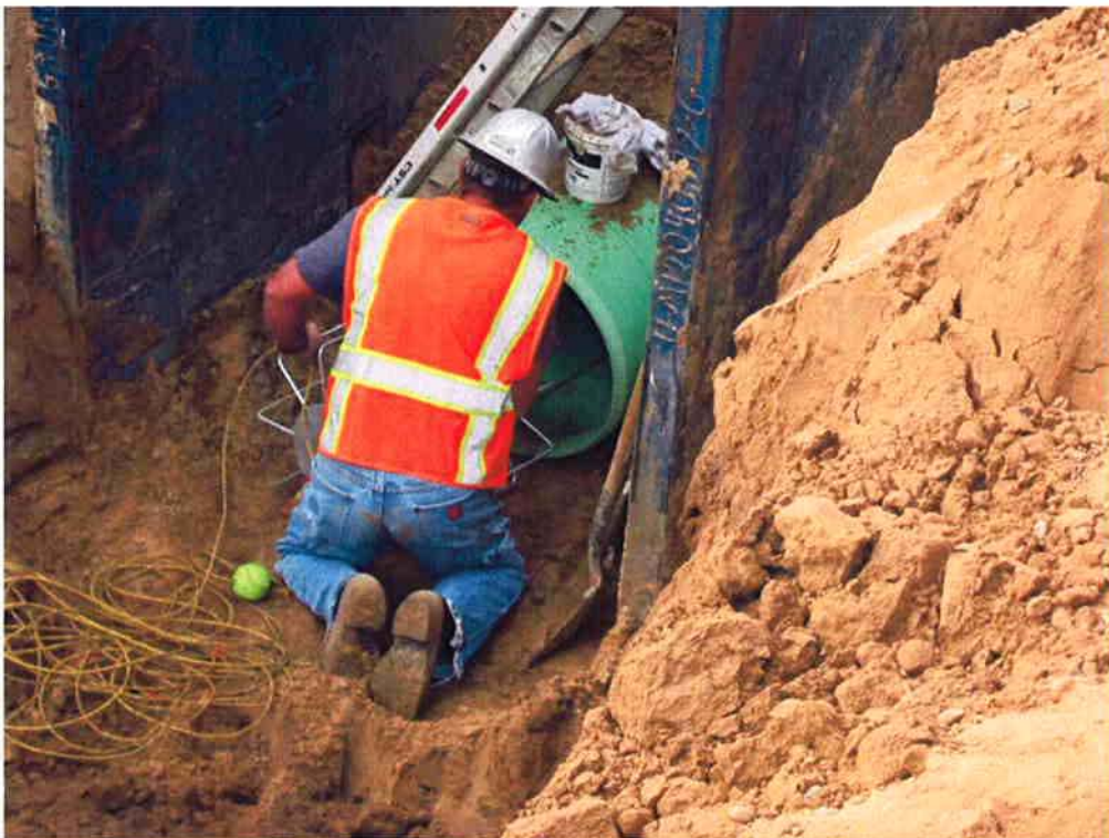
Removing mandrel from 24" SE2 pipe after deflection testing.
