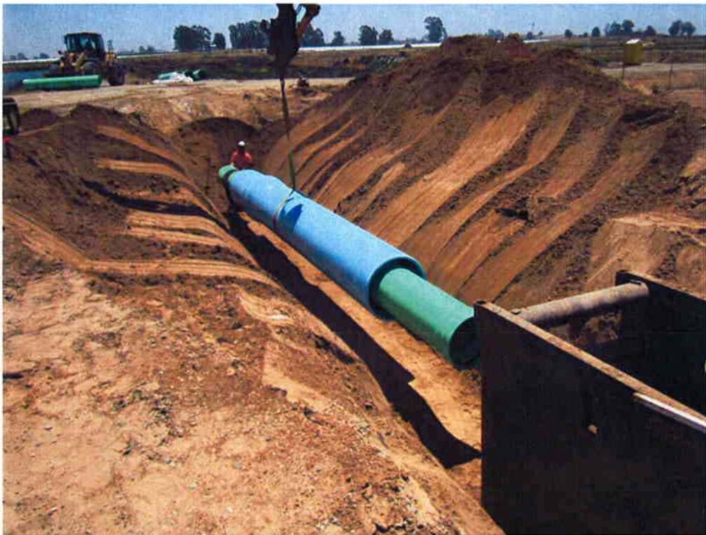
Installing the 24" SE2 pipe and casing across the DWR easement.
