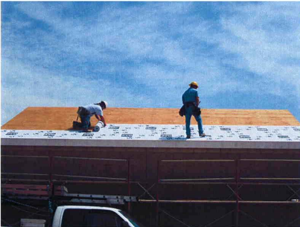
Roofing subcontractor, Dueck Construction installing moisture barrier over plywood.
