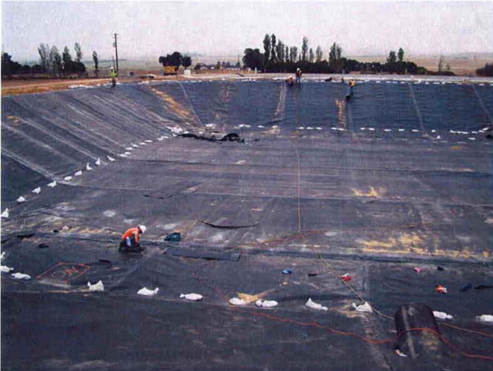
Liner installation and testing at Aeration Basin #1.
