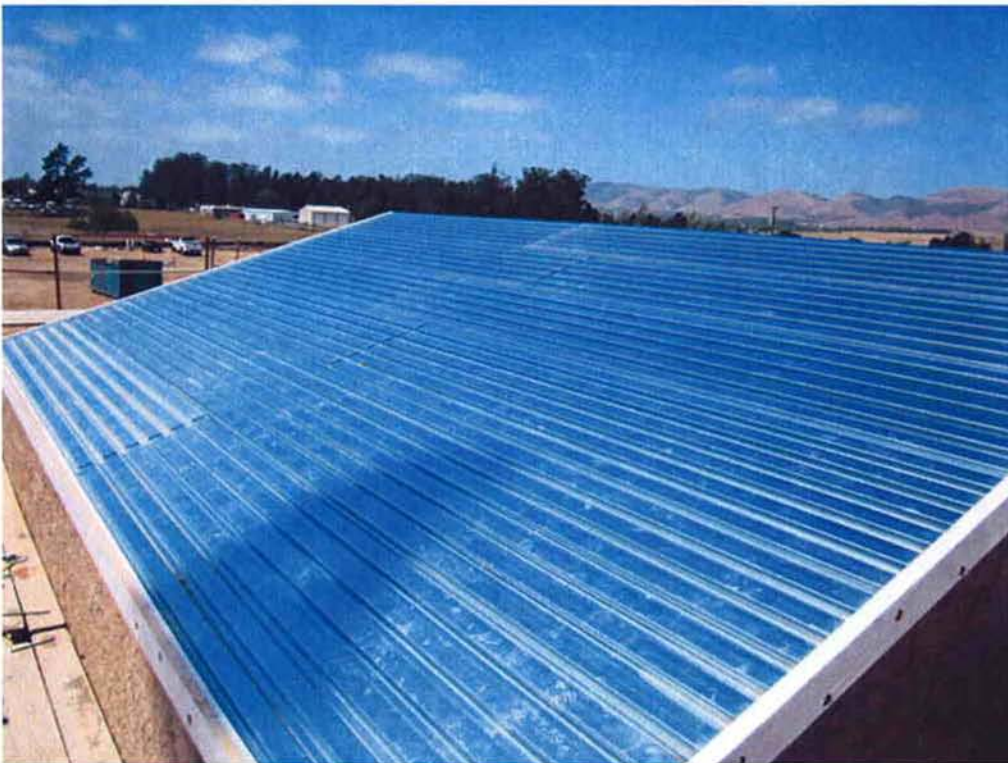
Metal decking installed before crimping.
