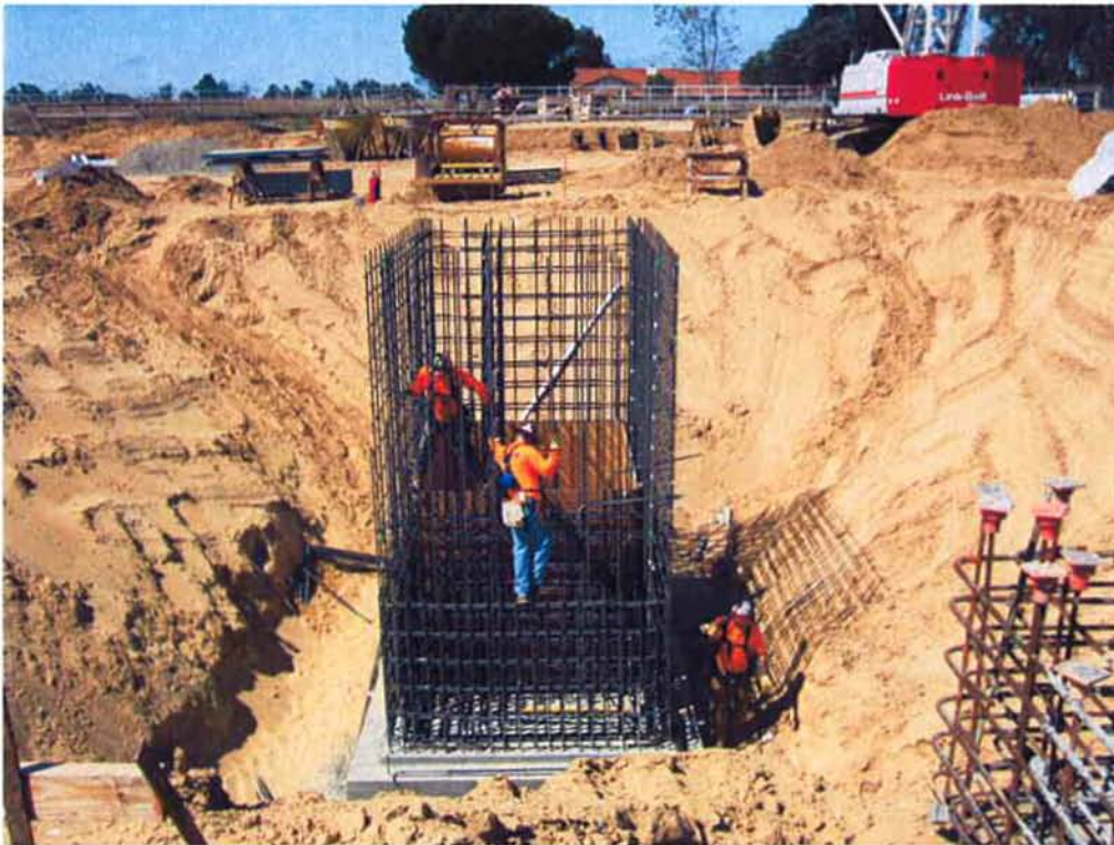
Subcontractor, CMC Rebar installing rebar for walls of Processed Water Pump Station.
