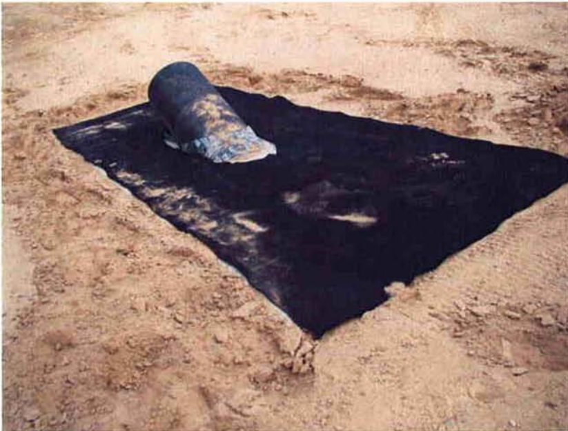
Felt pad installed over concrete at inlet pipe to protect liner from rubbing and wear.
