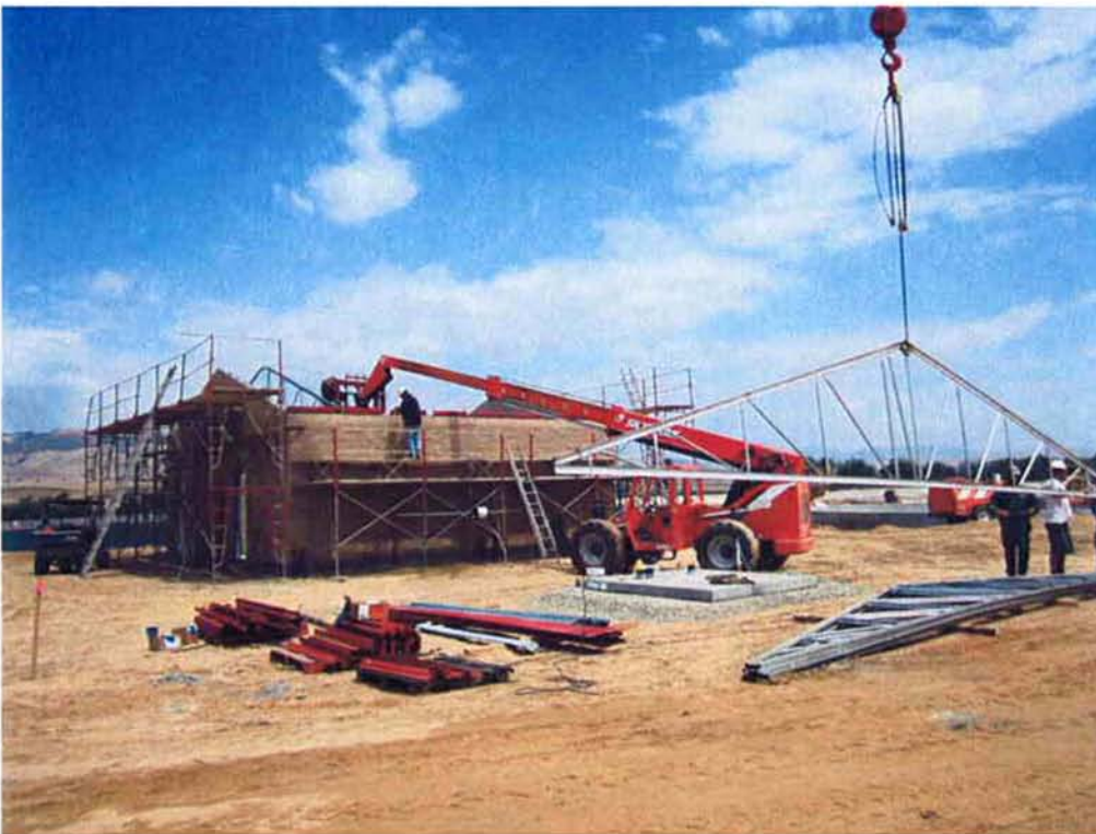
Cushman installing metal roof trusses.
