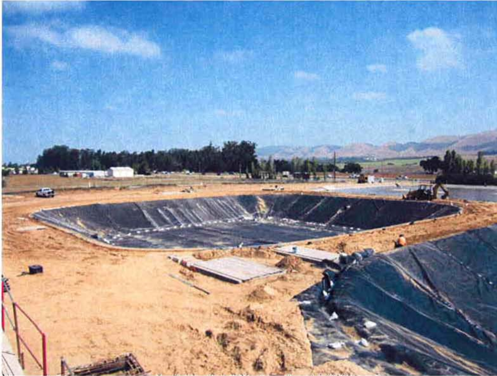
Lining installation completed in Aeration Basin #1 and Cushman compacting lining anchor with backhoe.
