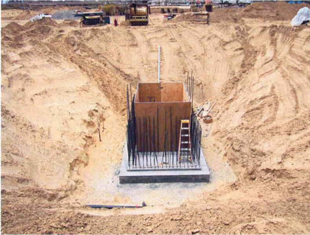
Foundation of Processed Water Pump Station poured and wall forming started.
