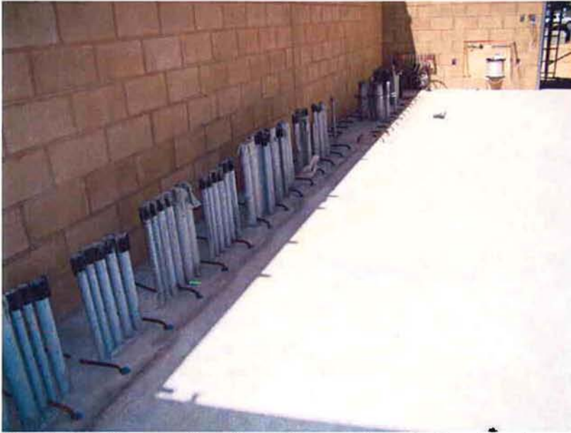
Conduit and epoxy dowels set for pouring electrical equipment pad.
