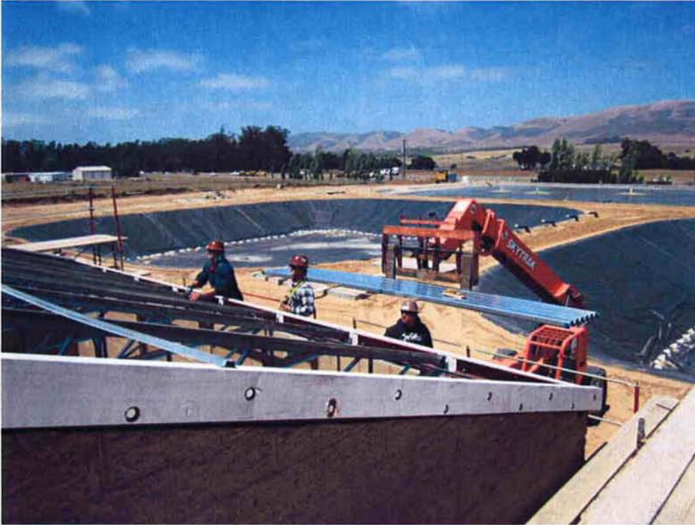
Cushman installing metal decking on truss system.
