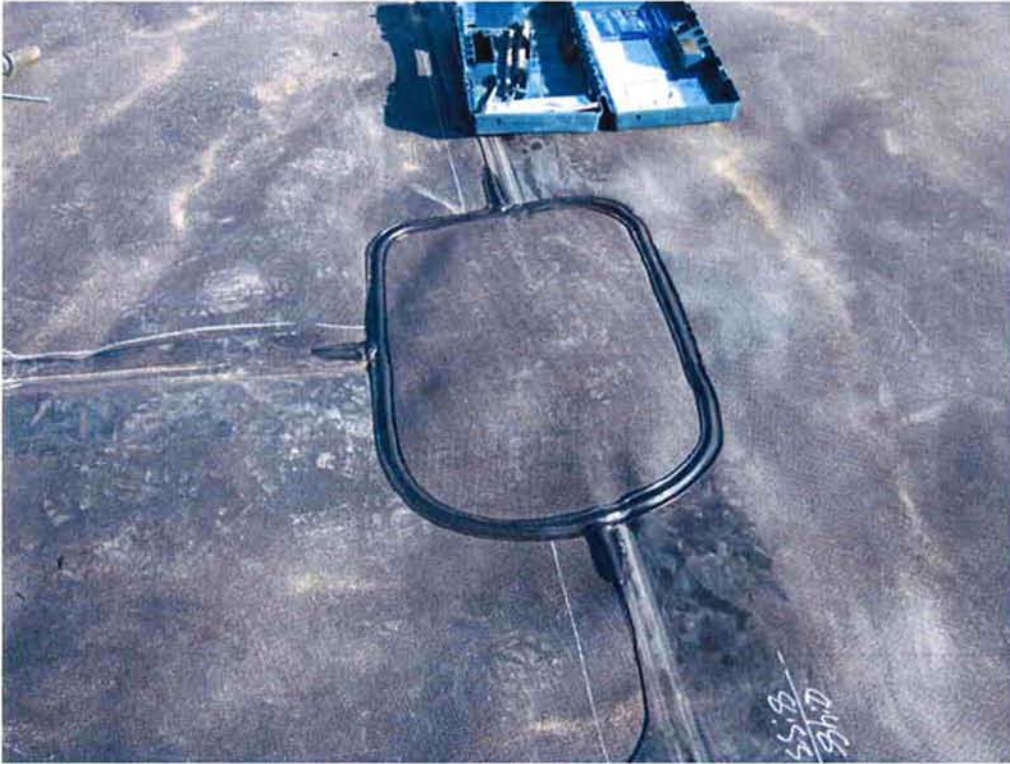
Patch made with extrusion weld at destructive double fusion weld test location.
