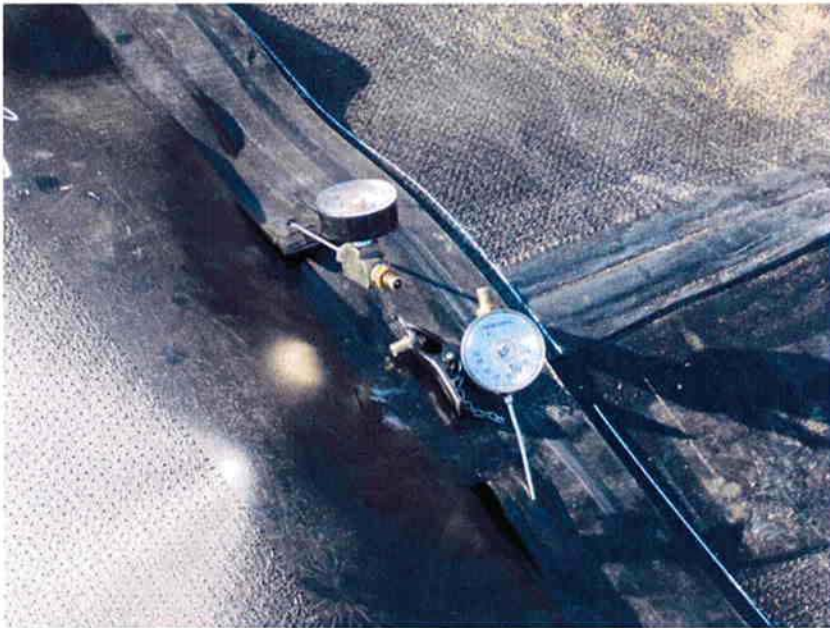
Air testing double fusion welds as liner is installed.
