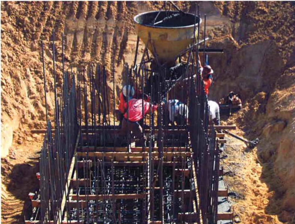
Construction pouring foundation of Processed Water Pump Station.
