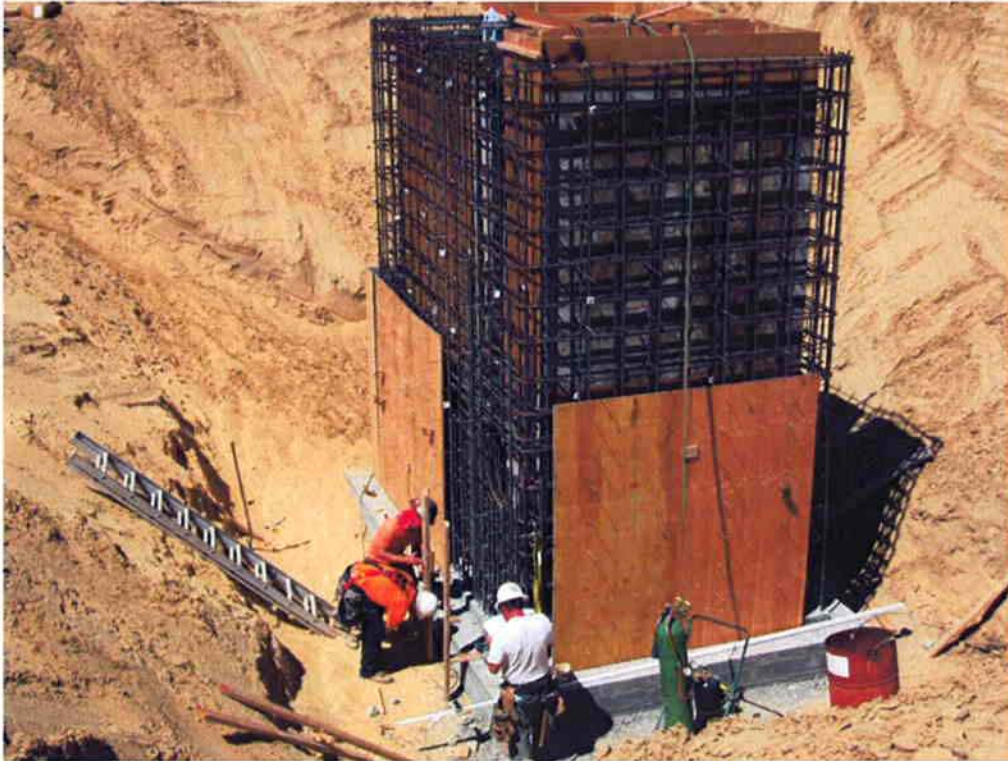
Completing wall forms for Processed Water Pump Station.
