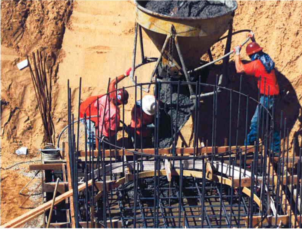
Pouring foundation of the Scum Well.
