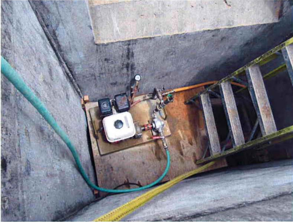
Pressure testing the 24" MDPE pipe at Distribution Box #2.
