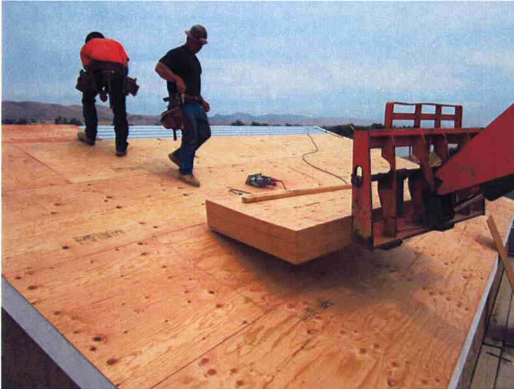
Cushman installing plywood sheeting over metal decking.
