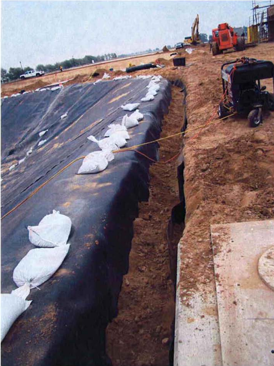
Backfilling liner anchor at the top of Aeration Basin #1.
