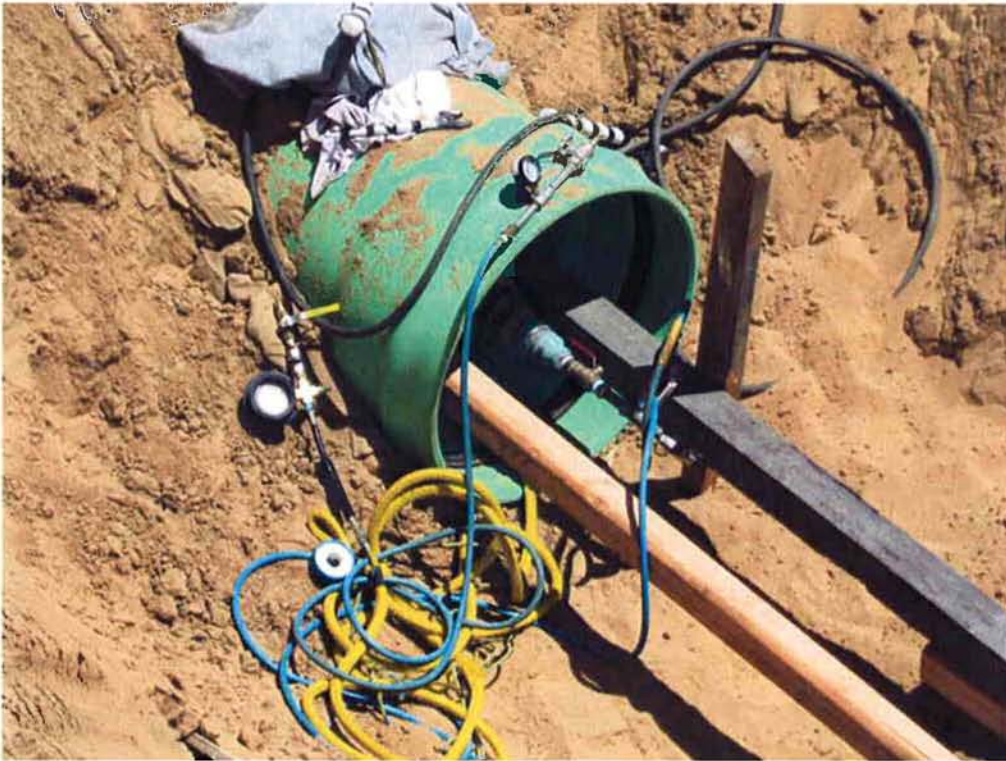
Pressure testing the 24" SE2 pipe.
