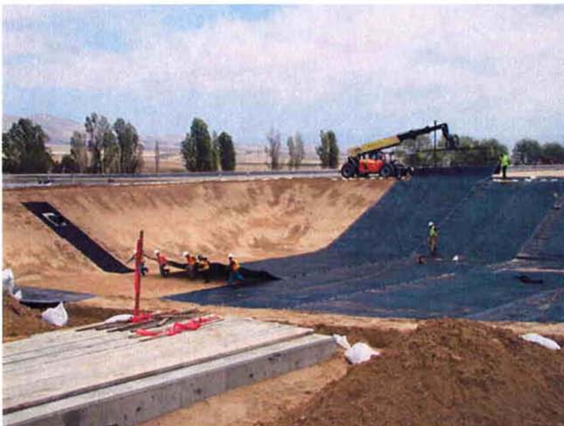
Subcontractor Barber-Webb pulling the liner sheets into place across the Emergency Holding Basin.
