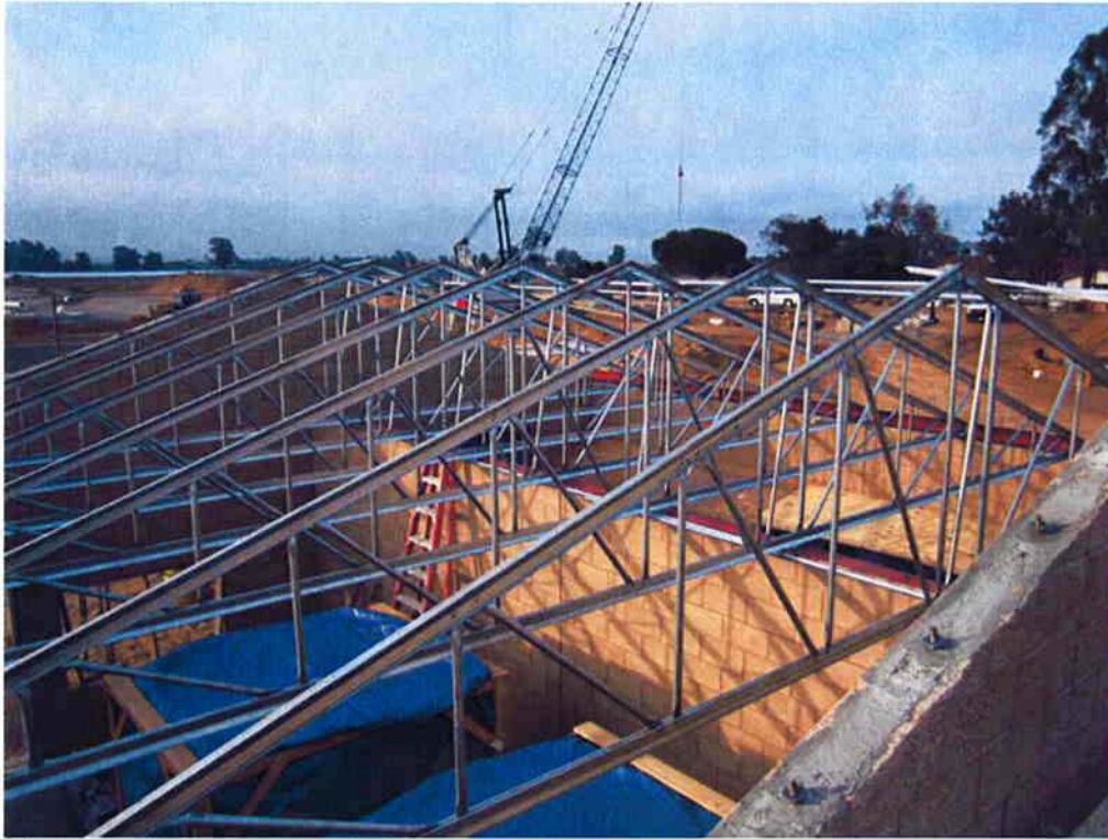
Metal roof trusses installed.
