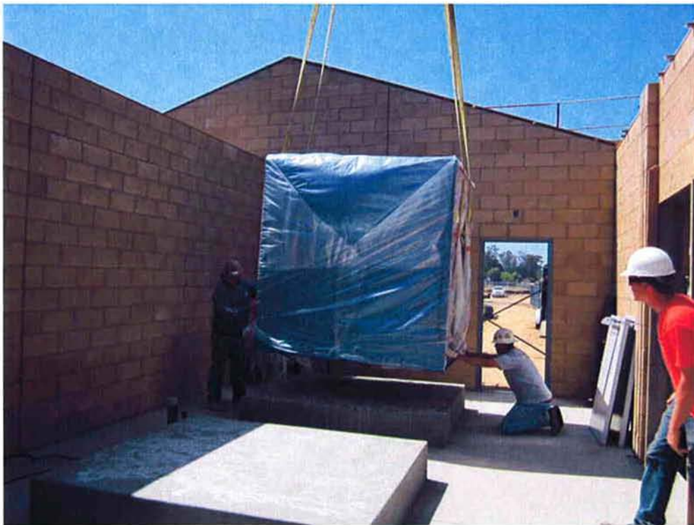
Cushman and Bergelectric setting blowers on equipment pads before installing the roof.
