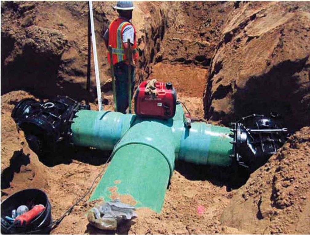
Cushman installing a tee on the 24" SE2 pipe.
