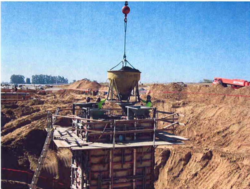
Cushman pouring the Scum Well walls.
