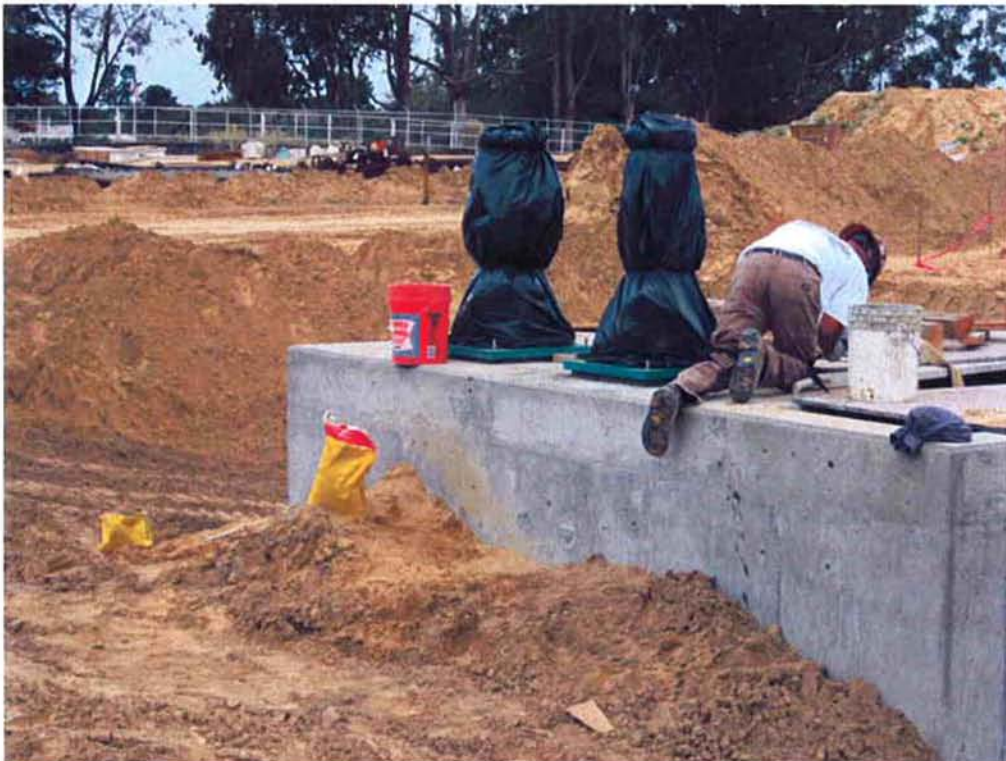
Cushman dry packing the mounting plates for the vertical turbine pumps at the Process Water Pump Station.
