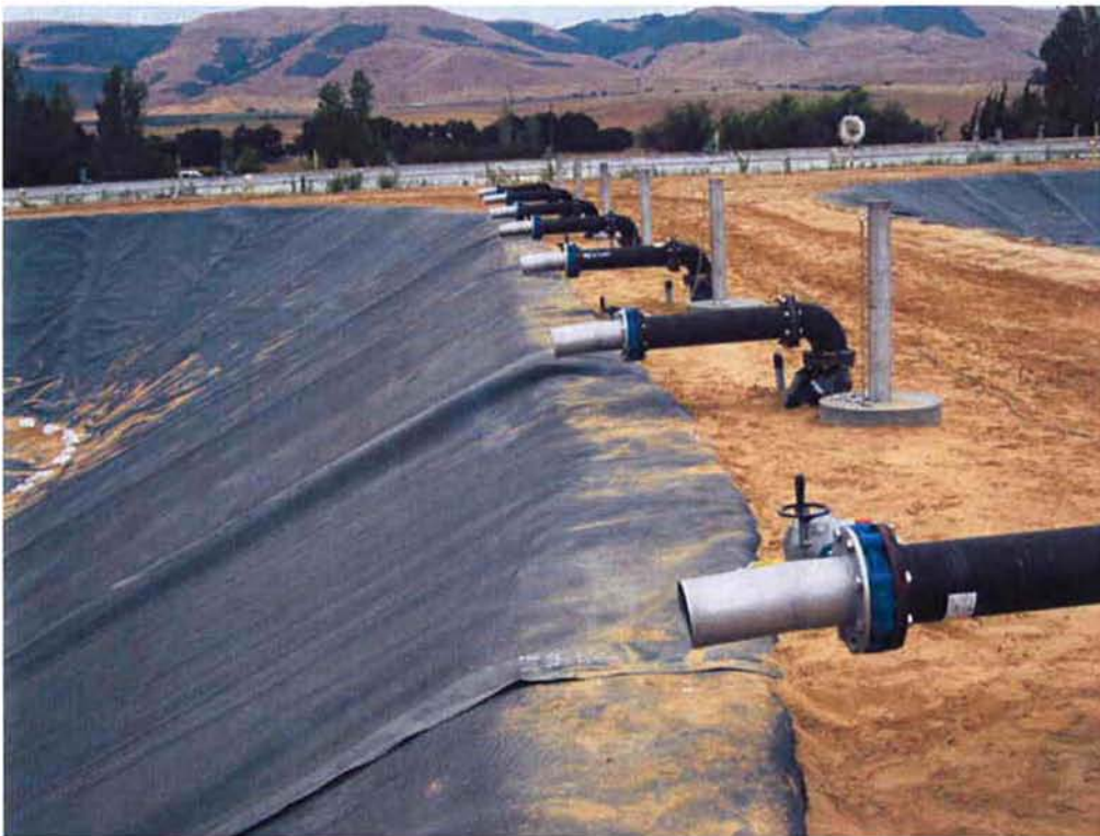
AR piping with valves and posts installed.
