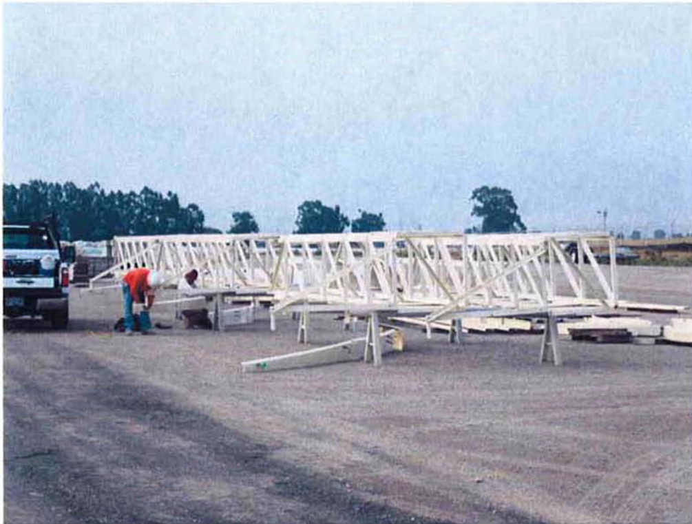
Cushman assembling clarifier mechanisms in preparation for installation inside clarifiers.
