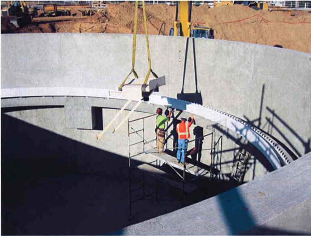
Cushman installing the scum trough inside Clarifier #1.
