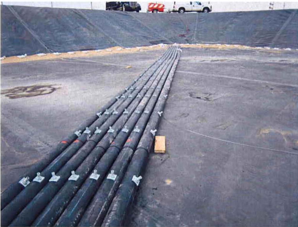
HDPE pipe welding complete and nipples installed on pipe.
