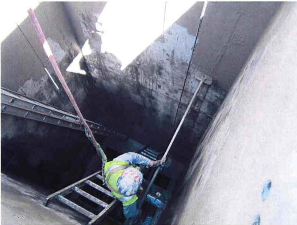
KNK Coating applying Xypex to the inside of RAS/WAS Pump Station #2.
