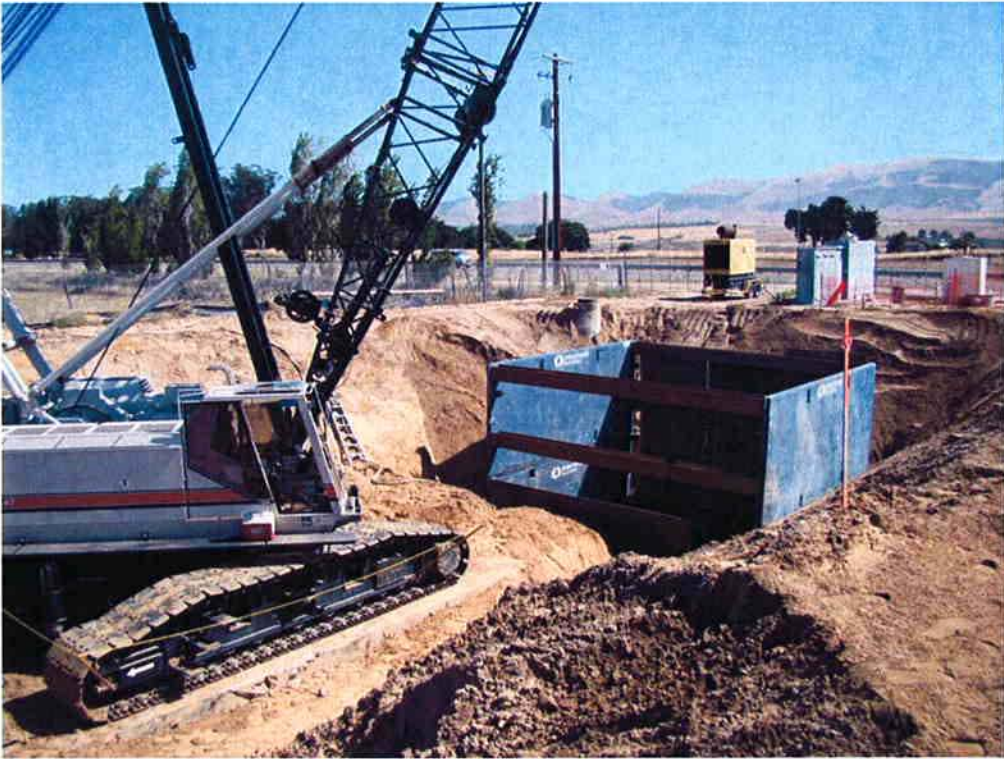
Installing second level of shoring.
