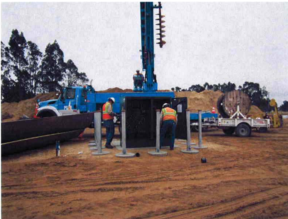
PG&E setting new transformer.
