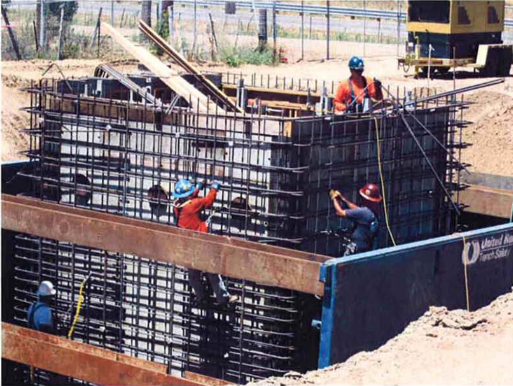
Installing rebar for walls.
