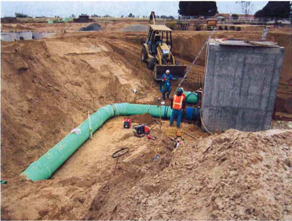
Connecting the 24" SE2 piping to the Process Water Pump Station.
