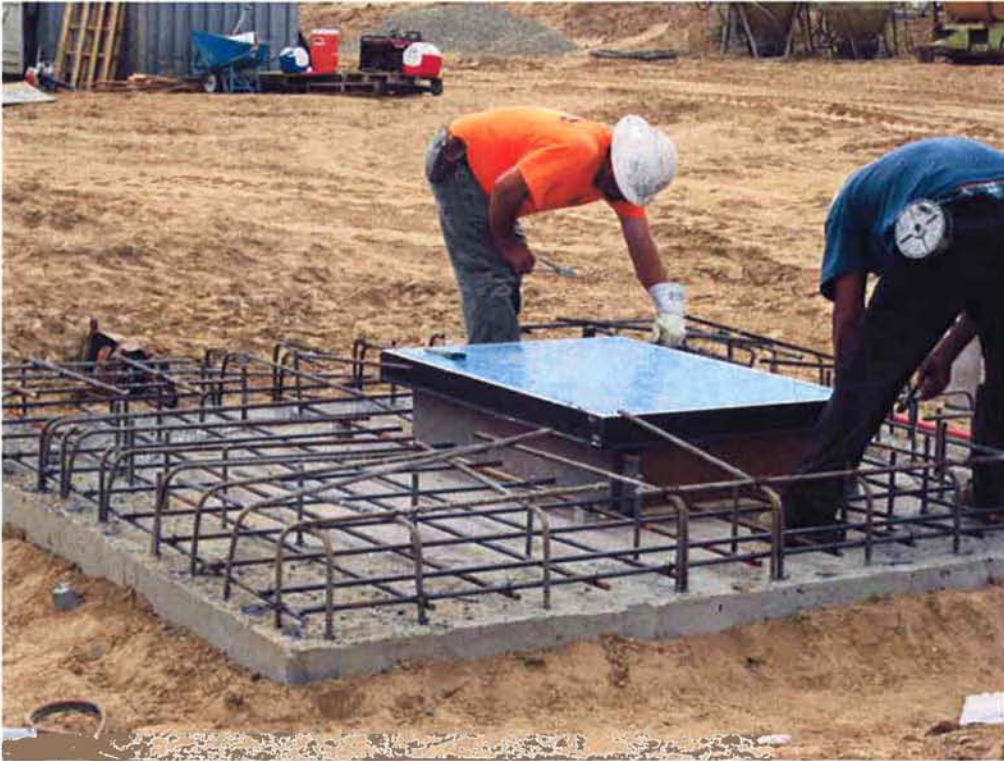
Cushman installing the hatch on the top of the Scum Well.
