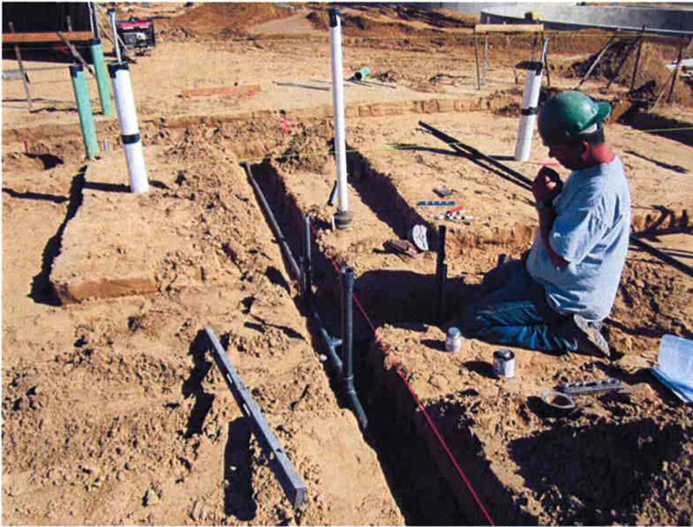
Cushman installing the under slab plumbing for the Sodium Hypochlorite Storage building.
