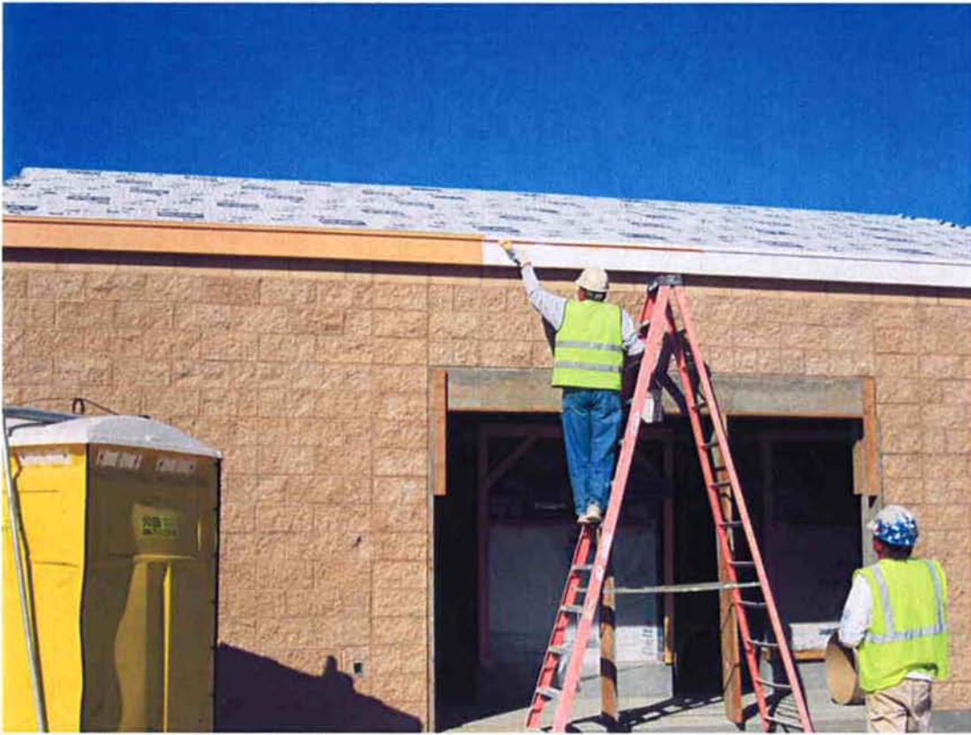
KNK Coating painting fascia.
