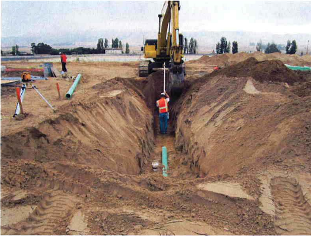
Excavating for the 6" DR pipe.
