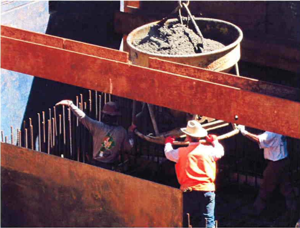
Pouring concrete for the slab.
