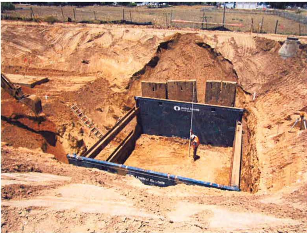
Installing first level of shoring.
