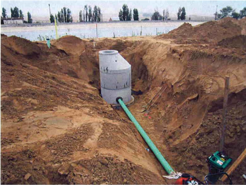
Manhole #6 installed with 6" DR piping to Manhole #7.
