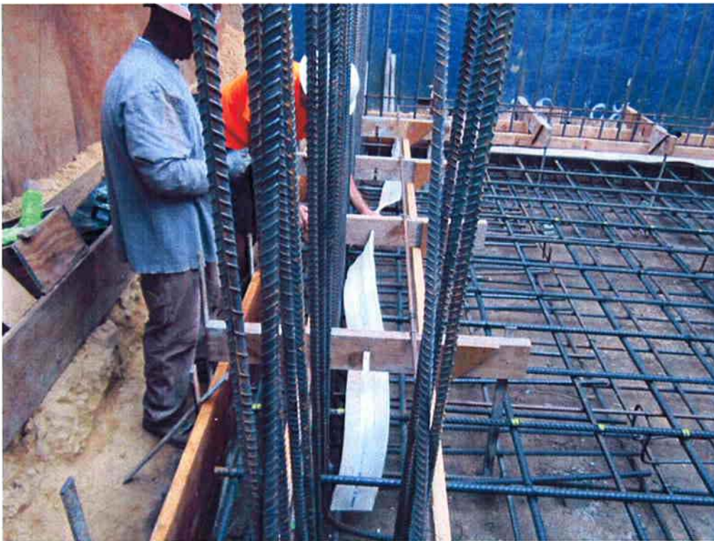
Installing water stop at base of wall and slab.
