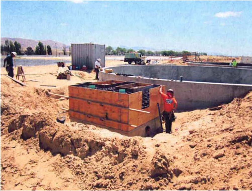
Forming the top of RAS/WAS Pump Station #2.
