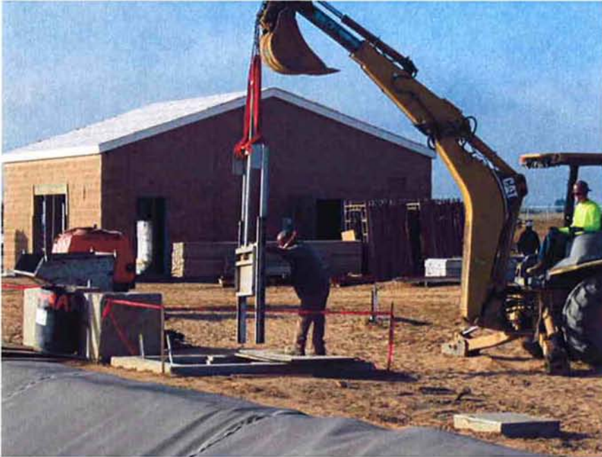
Cushman installing the weir gate at the Weir Box for Aeration Basin #1.
