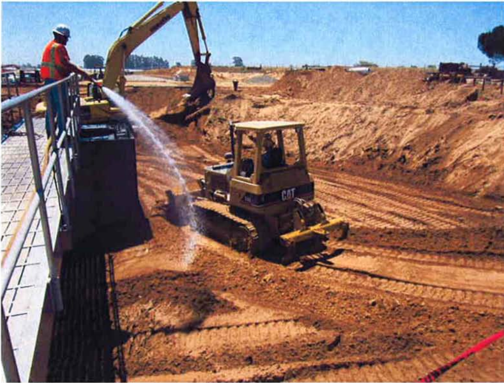
Backfilling around the Scum Well.
