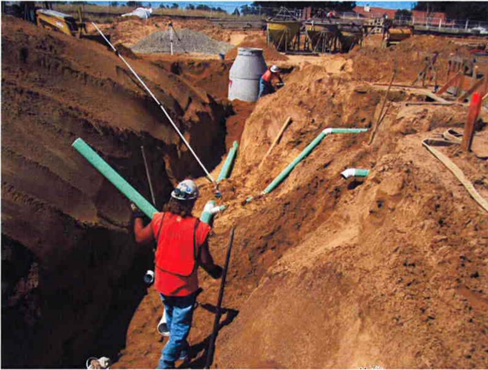
Cushman installing the 6" DR piping from Manhole #7 and connecting to the Sodium Hypochlorite Storage building drains.
