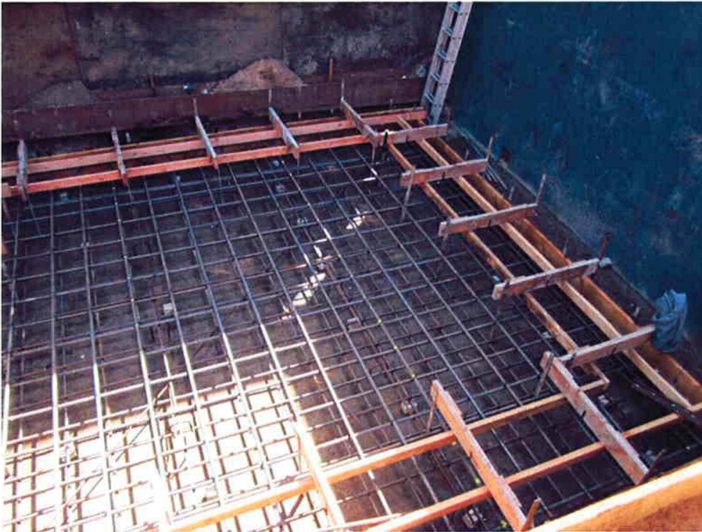
Forms and reinforcing for the slab.
