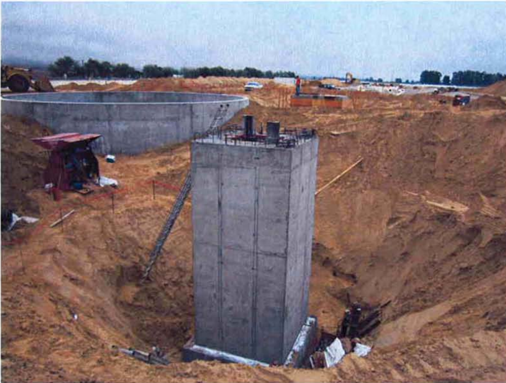
Scum Well wall forms removed.
