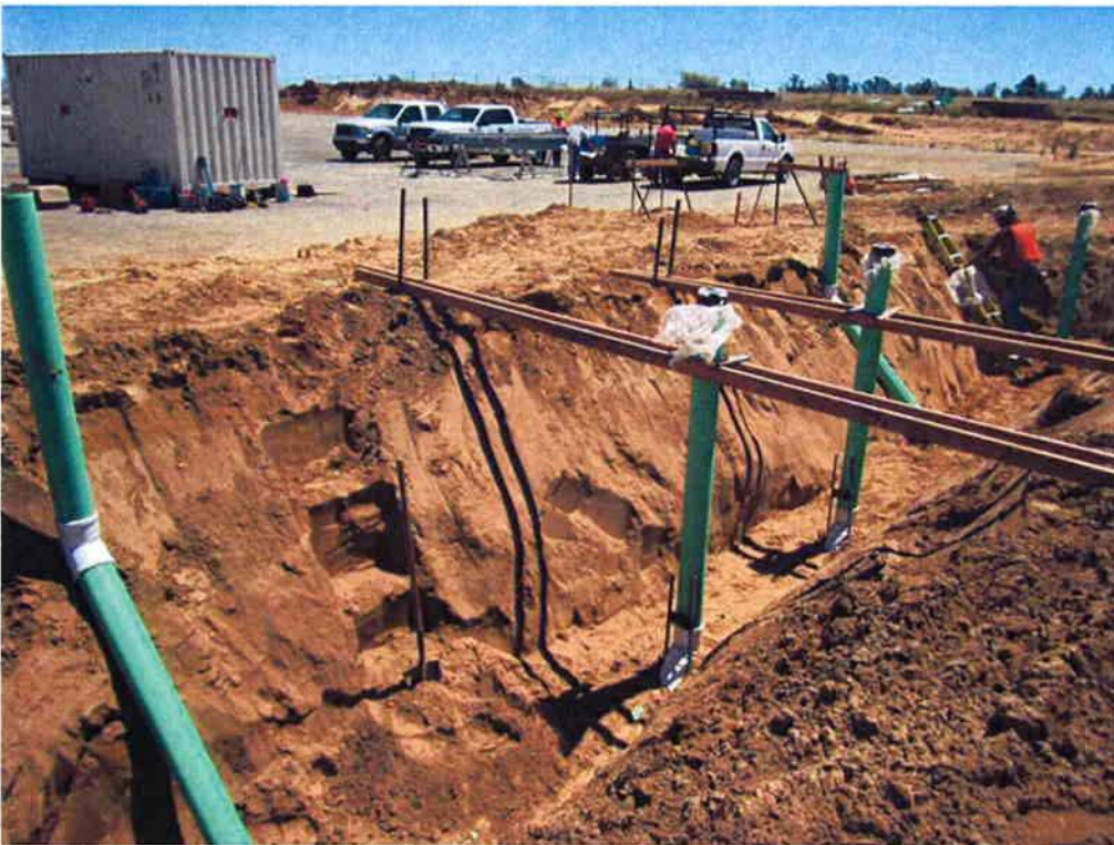
Installation of 6" DR piping from Manhole #6 to the Sludge Thickening Building.
