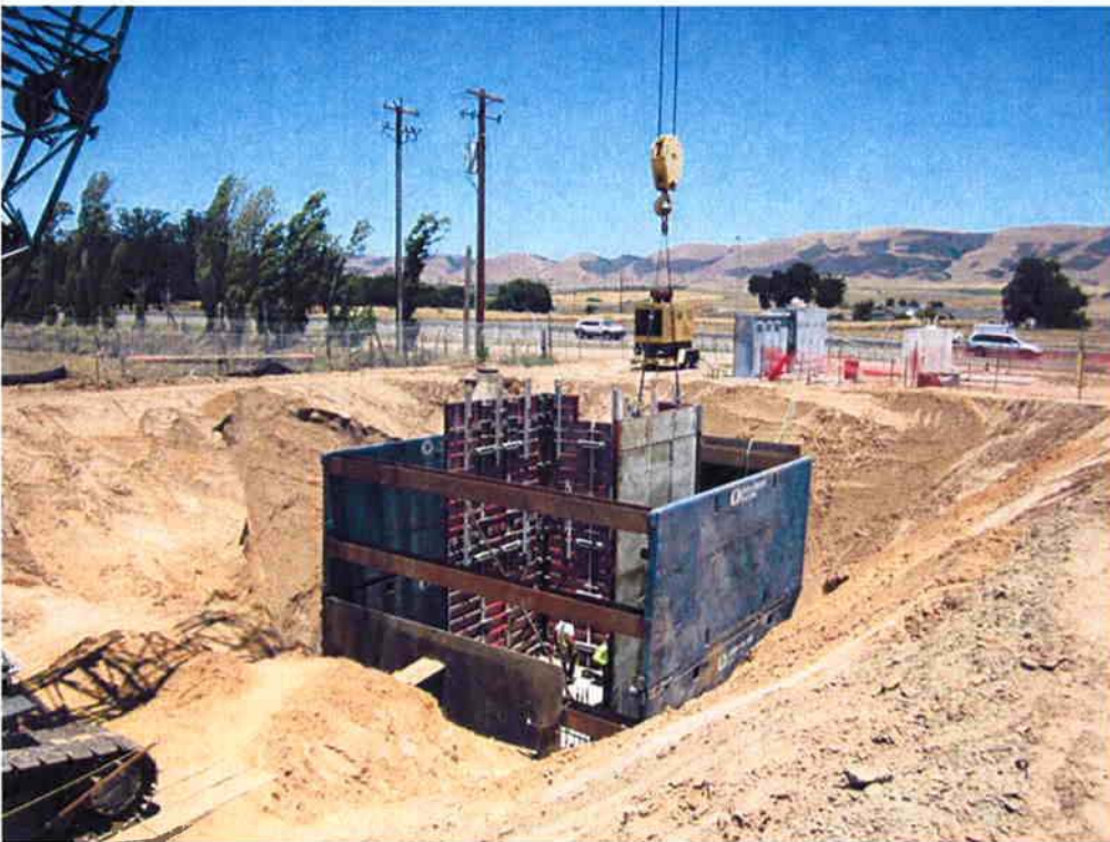
Installing interior wall forms.
