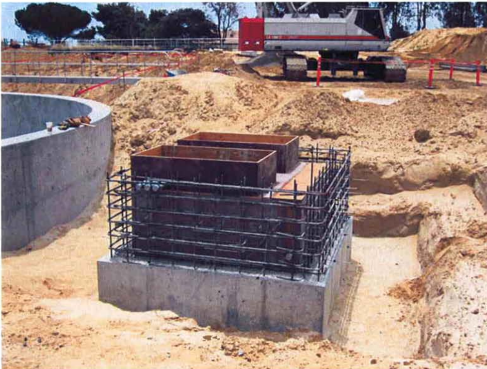
Forming the top of RAS/WAS Pump Station #2.
