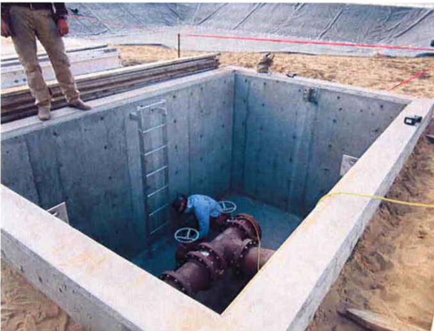
Cushman installing the access ladder inside the Air Meter Vault.
