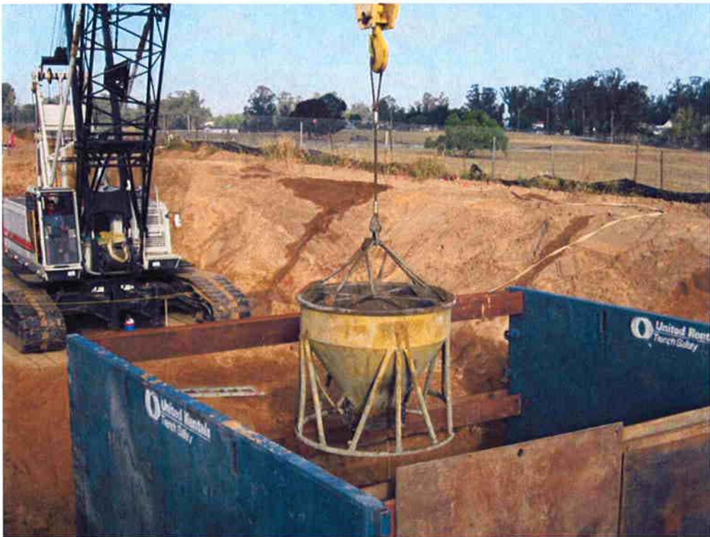
Installing base material.
