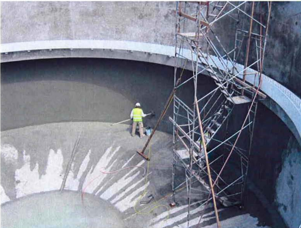
KNK Coating applying Xypex to interior of Clarifier #1.
