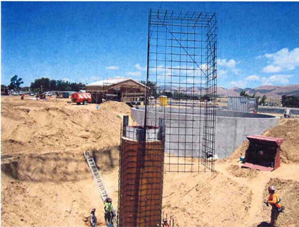
Installing reinforcing for the walls at the Scum Well.
