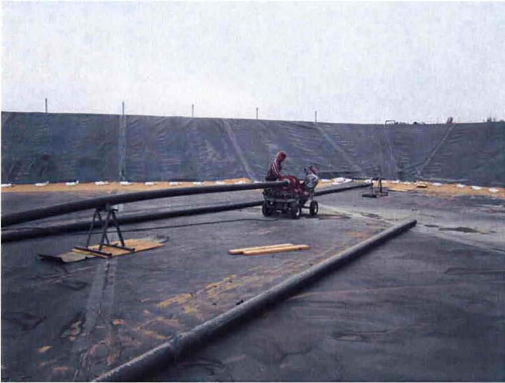
Cushman heat welding HDPE pipe for biofilters.
