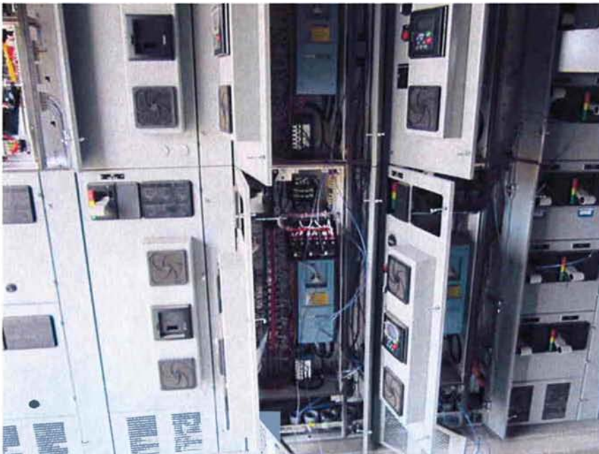
Bergelectric pulling wires inside MCC panels.
