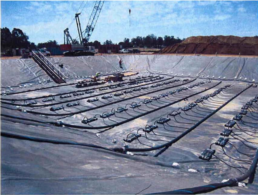
Biofusers assembled and wrapped with plastic for protection.
