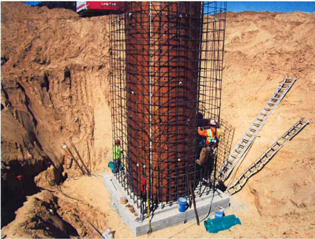
Tying reinforcing for the walls at the Scum Well.
