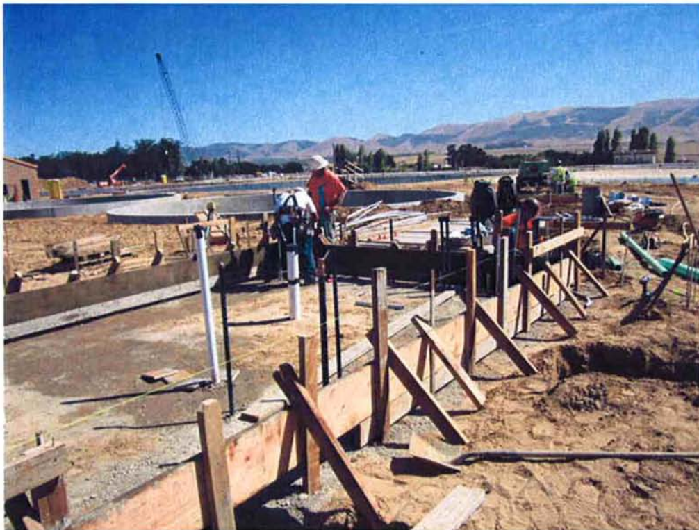
Cushman preparing forms for the Sodium Hypochlorite Storage building foundation.
