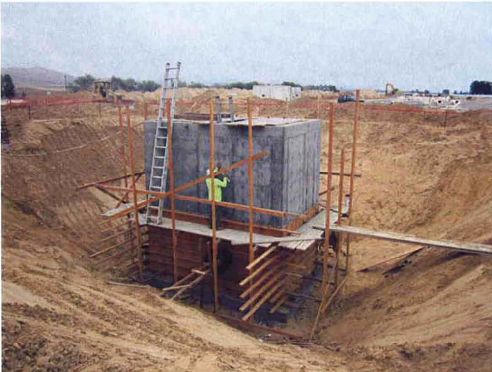
Removing wall forms from the Process Water Pump Station.
