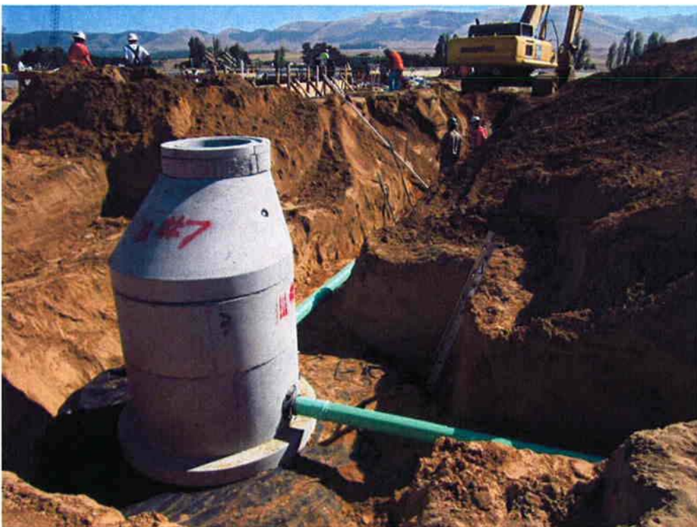
Cushman installing Manhole #7 and 6" DR piping.
