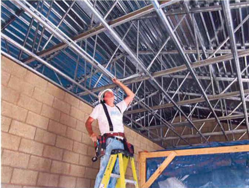
Bergelectric installing lighting conduit.
