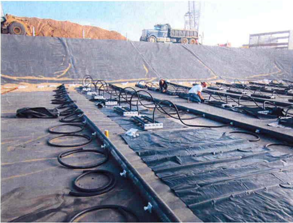
Cushman assembling the biofusers for the Biolac System.
