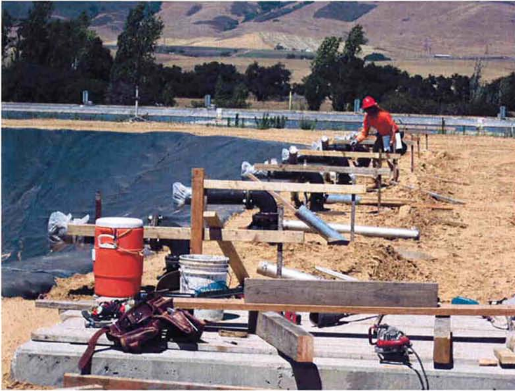
Installing anchor posts for the biofusers.
