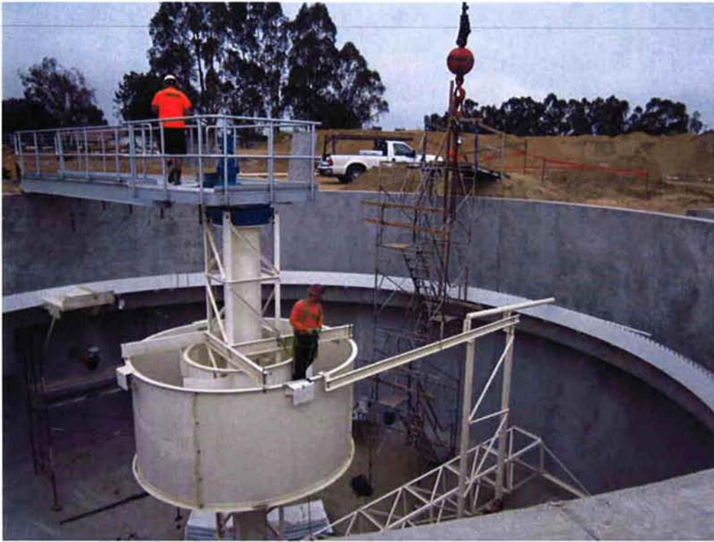
Installing mechanisms inside Clarifier #2.
