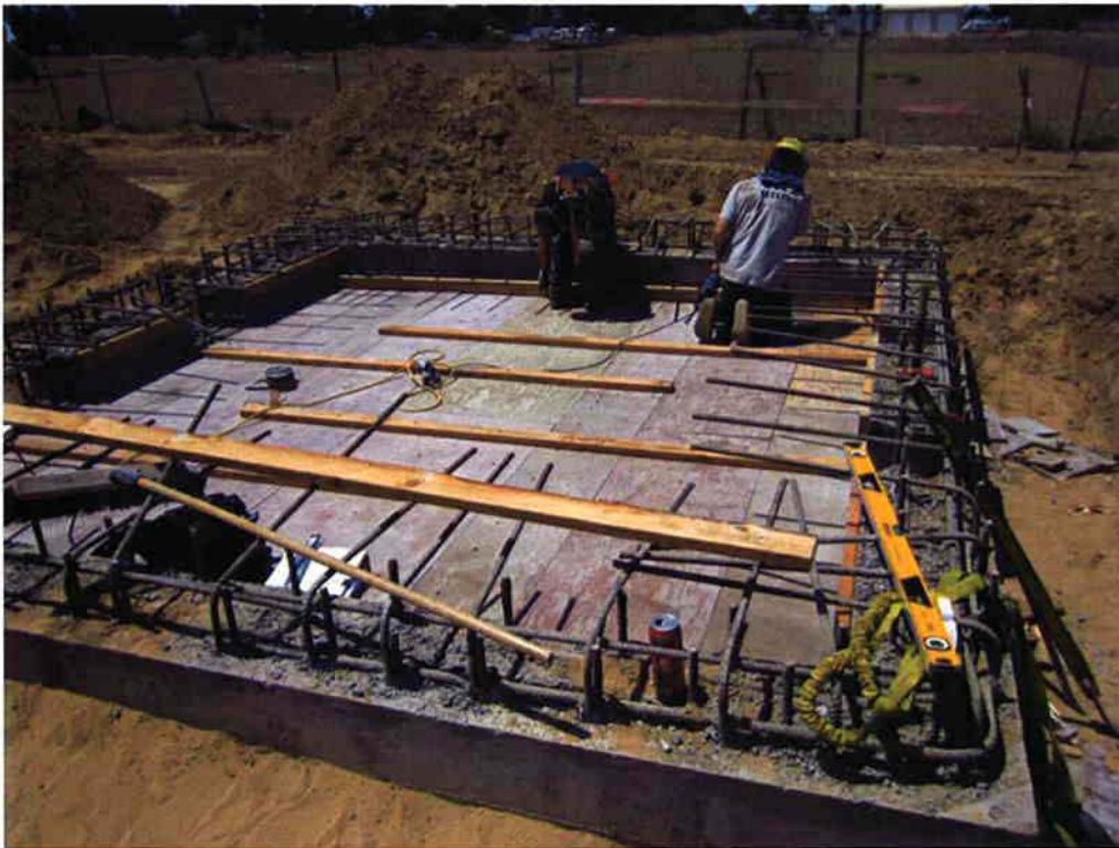
Setting shoring for pouring the deck of the Influent Pump Station.
