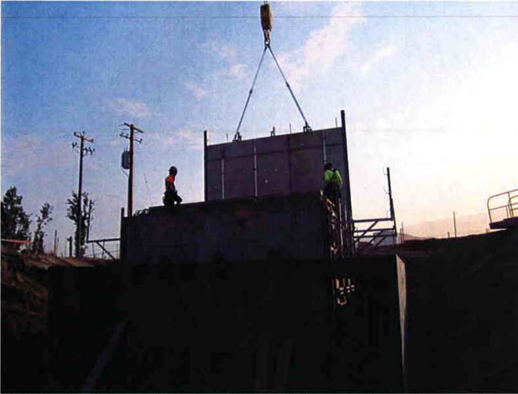
Stripping the forms at the Influent Pump Station after the wall pour.
