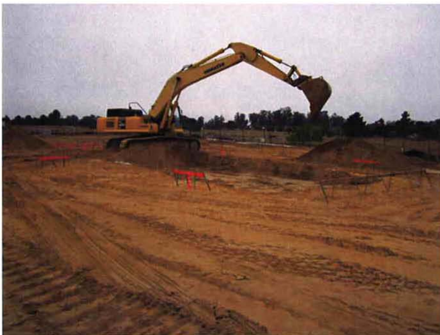
Excavating for headworks and grit removal system.
