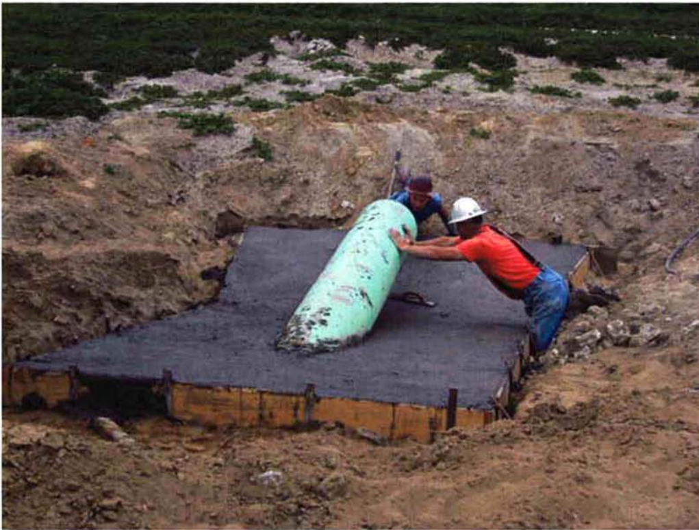
Pouring the inlet structure slab at Pond 1.
