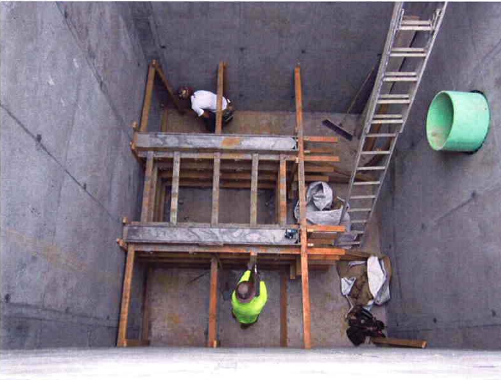
Stripping forms from the walls dividing the prerotation basins.
