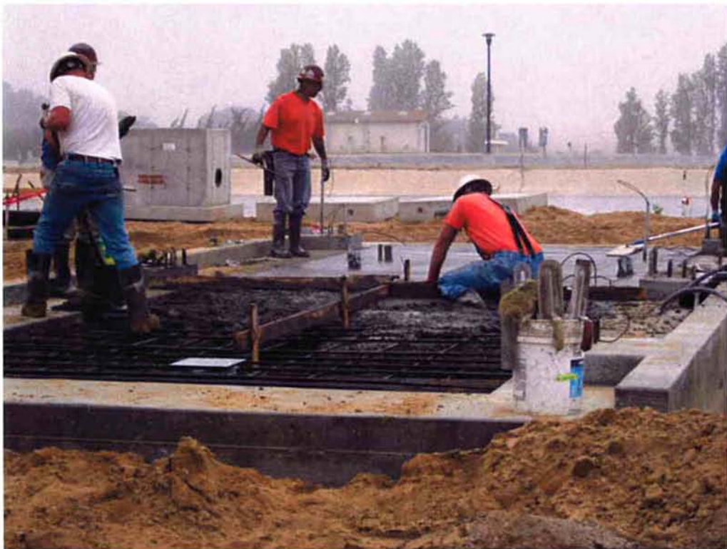
Cushman pouring concrete for Sludge Thickening slab.
