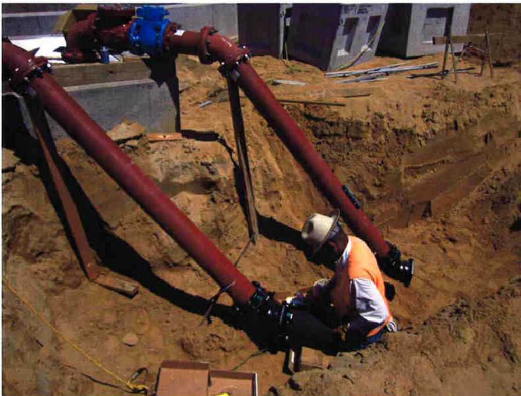
Cushman installing below ground piping at RAS/WAS Pump Station #1.
