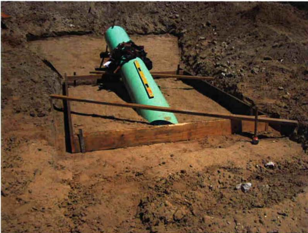
Forming for the 18-inch pipe inlet structure slab at Pond 1.
