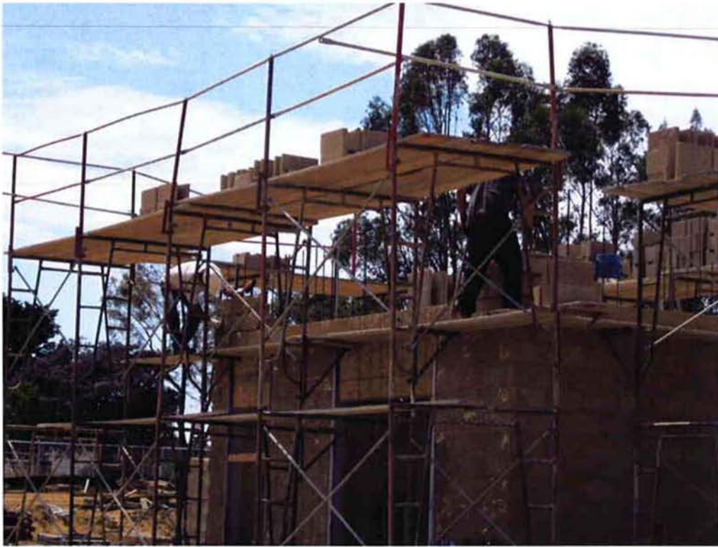
Building corner leads at the Sodium Hypochlorite Building.
