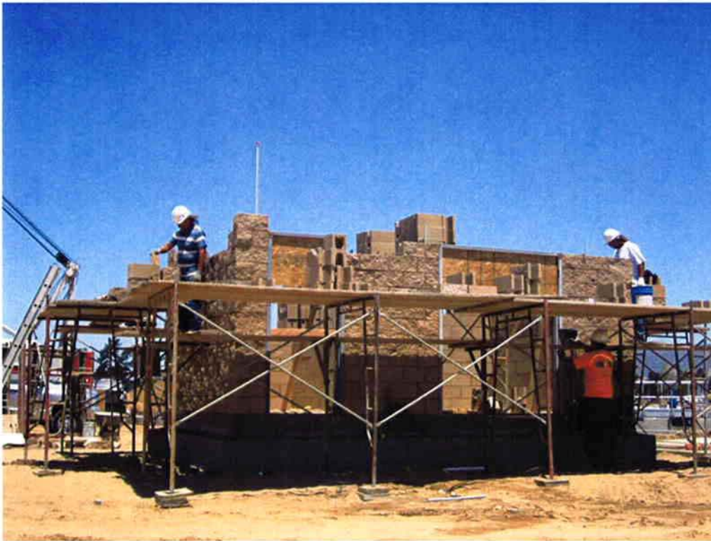
Beinscroth Masonry placing CMU at Sodium Hypochlorite Building.
