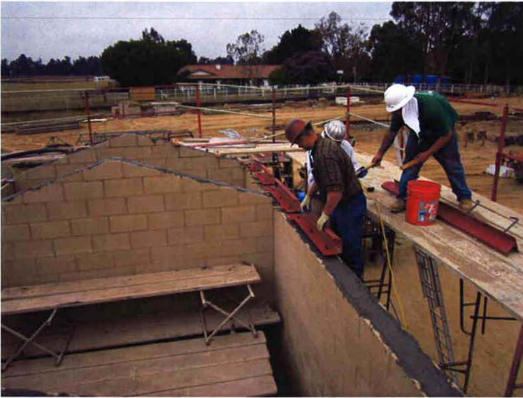
Cushman setting steel channels at Sodium Hypochlorite Building.
