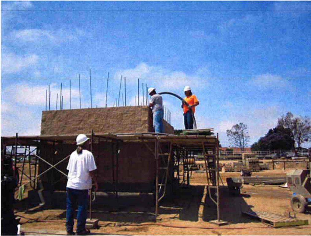
Installing reinforcing and pouring grout at the Sodium Hypochlorite Building.
