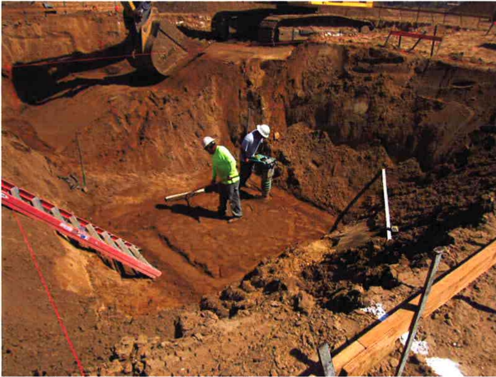
Excavating for the headworks and grit removal system.
