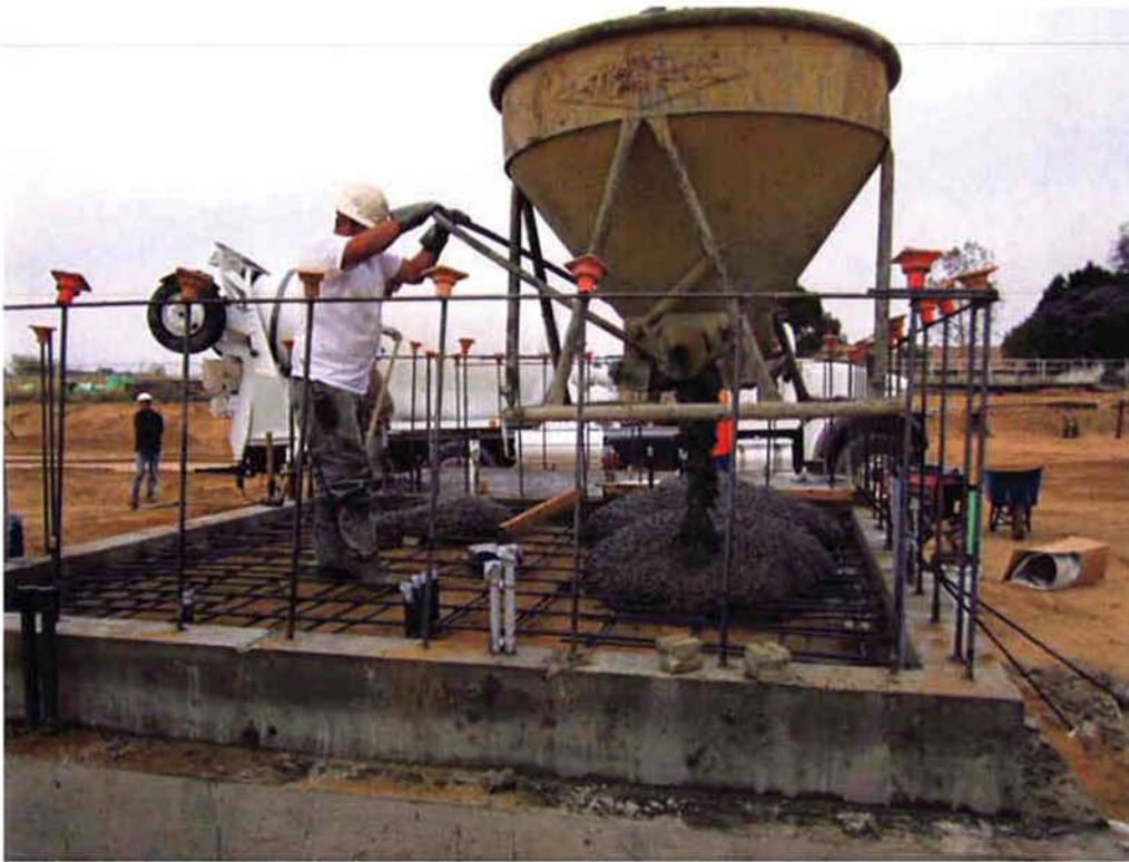
Pouring slab of the Sodium Hypochlorite Building.
