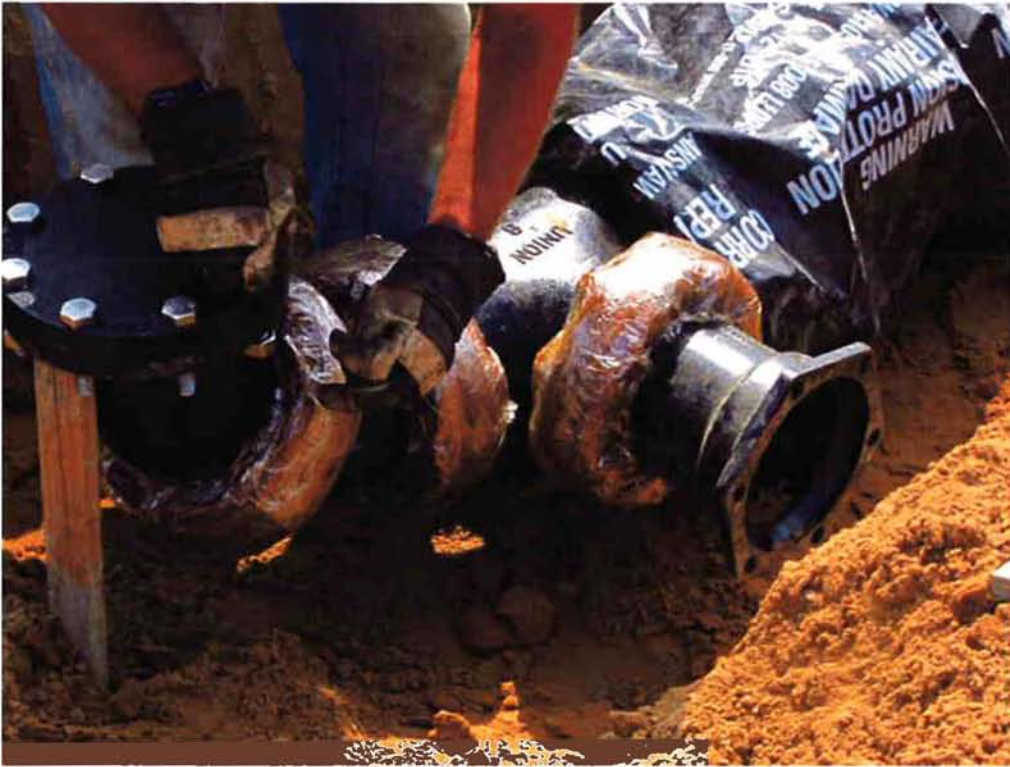
Cushman installing fittings on the 6-inch TWAS pipe.
