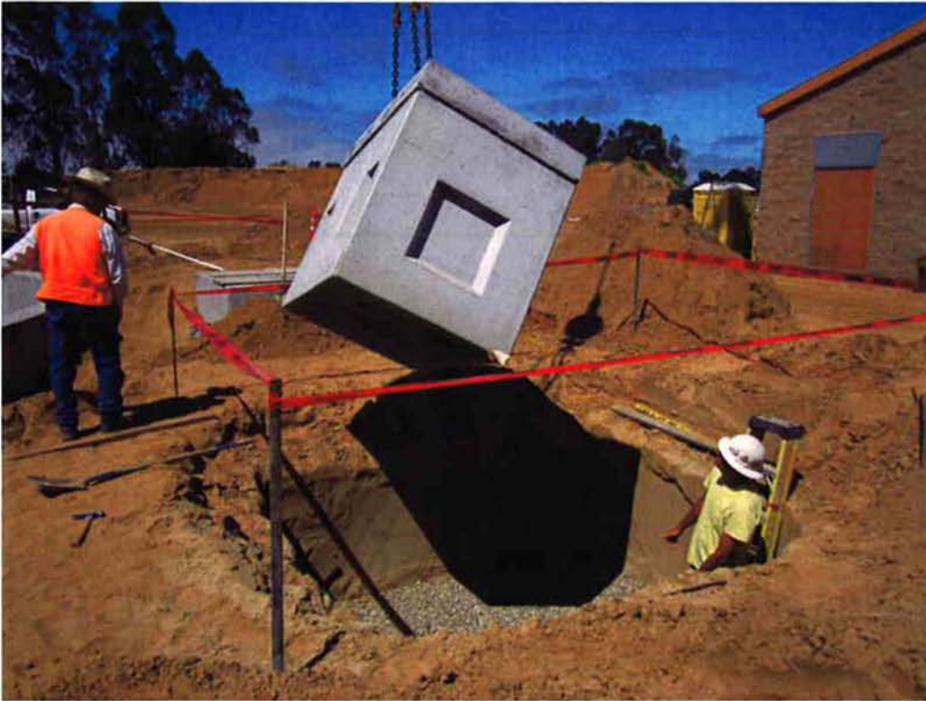
Bergelectric and Cushman installing Pull Box #25.
