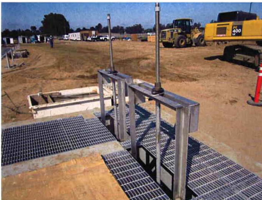
Weir gates and grating installed at Distribution Box #1.
