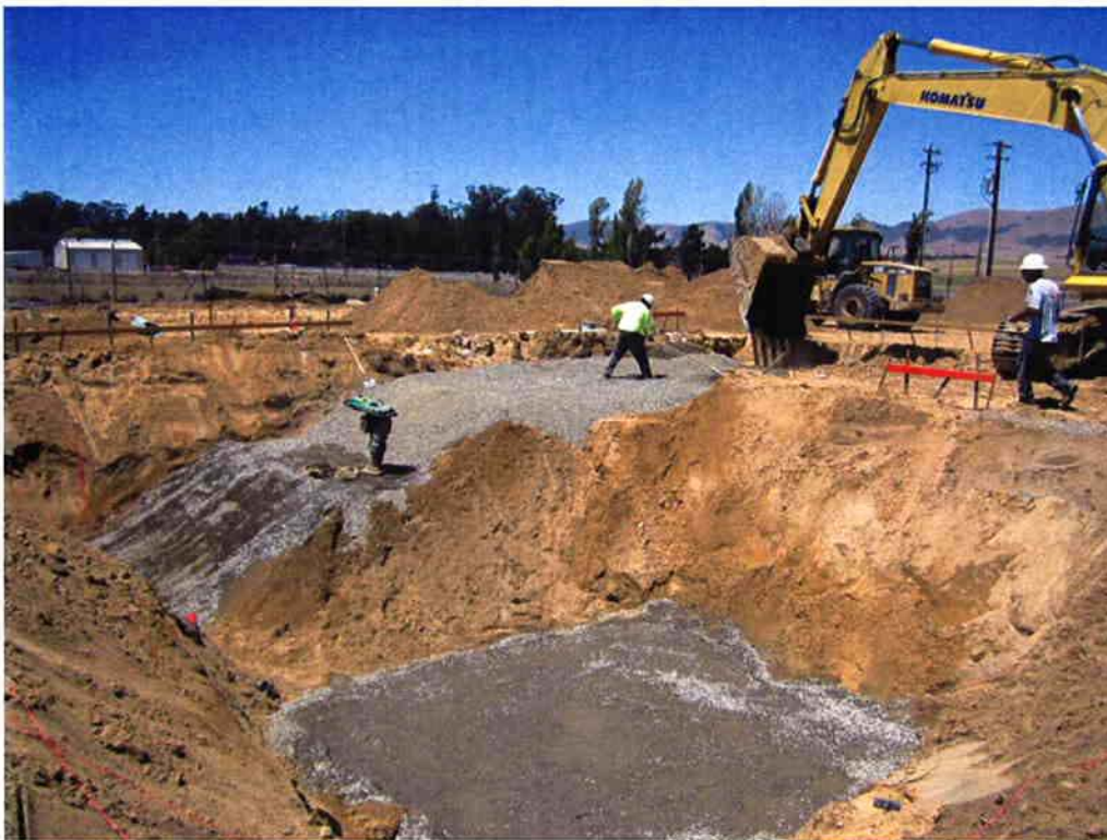
Placing and compacting base for headworks and grit removal system.
