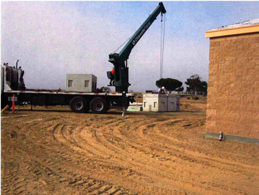
Bergelectric taking delivery of electrical pull box vaults.
