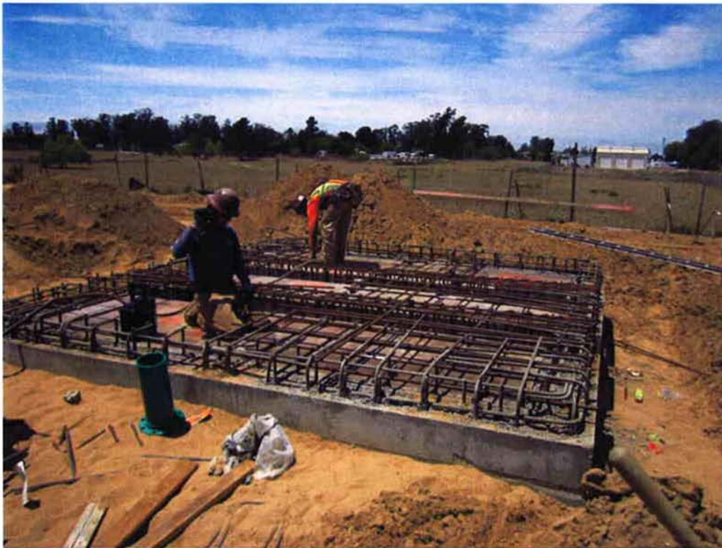
Installing the reinforcing for the Influent Pump Station deck.
