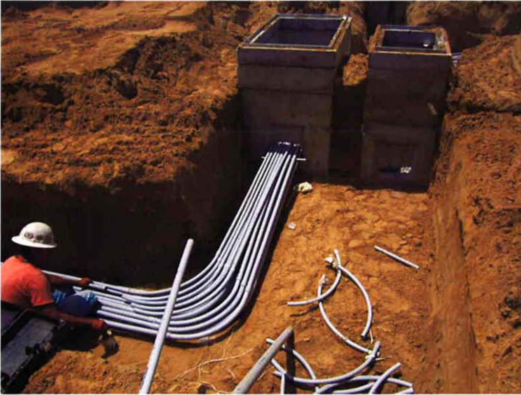
Bergelectric installing Duct Bank #22.
