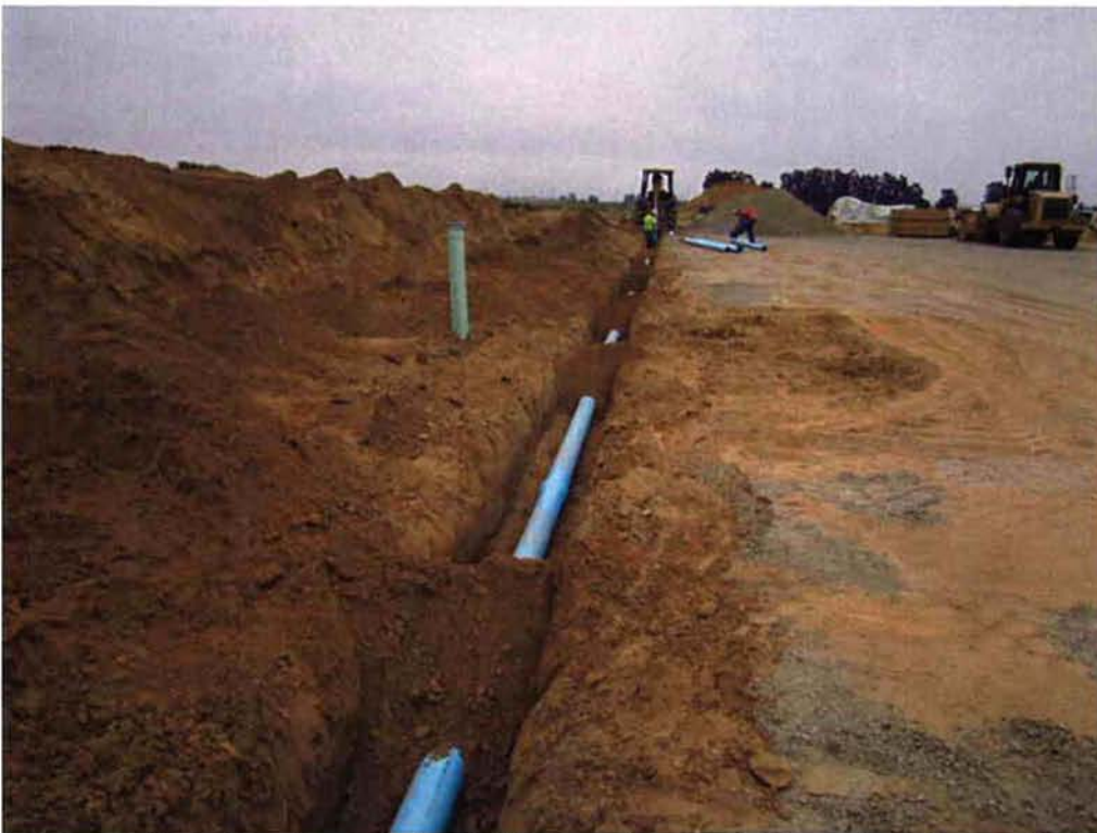
Cushman installing the 6-inch NPW along the east side of the Sludge Drying Beds.
