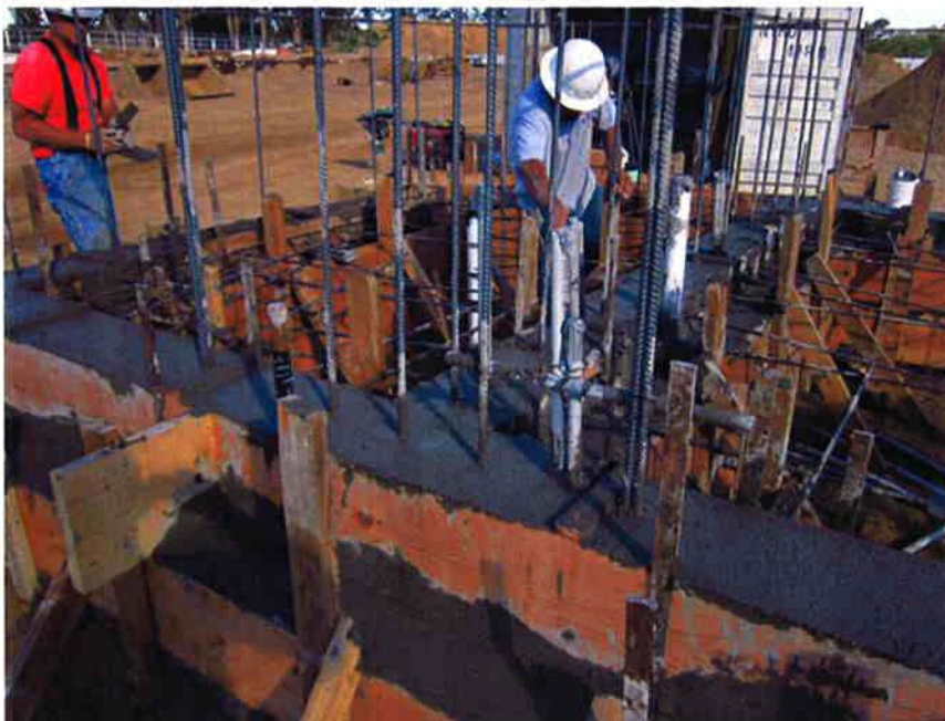
Cushman pouring concrete for the starter wall at the Sodium Hypochlorite Building.
