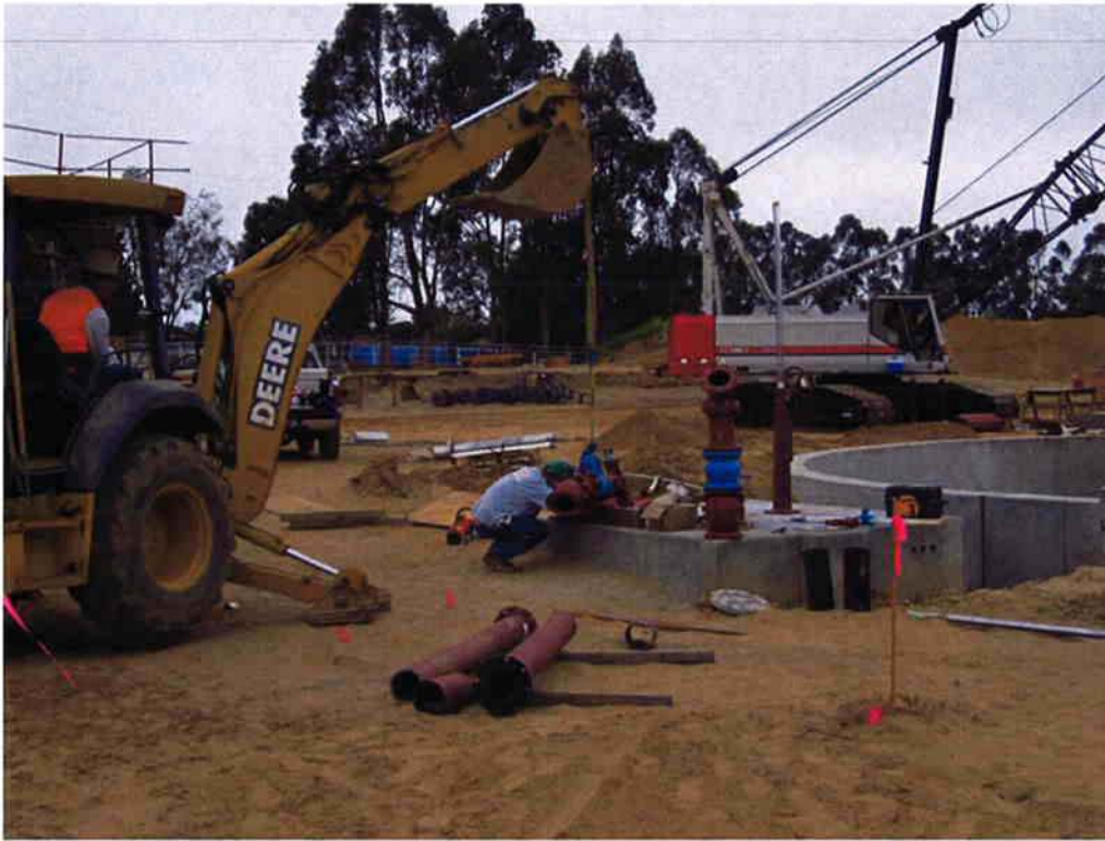
Cushman installing piping at RAS/WAS Pump Station #1.
