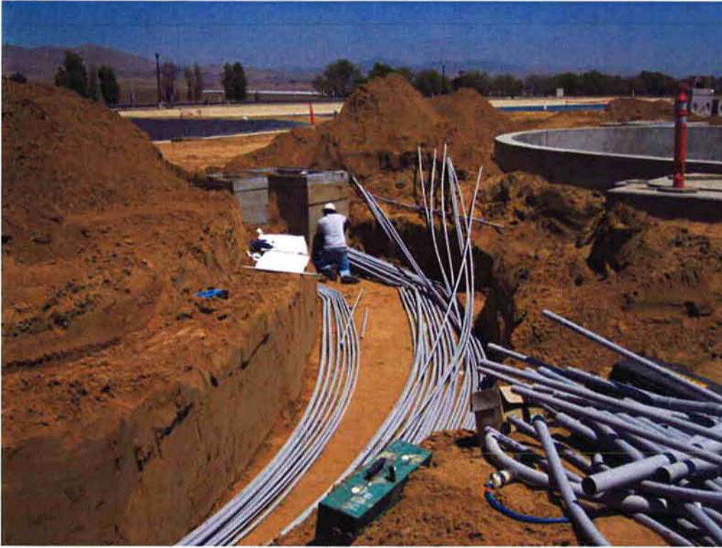
Bergelectric installing Duct Bank #25 into Pull Box #25.
