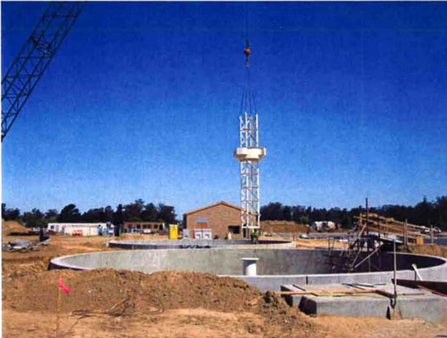
Installing mechanisms inside Clarifier #1.
