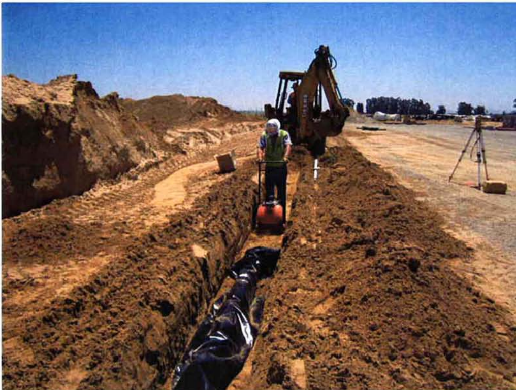
Cushman installing the 6-inch TWAS to the east of the Sludge Drying Beds.
