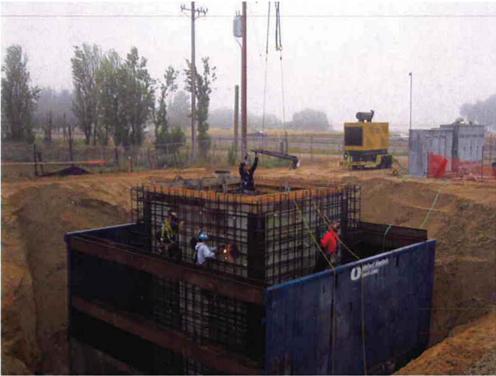
CMC Rebar tying wall reinforcing at the Influent Pump Station.
