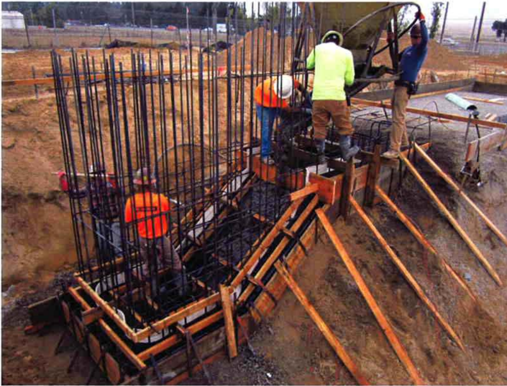
Pouring concrete for lower section of the headworks foundation.
