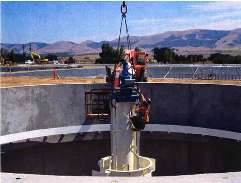
Installing motor for mechanisms inside Clarifier #2.
