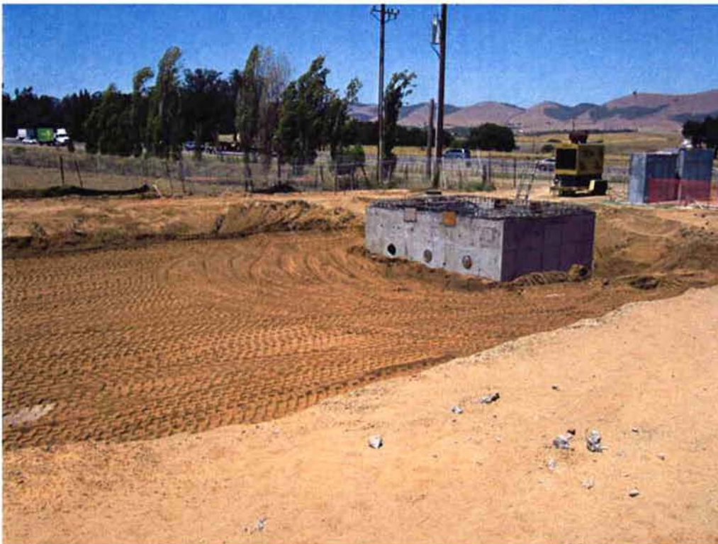
Backfilling around Influent Pump Station.
