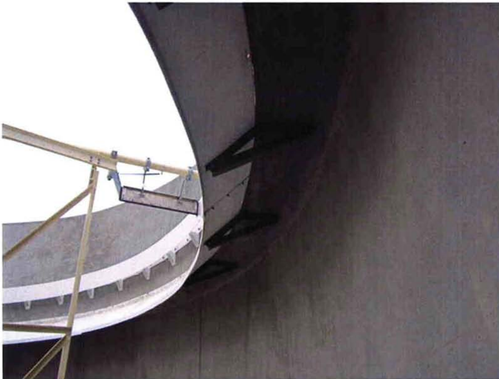
Installing the peripheral baffle inside Clarifier #2.
