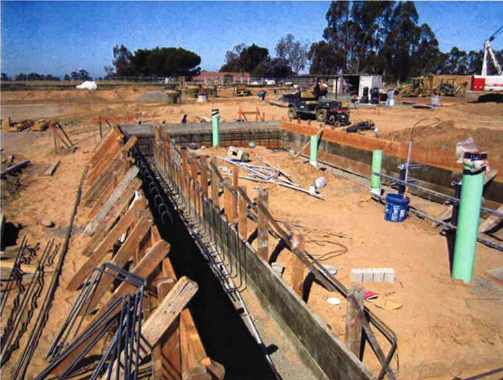
Reinforcement installation for the Sludge Thickening System footing.
