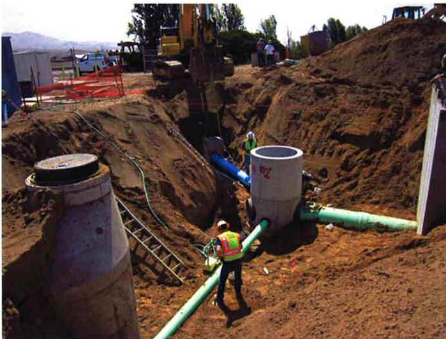
Cushman installing Manhole #1 and piping.
