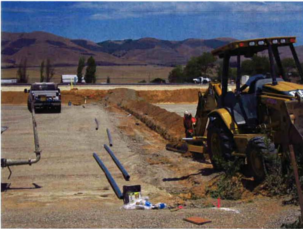
Cushman installing 3-inch NPW line between the Sludge Drying Beds.
