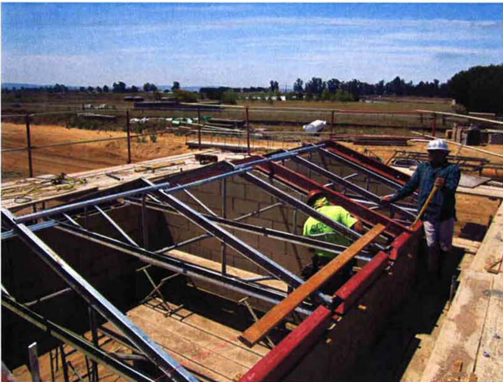
Cushman installing the metal roof trusses at the Sodium Hypochlorite Building.
