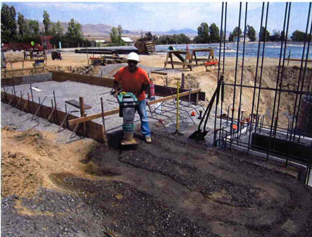
Compacting base under the upper headworks.
