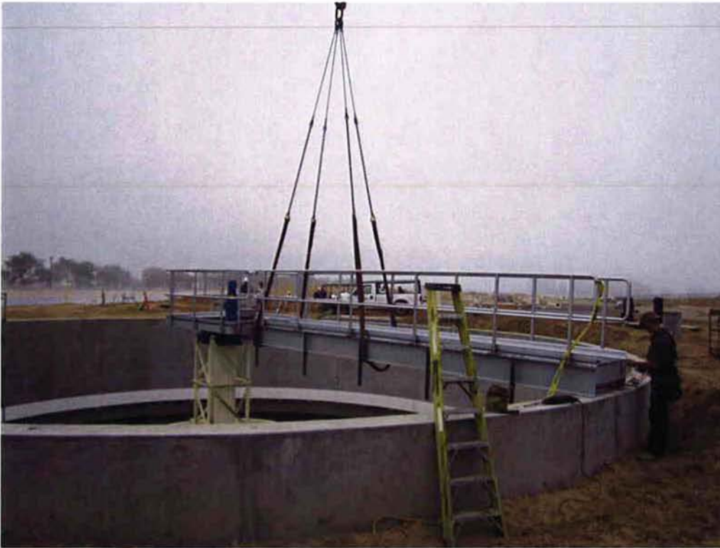
Installing the bridge for Clarifier #1.
