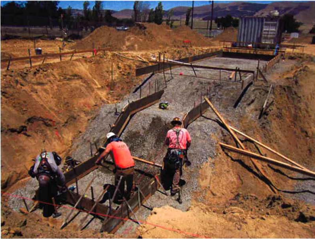
Forming lower level of headworks.
