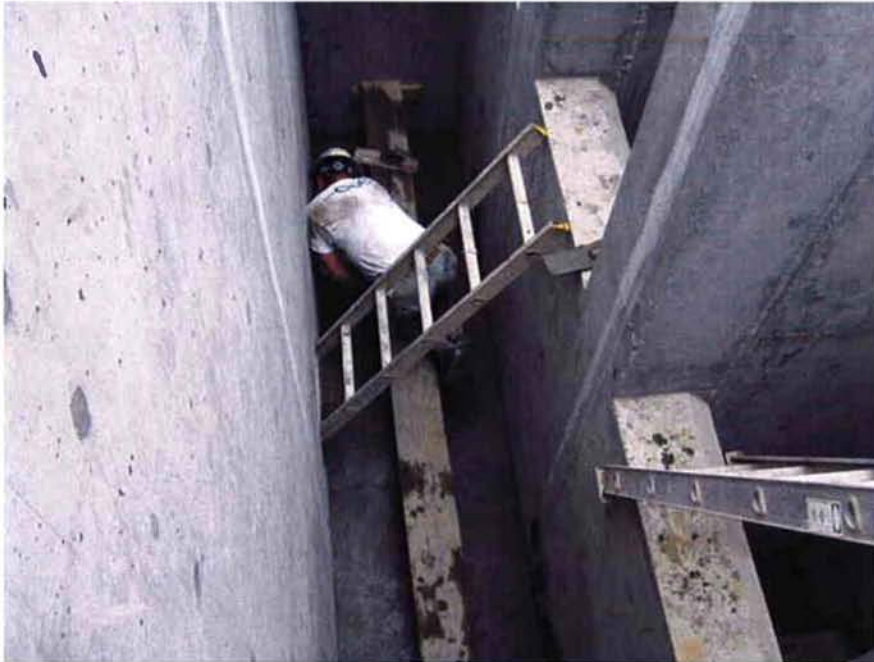
Cushman placing concrete fill inside Distribution Box #2.
