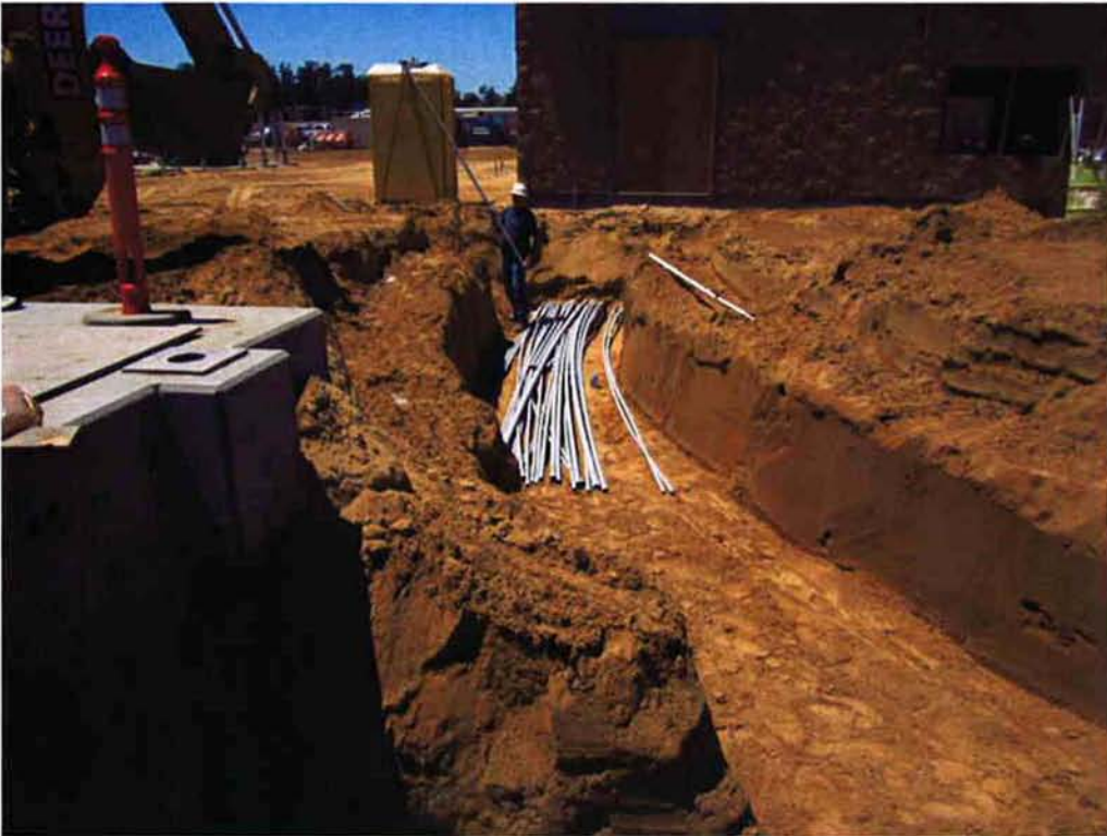
Bergelectric installing Duct Bank #25 from the Electrical/Blower Building.
