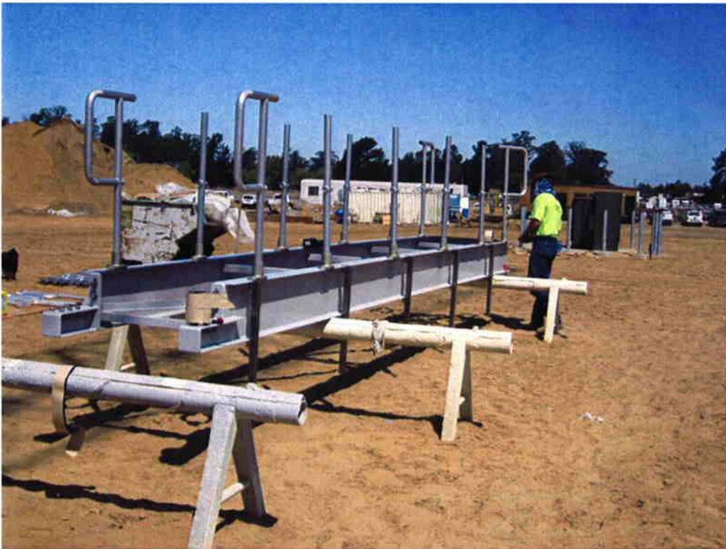
Assembling the metal bridge and handrail for the clarifiers.
