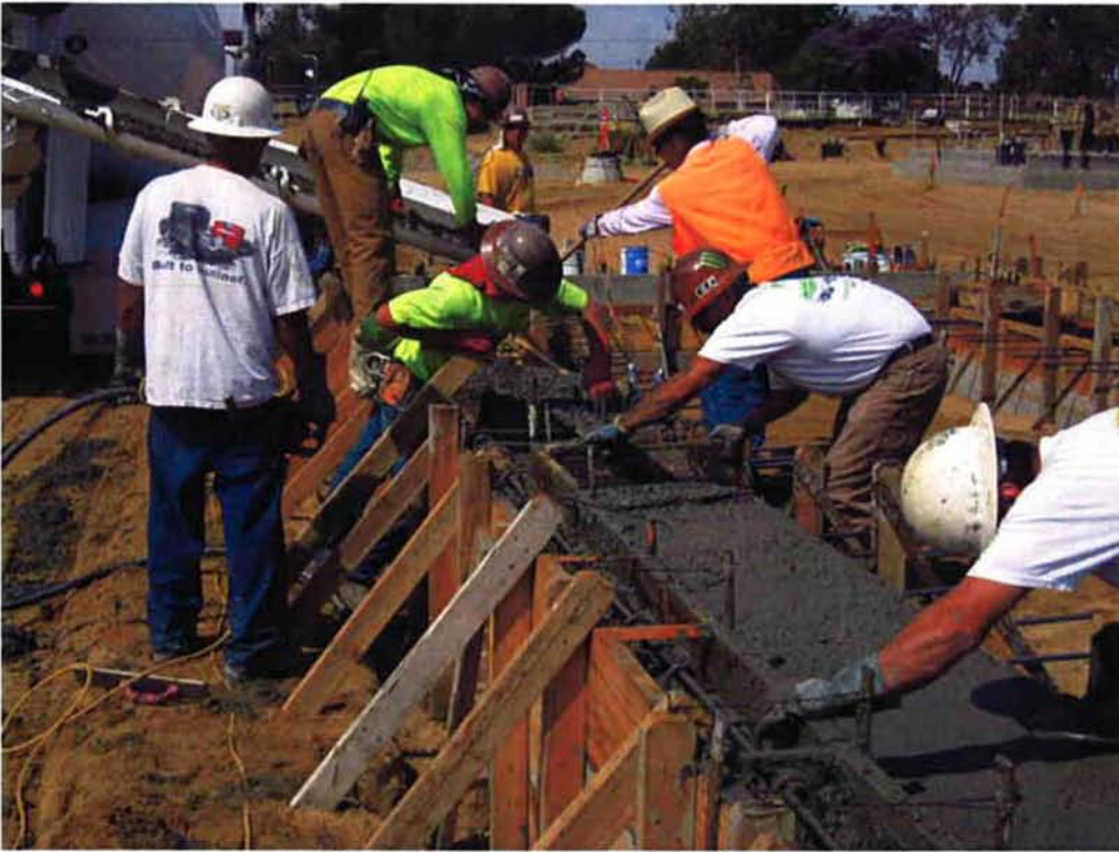
Cushman pouring the footing for the Sludge Thickening System.
