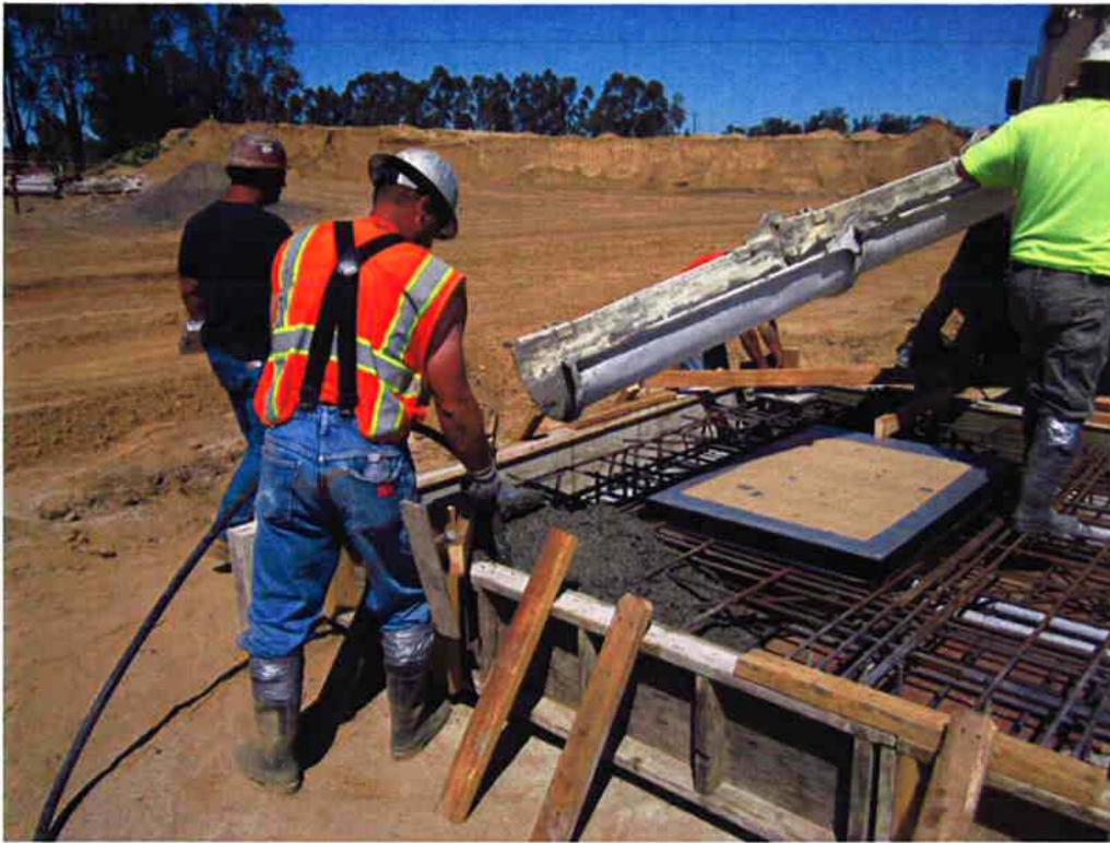
Cushman pouring concrete for the deck of the Scum Well.
