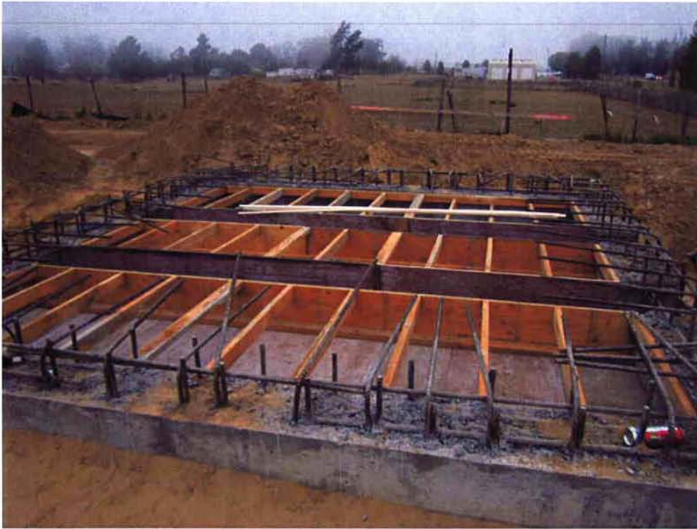
Forming deck of Influent Pump Station.
