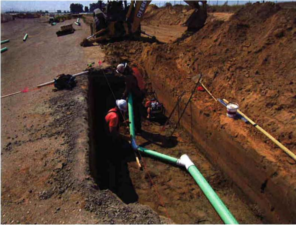
Cushman installing the 6-inch TWAS west of the Sludge Drying Beds.
