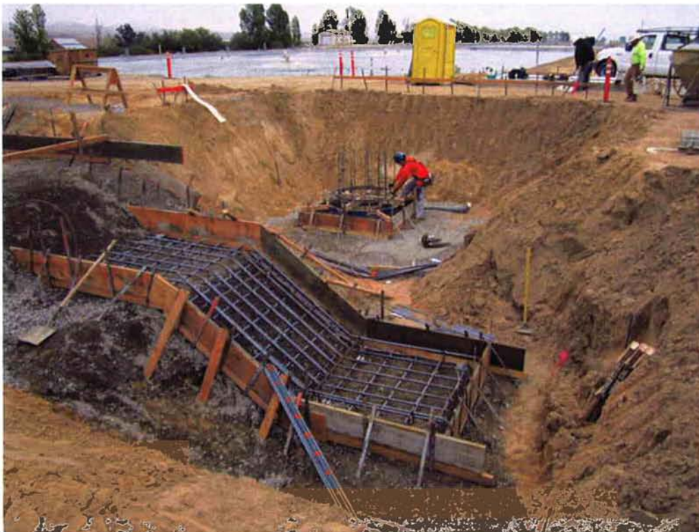
Reinforcing being installed at lower headworks and grit removal chamber.
