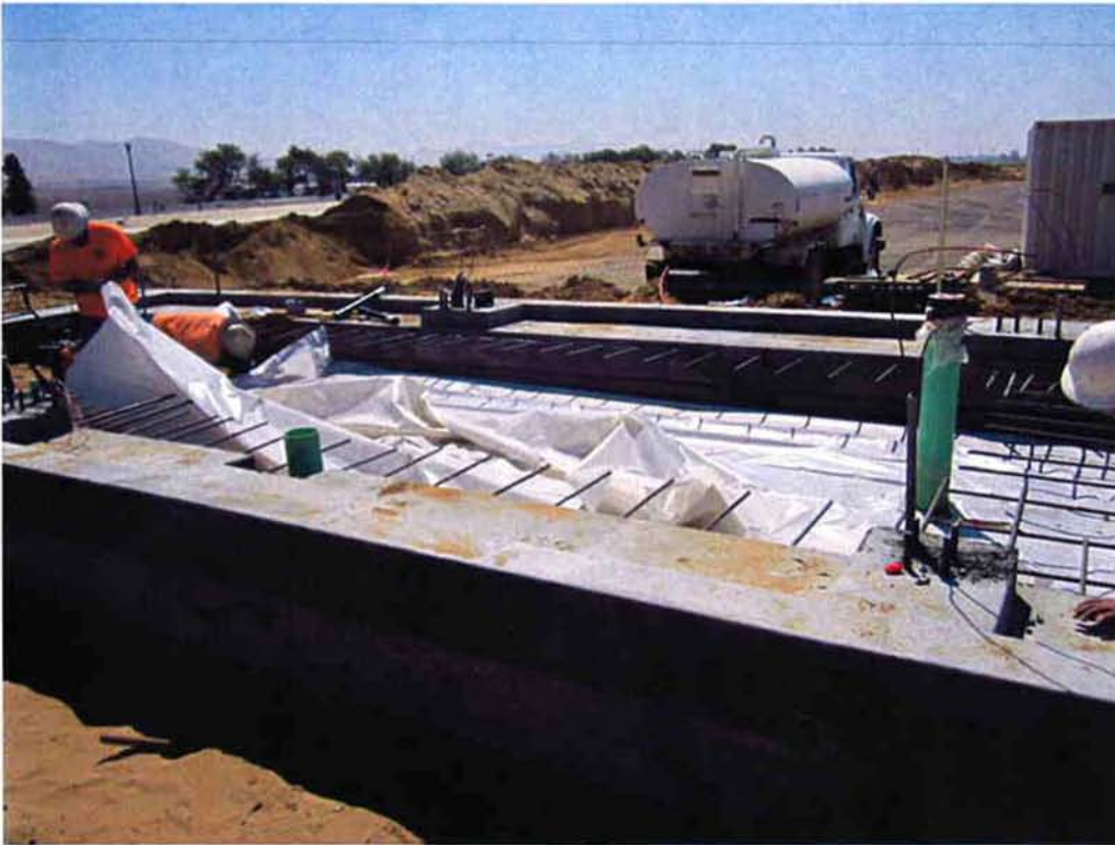
Installing the vapor barrier under the slab for the Sludge Thickening System.
