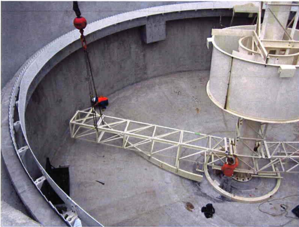
Installing mechanisms installed inside Clarifier #1.
