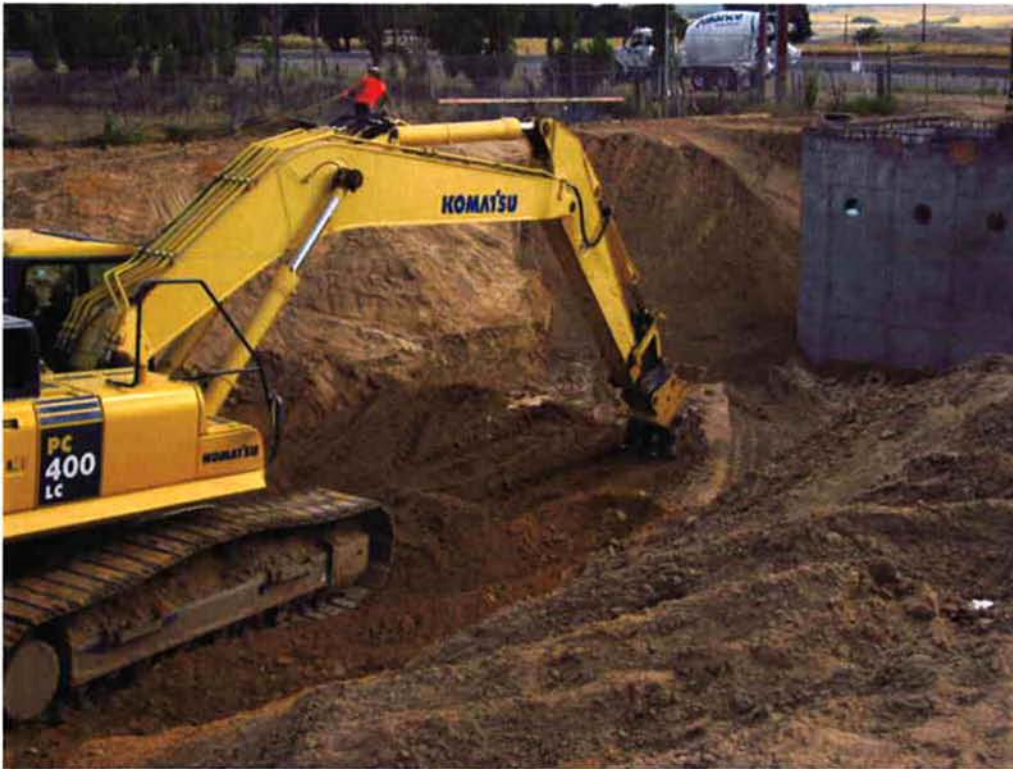
Backfill and compaction around the Influent Pump Station.
