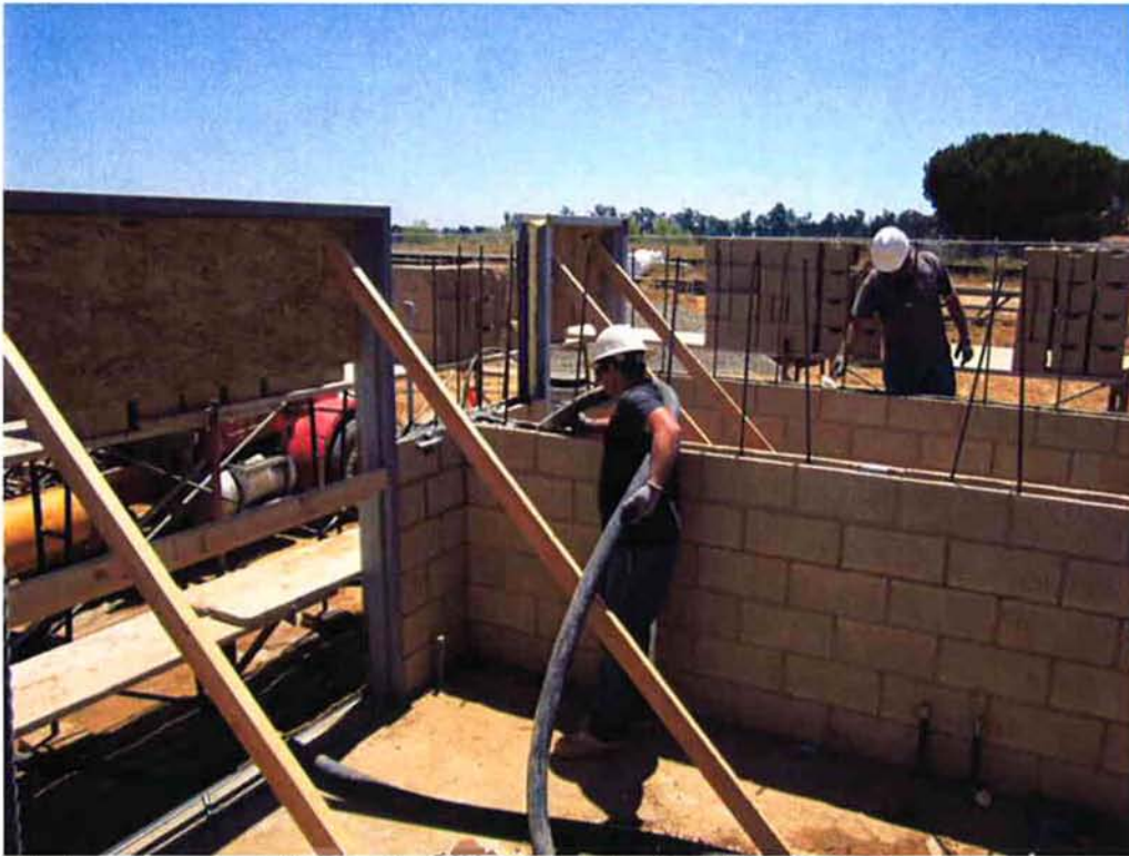
First grout pour at the Sodium Hypochlorite Building.
