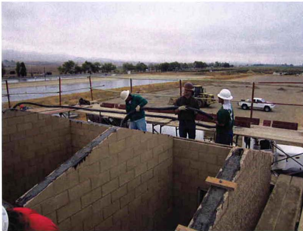
Last grout pour at Sodium Hypochlorite Building.
