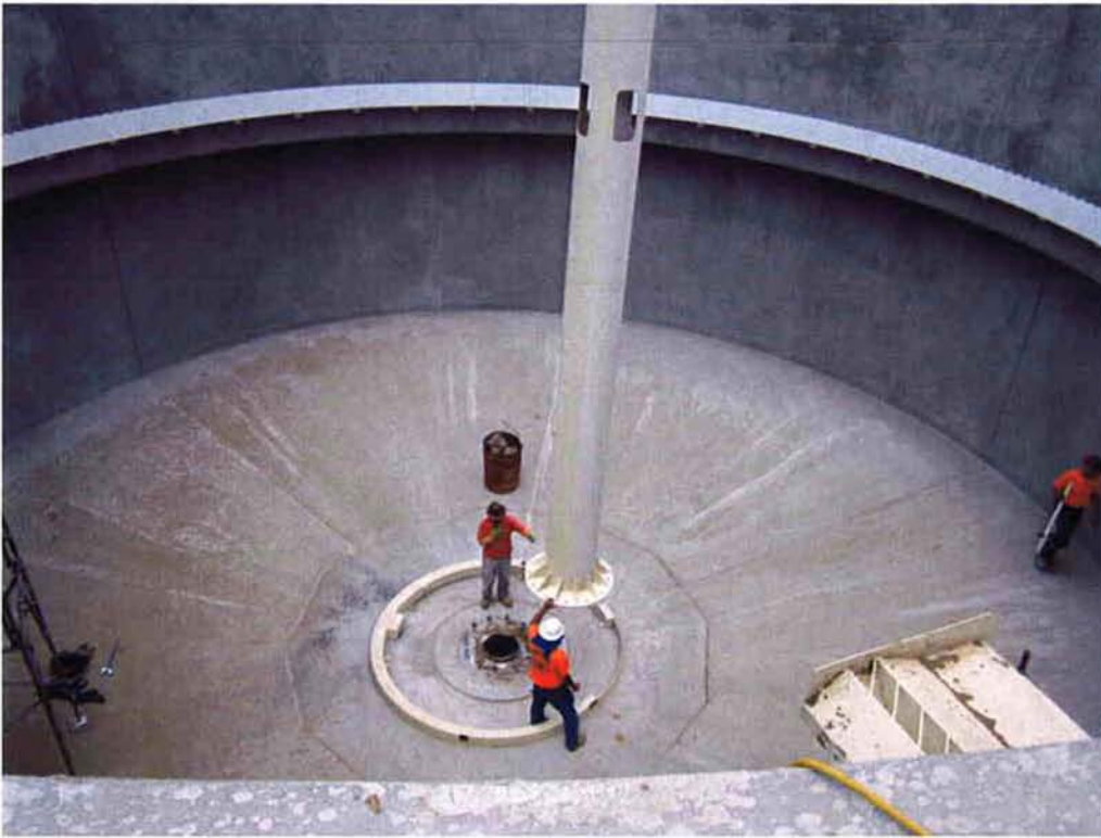
Installing center column inside Clarifier #2.
