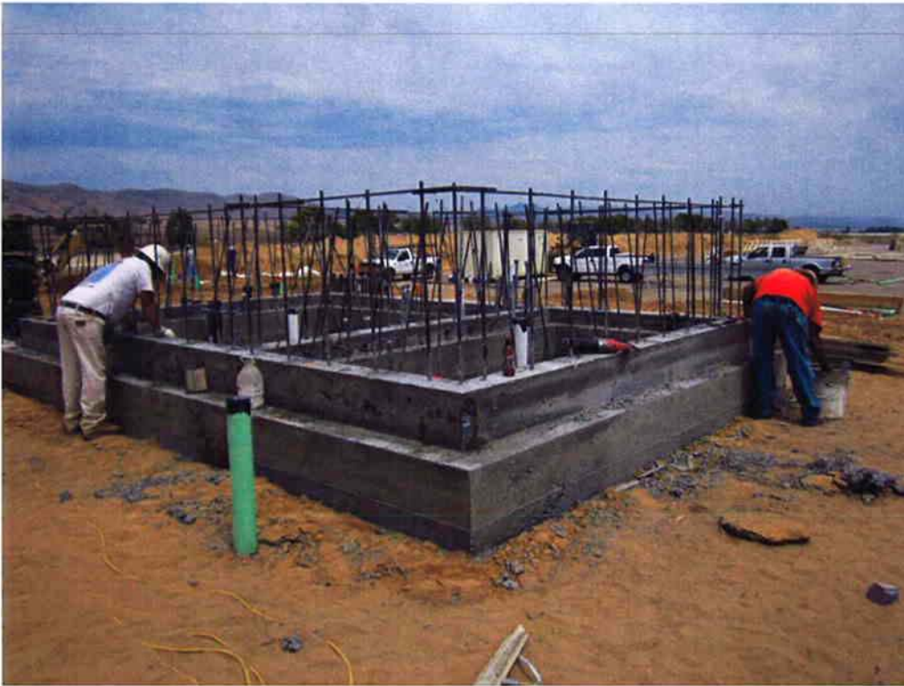
Cushman stripping forms from the concrete starter wall of the Sodium Hypochlorite Building.
