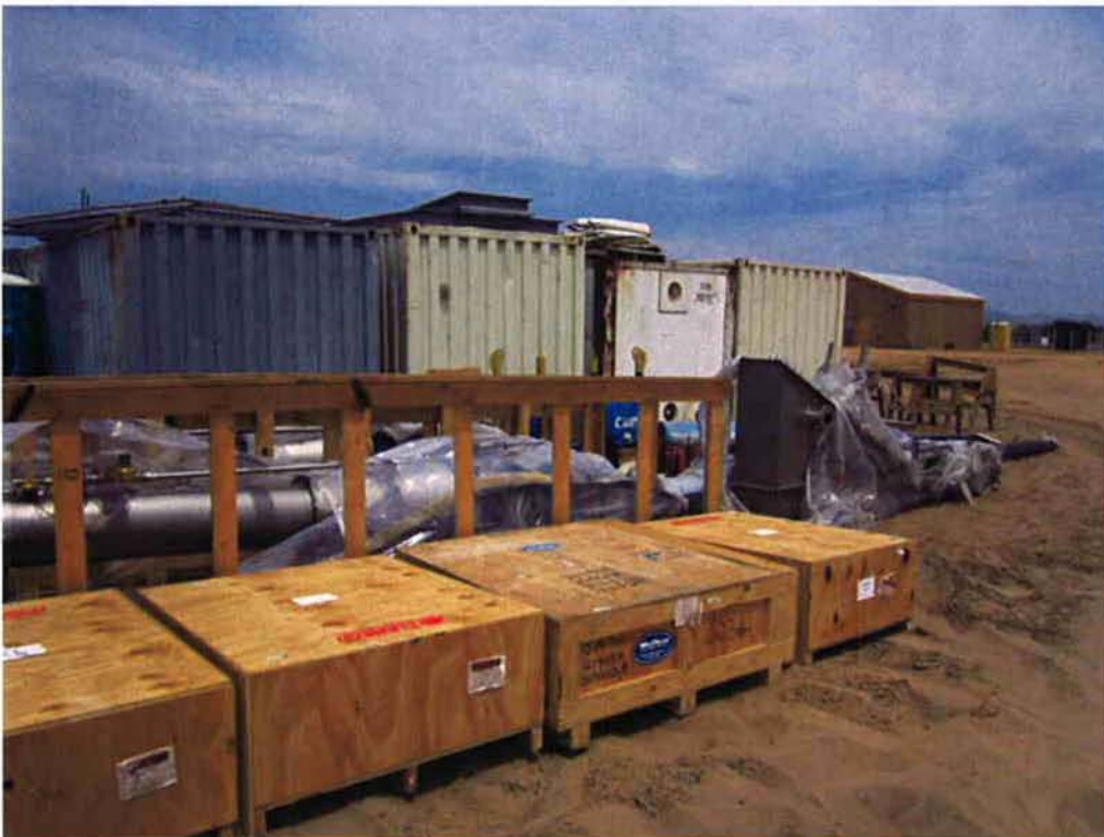
Receipt of screw conveyor and grit classifier.
