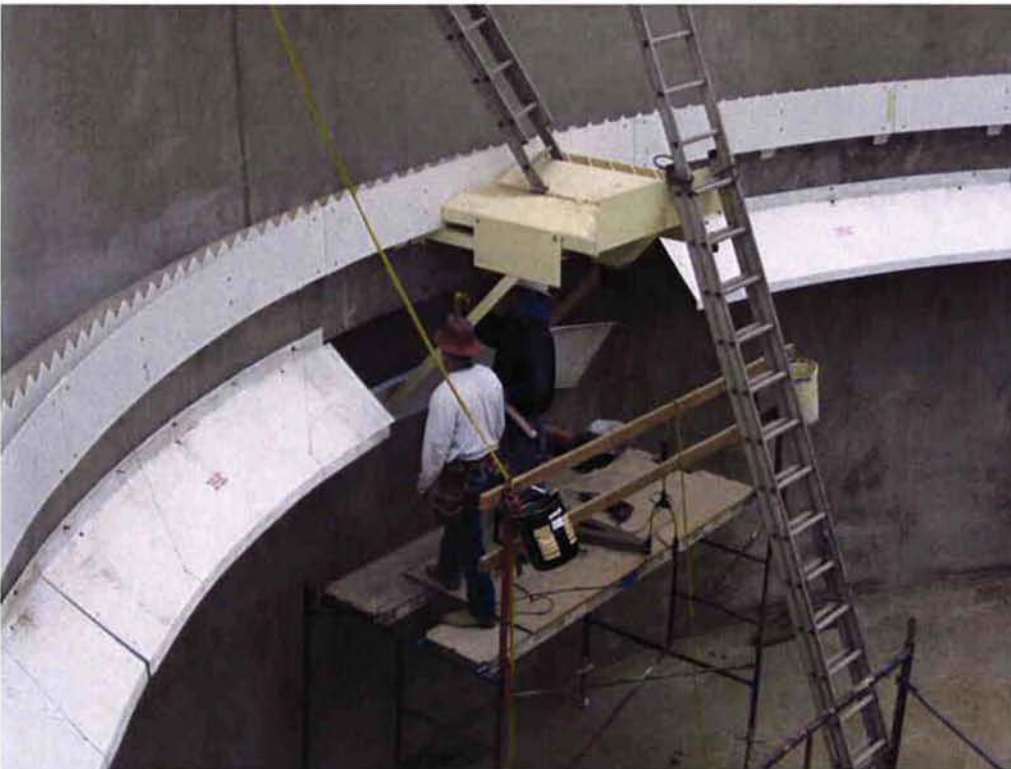
Installing the peripheral baffle inside Clarifier #1.
