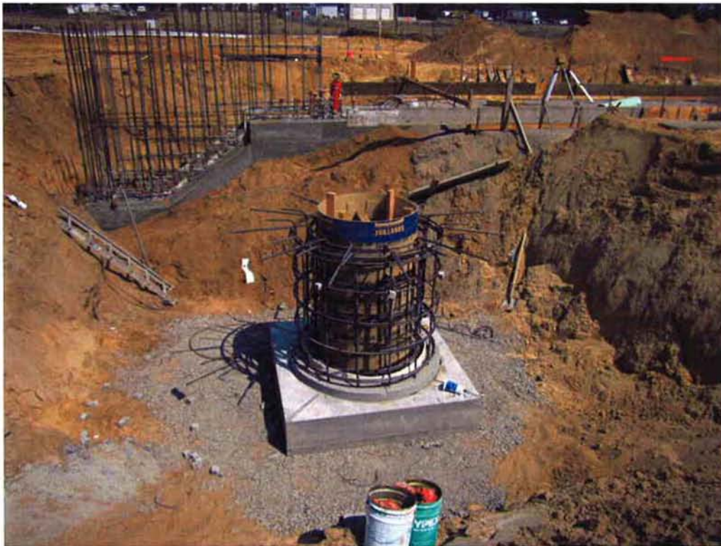
Reinforcing and wall forms for grit removal chamber.
