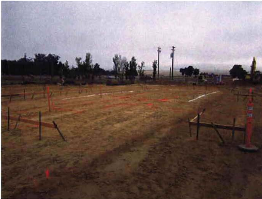
Laying out the headworks and grit removal system.
