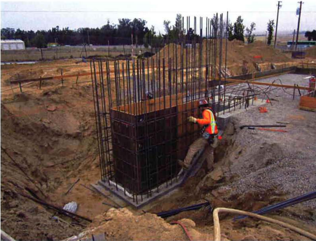
Forming the walls for the lower headworks.
