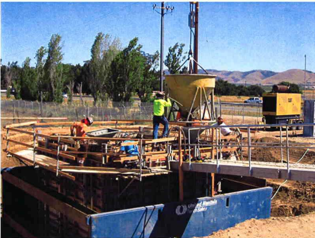
Cushman pouring the walls of the Influent Pump Station.
