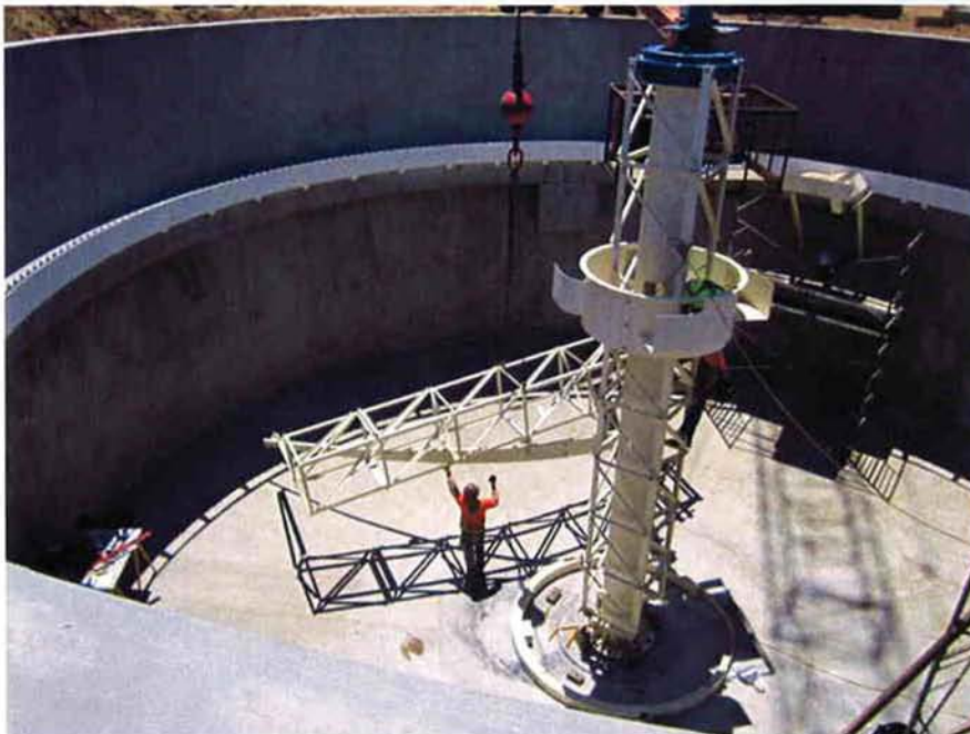
Installing mechanisms inside Clarifier #1.
