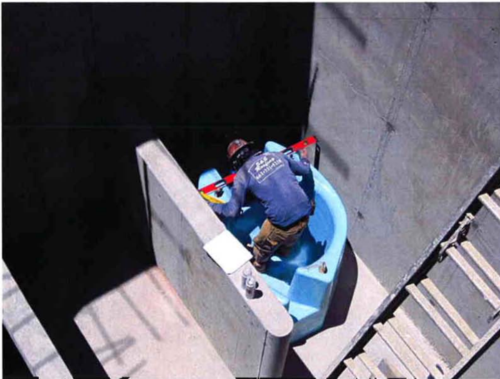
Aligning the prerotation basins inside the Influent Pump Station
