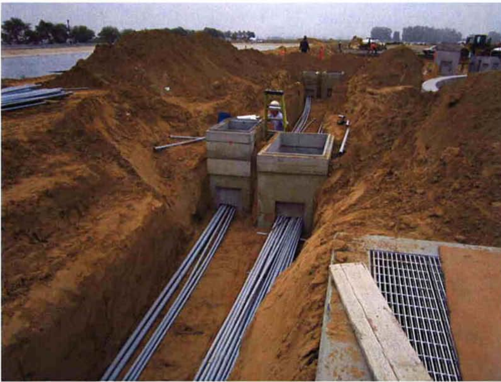
Bergelectric installing Duct Bank #16 conduit between Pull Boxes #11 and 22.
