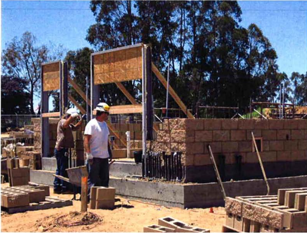
Beinscroth Masonry installing CMU block at the Sodium Hypochlorite Building.
