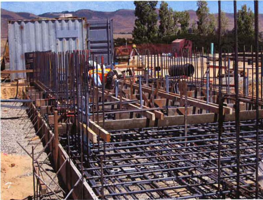
Forming starter walls at Headworks Screening System.
