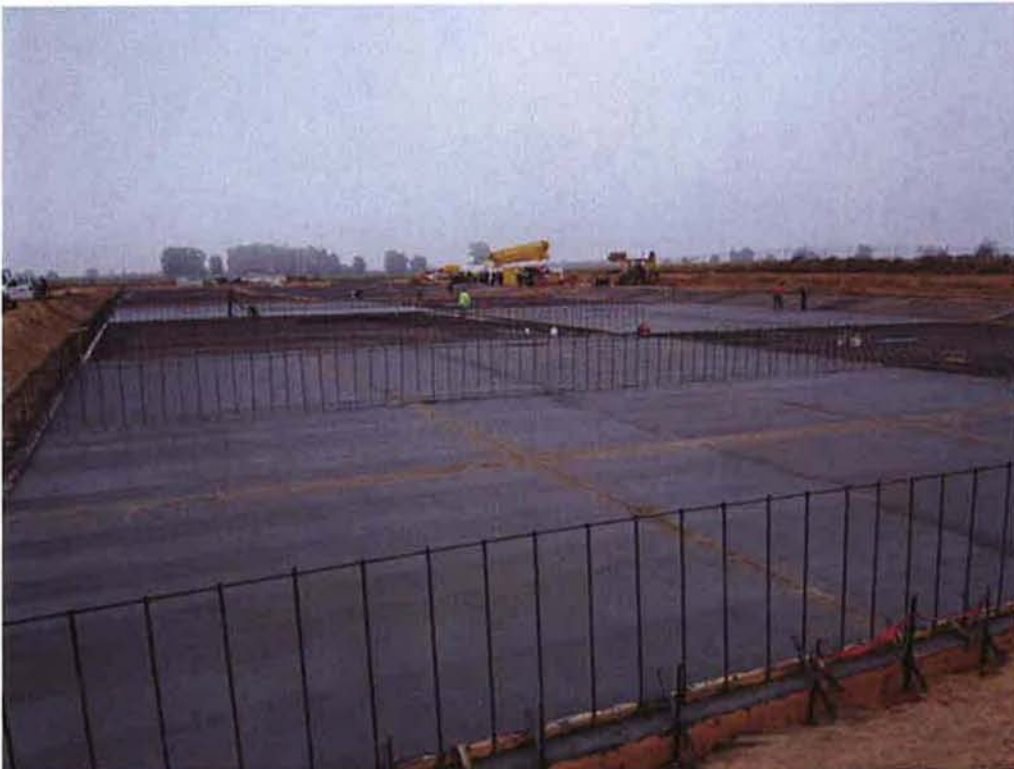
Slabs in Sludge Drying Bed #1 curing after first concrete pour.
