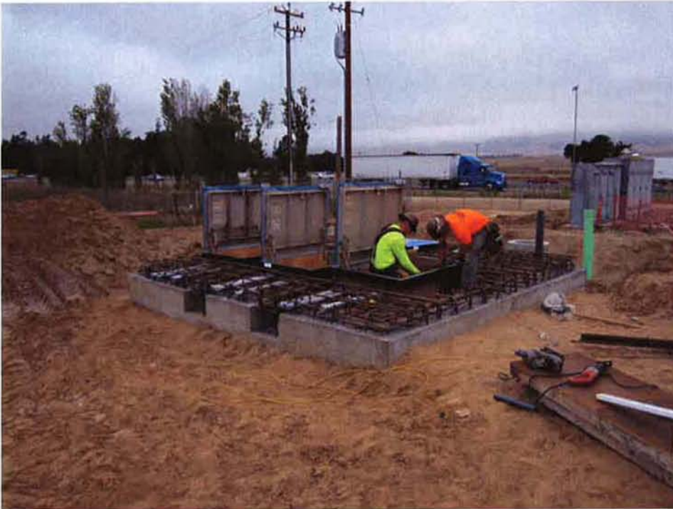
Cushman forming Influent Pump Station deck.
