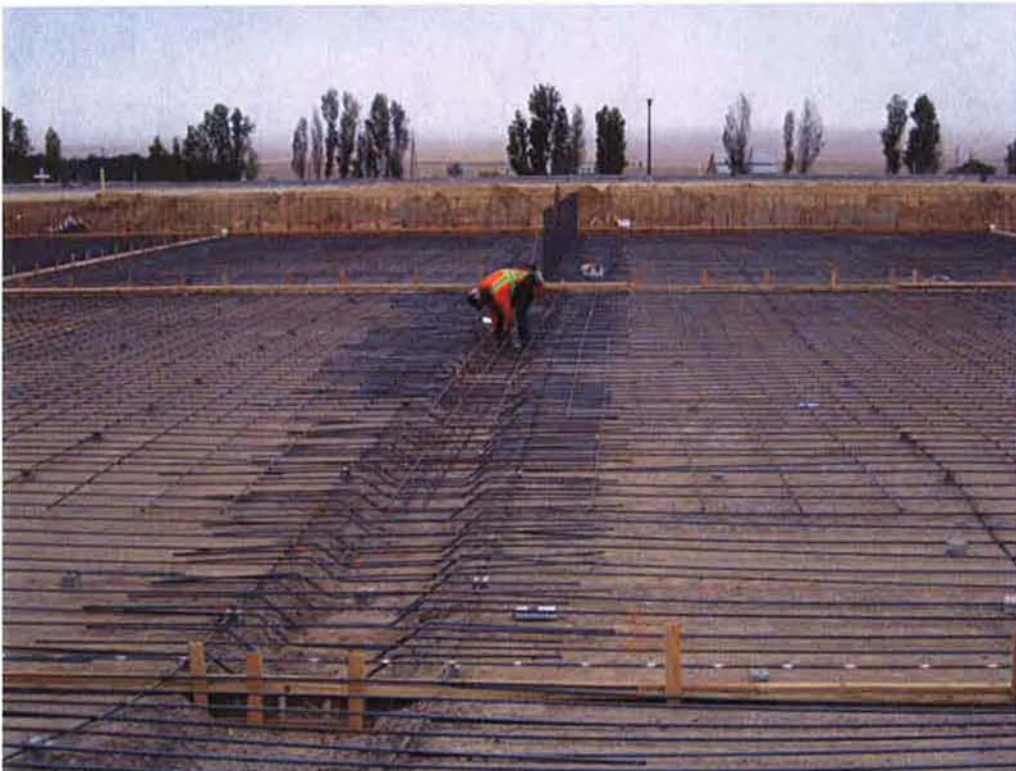
CMC Rebar tying reinforcement at the wall foundations of the Sludge Drying Beds.
