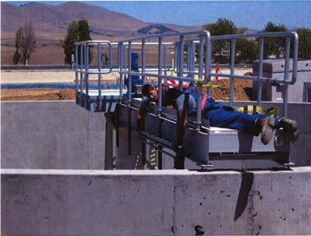
Bergelectric installing rigid conduit along the bridge at Clarifier #2.
