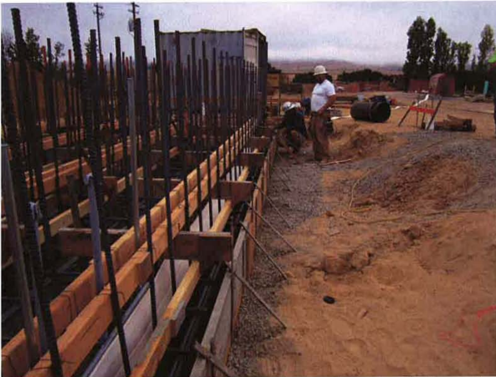
Cushman installing water stops at the Headworks Screening System walls.
