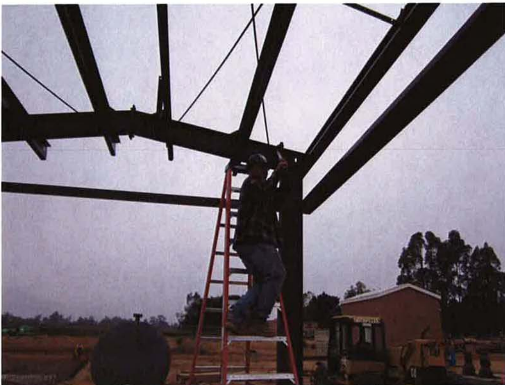
Fugro torque testing the bolts on the structural steel for the canopy.
