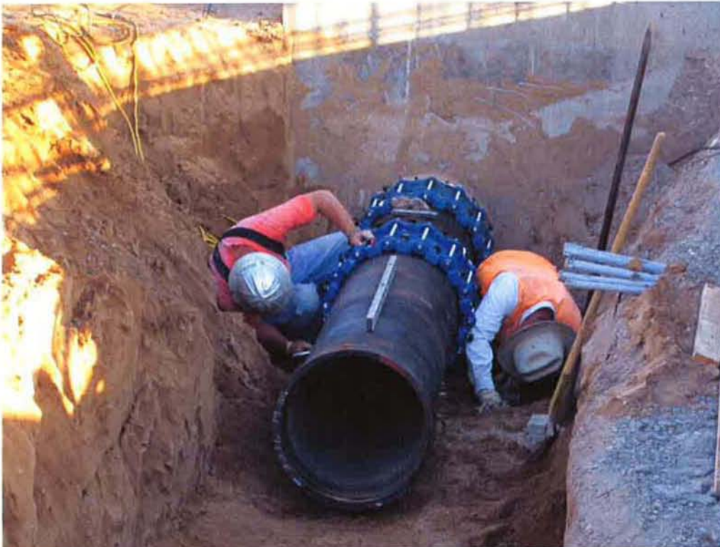
Cushman installing 20-inch SI pipe from Headworks to Distribution Box #1.
