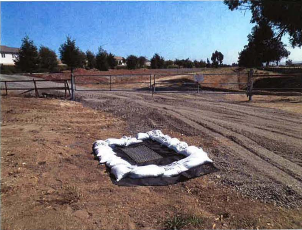
New 12' gate in SBCFC fence (for total width of 24'), and SWPPP installed at catch basin on the south side of the levee along the temporary access road constructed by ARB.
