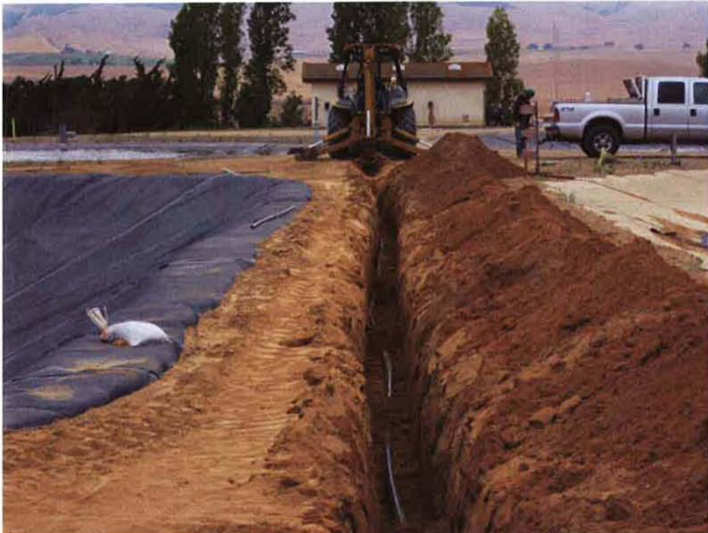
Installing 2-inch NPW line.
