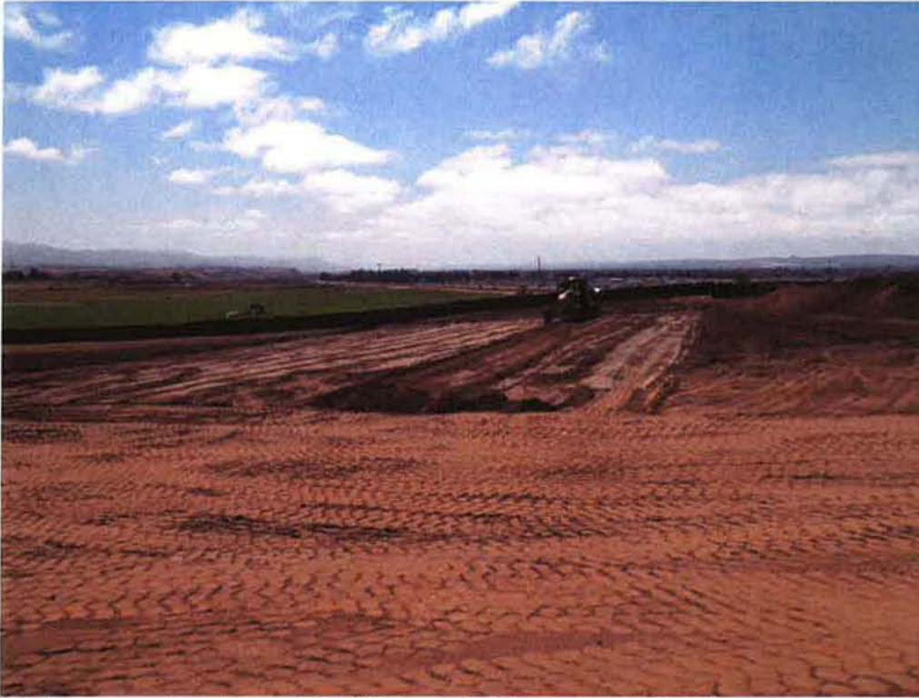
Burke excavating top soil to 18" deep inside pump station temporary construction easement and HDD work area.
