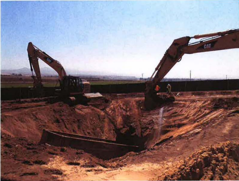
Backfilling around 54-inch diameter casing at the north side of the project.
