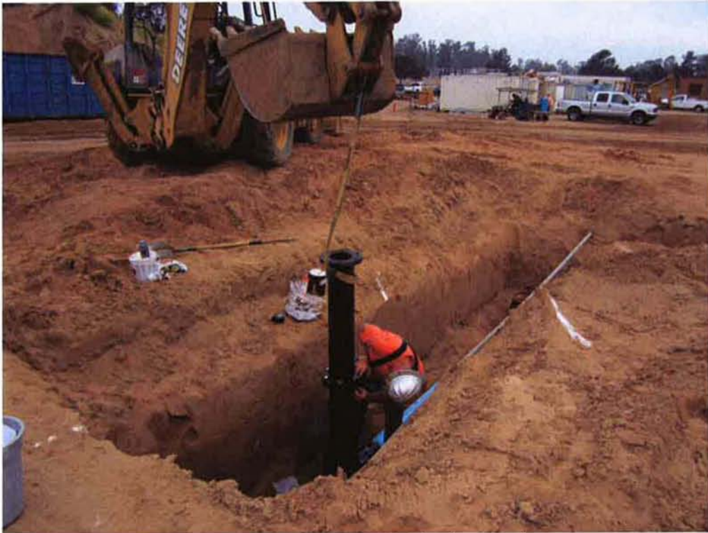
Cushman installing riser for fire hydrant off 6-inch waterline.
