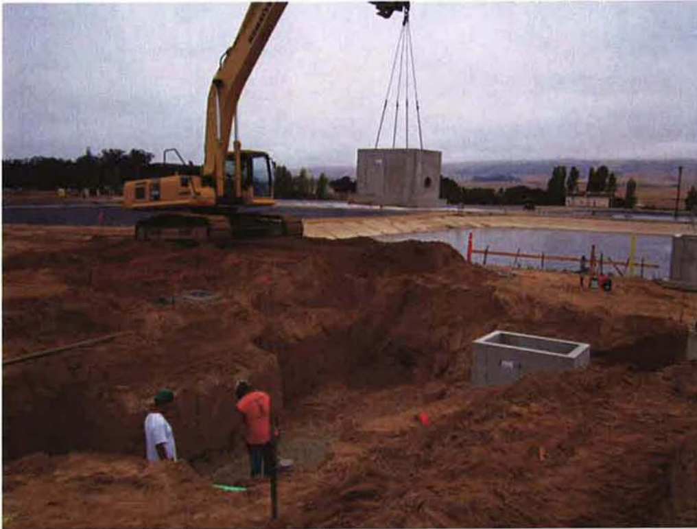
Cushman installing flow meter vaults.
