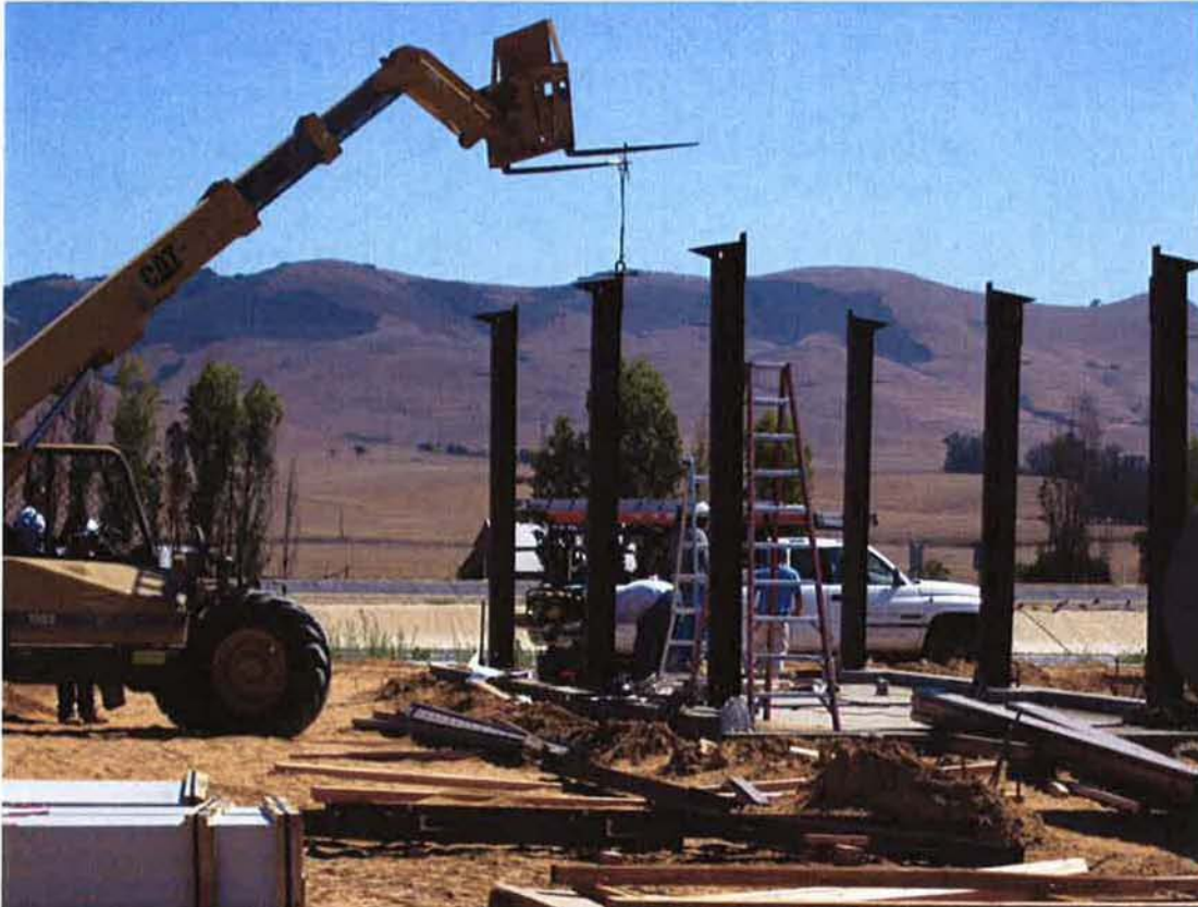
Dueck Construction erecting steel structure at Sludge Thickening System to support canopy.
