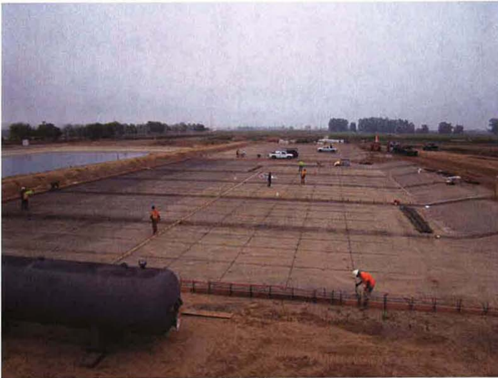
CMC Rebar tying reinforcement at the Sludge Drying Beds.
