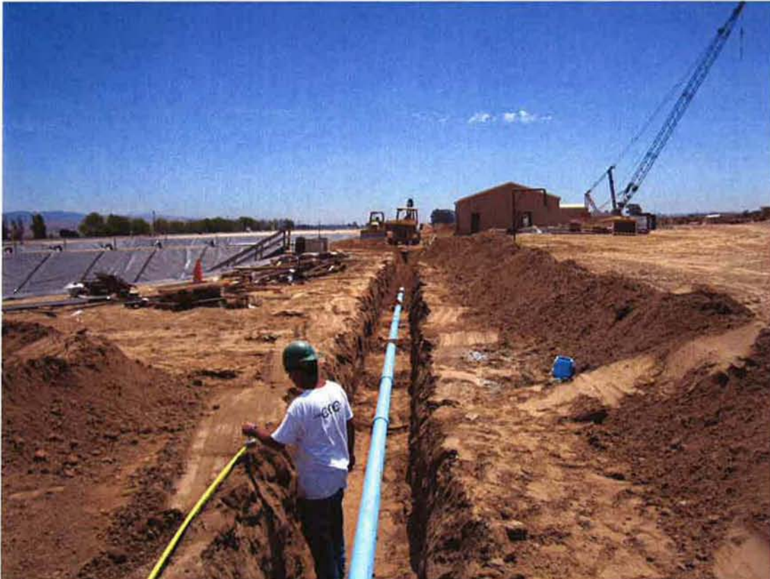
Cushman installing 6-inch water line.
