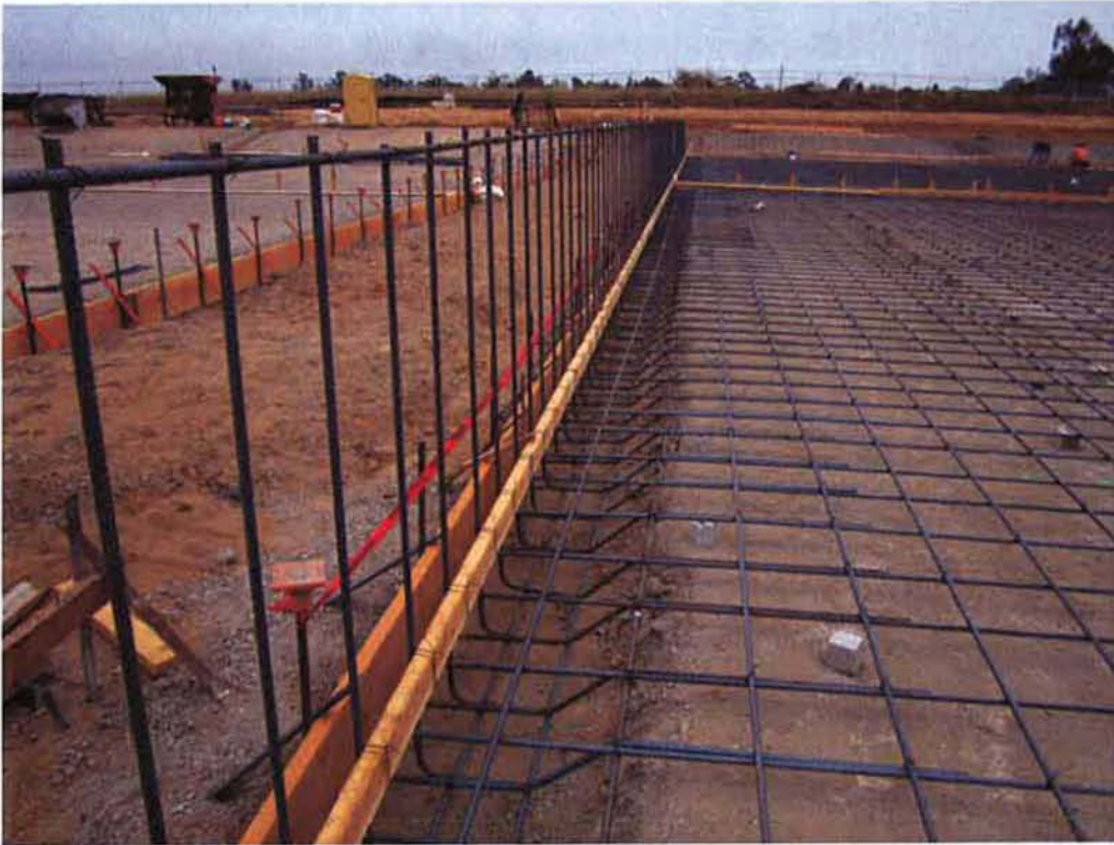
Reinforcement for walls and edge forms at Sludge Drying Bed #2.
