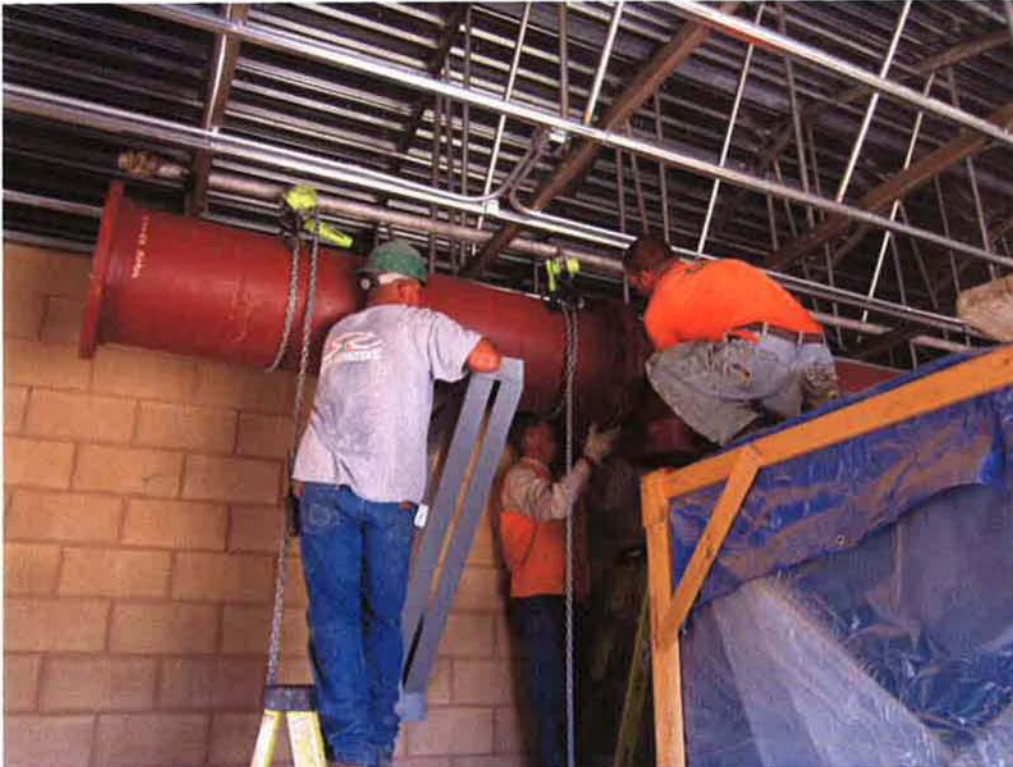
Cushman installing 18-inch AR piping inside blower room.
