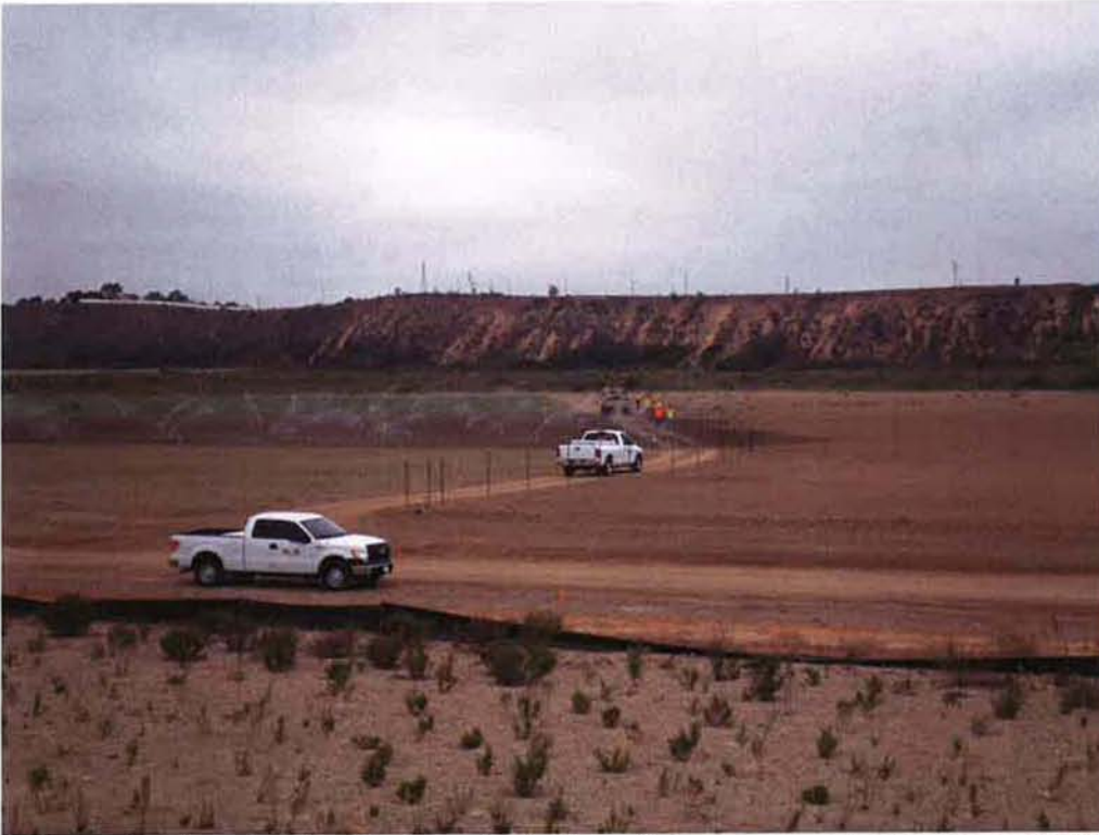
ARB and subcontractor Marborg installing silt fence along temporary construction easements at the south site.
