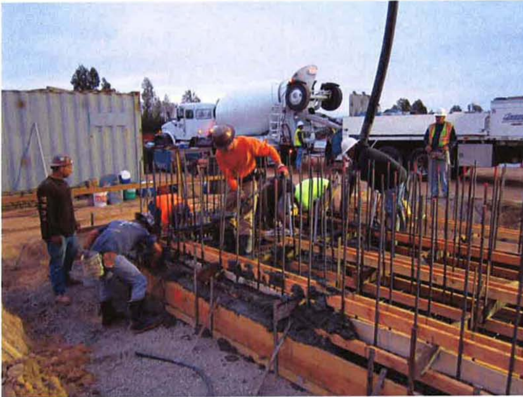
Cushman pouring concrete for slab at Headworks Screening System.
