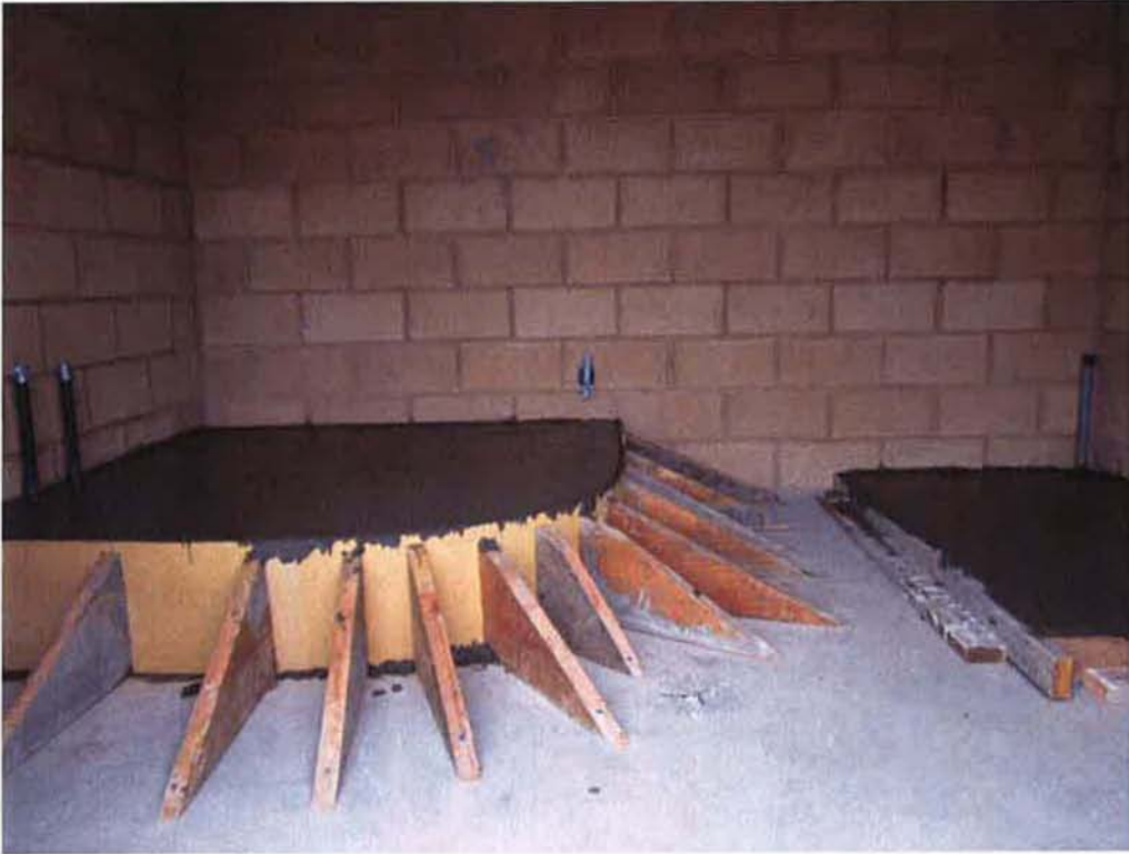
Pouring equipment slabs inside Sodium Hypochlorite Building.
