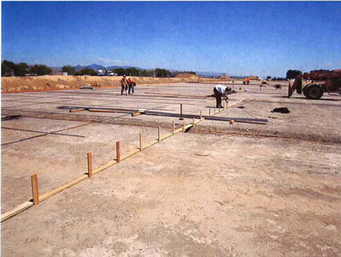
Cushman forming footings and control joints at Sludge Drying Beds.
