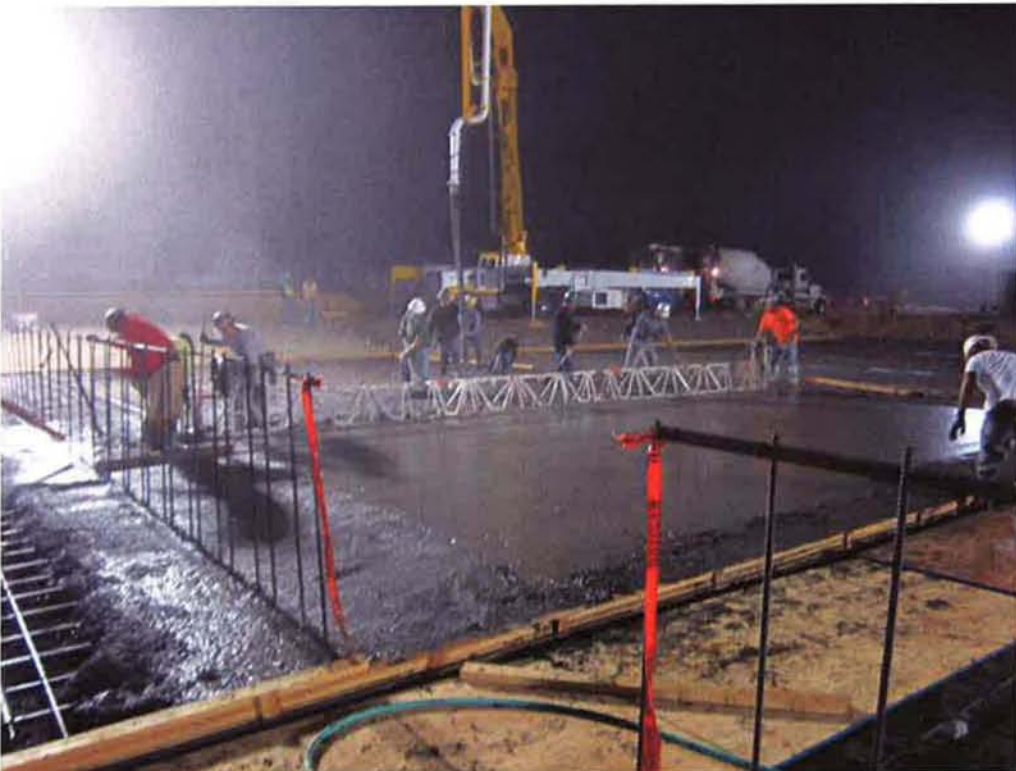
Skreeding concrete of first slab section in Drying Bed #1.
