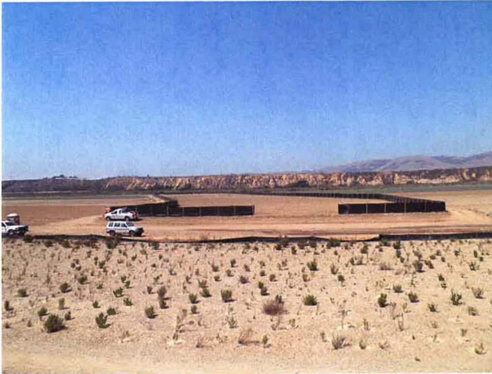
Silt fence installed on south side of project.
