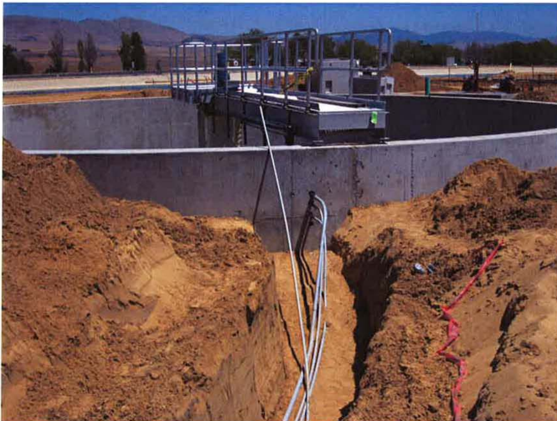
Conduit being installed to Clarifier #1.
