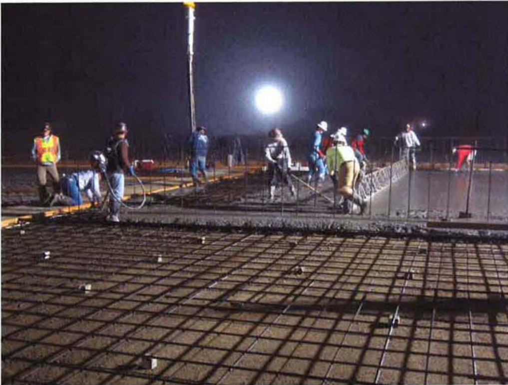
Cushman skreeding slab section of Sludge Drying Bed #2.
