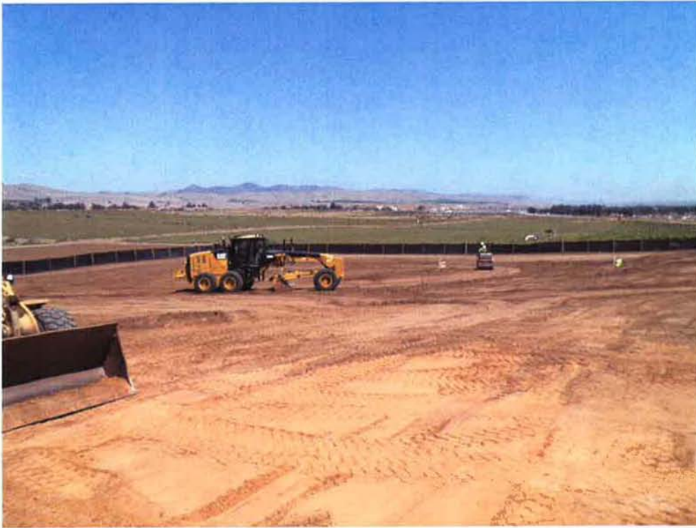
North side of the site at future pump station prepped for installation of the 54-inch diameter casing.
