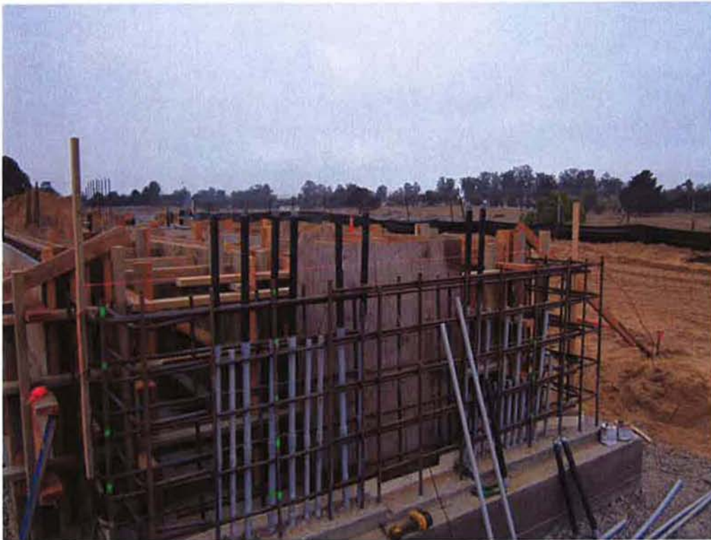
Bergelectric installing through-wall conduit at Headworks Screening System
