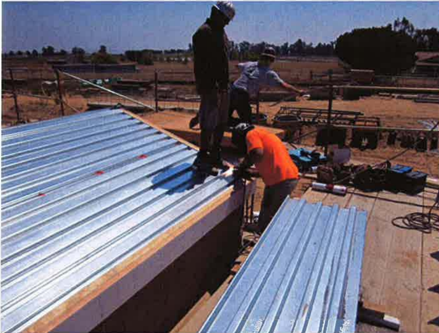
Cushman puddle welding metal deck for roof on Sodium Hypochlorite Building.
