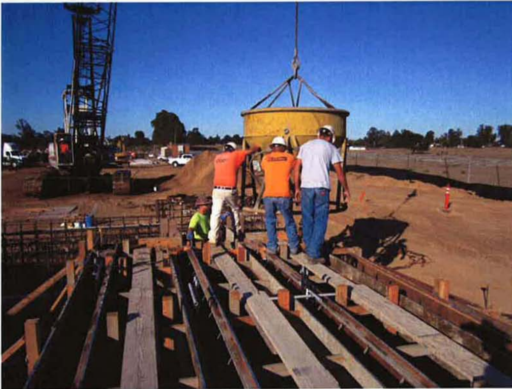
Concrete placement for walls at Headworks Screening System.
