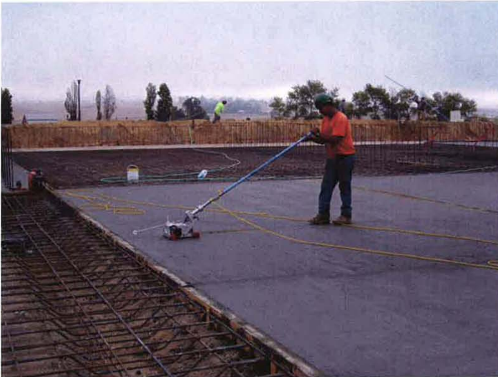
Cushman cutting joints in Sludge Drying Bed #1 after first concrete pour.
