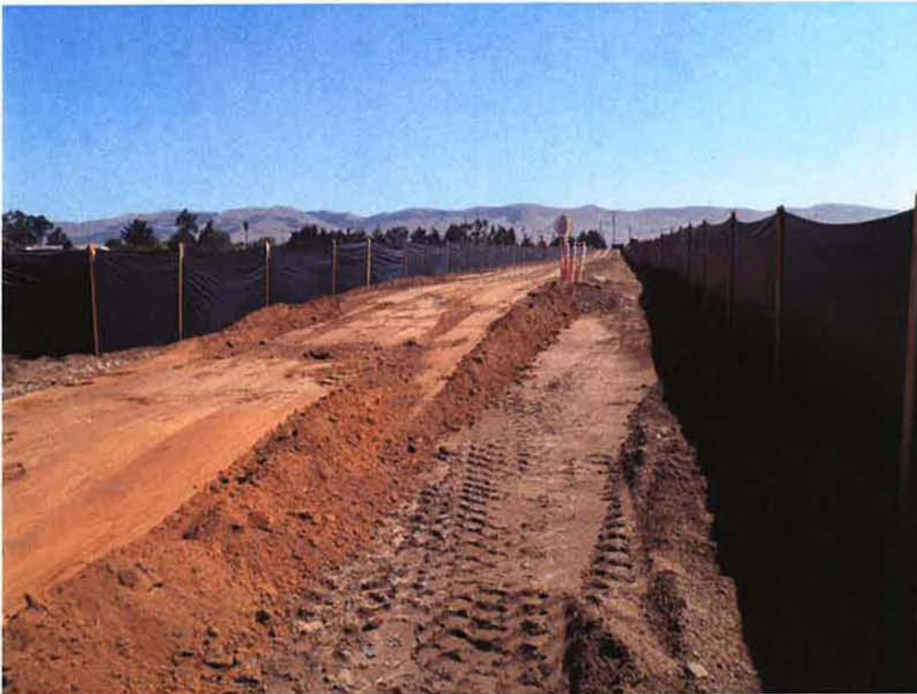
Building up road to protect existing Phillips 66 oil line.
