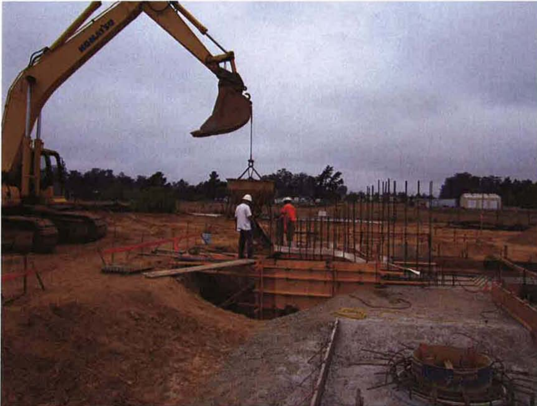
Cushman pouring concrete for lower walls of Headworks Screening System.
