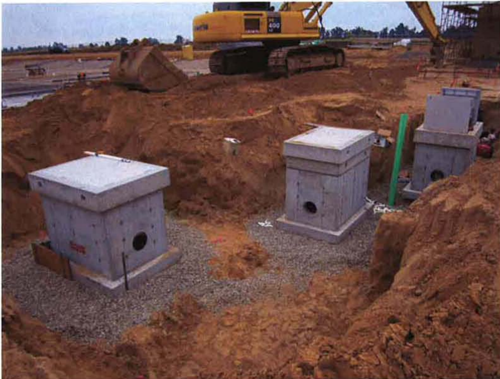
Flow meter vaults installed.
