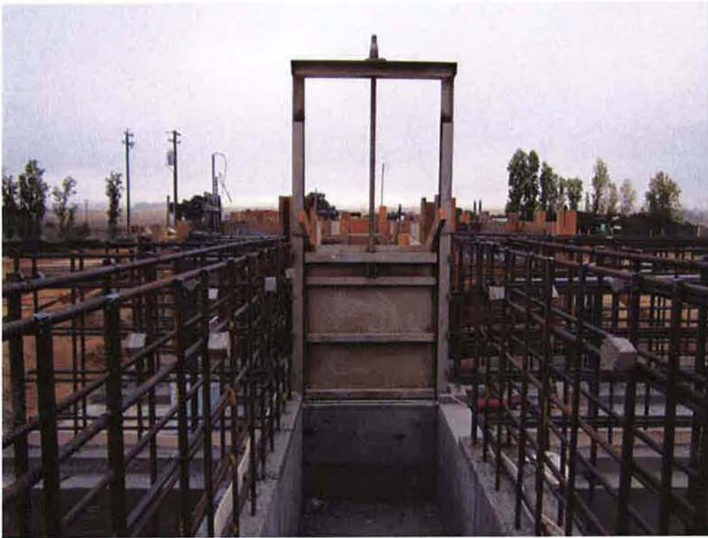
Center channel gate installed at Headworks Screening System .
