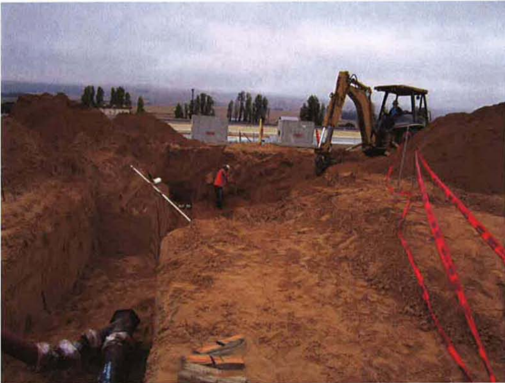
Cushman excavating for flow meter vaults.
