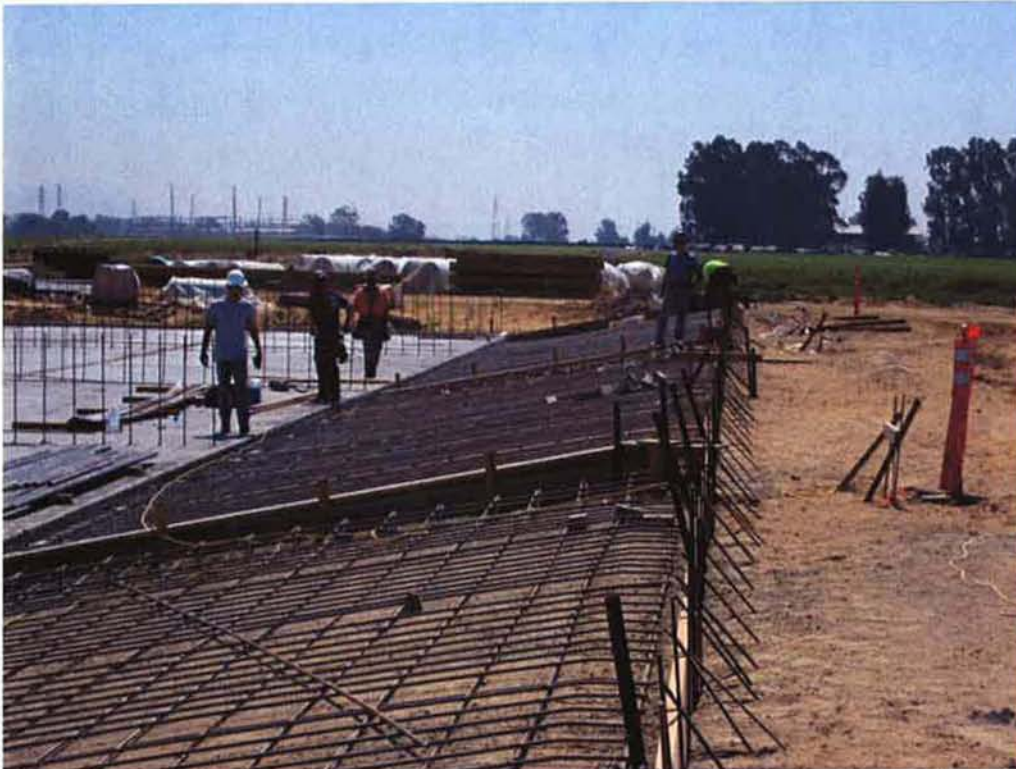
Cushman setting footing edge board along ramp at Sludge Drying Beds.
