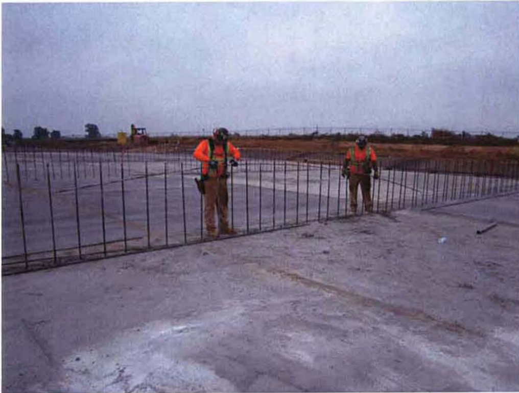
CMC Rebar tying reinforcement for walls at Sludge Drying Beds.
