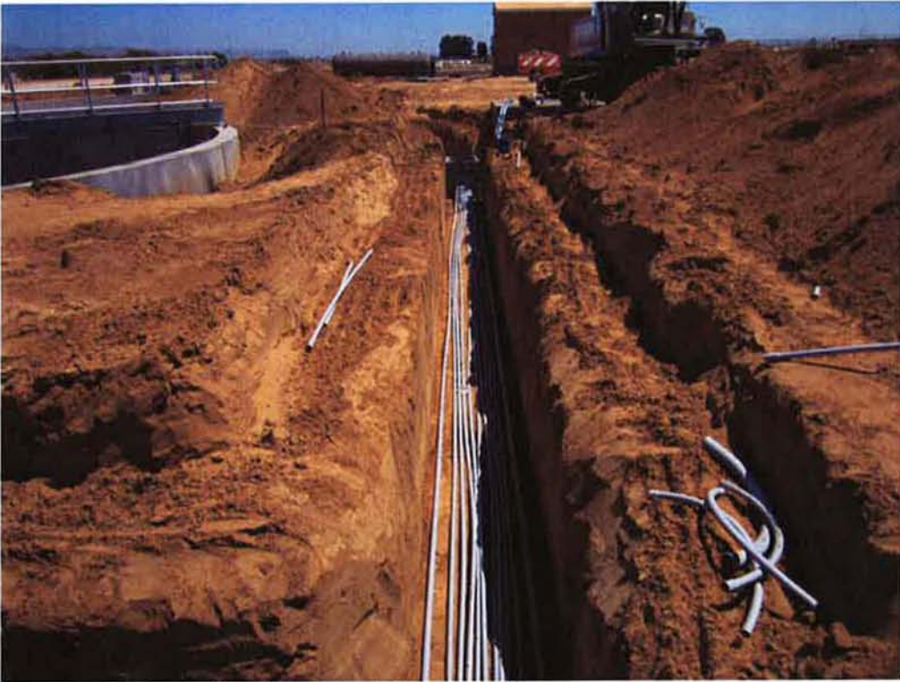
Bergelectric installing Duct Bank 24 (DB-24).
