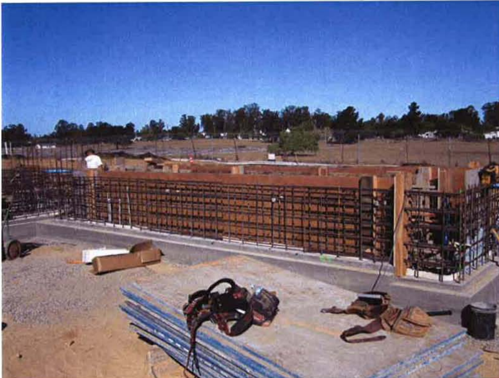
Forming interior walls of the Headworks Screening System.
