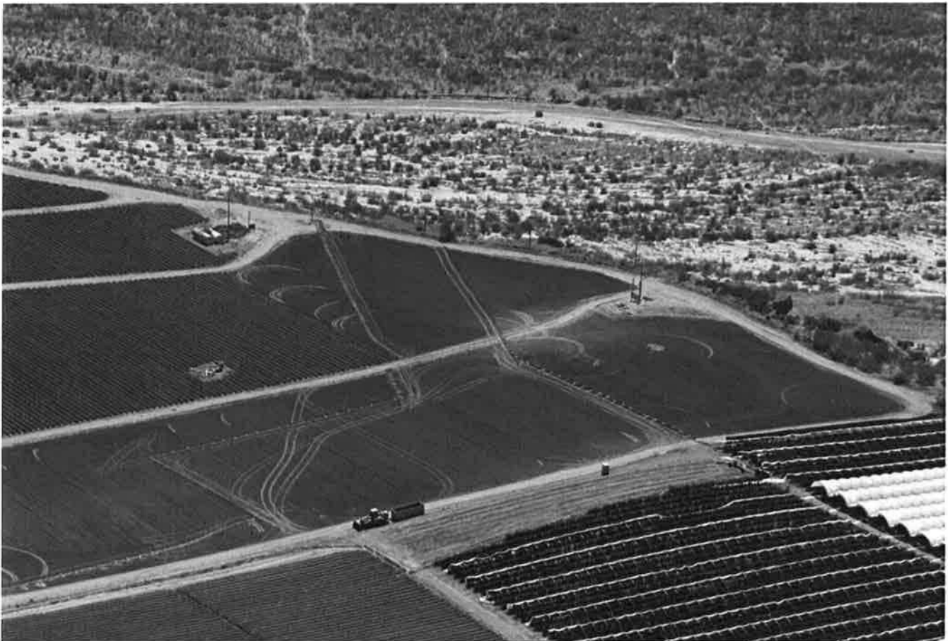
Aerial view of the north side of the project at the future pump station site.
