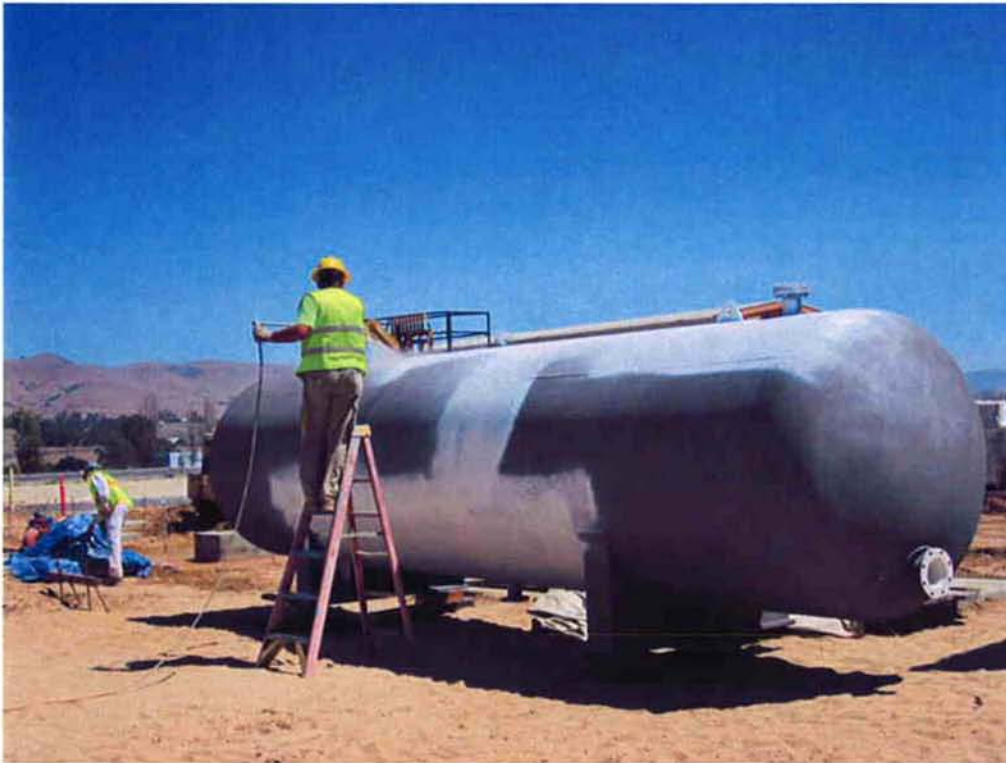
KNK Coating applying primer to the hydropneumatic tank.
