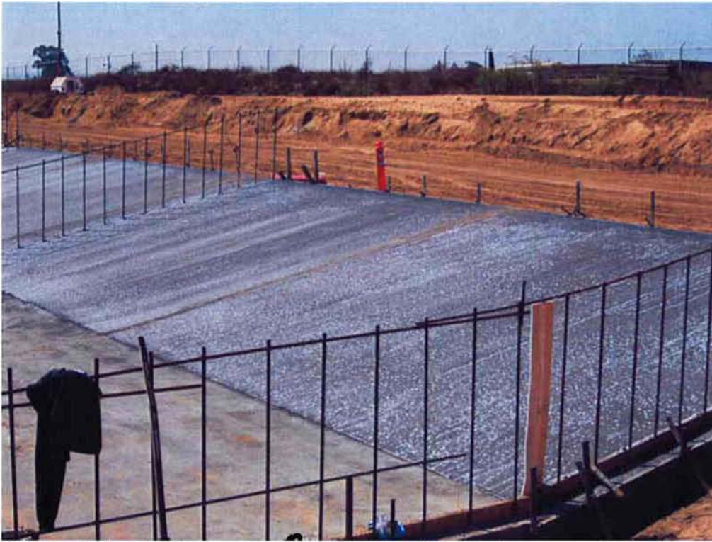
Sludge Drying Bed ramp pours complete and concrete cure applied.
