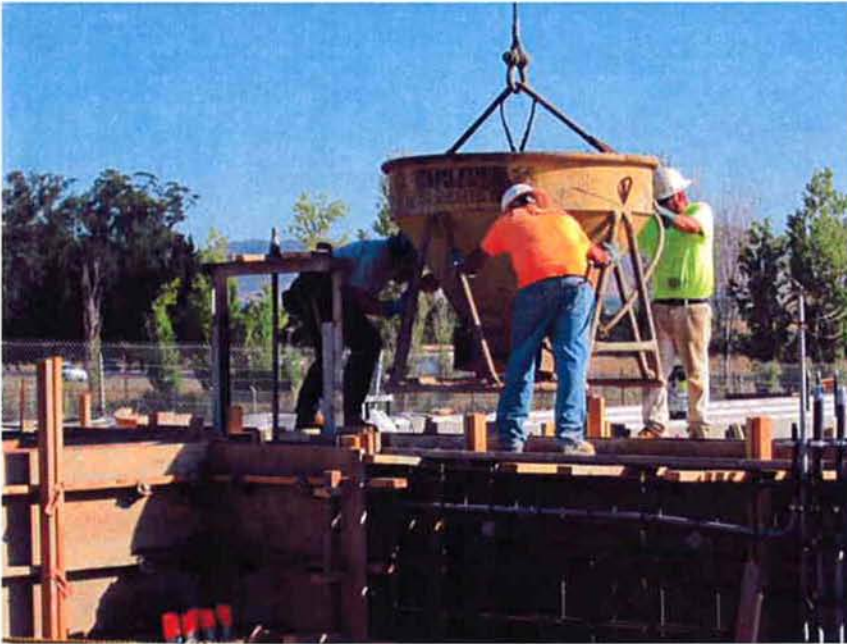
Cushman pouring channel walls to the Vortex Grit Tank.
