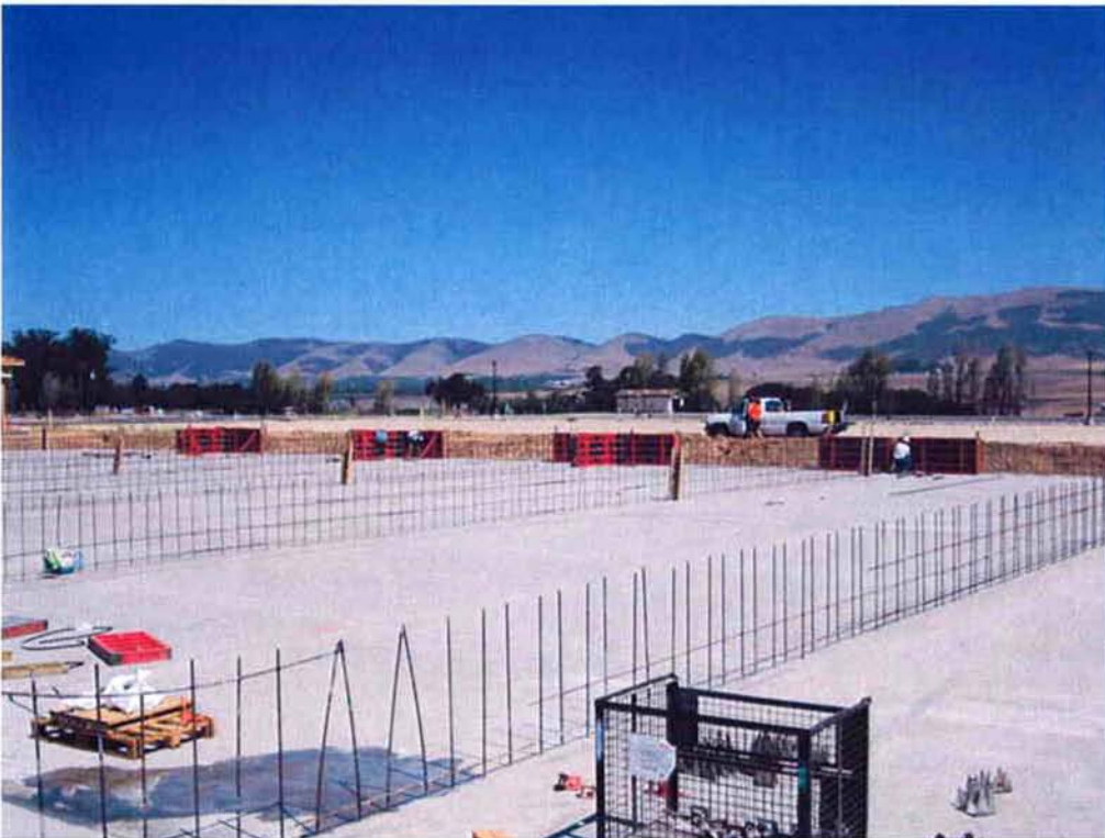
Divider wall intersection forms installed at Sludge Drying Beds.
