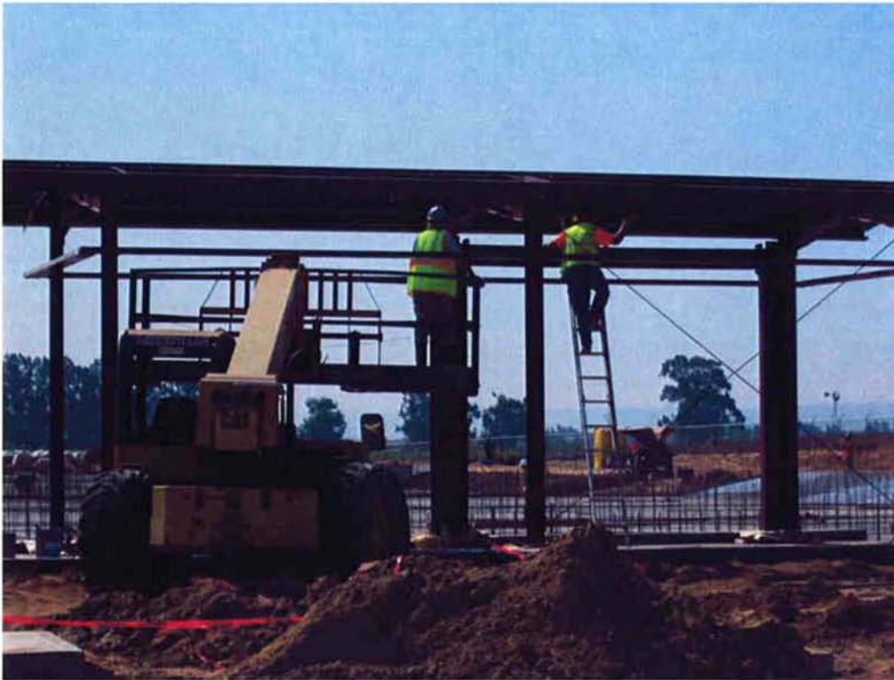
KNK Coating sanding the Sludge Thickening Building in preparation for applying the prime coat.
