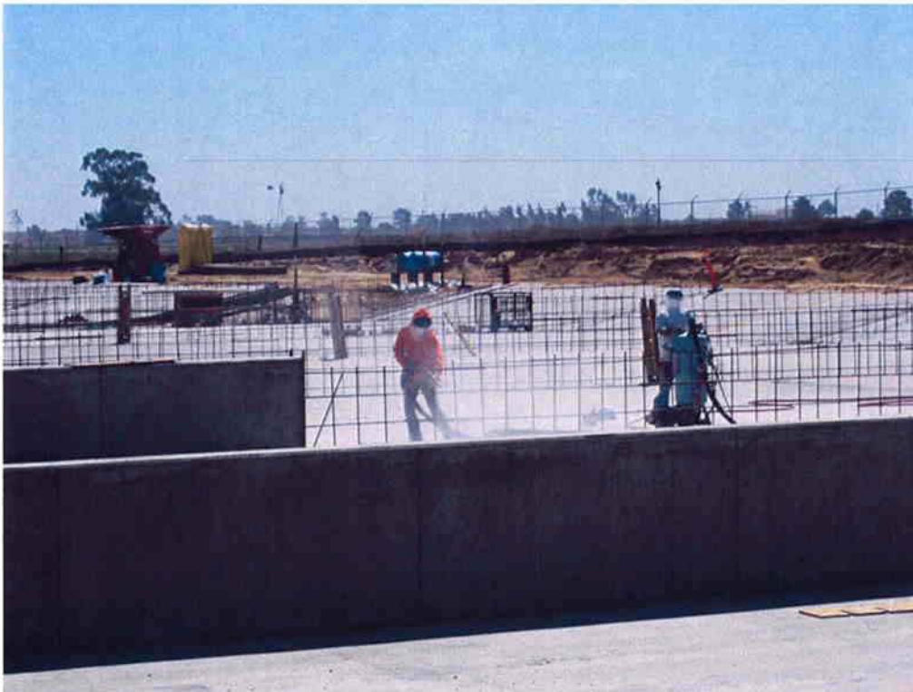
Cushman sandblasting rebar and concrete before next divider wall pour at Sludge Drying Beds.
