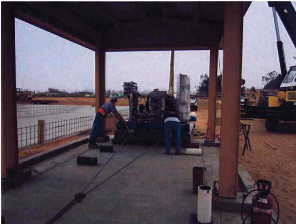
Cushman moving sludge thickening equipment into place at Sludge Thickening Building.
