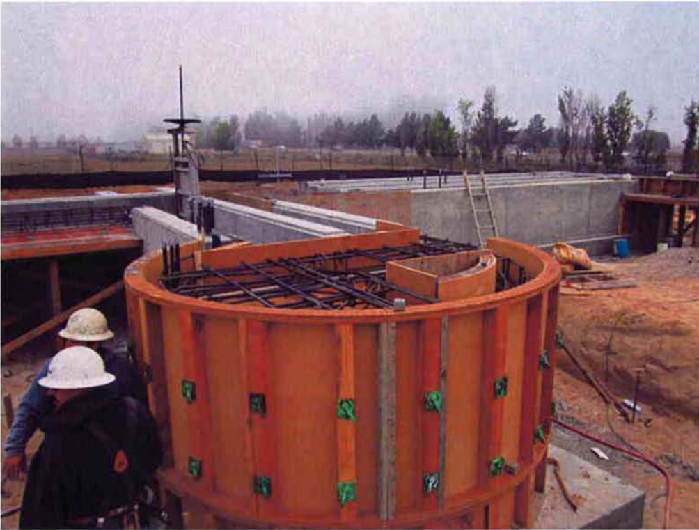
Completing forms for the Grit Chamber.
