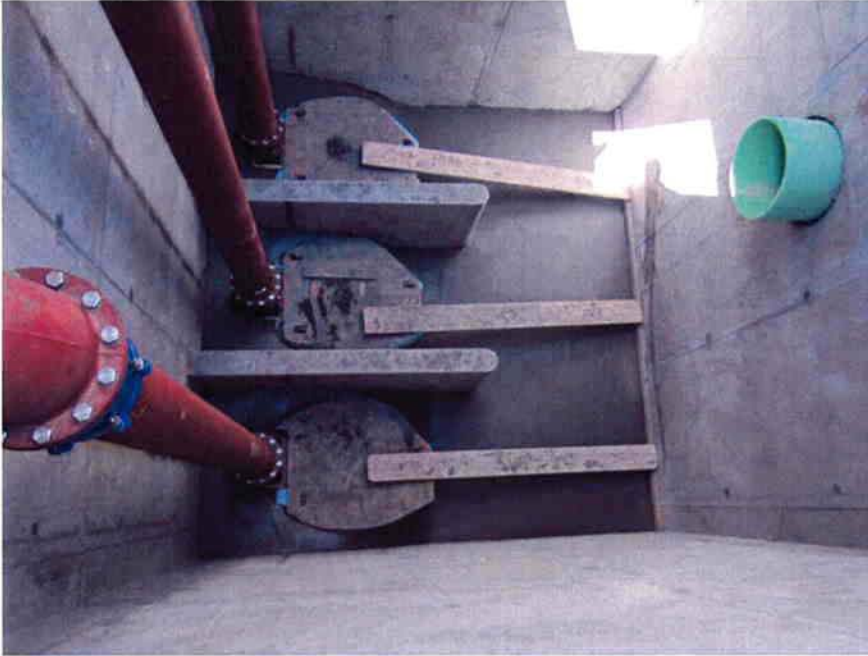
Cushman pouring concrete fill at the Influent Pump Station.
