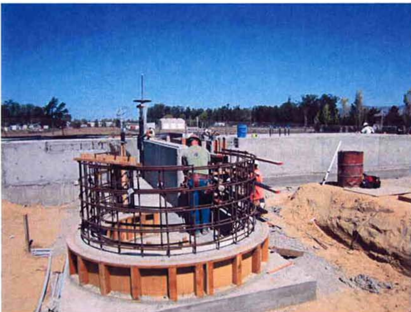
Cushman forming Grit Chamber walls.
