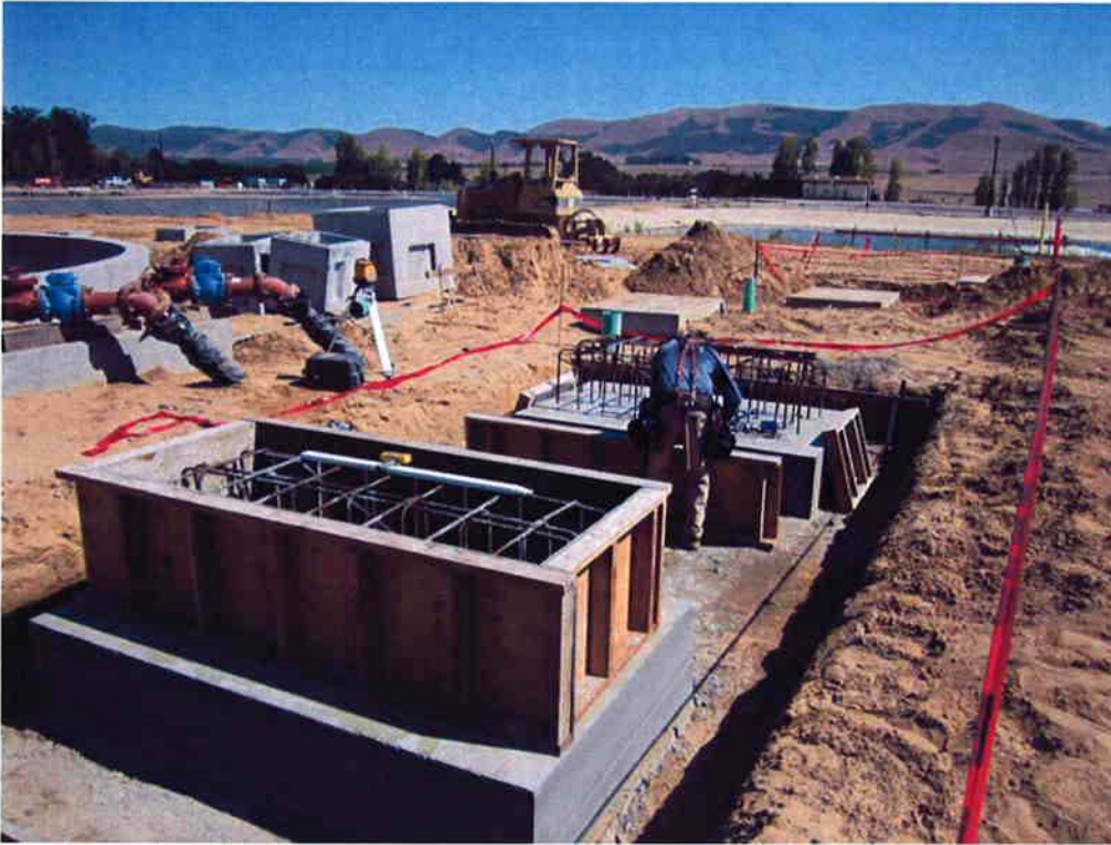
Cushman forming hydropneumatic tank supports.
