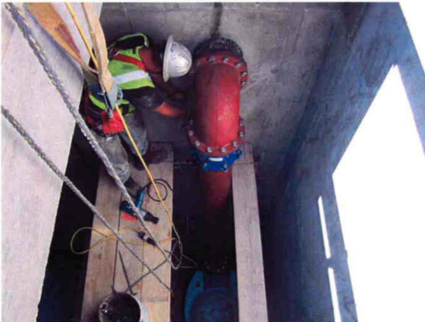
Cushman installing 10-inch RW piping at the Influent Pump Station.
