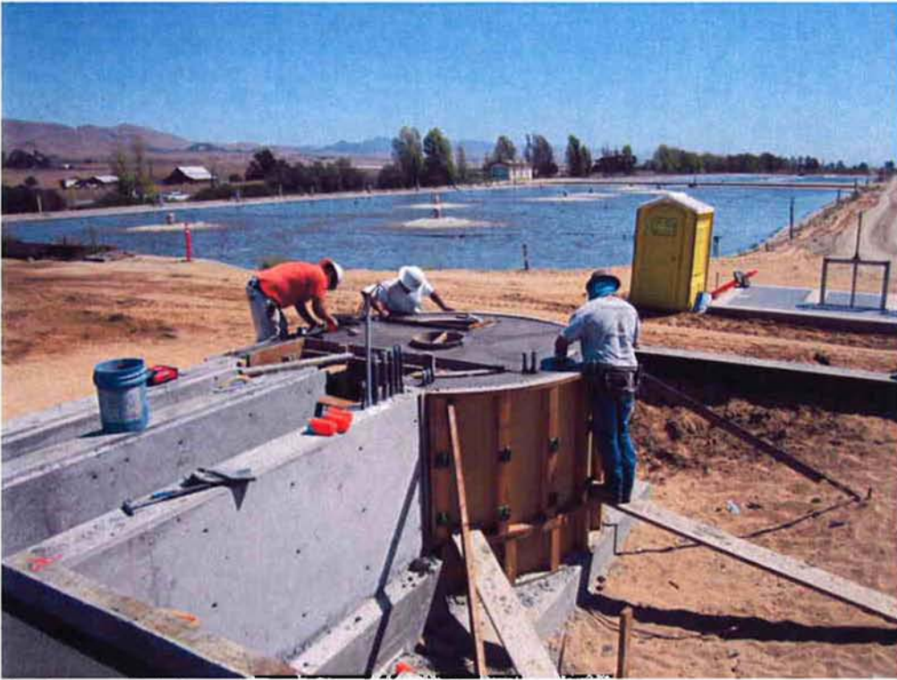
Cushman finishing the surface of the Grit Chamber.
