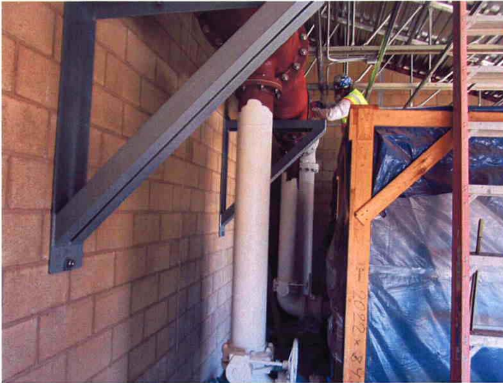
KNK Coating priming AR piping in Blower Room of Electrical/Blower Building.
