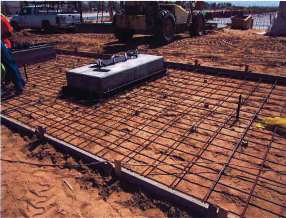
Cushman forming the hydropneumatic tank slab, and CMC installing reinforcing.
