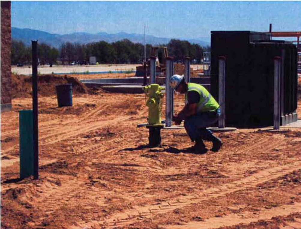
Cushman installing the fire hydrant near the Electrical/Blower Building.
