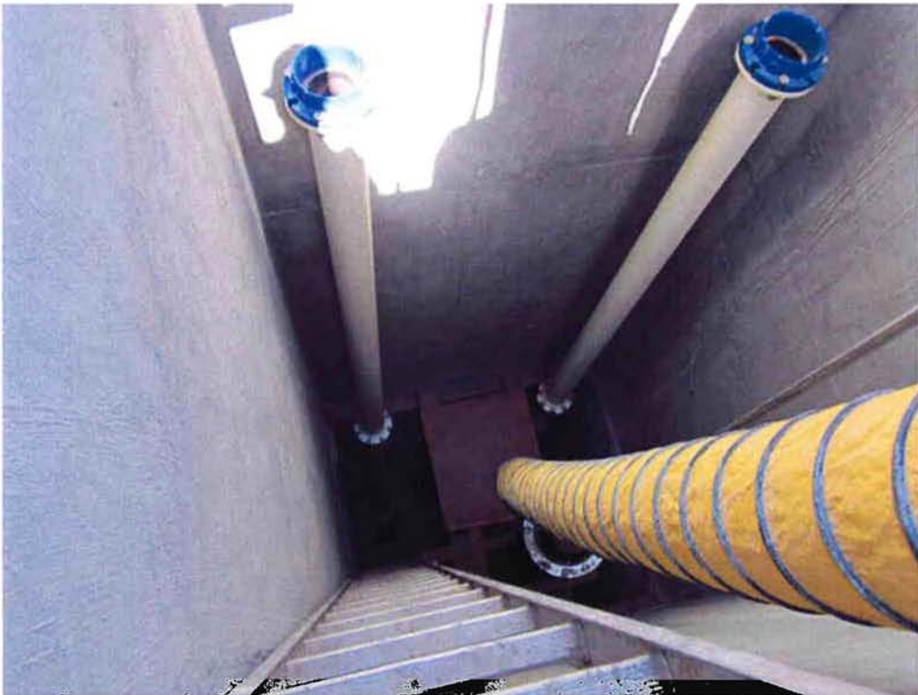
Cushman installing RAS/WAS Piping inside RAS/WAS Pump Station #2.
