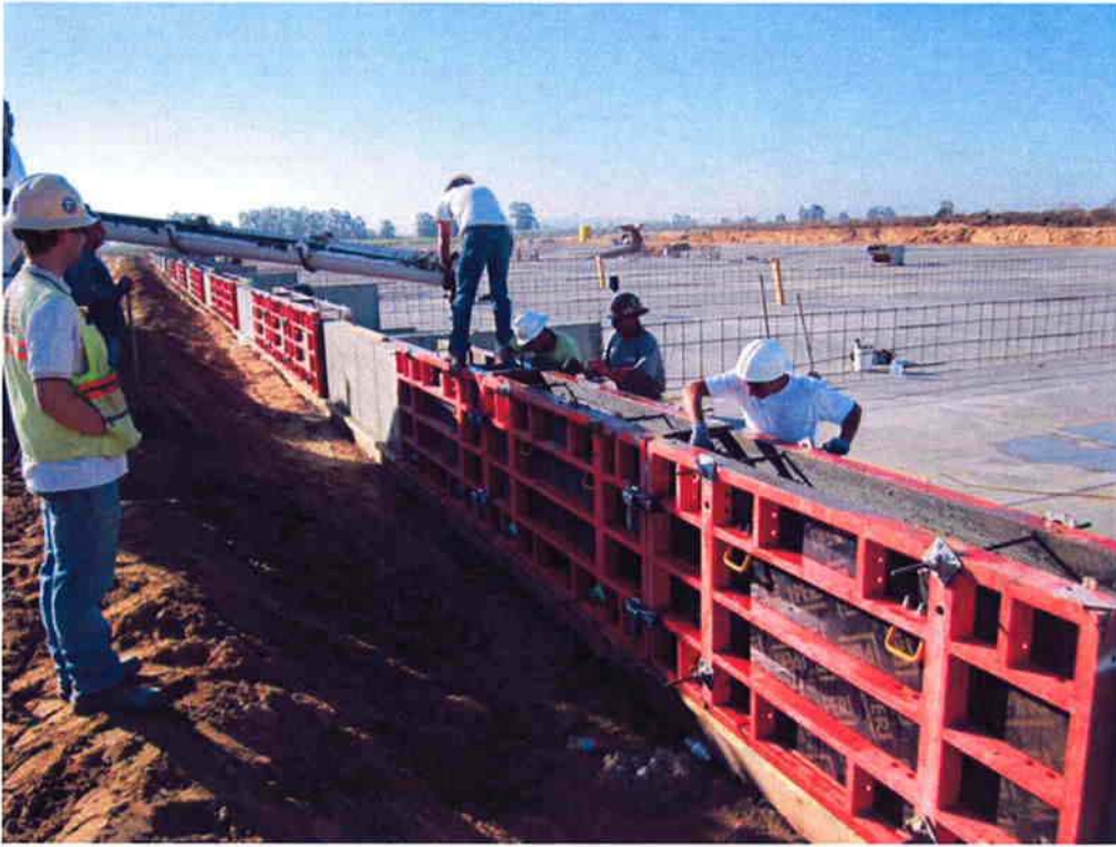
Cushman pouring west wall along the Sludge Drying Beds.
