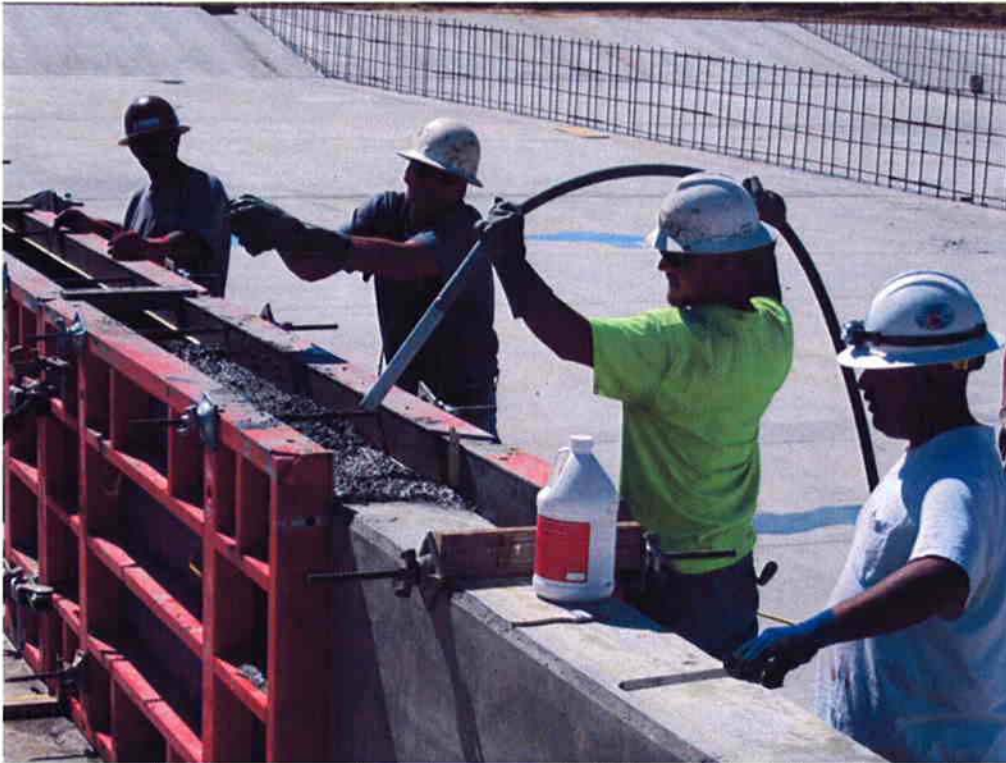
Cushman vibrating concrete during pour of divider walls at the Sludge Drying Beds.
