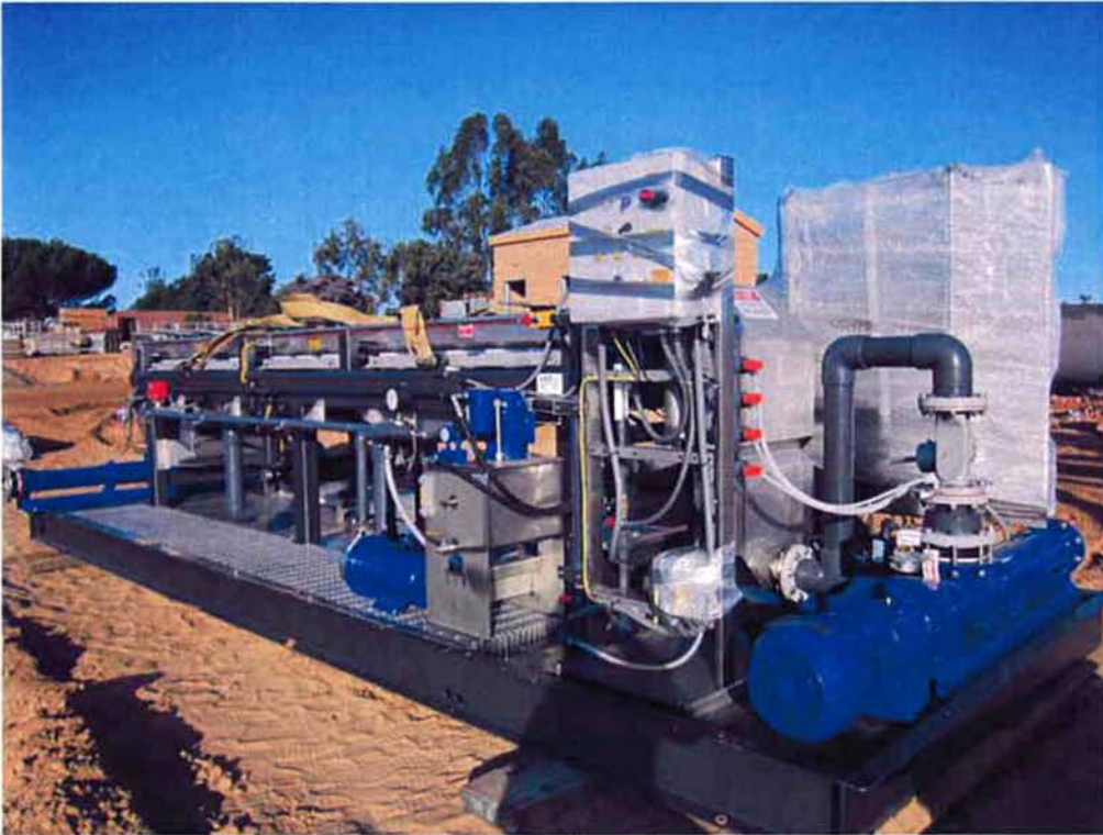
Sludge thickening equipment delivered to site.
