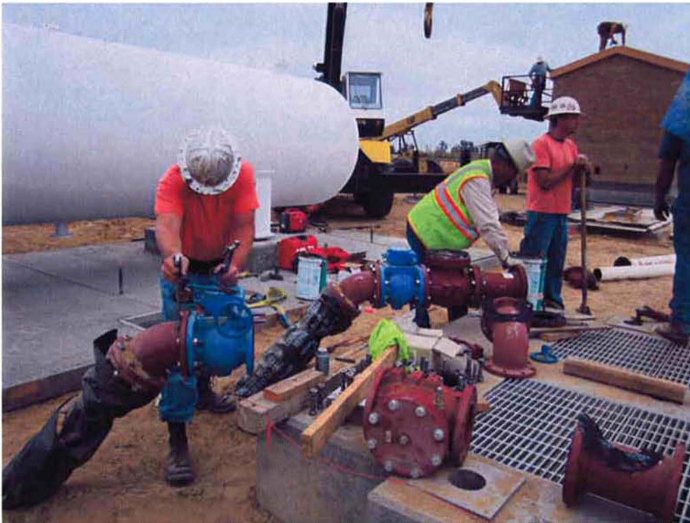
Cushman installing RAS/WAS piping from the RAS/WAS Pump Station #1.
