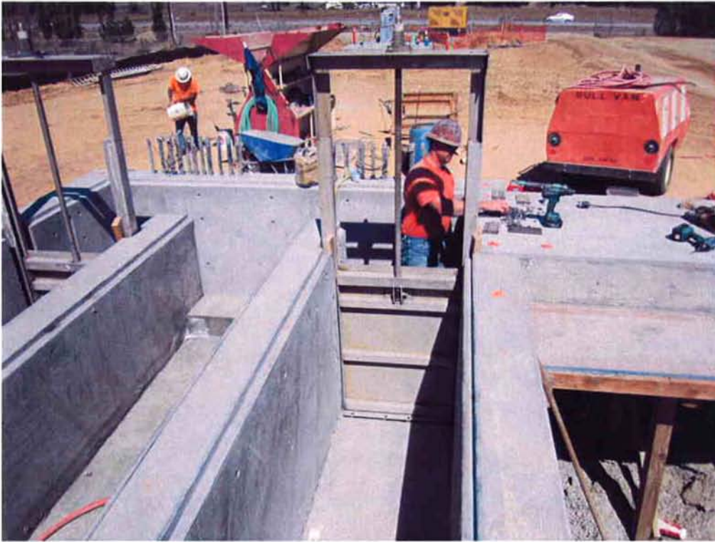
Cushman installing slide gates at the Headworks.
