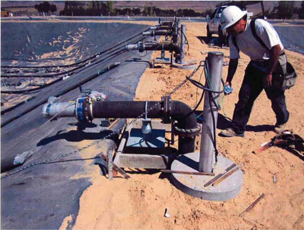
Cushman forming pads for pipe supports and disconnect switches at the AR piping for the Aeration Basin.
