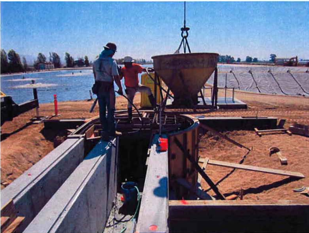
Cushman pouring the Grit Chamber structure.
