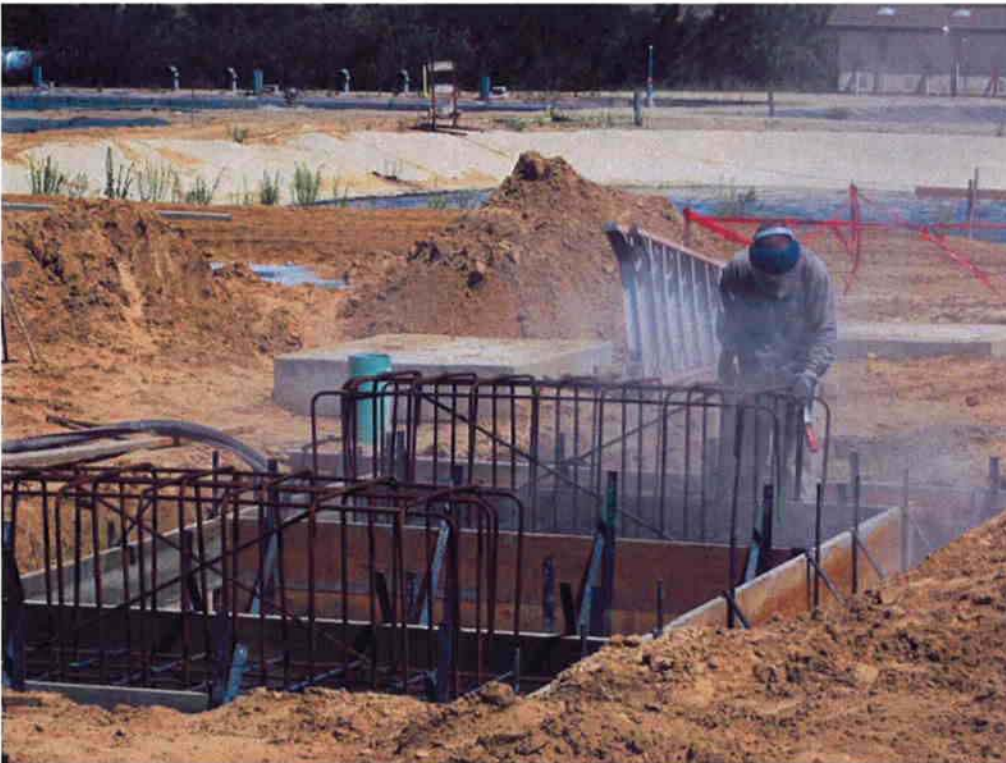
Sandblasting foundation for hydropneumatic tank supports.
