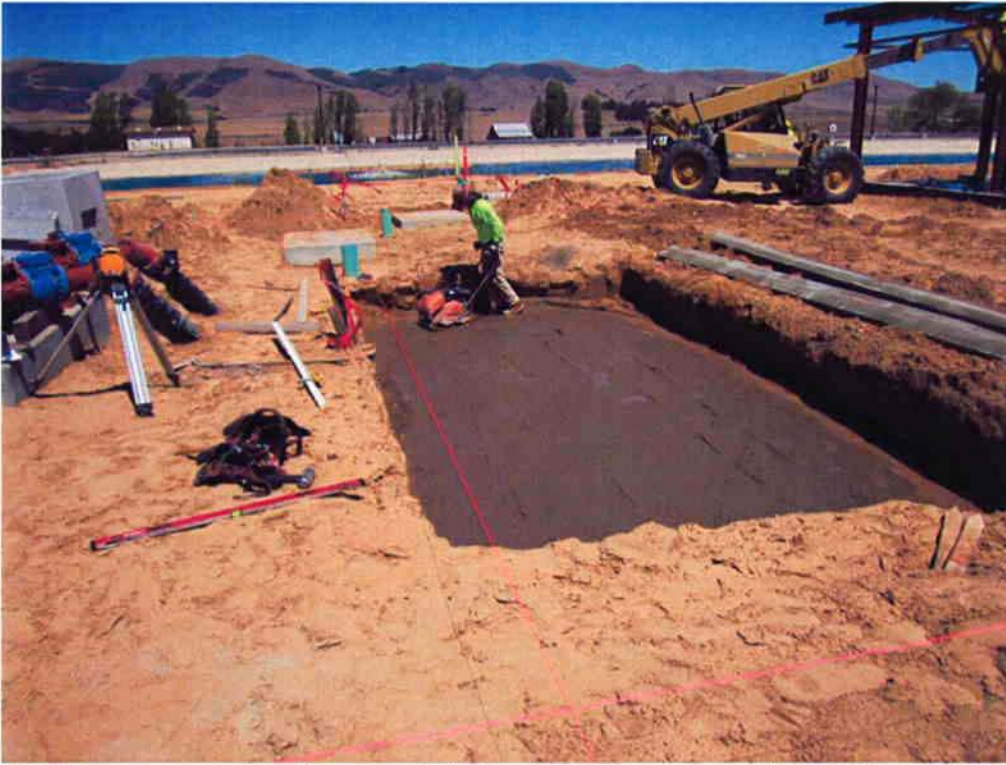
Cushman compacting base material under hydropneumatic tank foundation.
