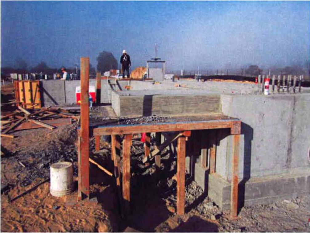
Cushman pouring stair landings at Headworks.
