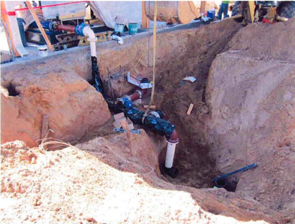
Cushman installing 6-inch WAS and SC piping at Sludge Thickening Building.
