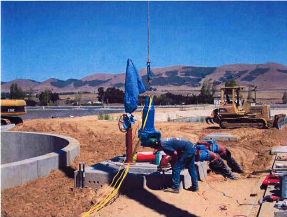
Cushman installing RAS/WAS Pump #1.
