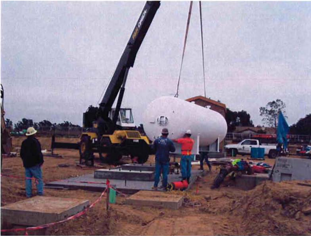
Cushman mounting hydropneumatic tank on supports.
