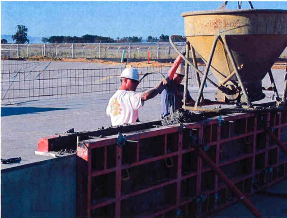
Cushman pouring divider walls at Sludge Drying Beds.
