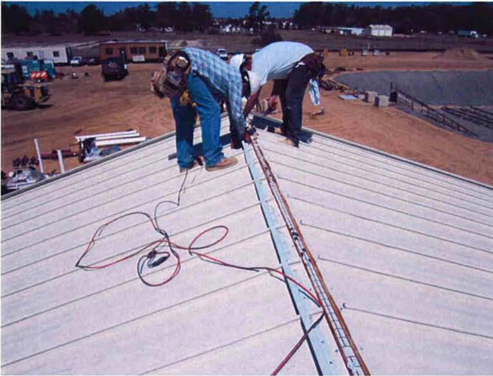
Dueck Roofing installing the ridge on the Electrical/Blower Building.
