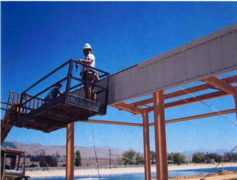
Dueck Roofing installing the shade canopy on the Sludge Thickening Building.
