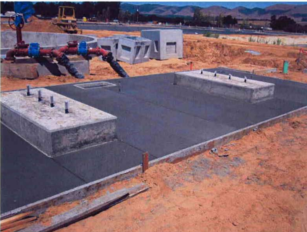
Hydropneumatic tank slab finished.
