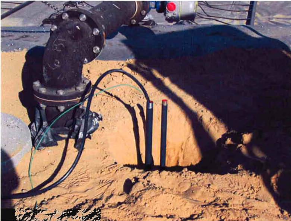
Conduit and wire installed to motorized valves at Aeration Basin.
