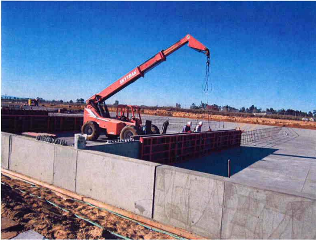
Cushman setting reusable forms for divider walls at the Sludge Drying Beds.
