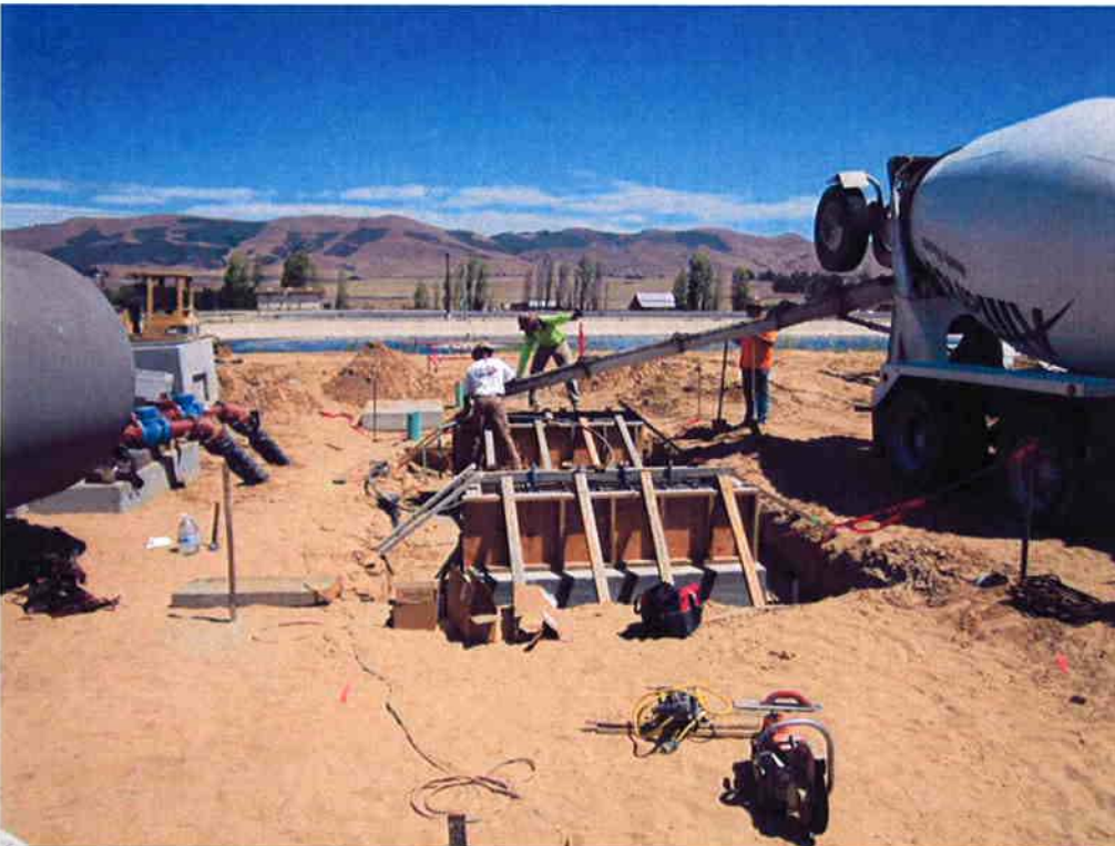
Cushman pouring the hydropneumatic tank supports.
