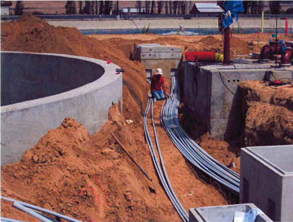
Bergelectric installing Duct Bank 12 (DB 12).
