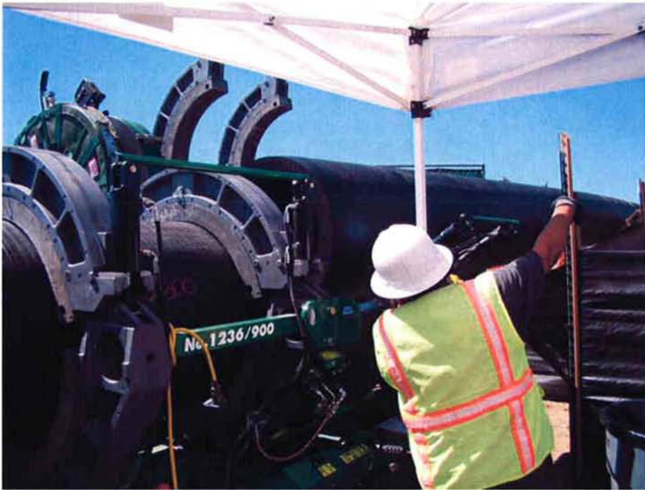
ARB fusion welding operator directing placement of the next section of pipe for welding.
