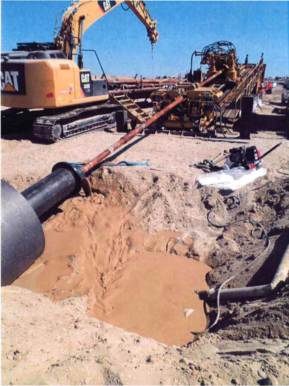
Pilot hole drilling in progress.
