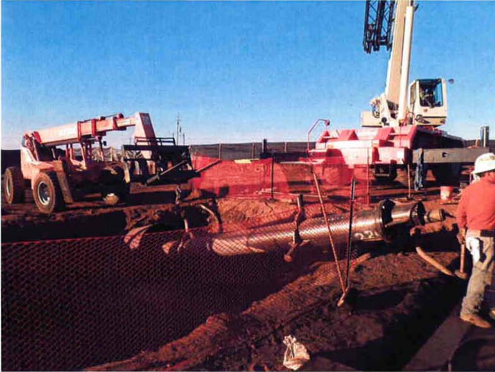
ARB removing centralizer from 54-inch casing to allow the 26-inch drill to come out of the casing.
