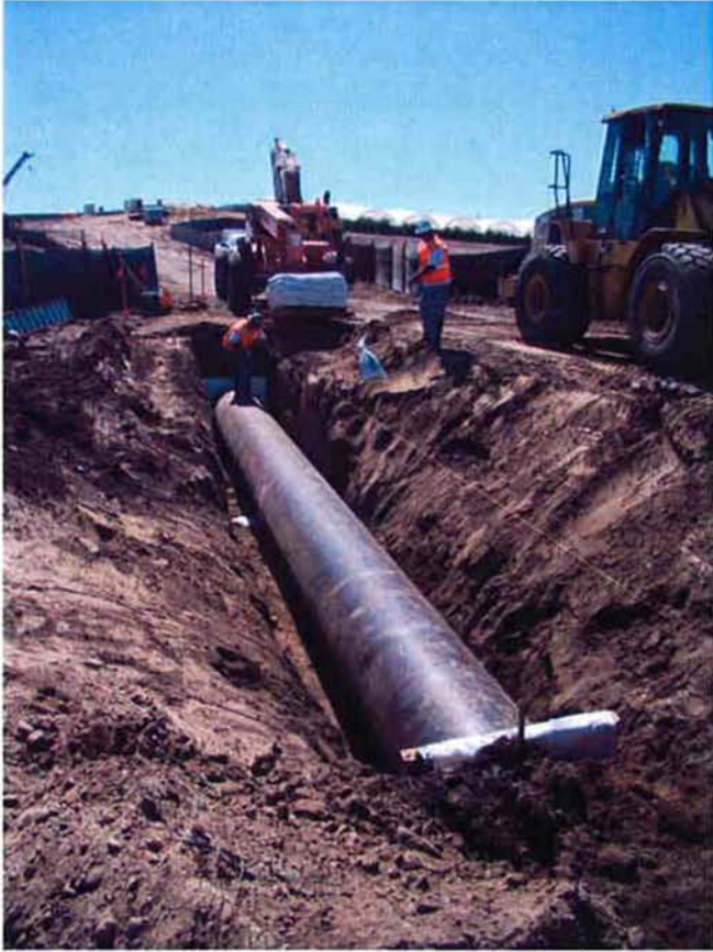
Steel casing installed with ends blocked.
