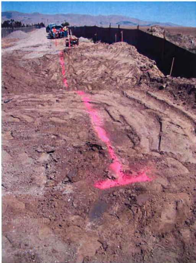
ARB layout for 36-inch diameter steel casing.
