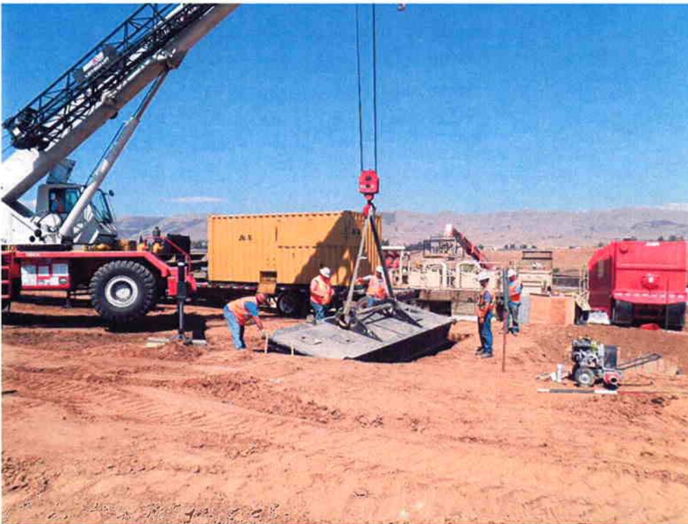
ARB unloading deadman front section which supports the drill rig.
