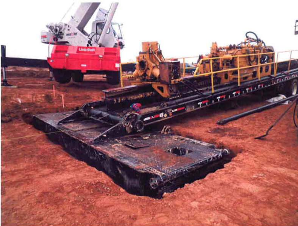
ARB positioning drill rig on front deadman.
