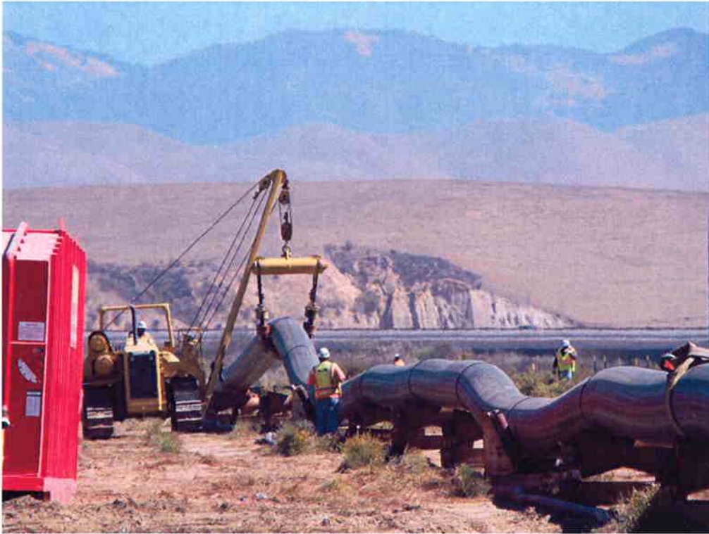
Machine used to pull pipe along rollers when a weld is completed.
