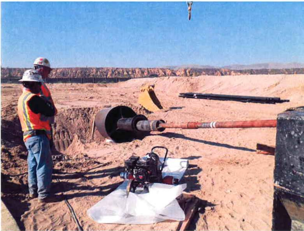
12-inch casing drilled into place inside the centralizer and 54-inch casing.
