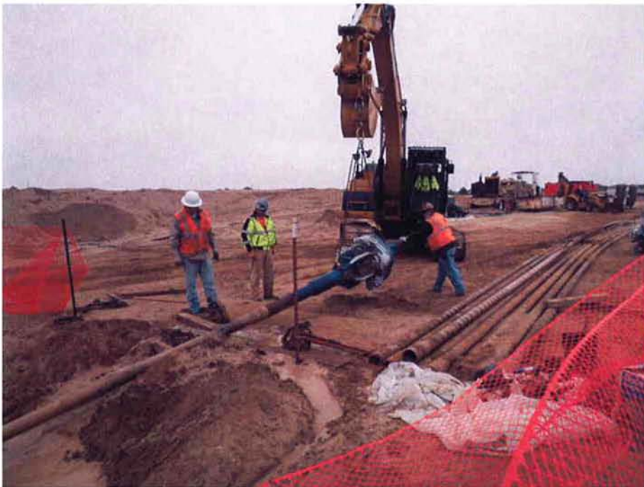
ARB positioning 36-inch drill.
