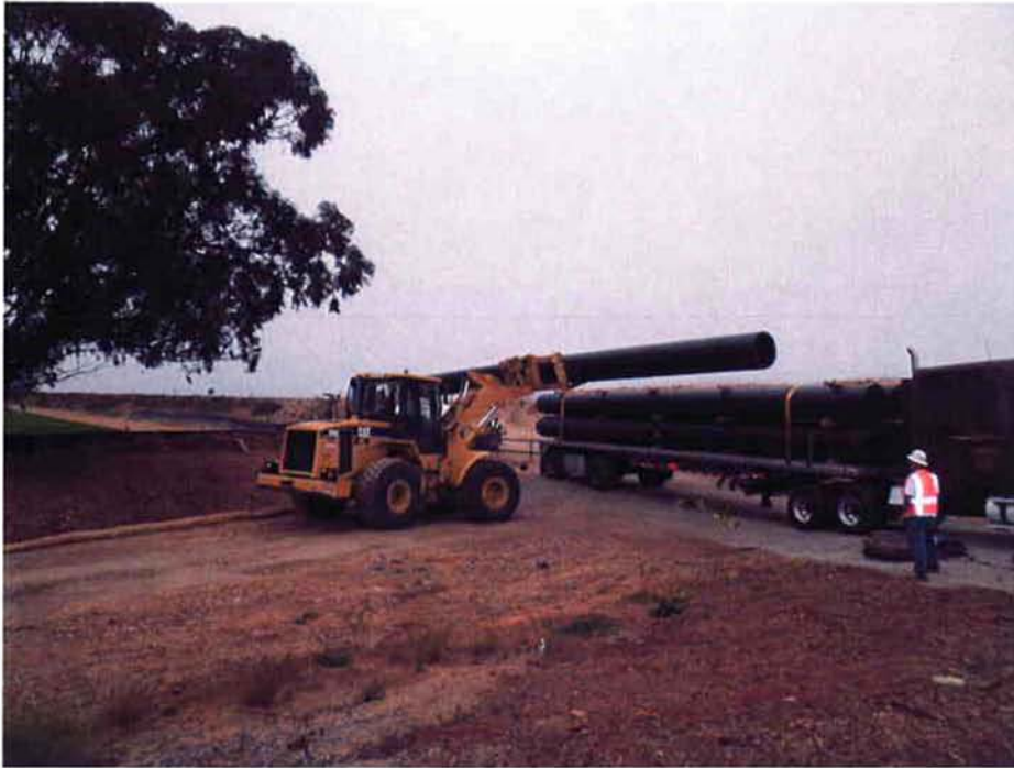
HDPE pipe being unloaded.
