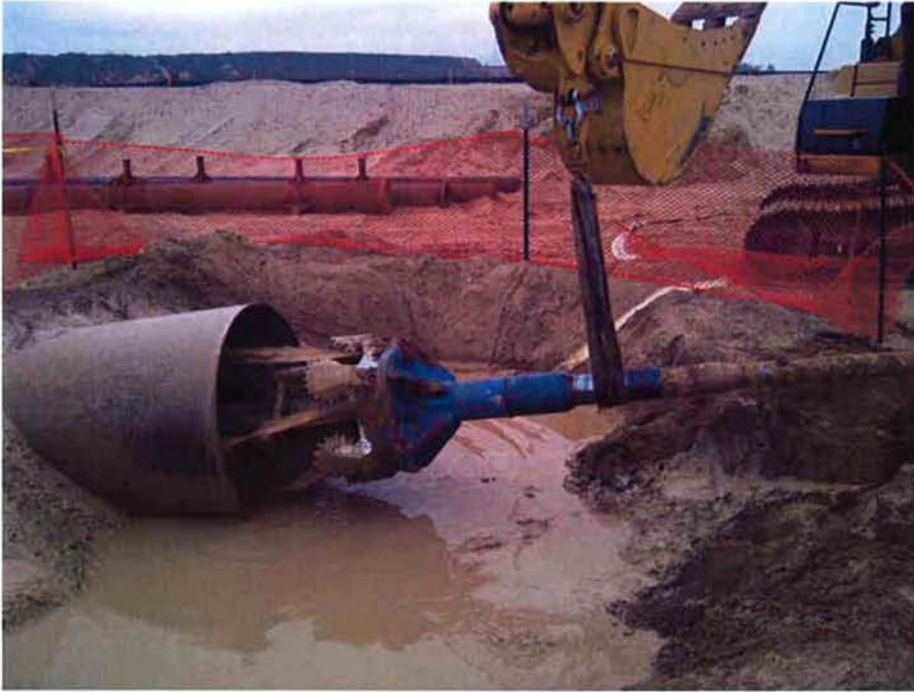
36-inch drill entering 54-inch casing to start next reaming pass from south to north.
