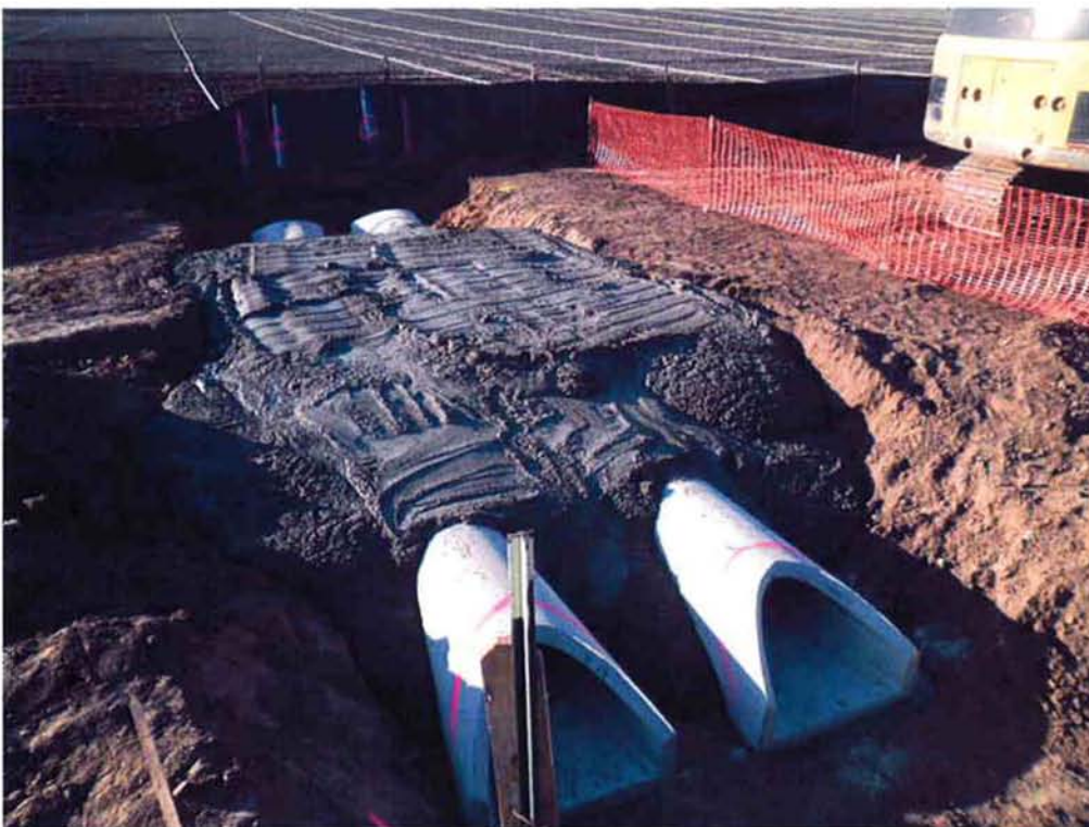
Slurry placed over the 18-inch RCPs.
