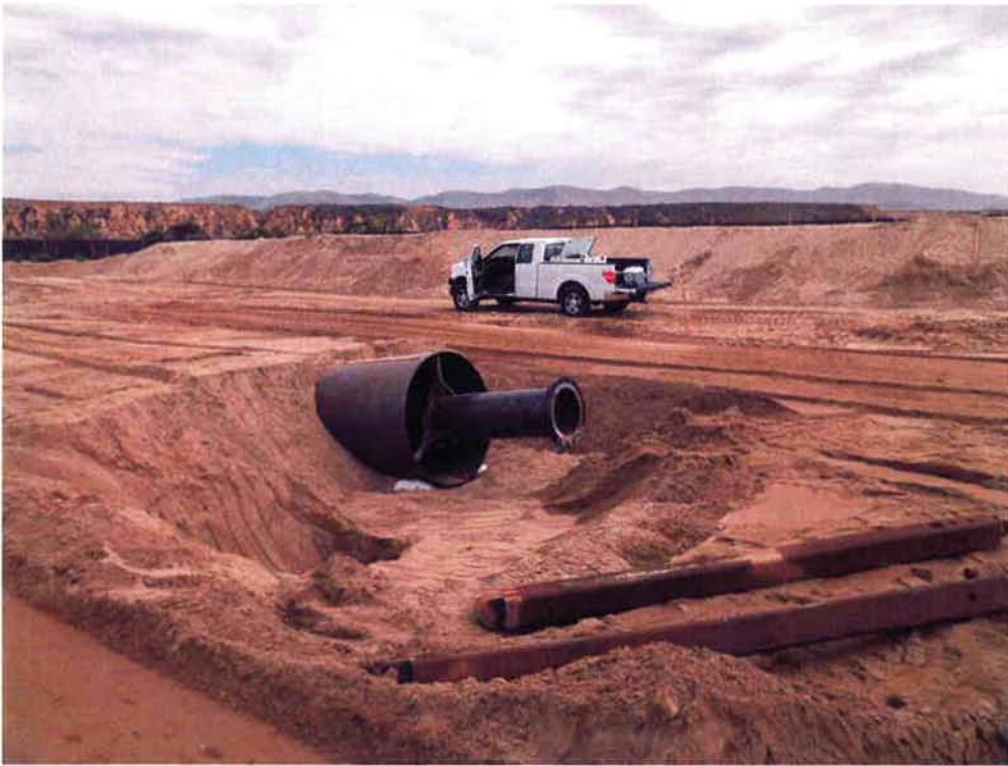
54-inch casing with centralizer installed.
