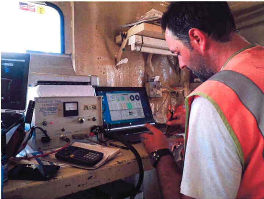
Horizontal Technology, Inc. surveyor in control room monitoring progress of pilot hole drill.
