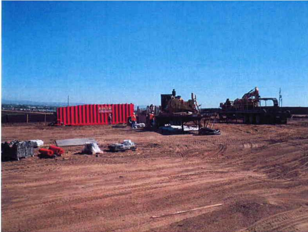
ARB drill equipment mobilizing to north site.
