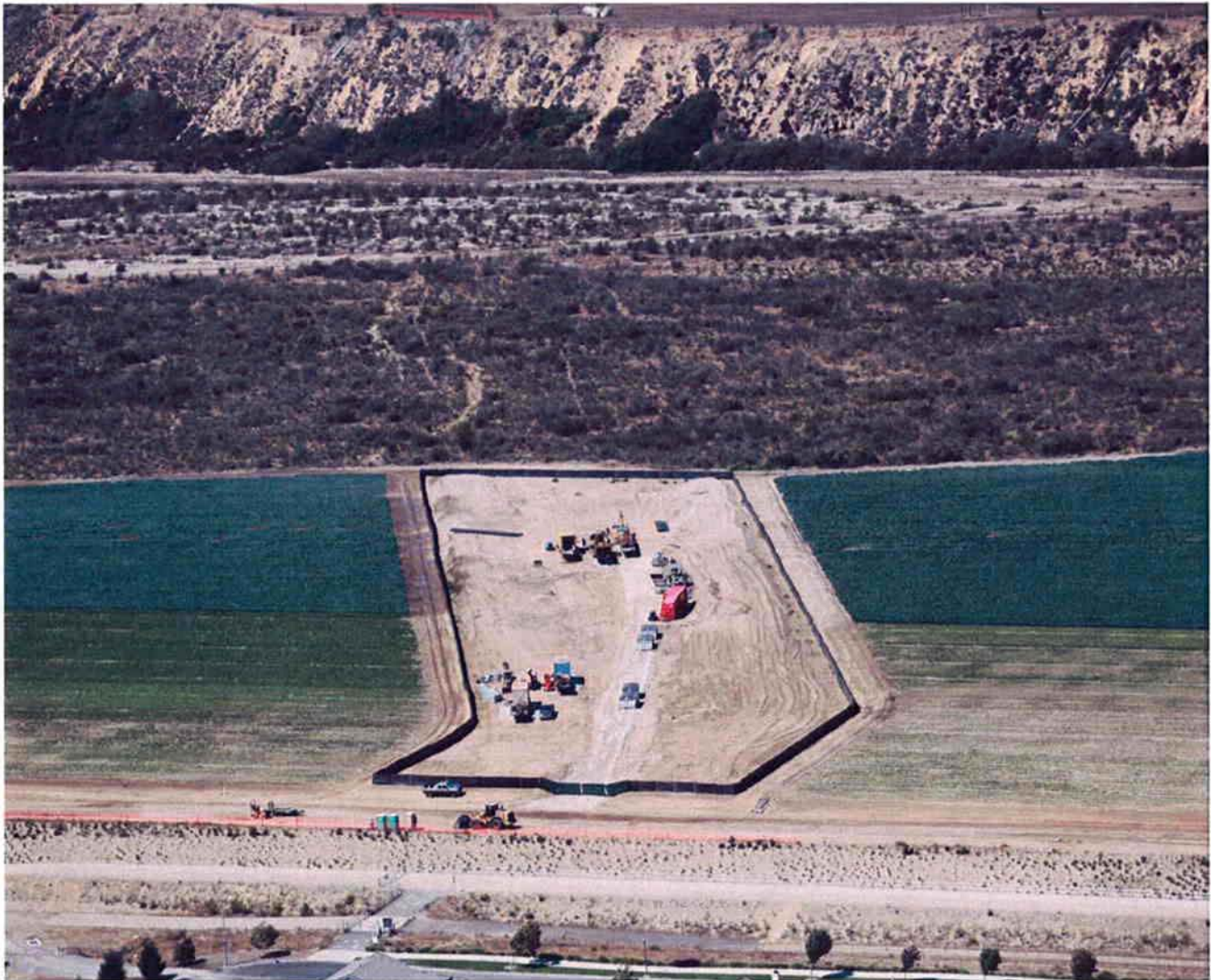
Aerial photo of the south side with ARB drill rig and equipment mobilized.
