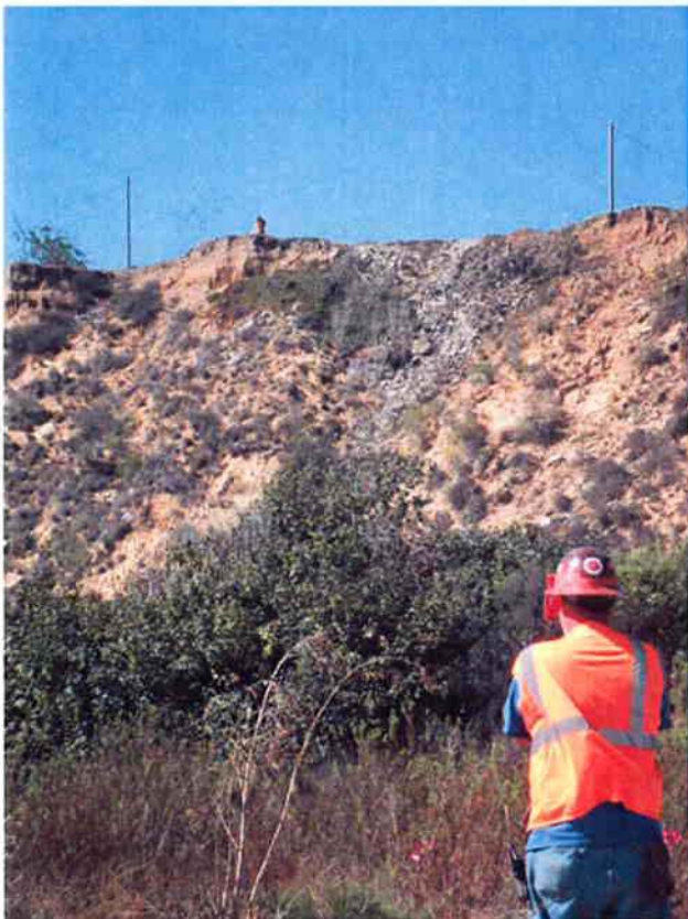
Surveyors from Horizontal Technology, Inc. placing stakes for tracing wires by using MNS Engineers survey stakes for pipe centerline.
