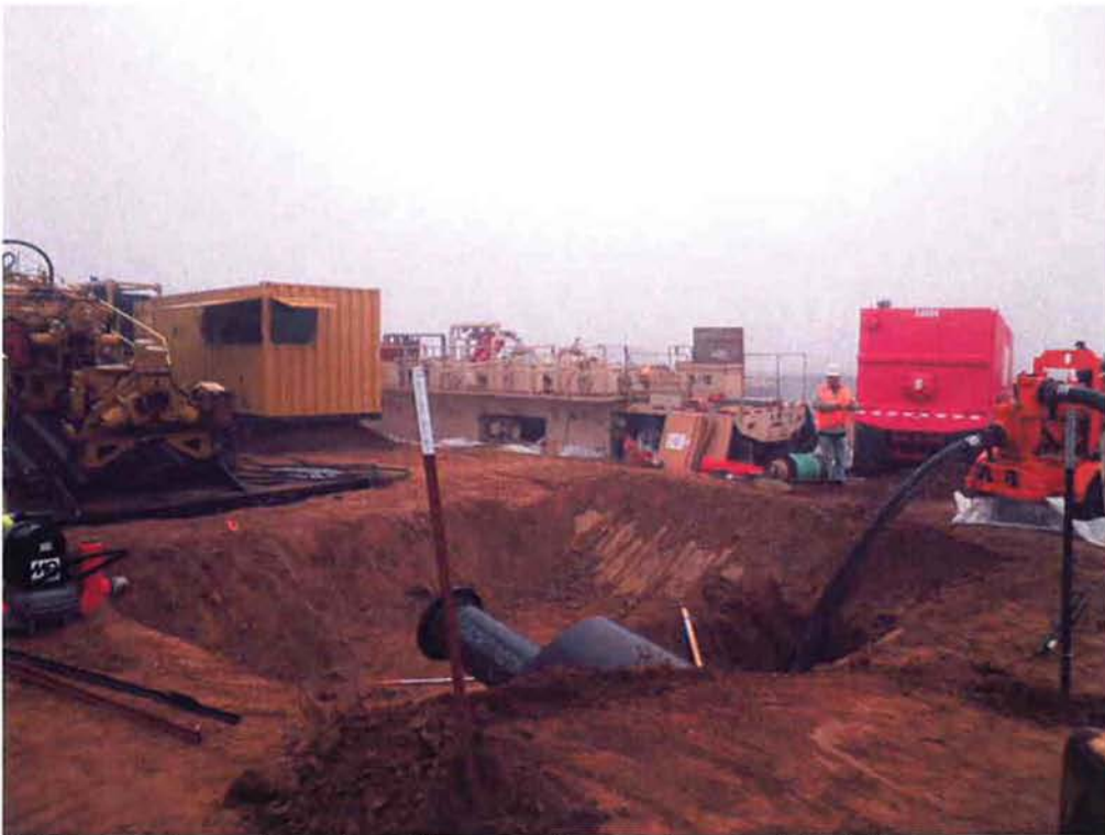
Drilling equipment, casing with centralizer and mud pit installed.
