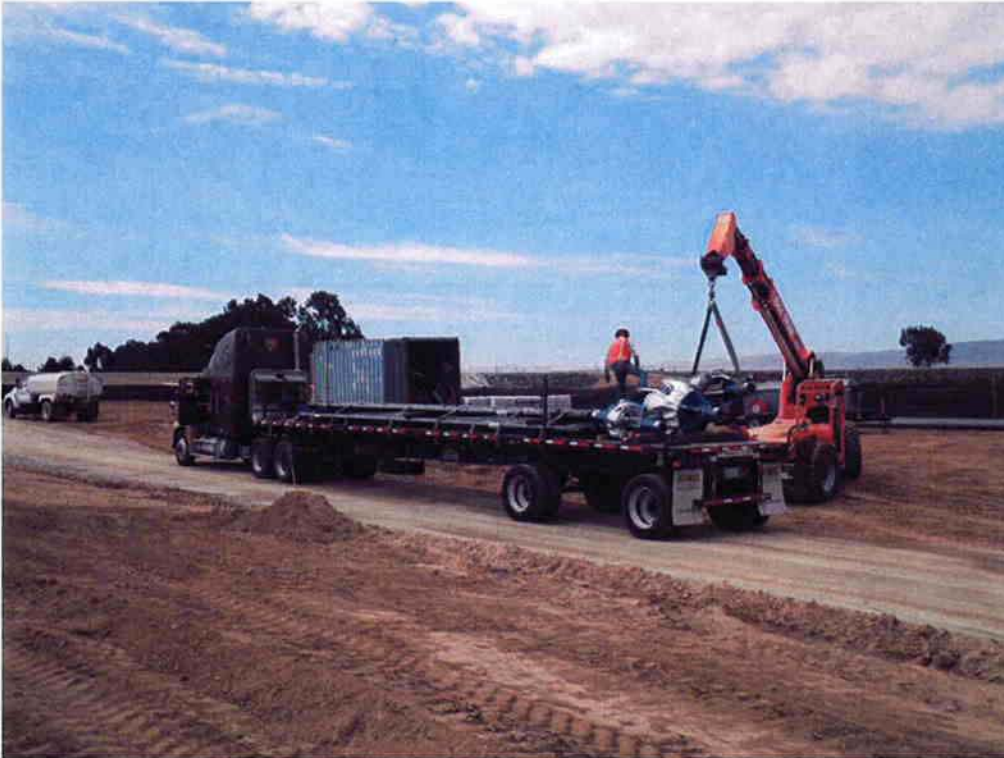
Drill heads delivered to site.
