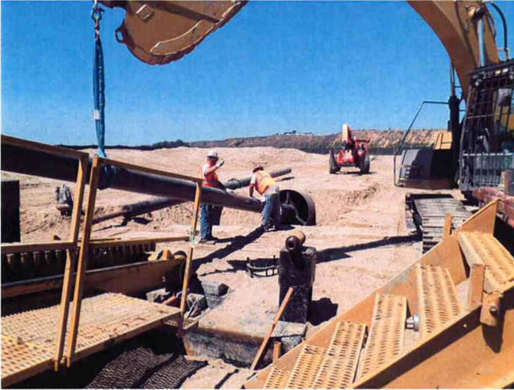
ARB installing 12-inch casing with steel "teeth" into centralizer.
