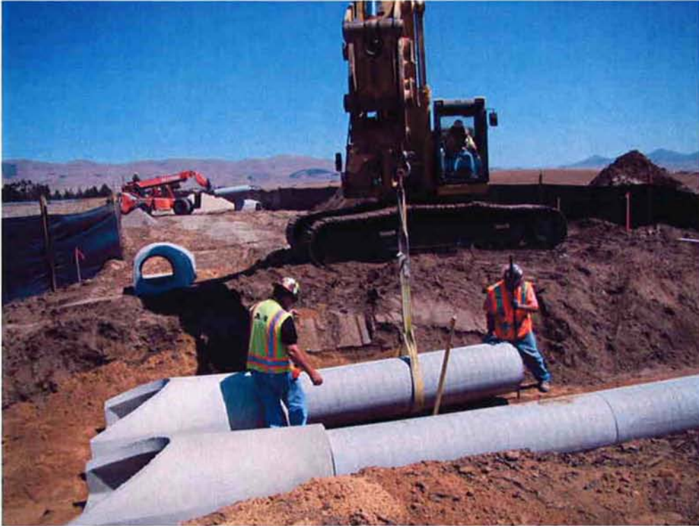
ARB installing the 18-inch RCPs with flared ends over the steel casing.
