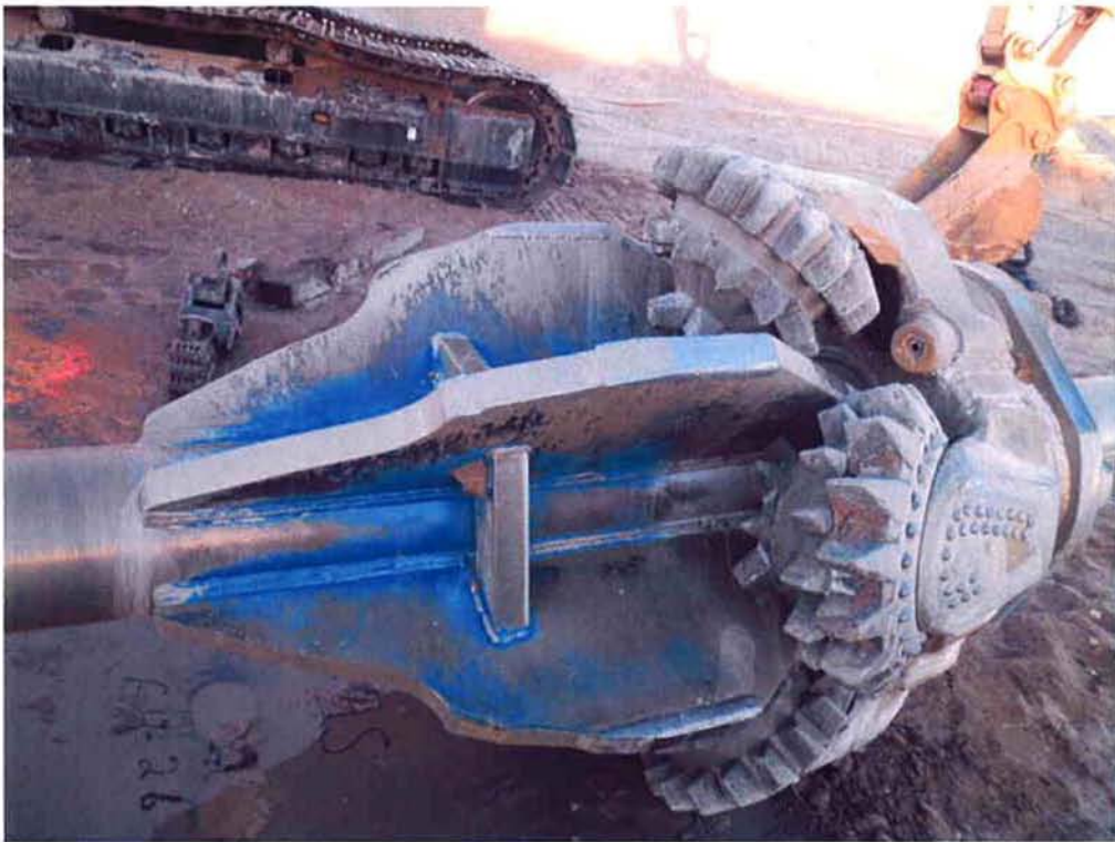
The 42-inch drill removed prior to completion of the reaming pass from south to north, after difficulty drilling through cobble, rock and the Paso Robles formation.
