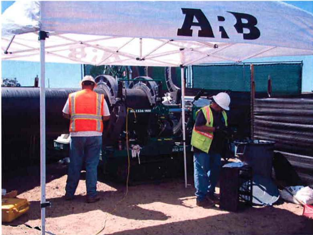
ARB fusion welding equipment and operator welding the HDPE carrier pipe.
