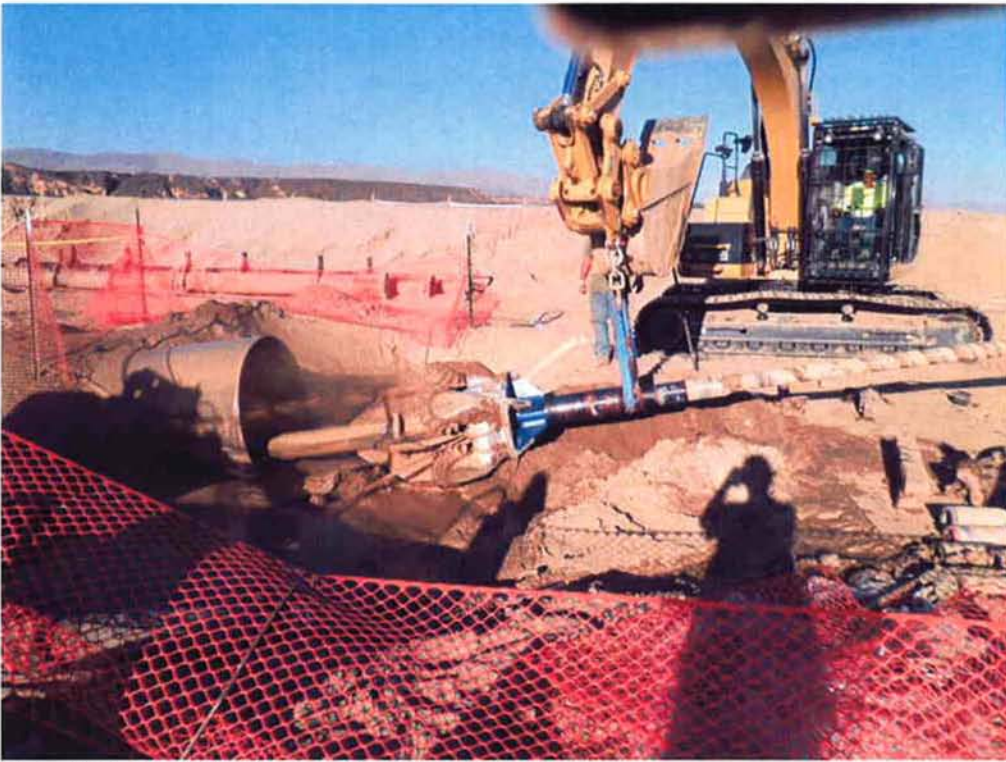
The 42-inch drill entering the 54-inch casing.
