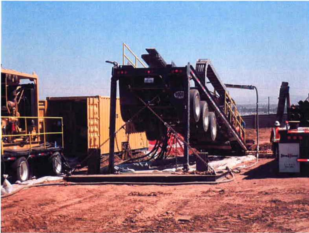
Drill rig being raised into place from rear deadman.
