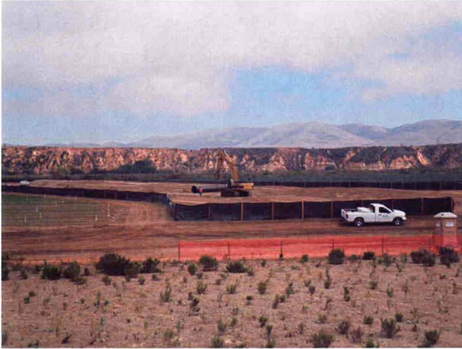
ARB mobilizing the casing to the drill entrance area for installation.
