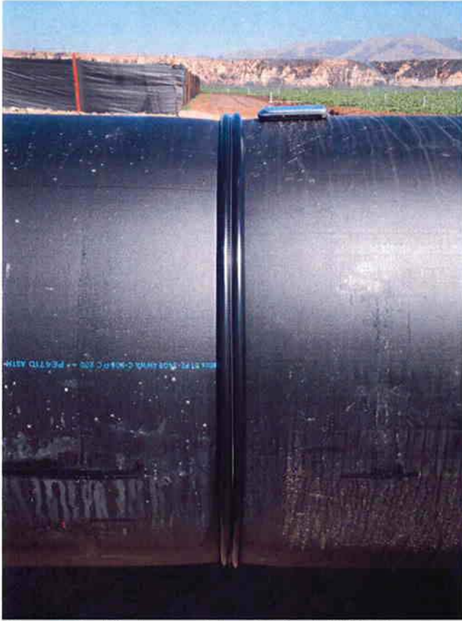
Completed fusion weld on 24-inch HDPE carrier pipe (outer diameter 30-inches).
