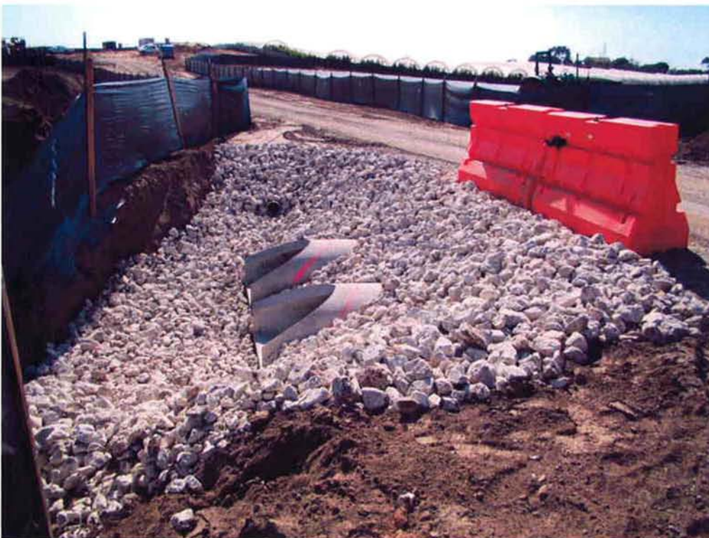
Rock rip-rap placed at both flared ends of the 18-inch RCPs to control erosion.
