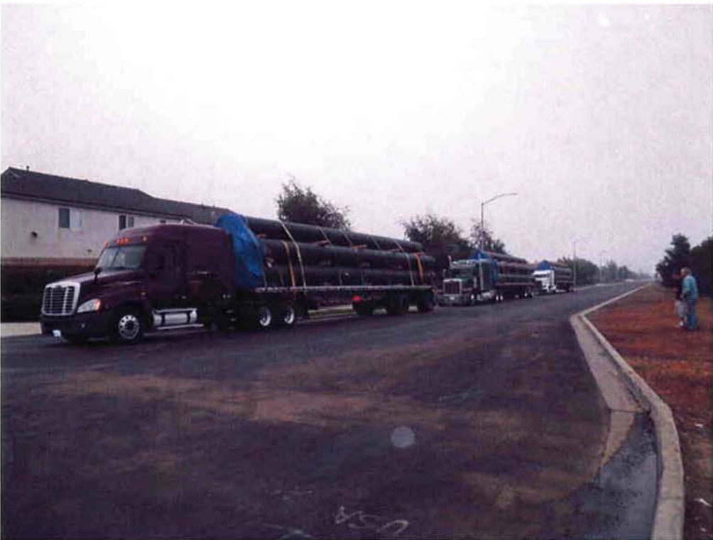
HDPE pipe arriving on site.
