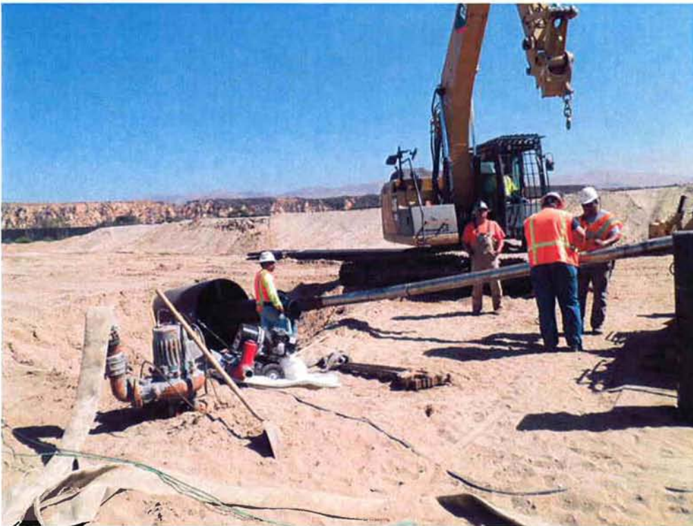
ARB preparing to start the pilot hole drill.
