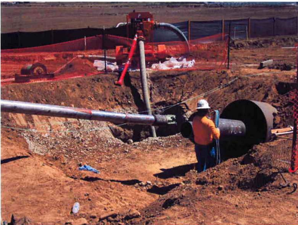
Starting pilot hole drill from the north site after demobilizing from the south site.
