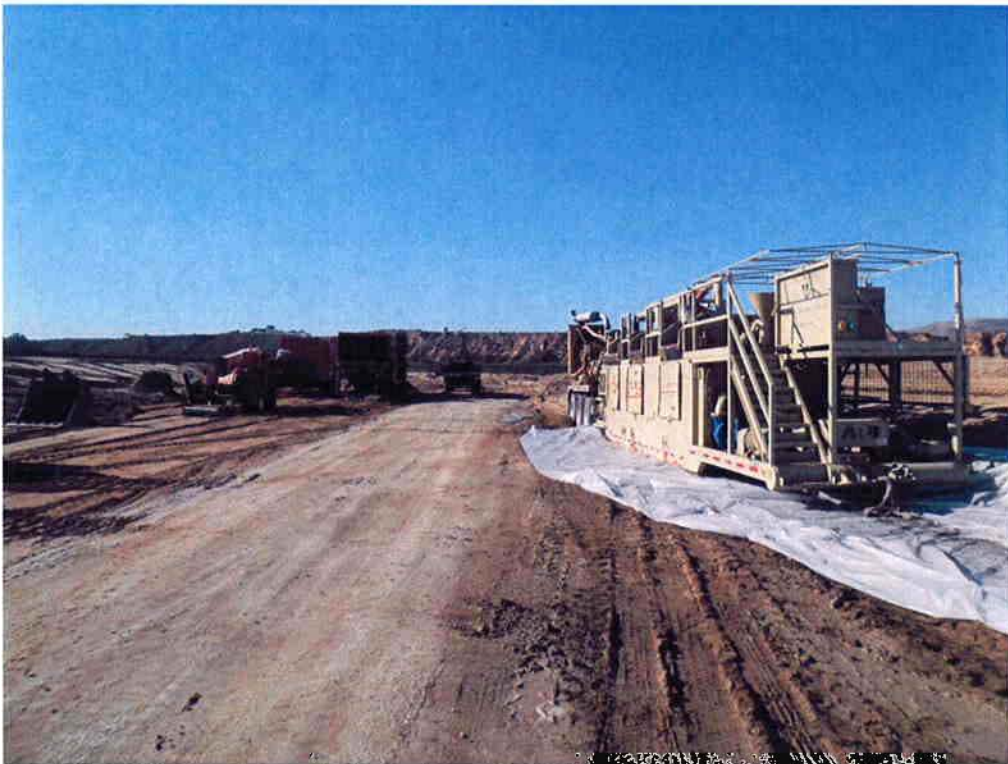
Mud cleaning equipment placed on plastic for environmental protection.
