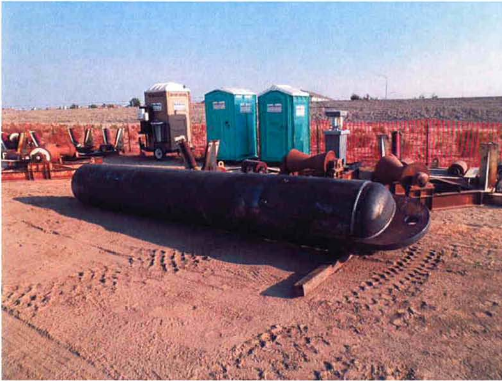
Pull head delivered to site.
