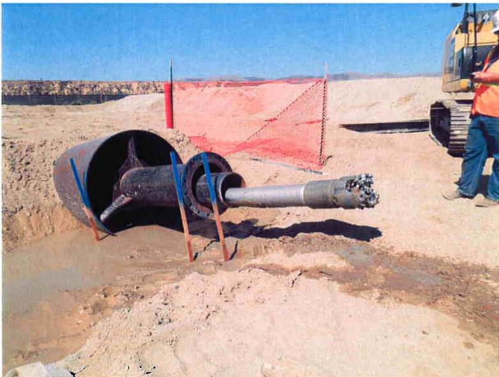
12-inch drill emerging from casing on south site, after drilling from the south site was terminated and started again for a successful completion from the north site to the south site.
