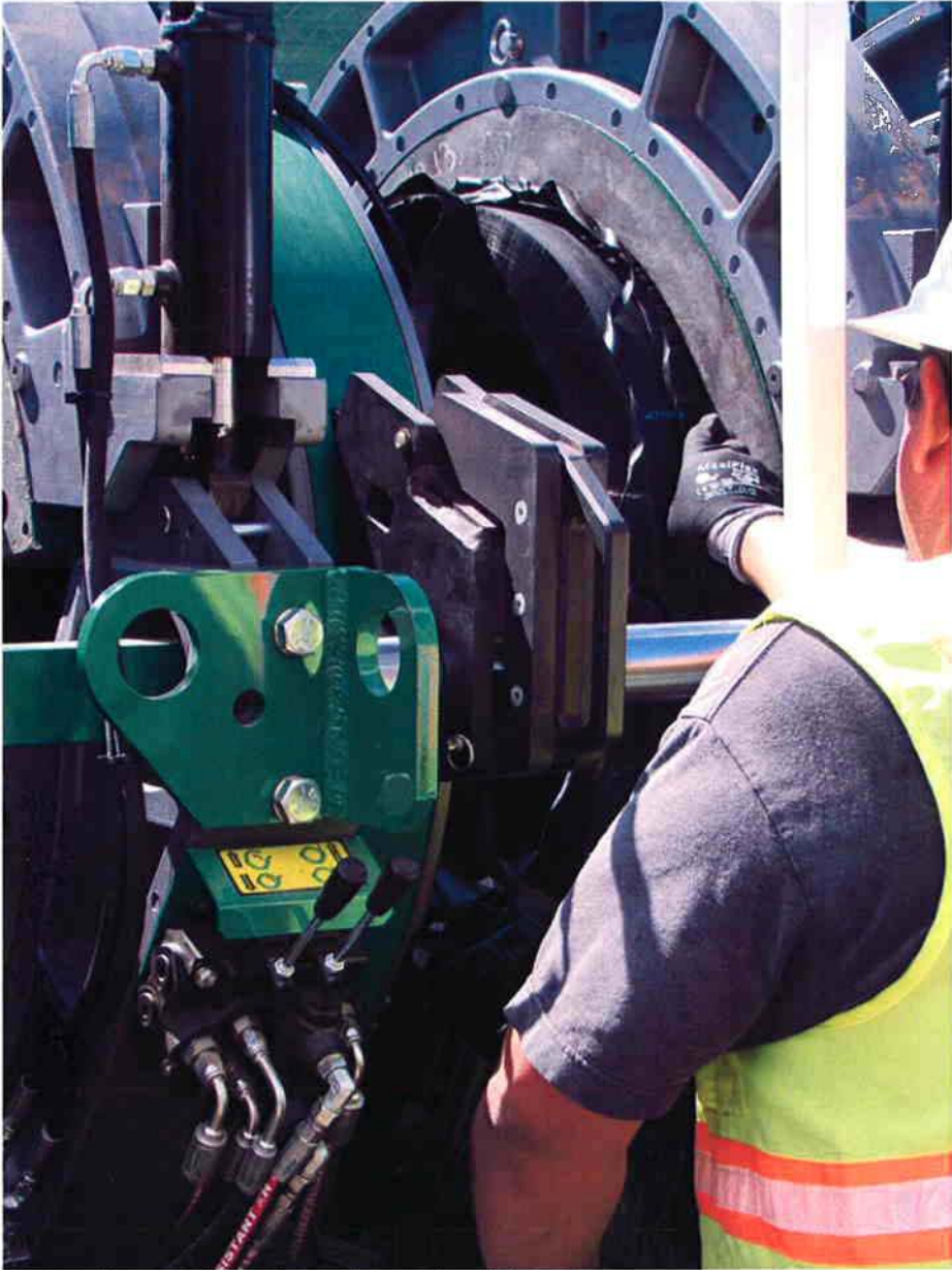
Removing cuttings from the ends of the pipe.
