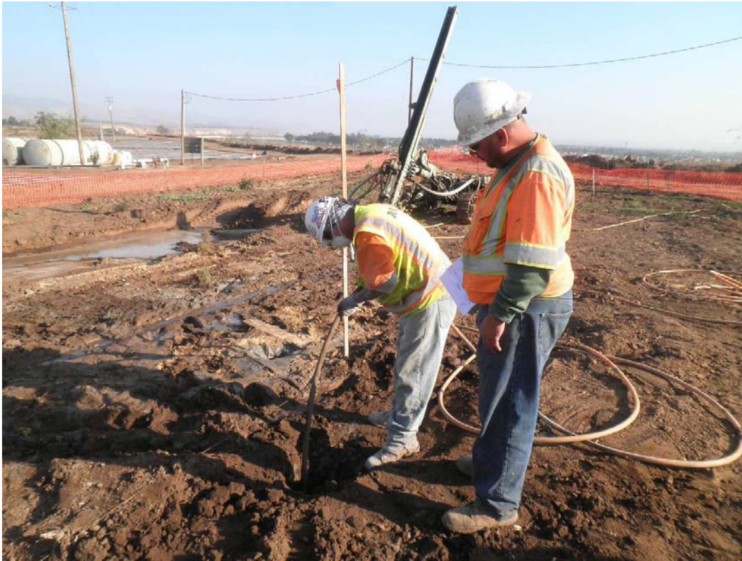
GeoGrout backfilling drill hole with cement grout.
