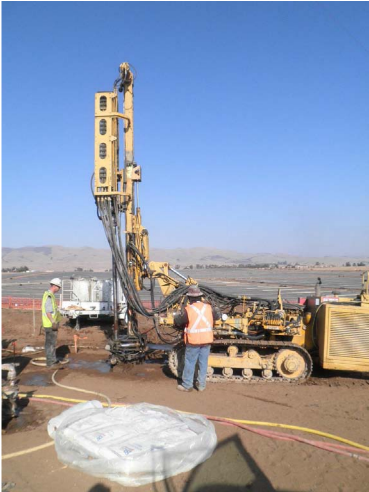
GeoGrout continuing permeation grouting injections.
