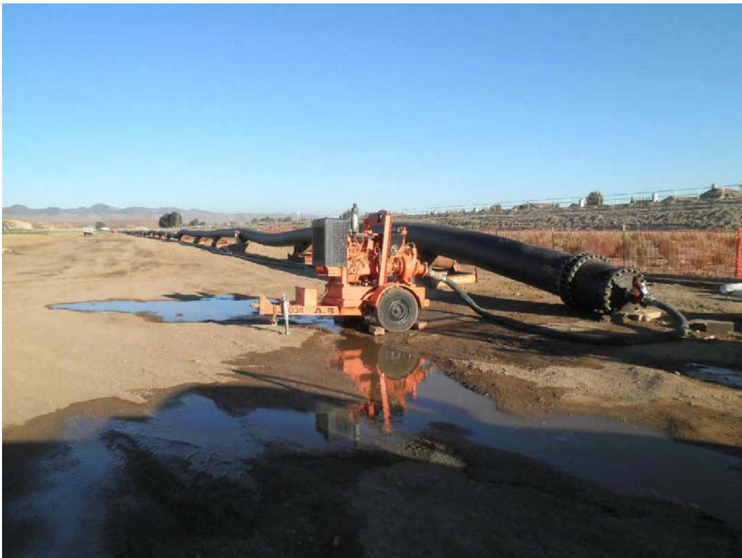
Pumping water out of HDPE pipe after successful hydrostatic pressure test.
