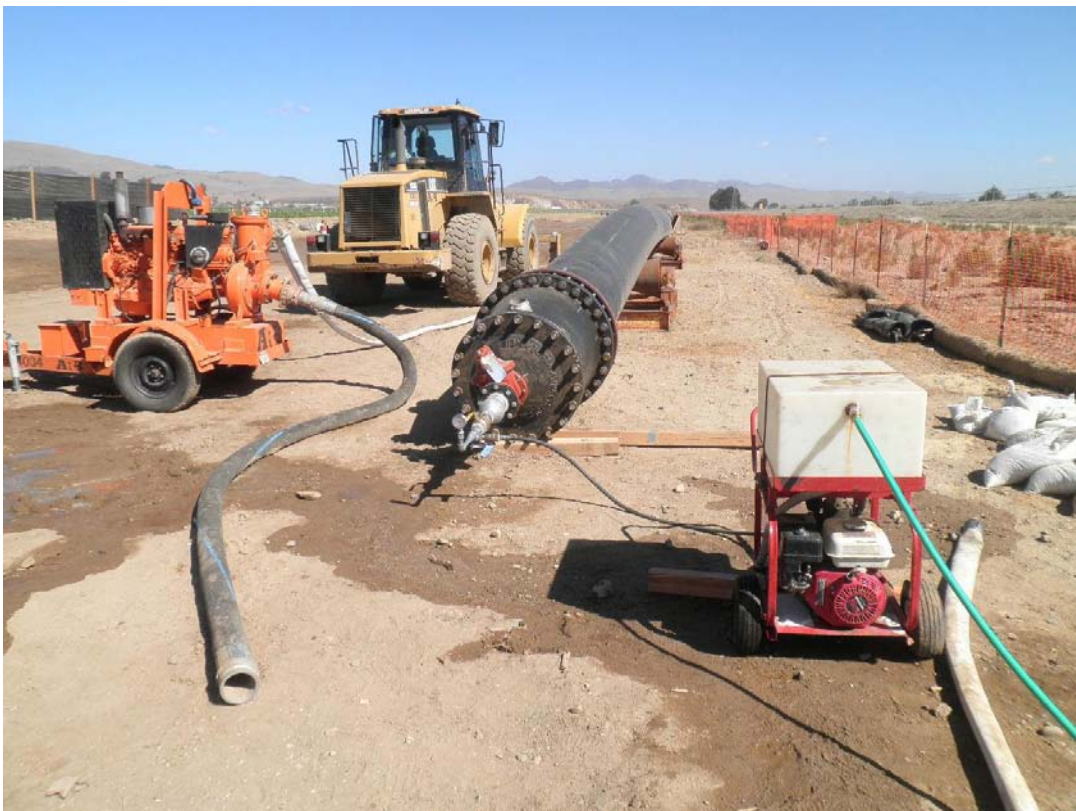
Pressurizing the HDPE pipe for the hydrostatic pressure test.
