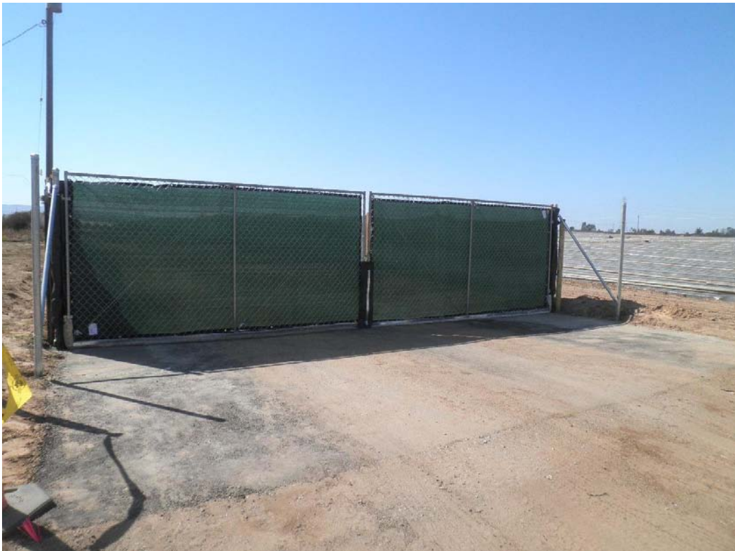
Gate installed by ARB to prevent CRLFs from entering the site.
