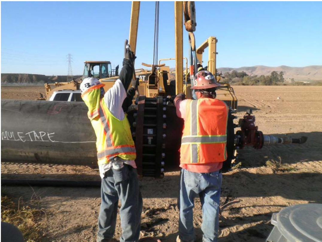
ARB bolting test fitting to the east end of the HDPE pipe.
