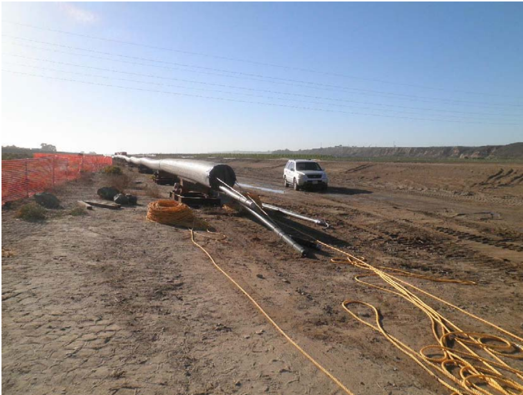
Ballast and vent pipes successfully inserted into HDPE pipe.
