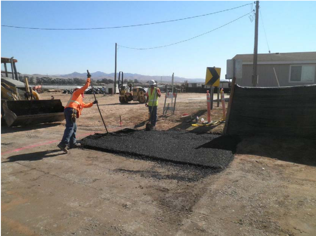
R. Burke Construction placing an AC apron under the gate to prevent CRLFs from entering the site.
