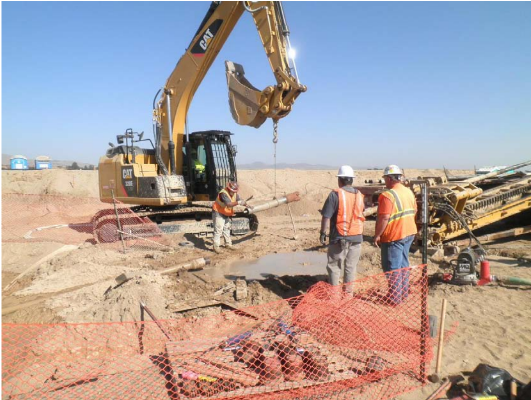
ARB installing 9-inch drill/mud jet to loosen the 42-inch drill.
