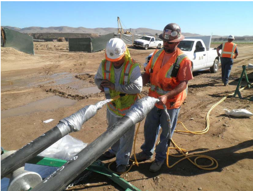
ARB attaching rope to the two 4-inch ballast and vent pipes in preparation for inserting them into the HDPE pipe.
