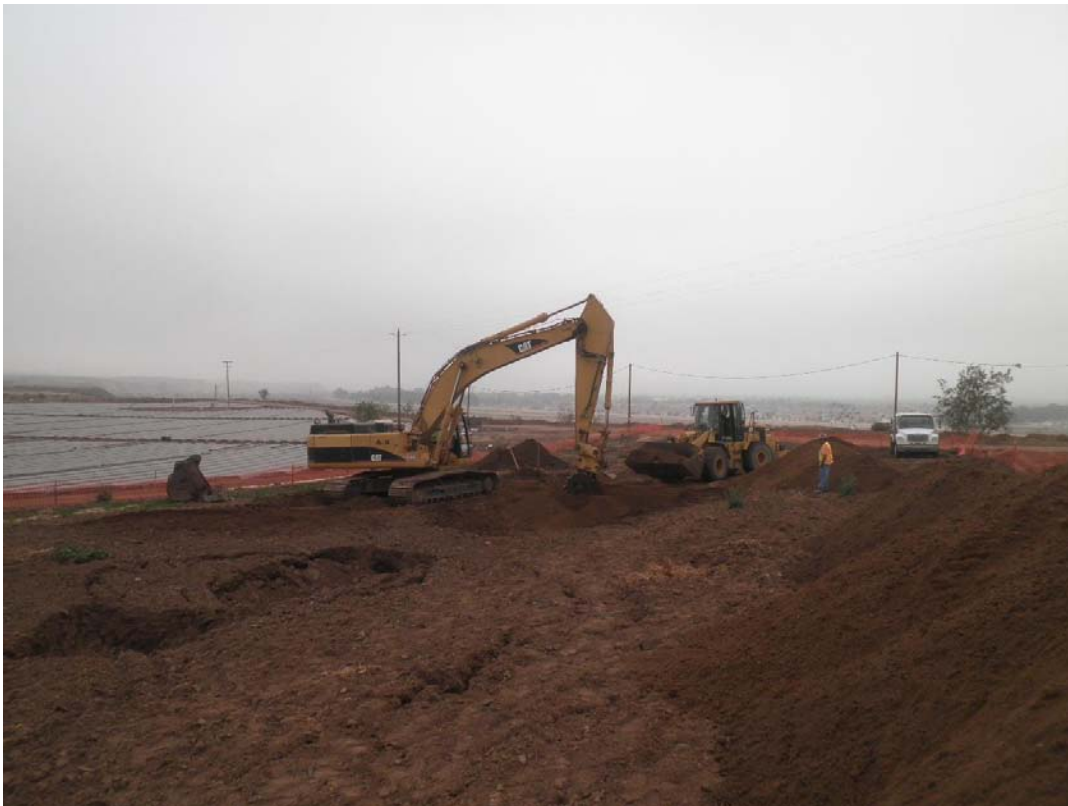
ARB backfilling sink holes with imported material in preparation for GeoGrout mobilization.
