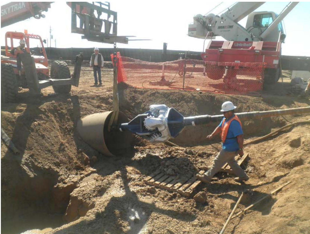
ARB inserting 42-inch drill for final attempt at completing the reaming from the north side on October 21.
