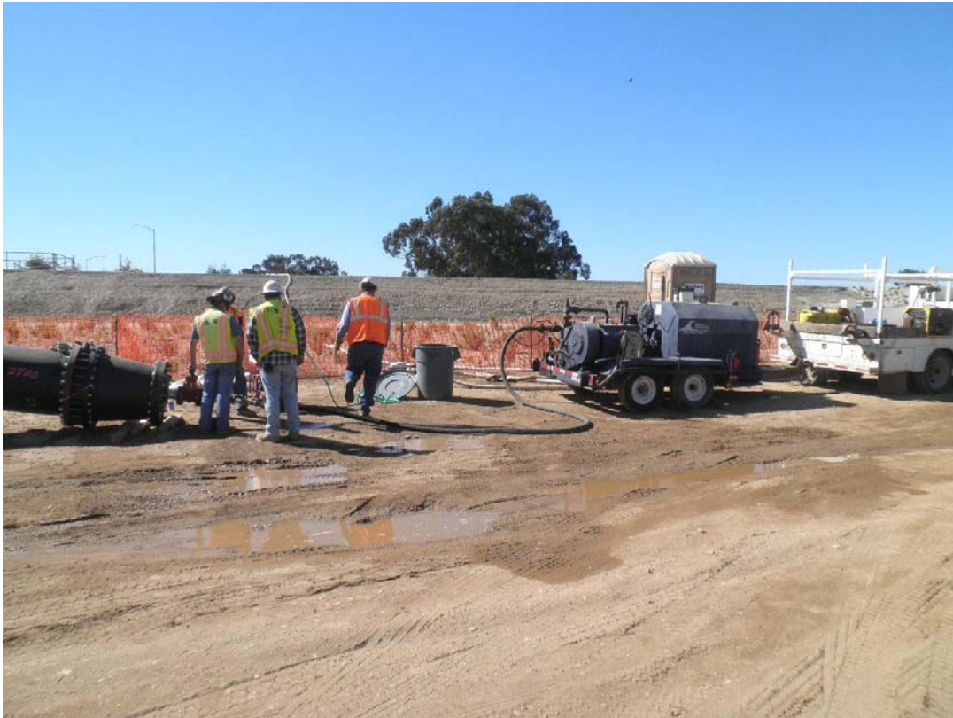
New pump brought in by ARB to reach hydrostatic test pressure of 152.5 psi.
