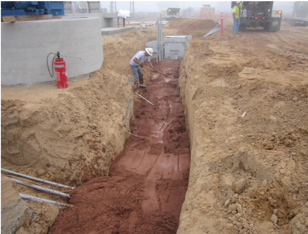
Bergelectric placing red slurry over DB 02.
