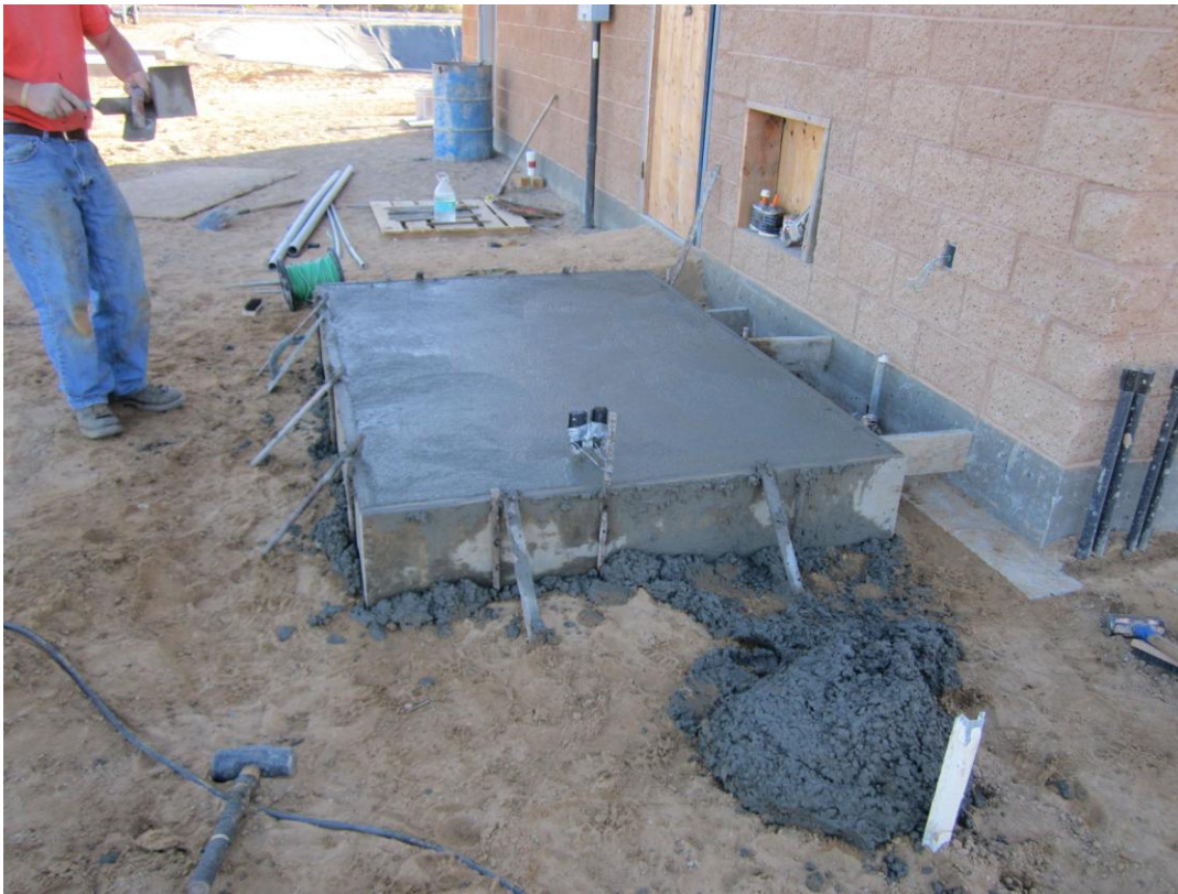
Cushman finishing the concrete slab for the air conditioning unit to the MCC room.
