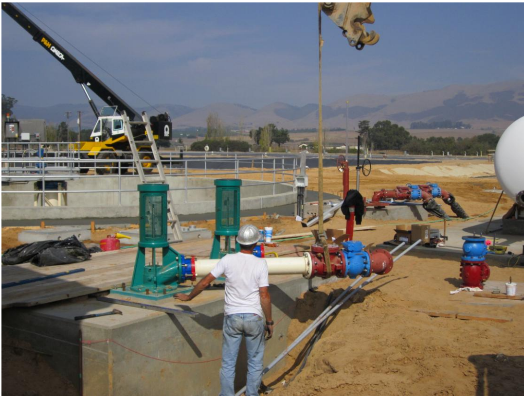
Cushman assembling NPW pipe from the Process Water Pump Station.
