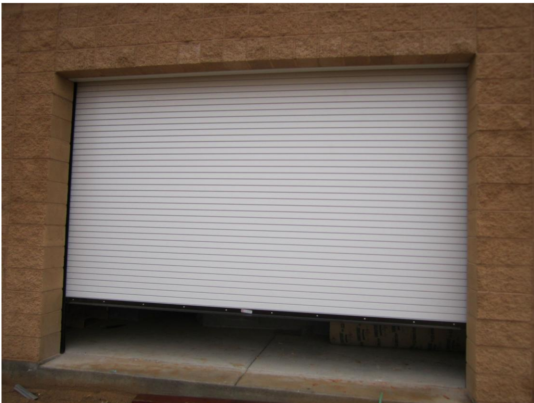
Roll-up door to blower room installed by Hamon Overhead Doors.
