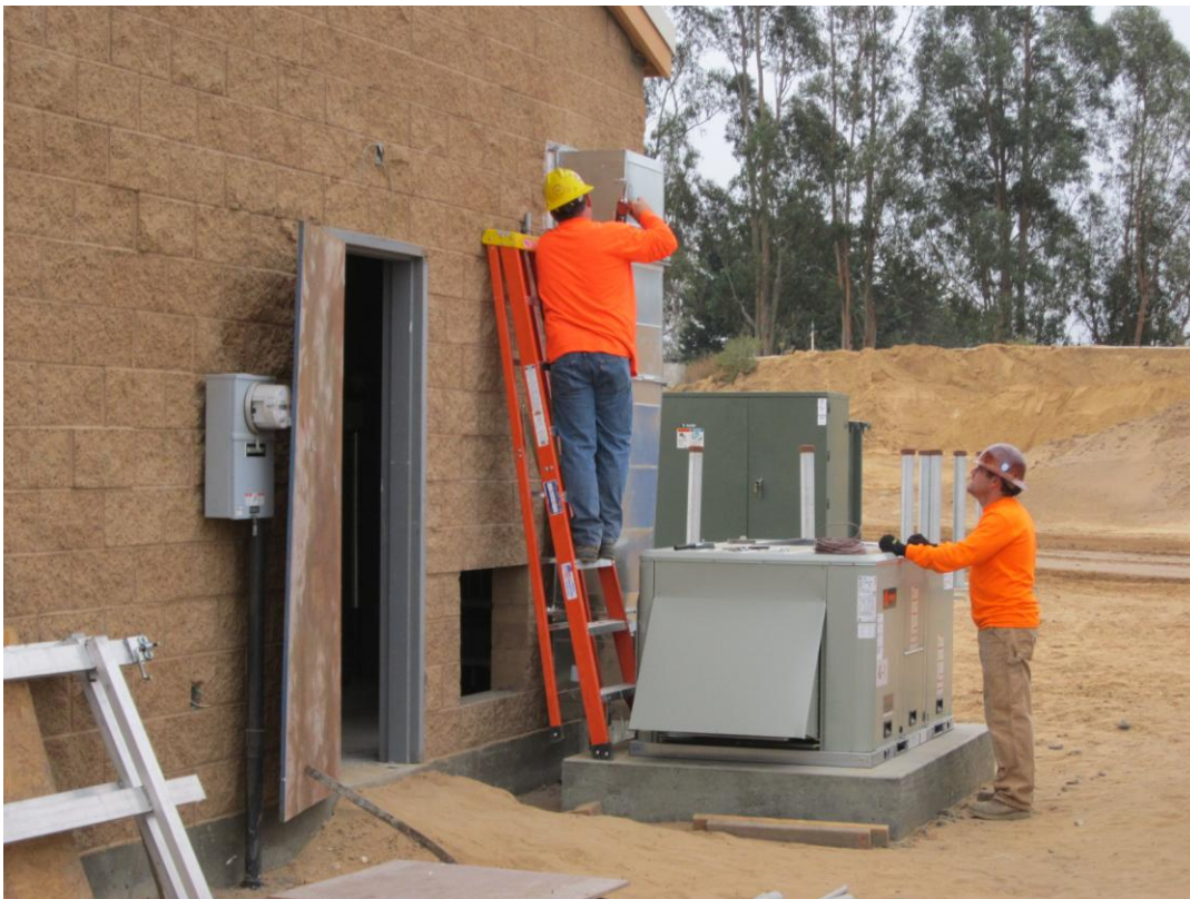
Cushman subcontractor Longs Construction installing the AC unit and ducts to the MCC room.
