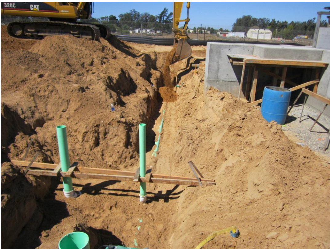
Installing 6-inch DR along Grit Classifier.
