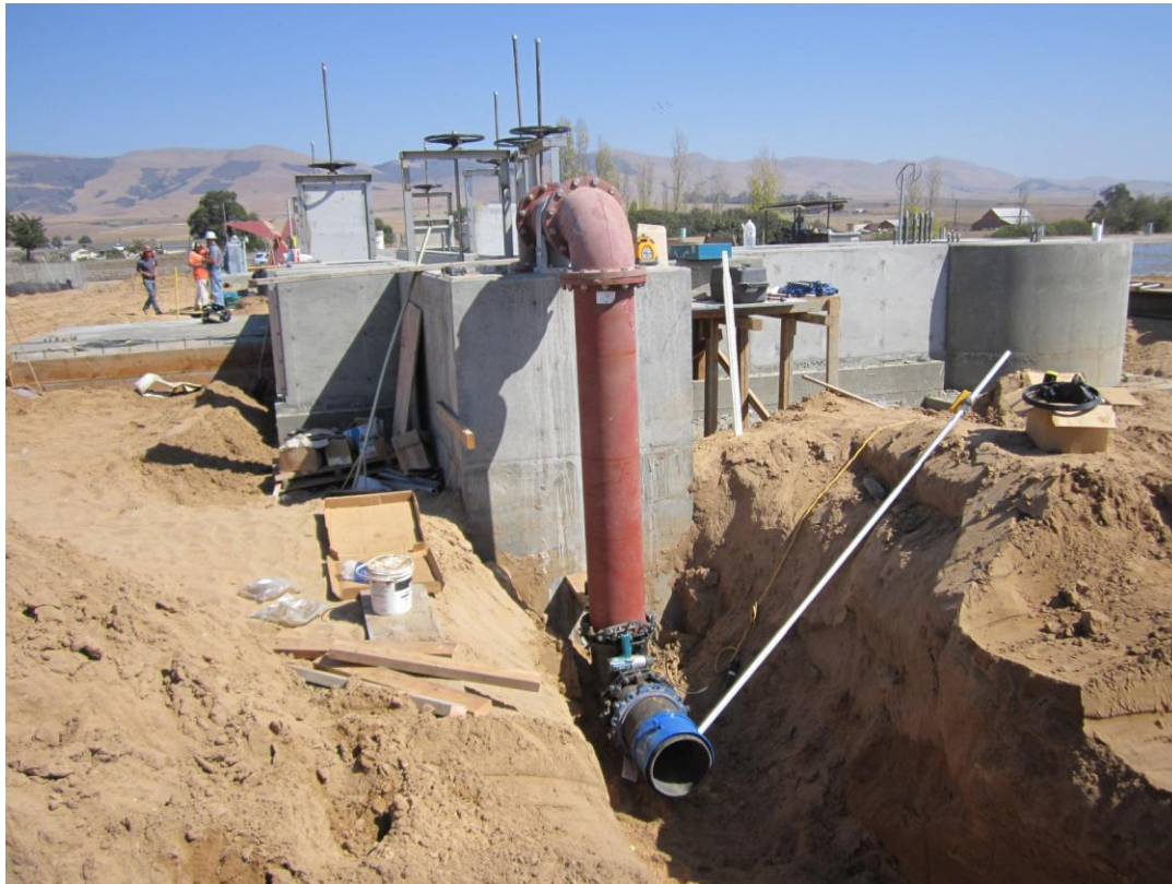
Installing 12-inch RAS piping from the Headworks.
