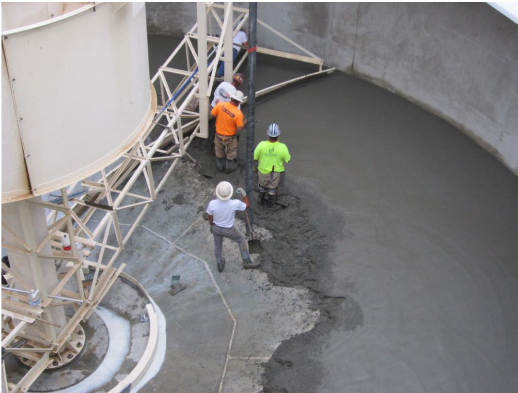
Cushman spreading grout in Clarifier #1.
