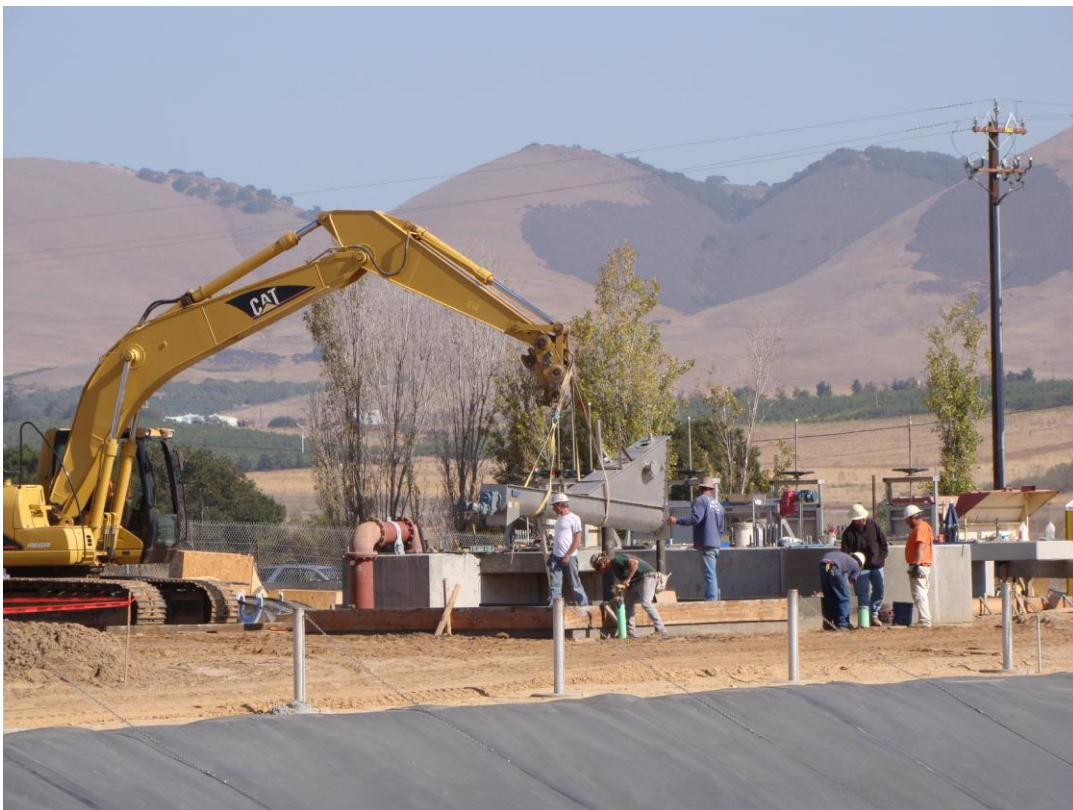
Cushman setting the Grit Classifier on the slab.
