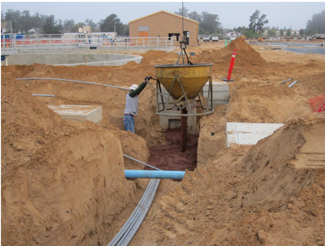
Bergelectric pouring red slurry over DB 11 and DB 12.
