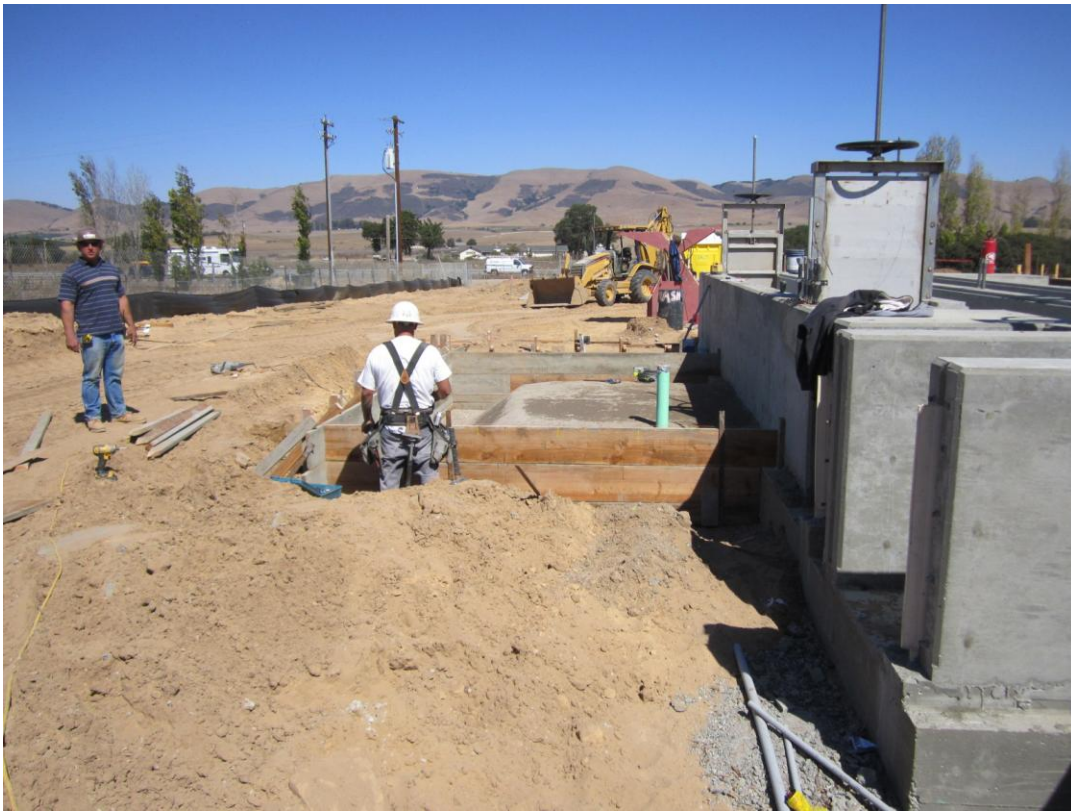
Cushman forming the trash enclosure slab at the Headworks.
