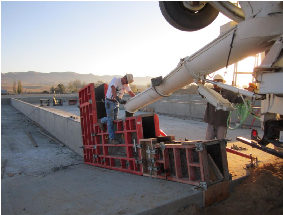
Cushman pouring ramp walls at Sludge Drying Beds.
