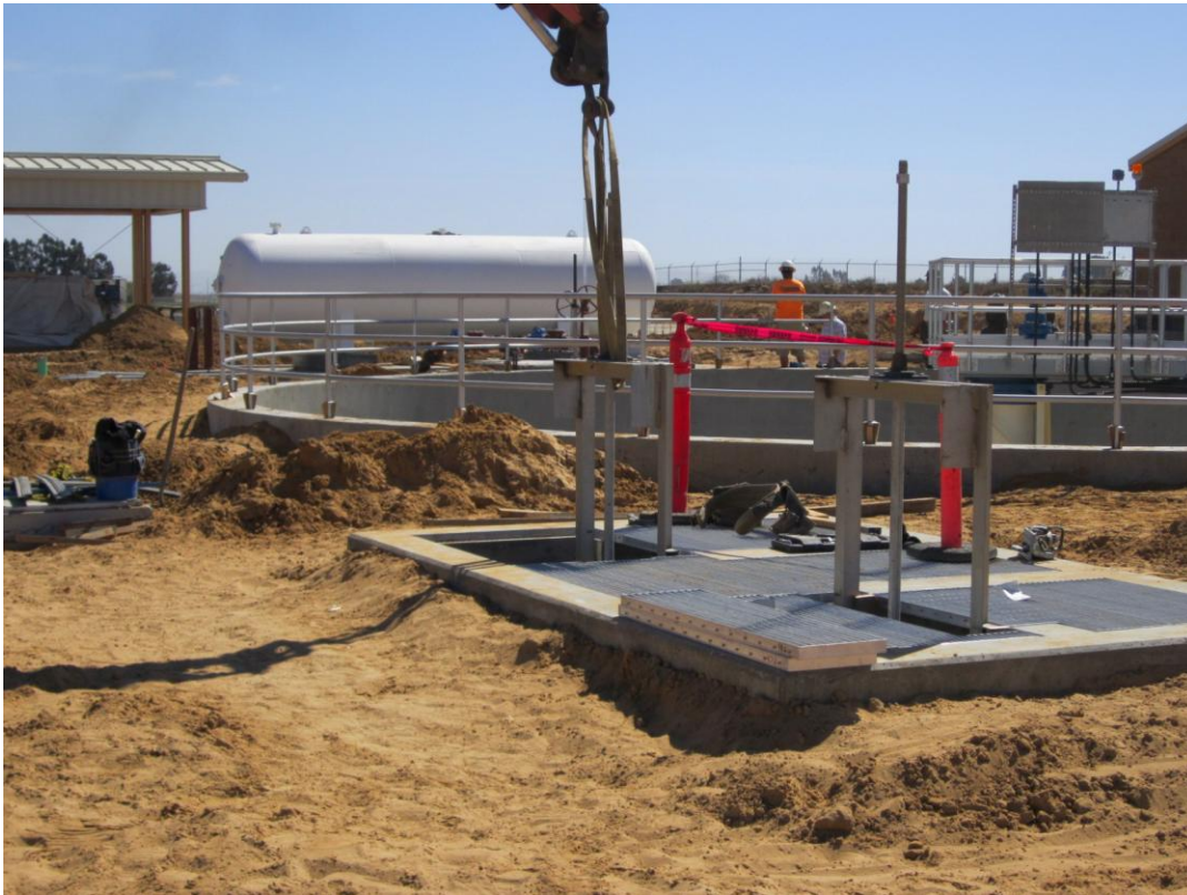
Installing slide gates at Distribution Box #2.
