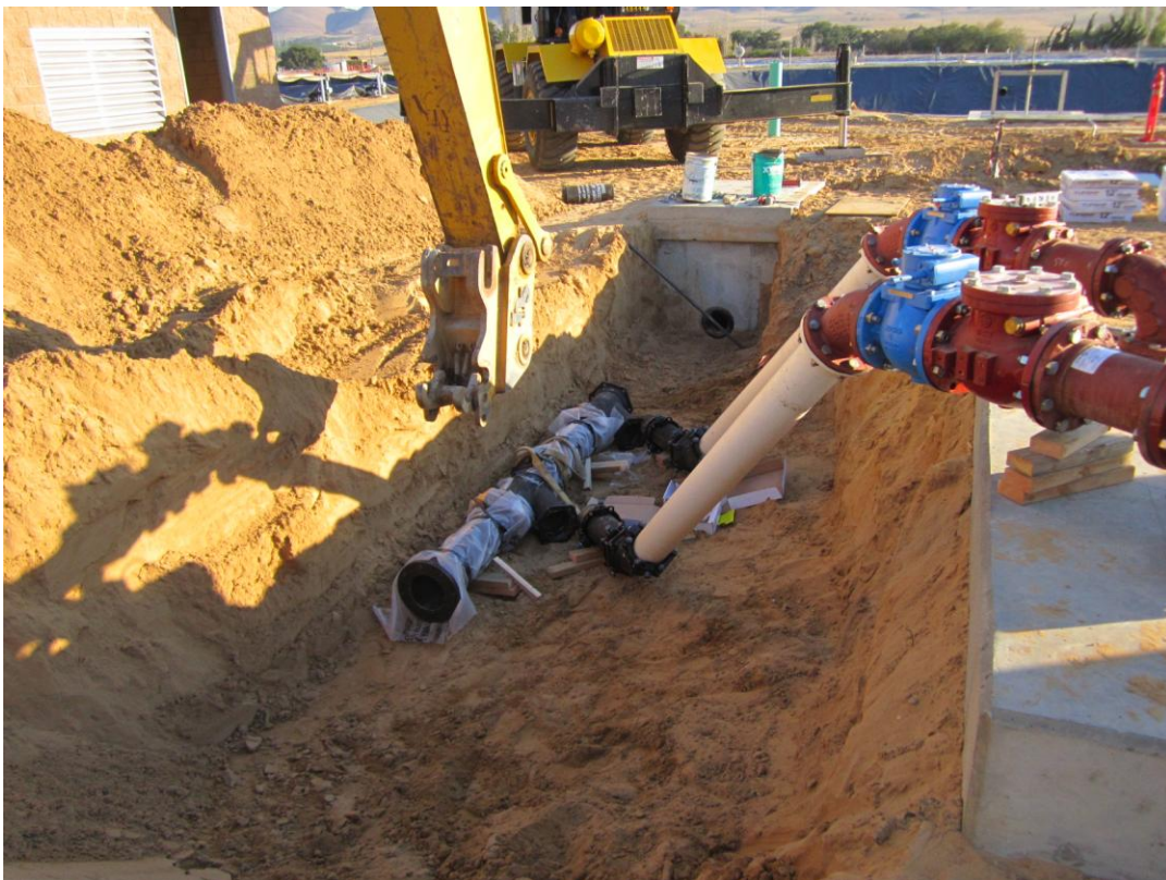
Piping and valves being installed at RAS/WAS Pump Station #2.
