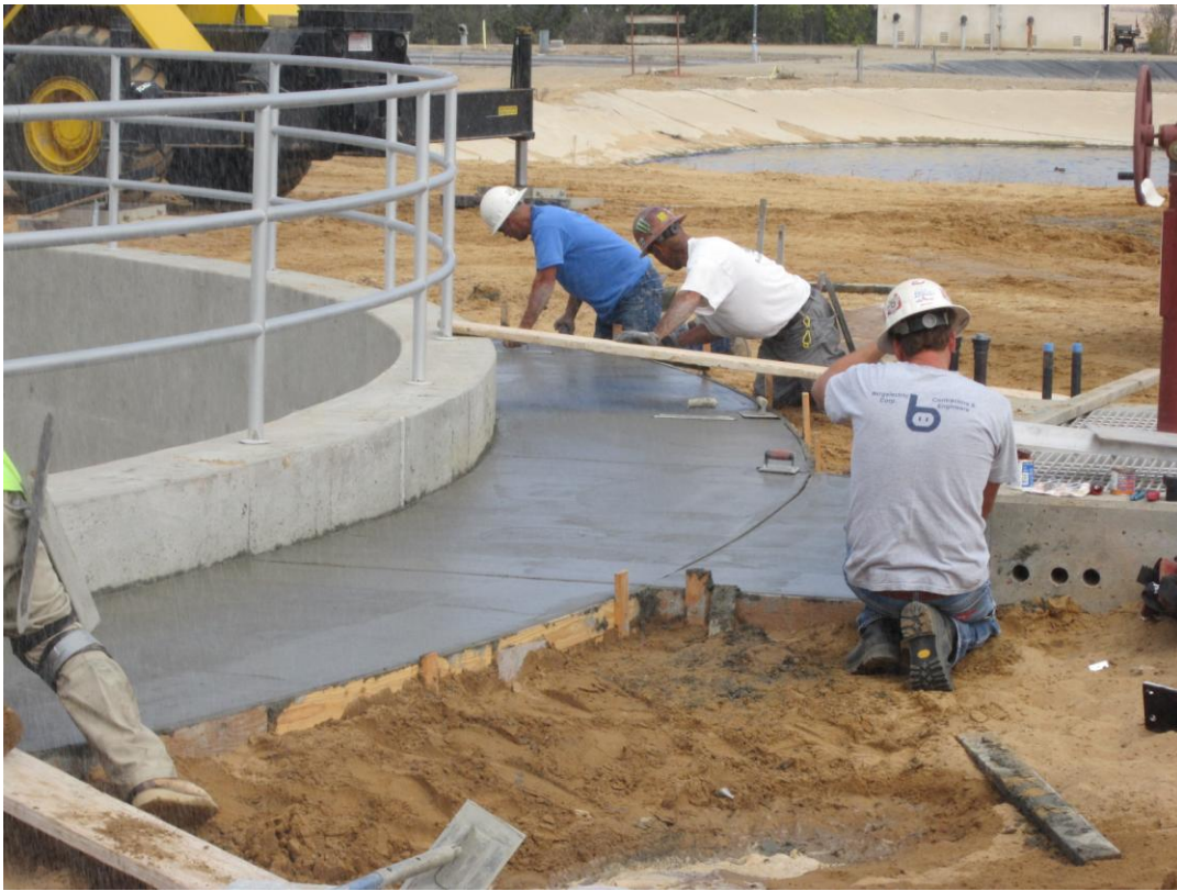
Cushman pouring sidewalk around Clarifier #1.
