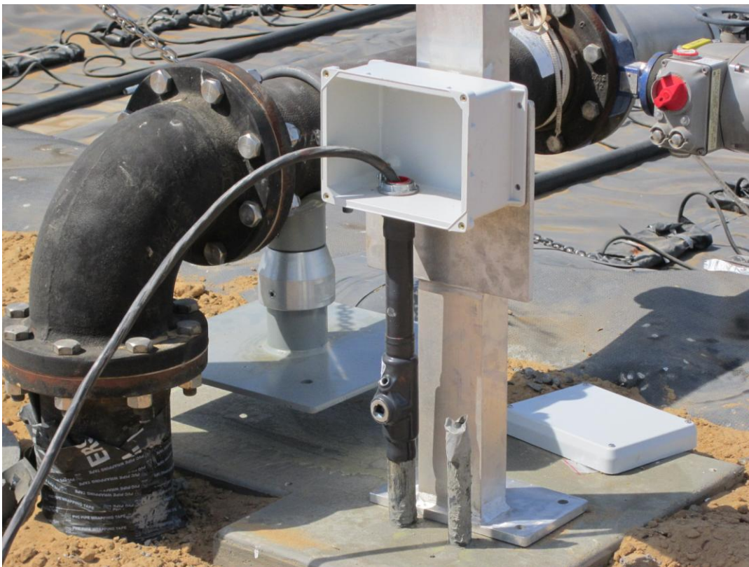
Bergelectric installing junction box and aluminum stand at AR piping.
