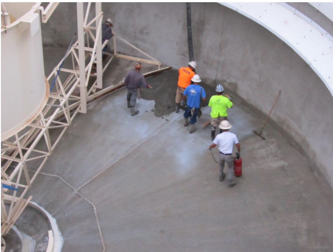
Cushman beginning grouting of Clarifier #1.
