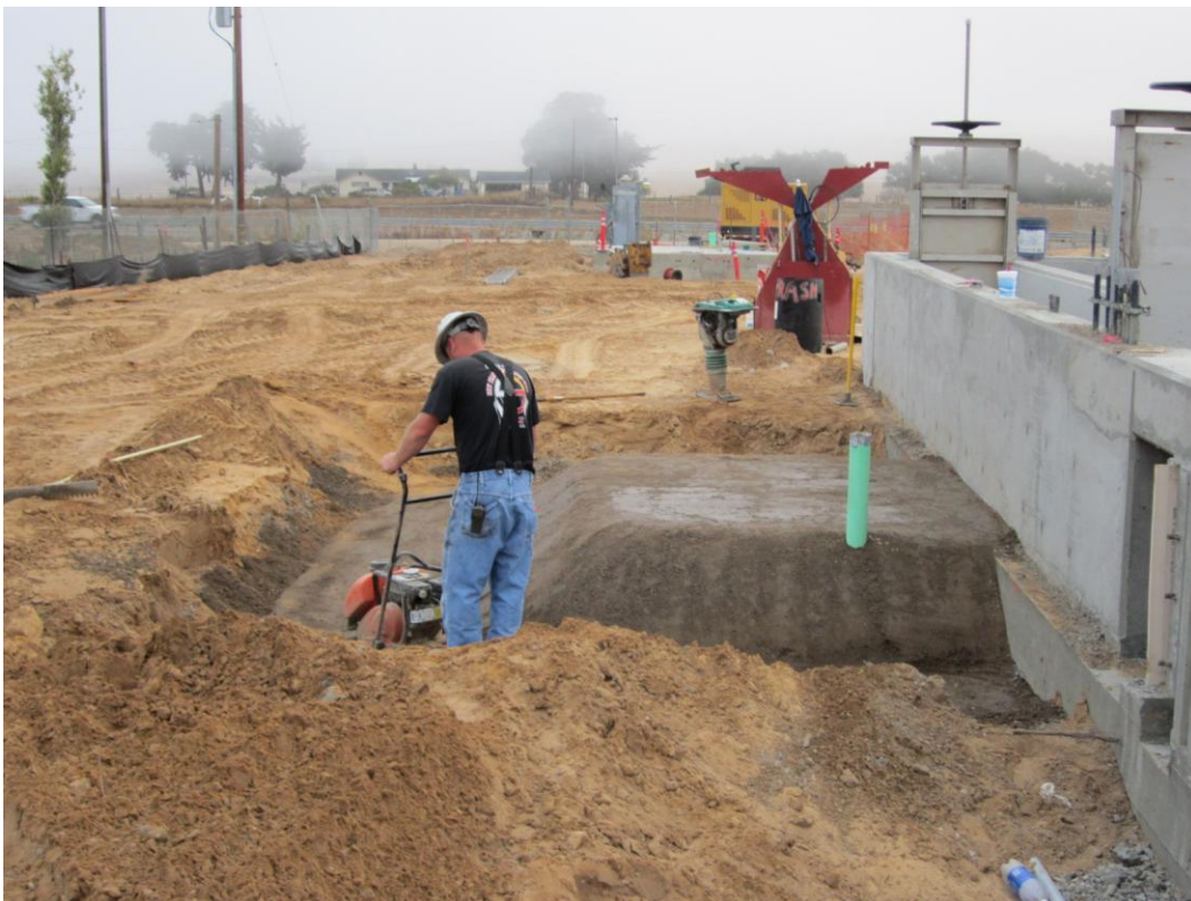
Cushman compacting base under future foundation for the trash enclosure slab.
