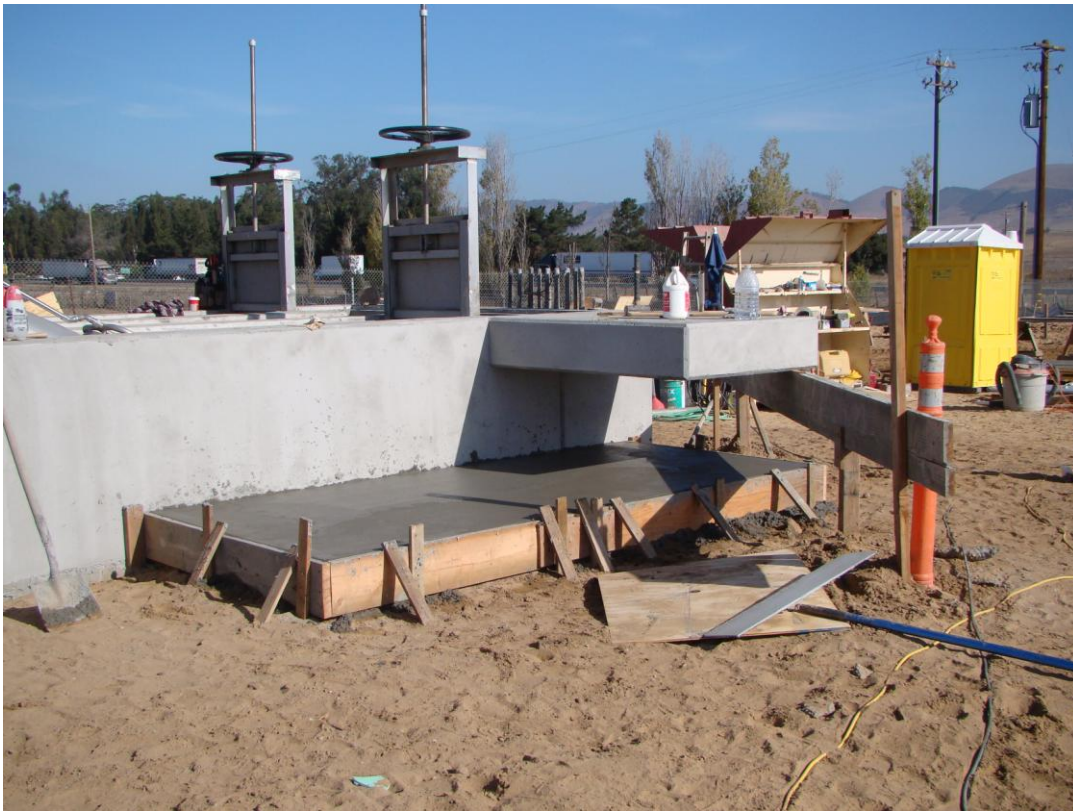
Slab poured for stair landing at the Headworks.
