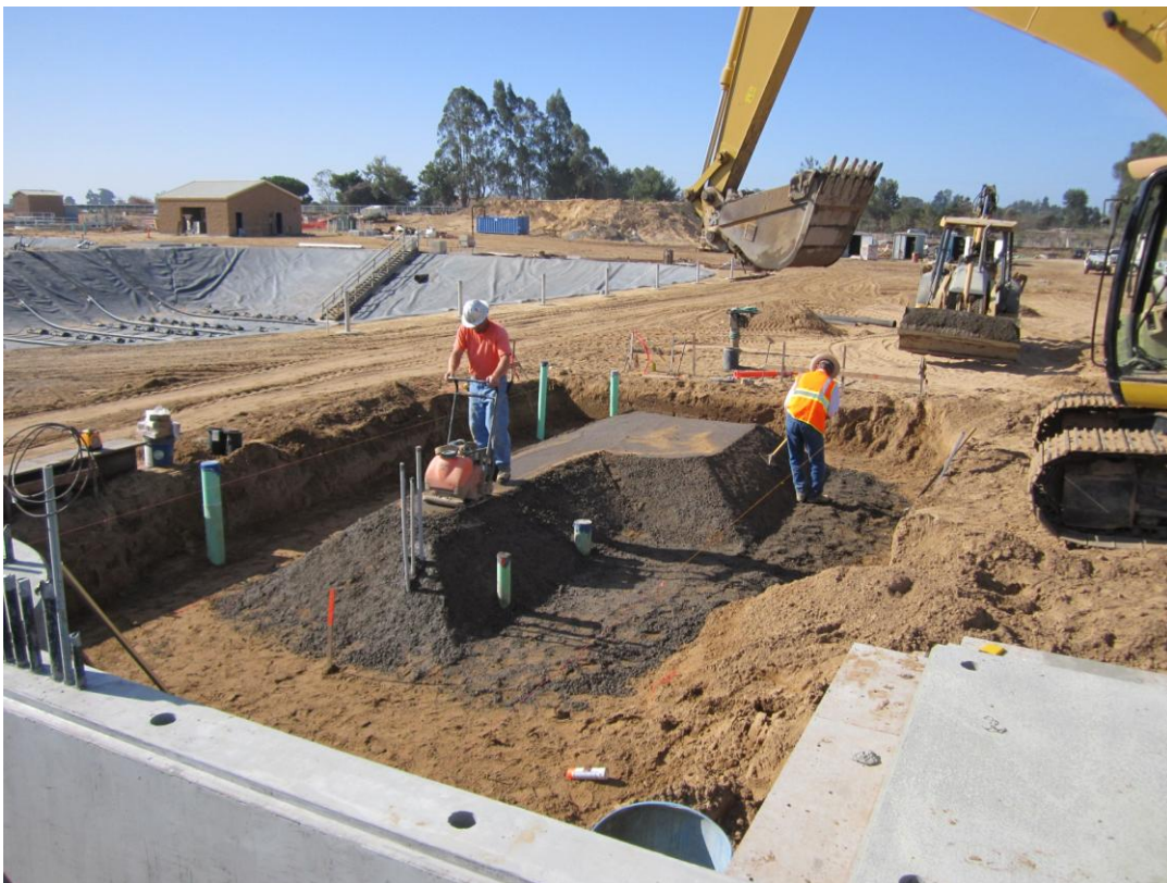
Cushman compacting base underneath foundation for Grit Classifier slab.
