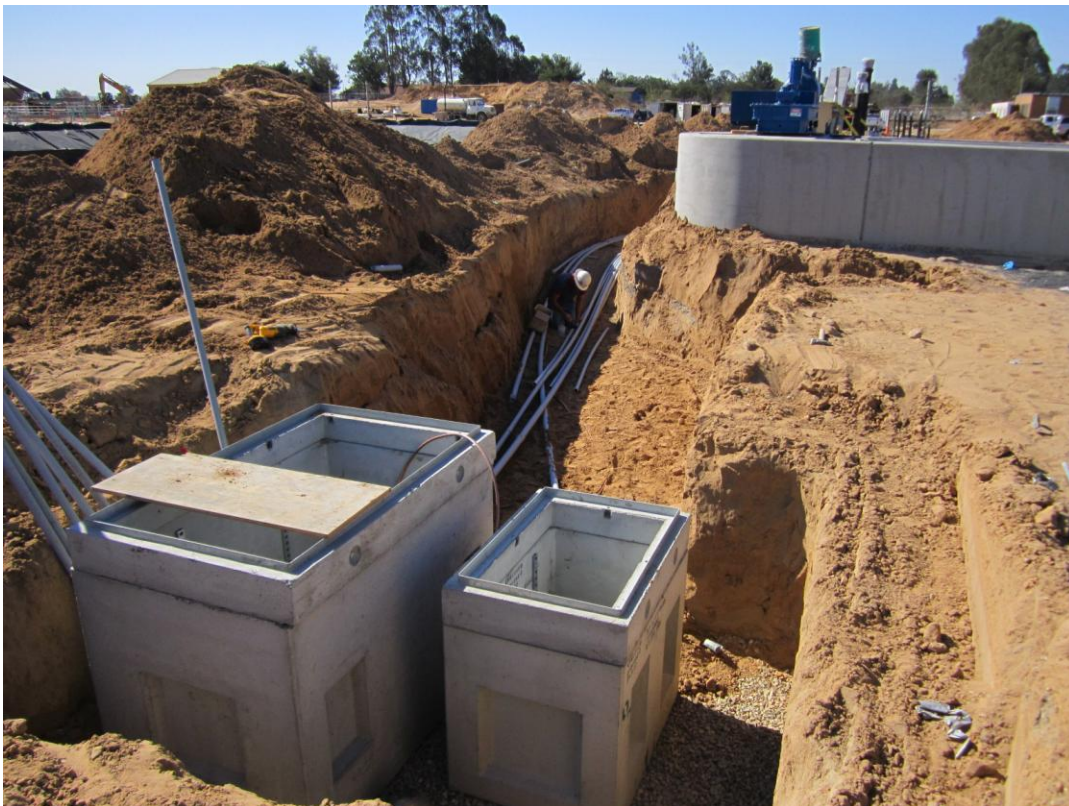
Installing more conduit for DB 02.
