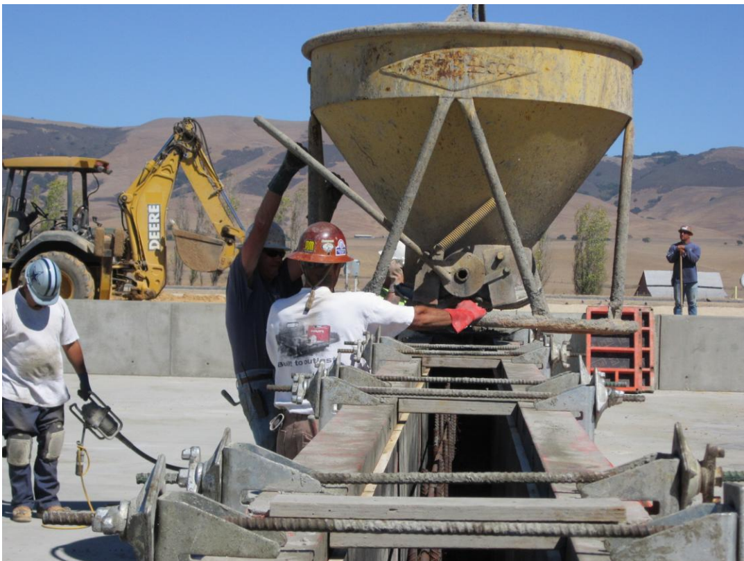
Cushman pouring wall sections at Sludge Drying Beds.
