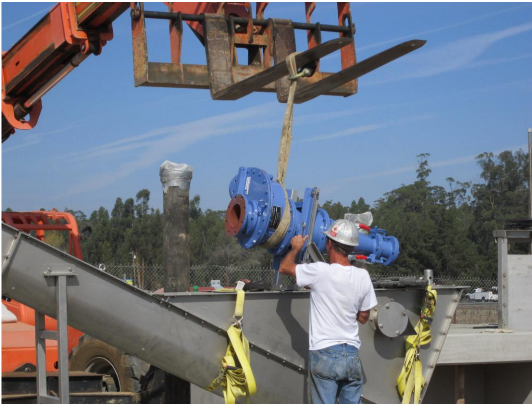
Installing Grit Classifier motor.
