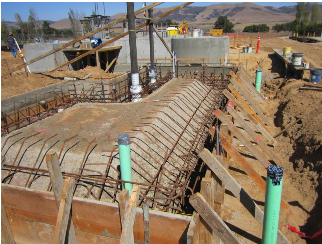
Installing forms and reinforcing for the Grit Classifier slab.
