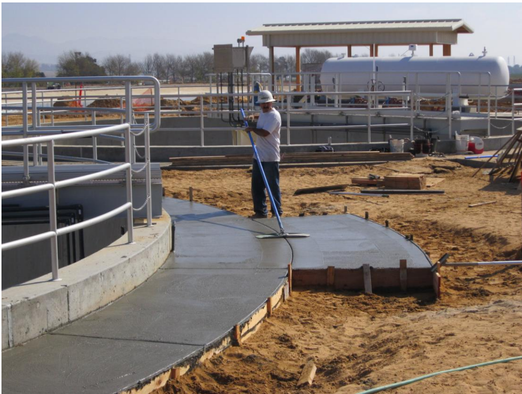
Cushman finishing concrete sidewalk around Clarifier #2.
