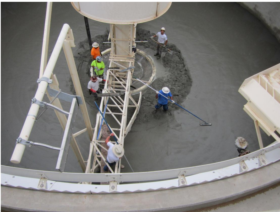
Cushman finishing grout in Clarifier #1.
