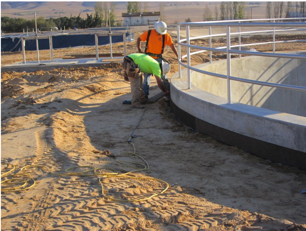
Cushman installing expansion material around Clarifier # 1.
