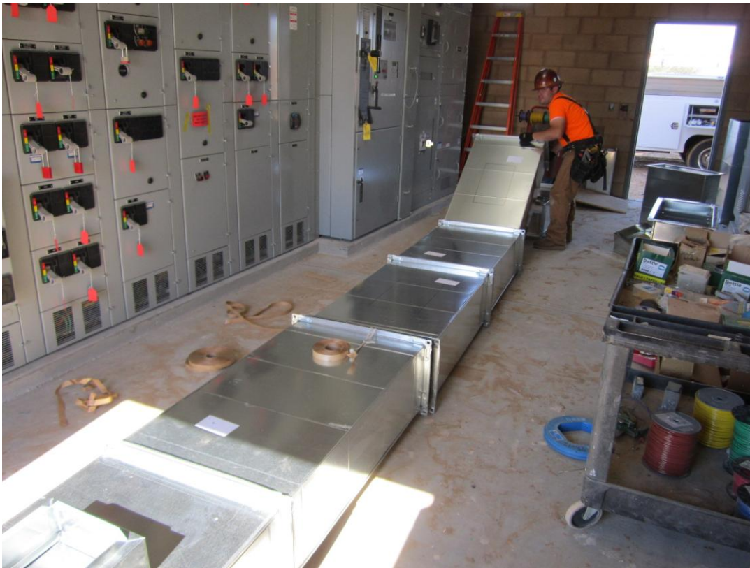
Longs Construction assembling the AC duct inside the MCC room.
