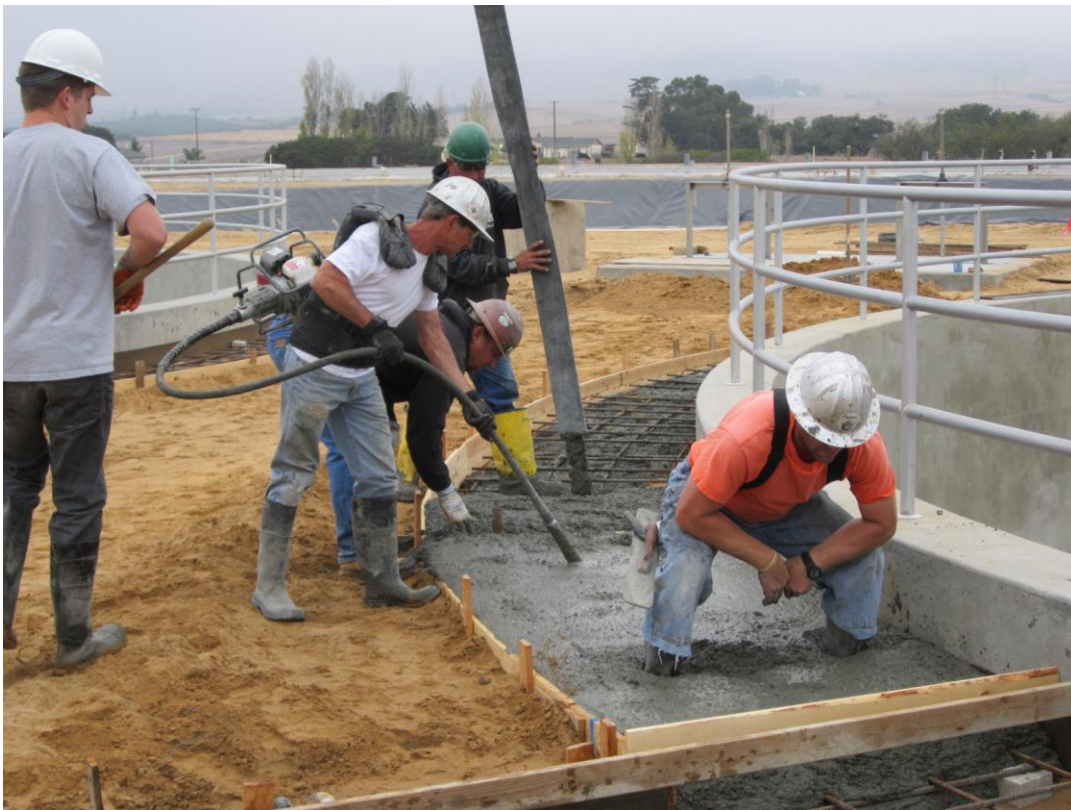
Cushman placing concrete for sidewalk around Clarifier #1.
