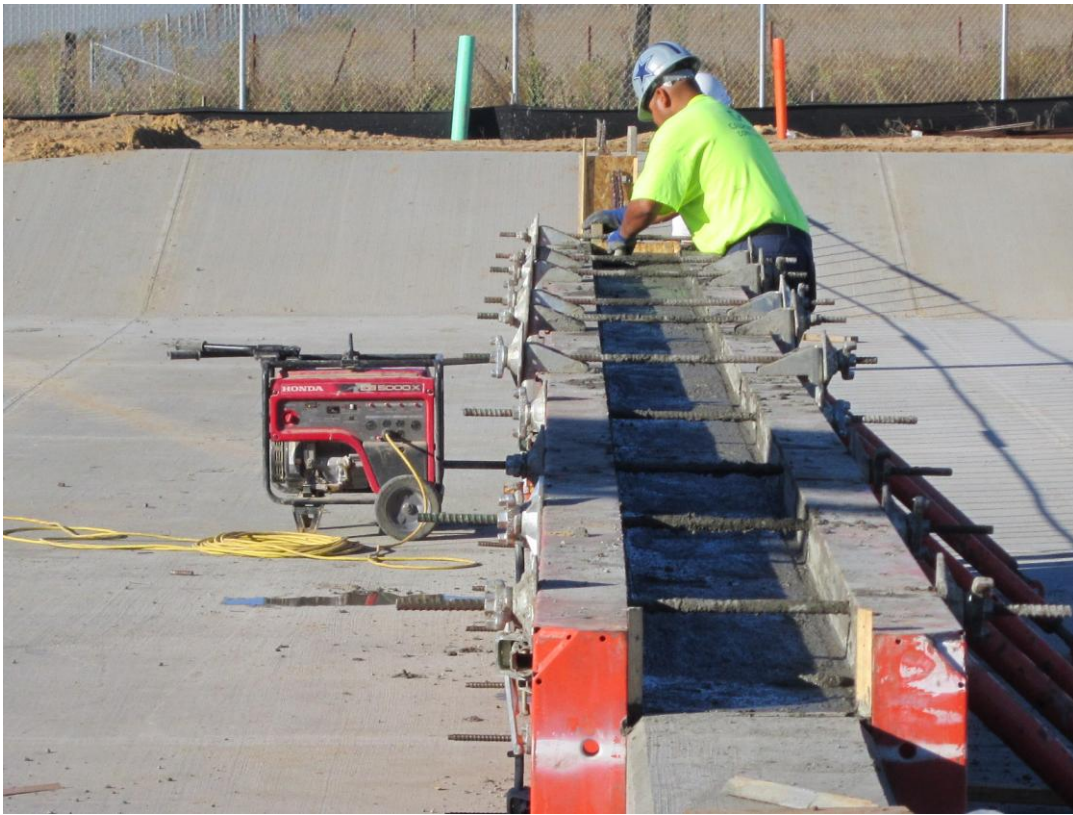
Cushman finishing the top of one of the drying bed walls.
