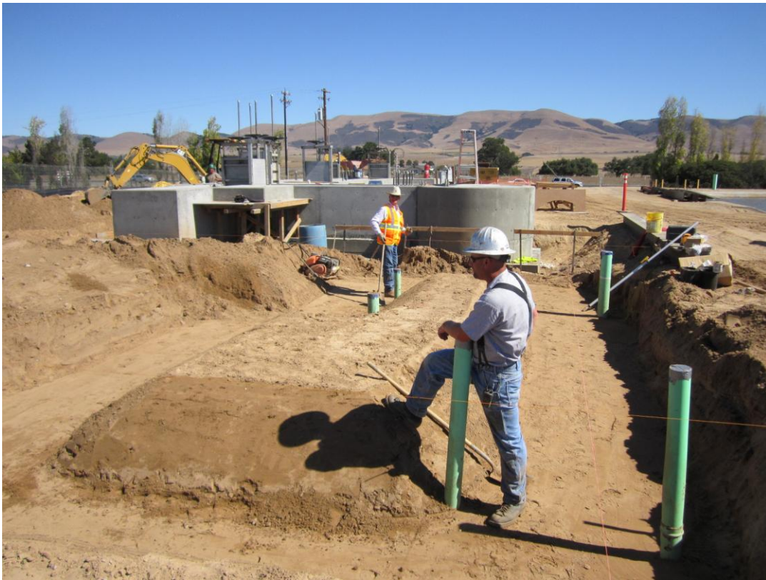
Cushman excavating for Grit Classifier slab foundation.
