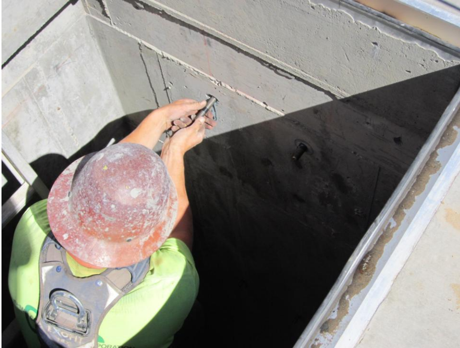
Cushman installing epoxy bolts for access ladder inside the Influent Pump Station.
