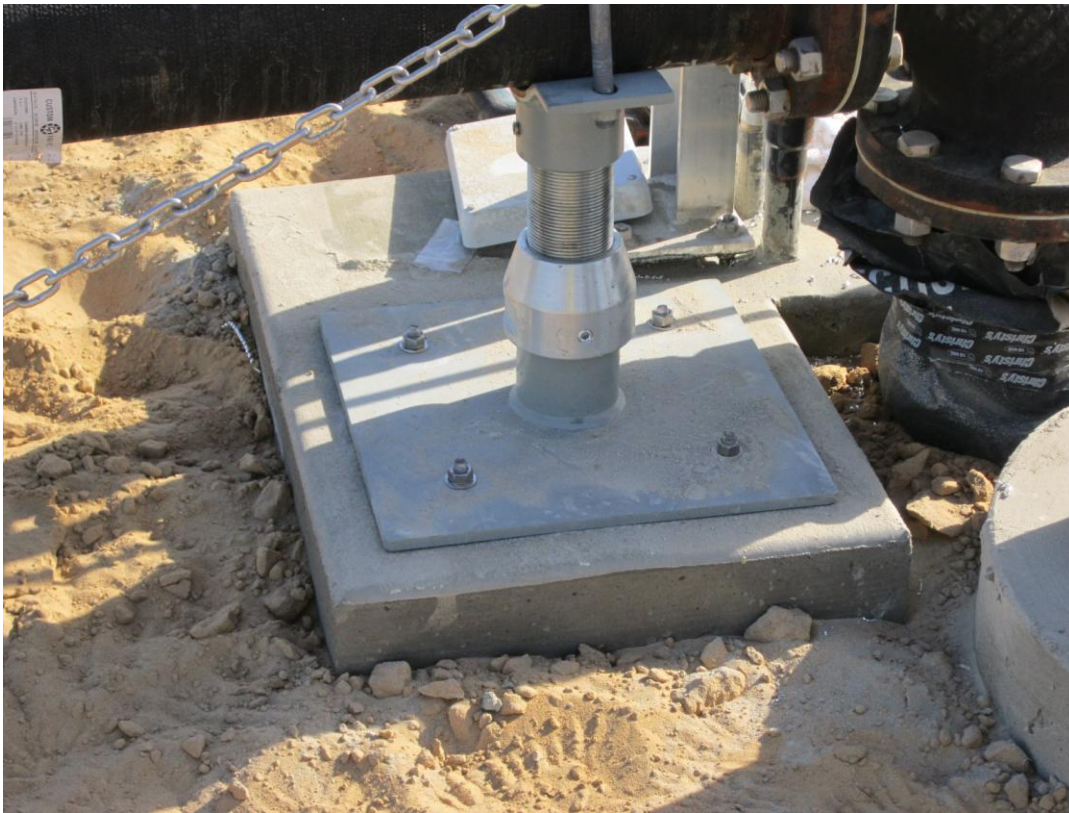
Installing AR pipe supports.
