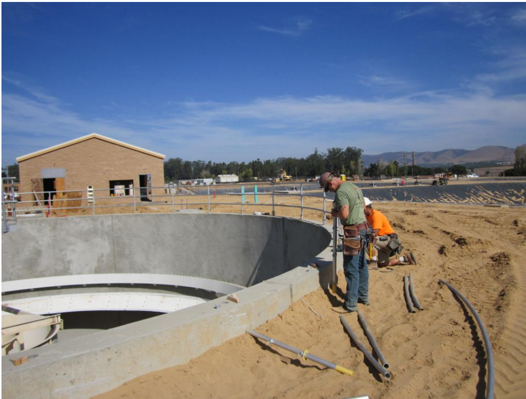
Cushman installing hand rails around top of clarifiers.
