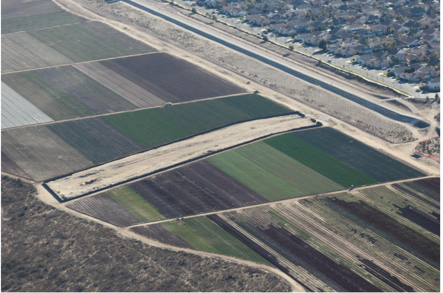
Aerial photo of the south side with all ARB equipment demobilized and the site rough graded.
