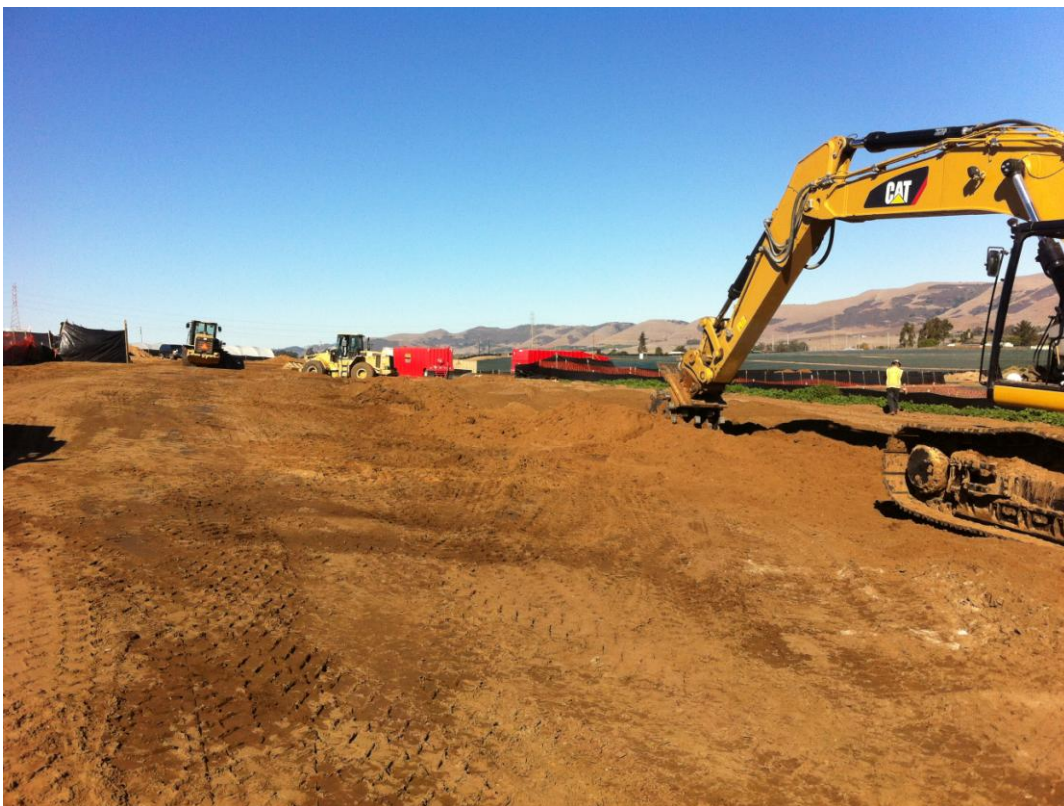
Final compaction over sink holes.
