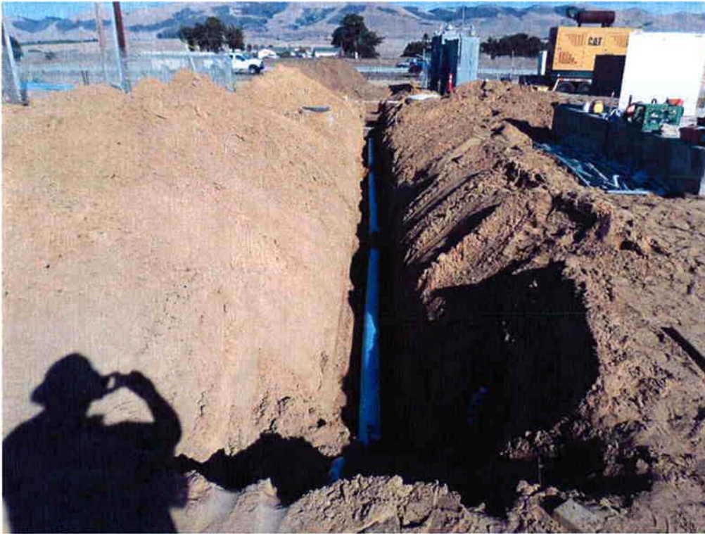
Cushman installing 6-inch potable waterline near Influent Pump Station.
