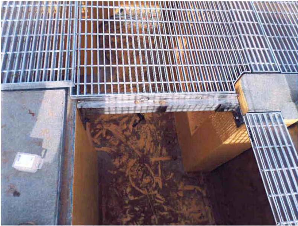
Cushman installing grating support beams.
