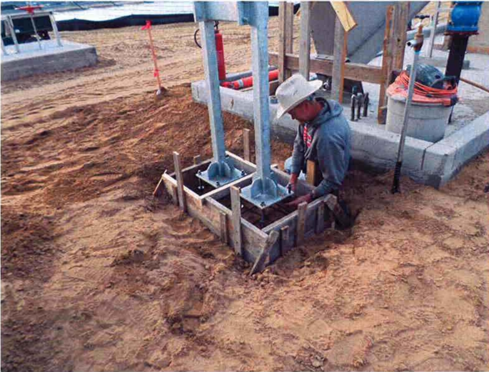
Cushman preparing forms for pipe support pad for the grit piping.
