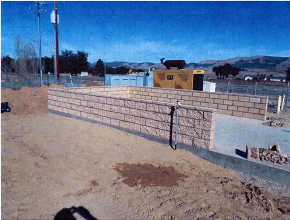
Truck wash down station wall completed.
