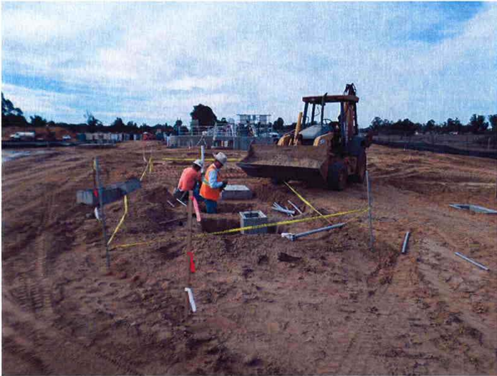
Cushman and Bergelectric setting boxes for PB01.
