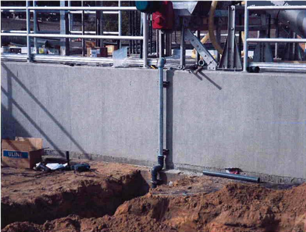
Cushman installing the non-potable water to the Headworks.
