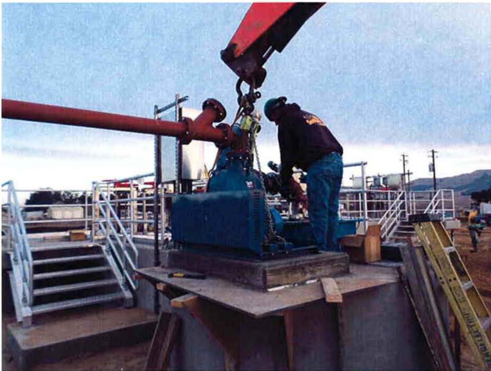
Cushman mounting the Grit Pump on the new concrete pad.
