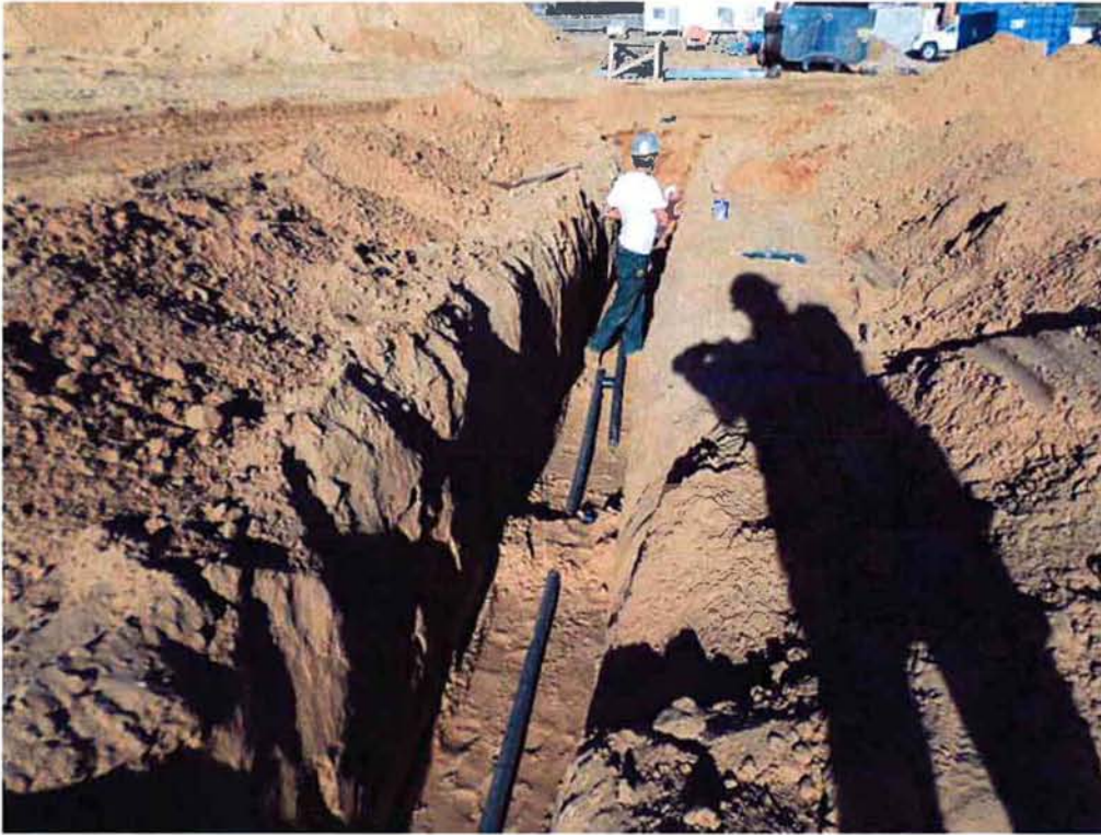
Cushman installing 2-inch non-potable water line.
