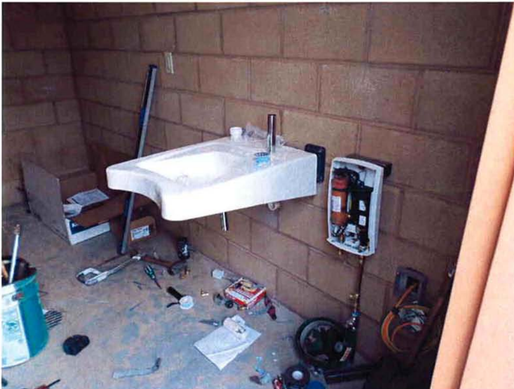
Cushman installing the sink and water heater in the bathroom at the Sodium Hypochlorite Storage Building.
