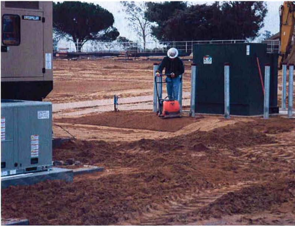
Cushman grading around the Electrical/Blower Building.
