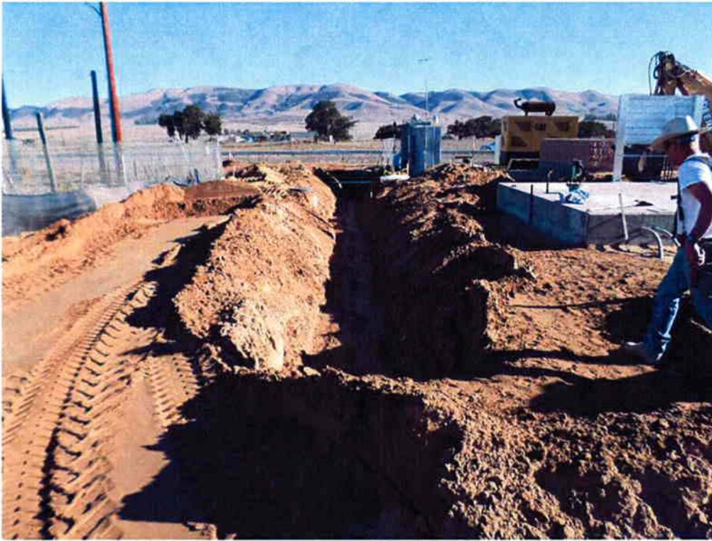
Cushman backfilling and compacting at the 6-inch potable water line.
