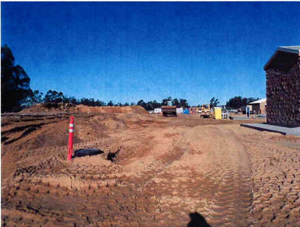
Cushman performing site grading work to the west of the Electrical/Blower Building and Sodium Hypochlorite Storage Building.
