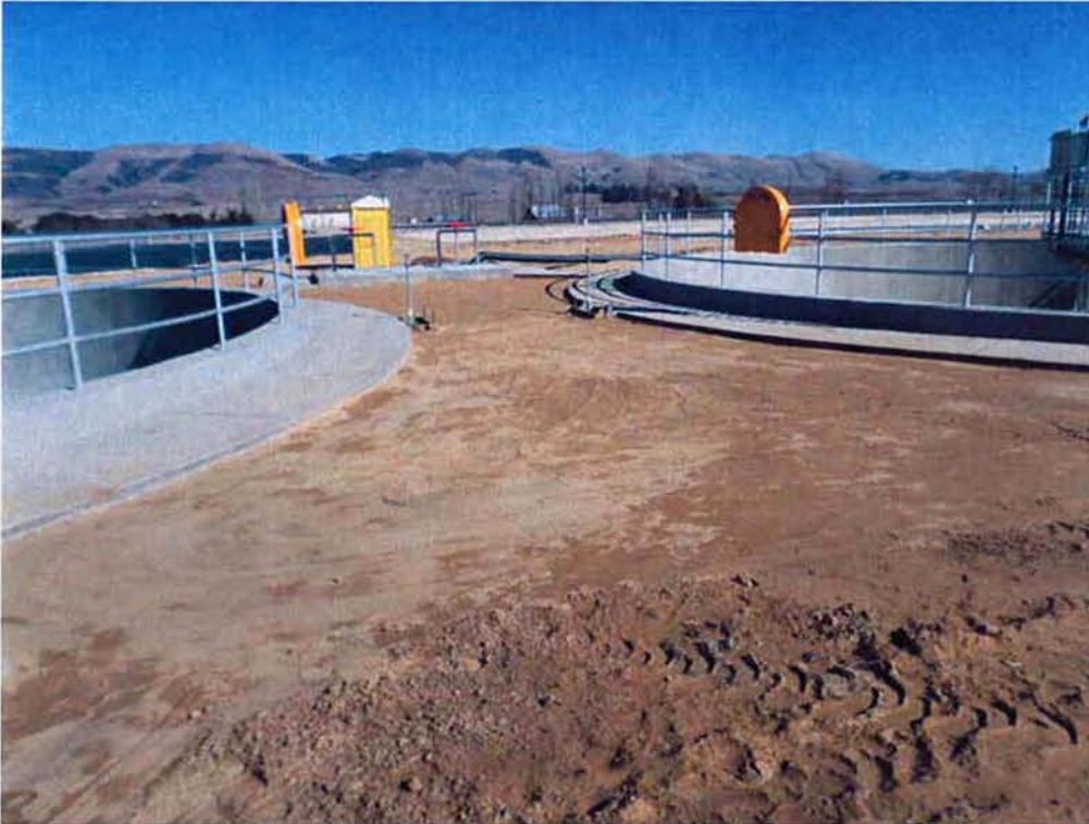
Grading between the clarifiers.
