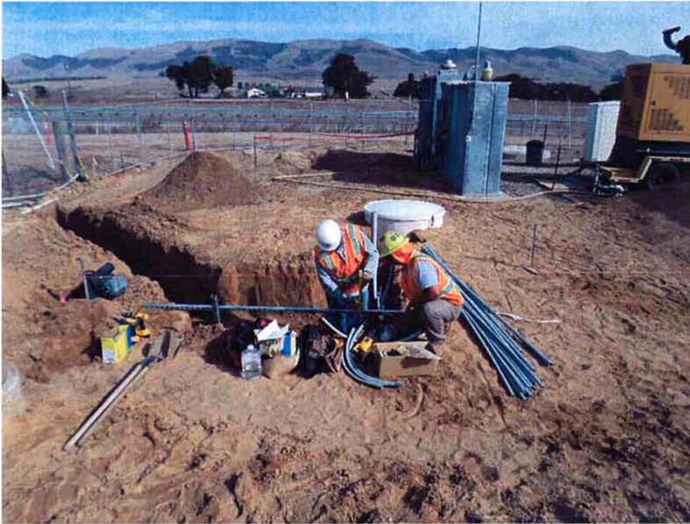
Bergelectric installing conduit at the Influent Sampler.
