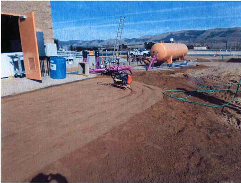
Cushman grading around the Sodium Hypochlorite Storage Building.
