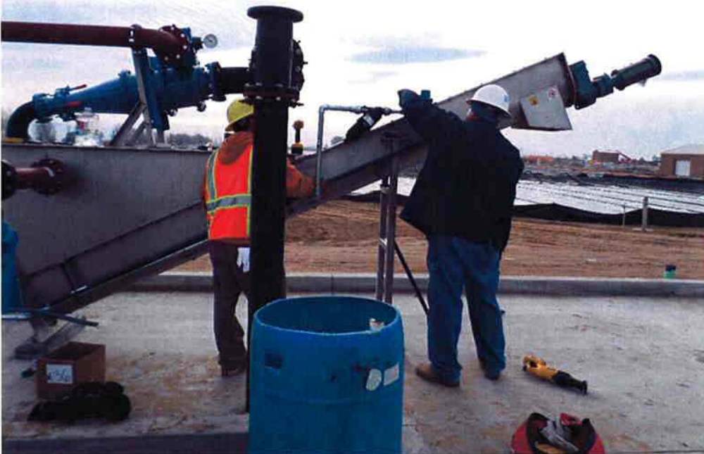
Bergelectric installing conduit to the solenoid valve at the Grit Classifier.
