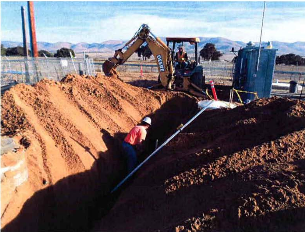
Cushman installing the 6-inch potable water line.
