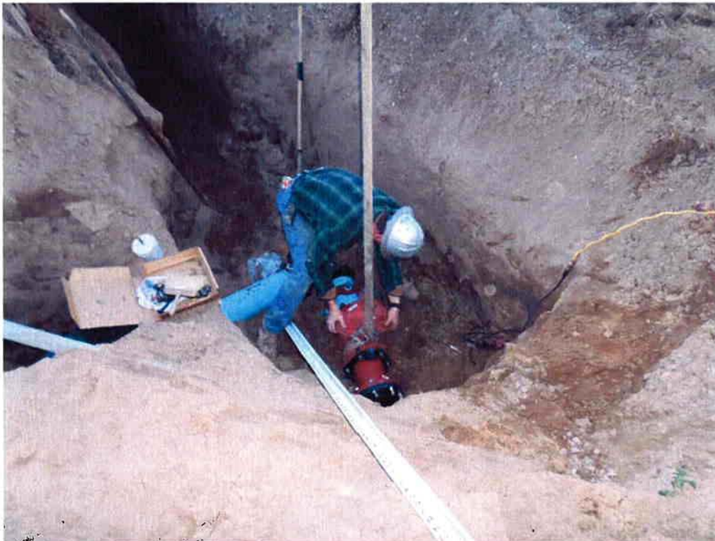
Cushman installing the 6-inch potable waterline with valves.
