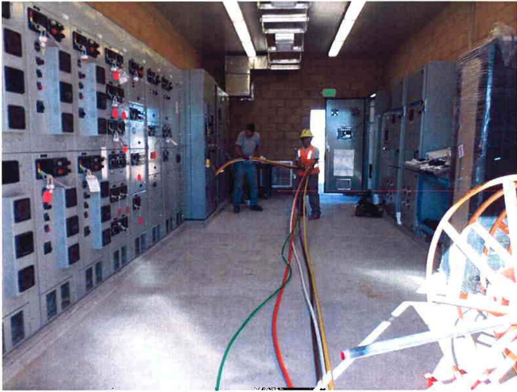
Bergelectric pulling generator feed cables in the MCC Room.
