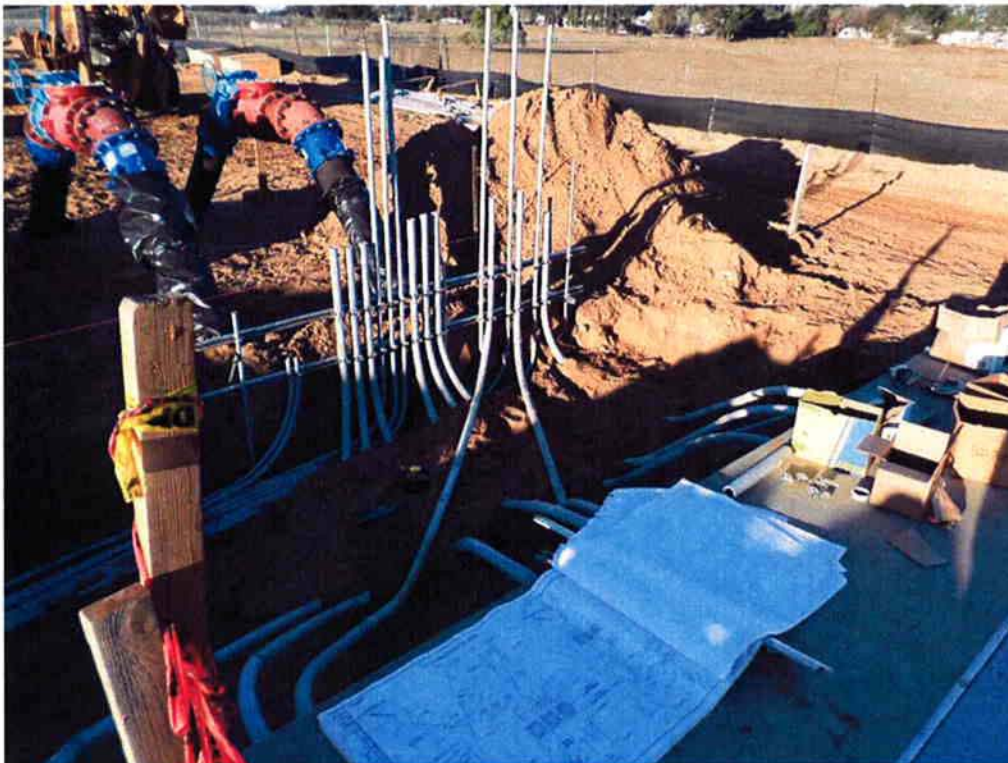
Bergelectric installing under slab conduits to the control panel for the Influent Pump Station.
