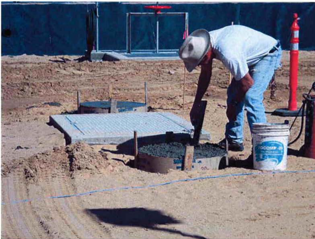
Cushman pouring collars at valve cans.
