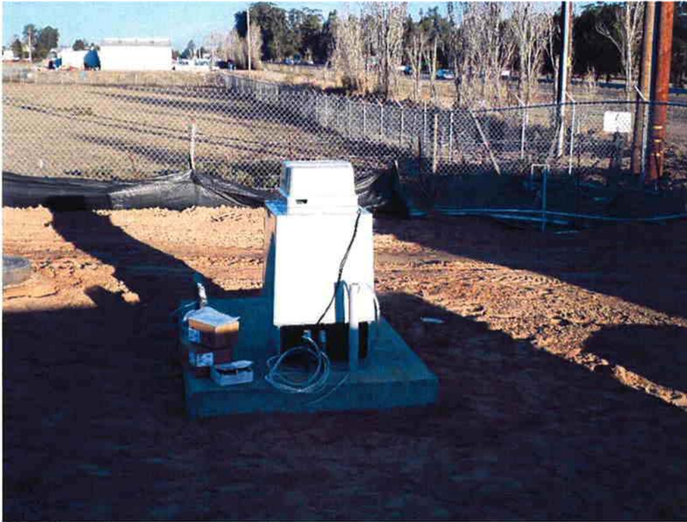
Installing influent pump sampler.
