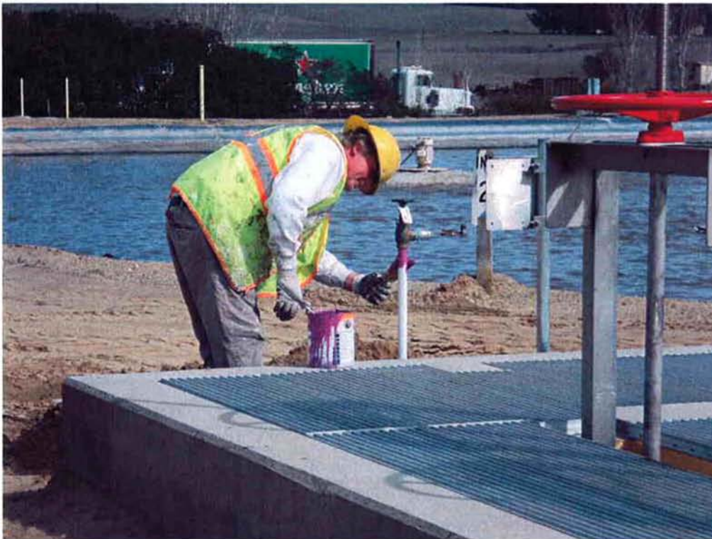
KNK Coatings painting non potable water piping.
