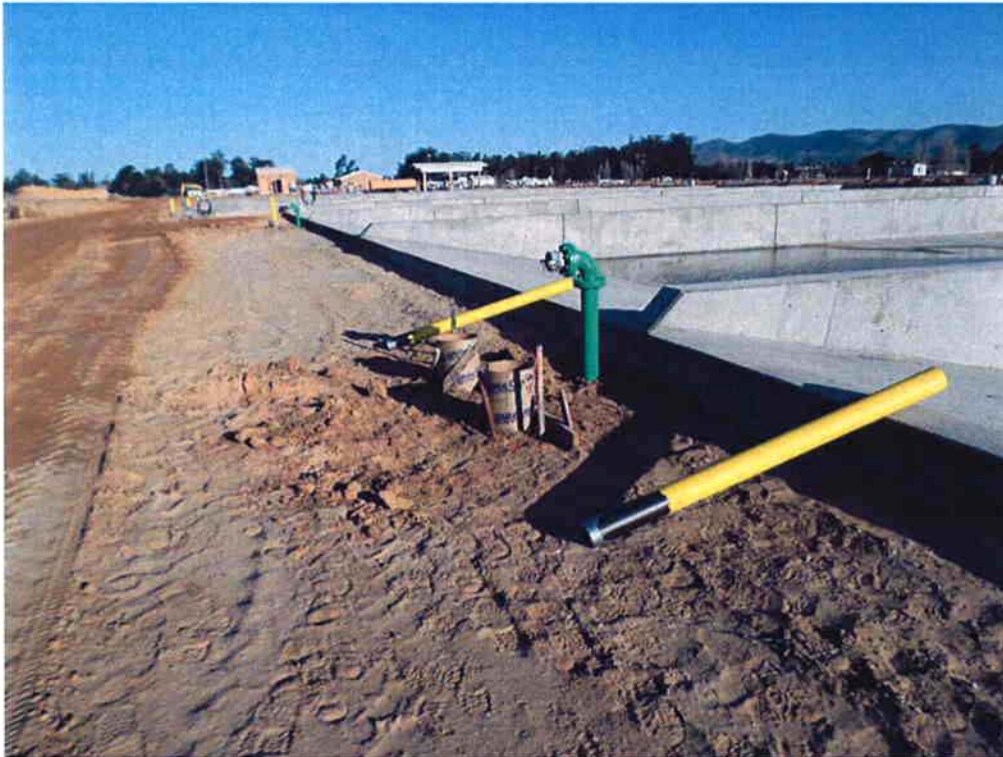
Cushman installing bollards at the drain pipes.
