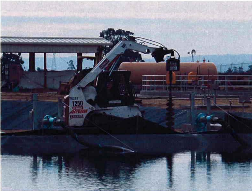
Cushman boring holes for street light bases between Aeration Basin #1 and the Emergency Basin.
