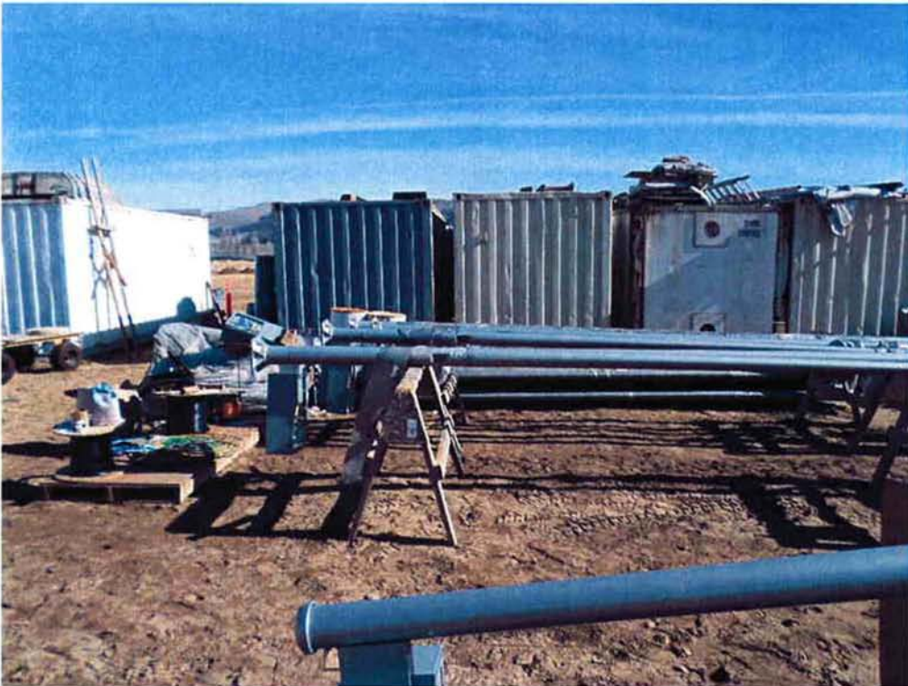
Cushman assembling street light poles.
