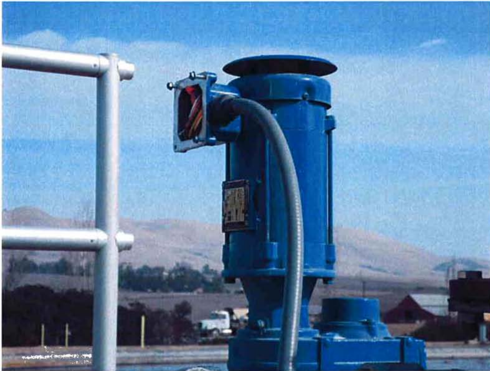
Bergelectric terminating wires to grit motor.
