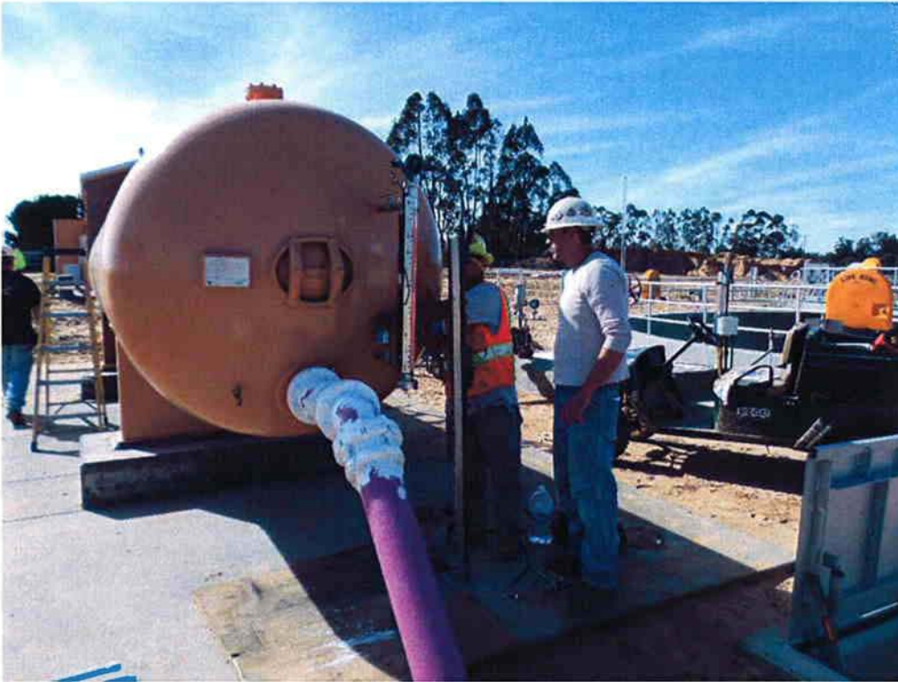
Bergelectric terminating the level indicator on the pneumatic tank.
