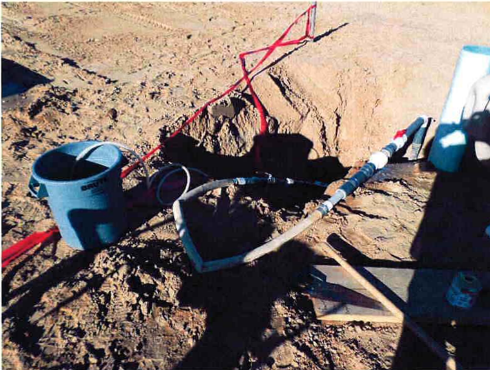
Cushman disinfecting the 2-inch potable water line.
