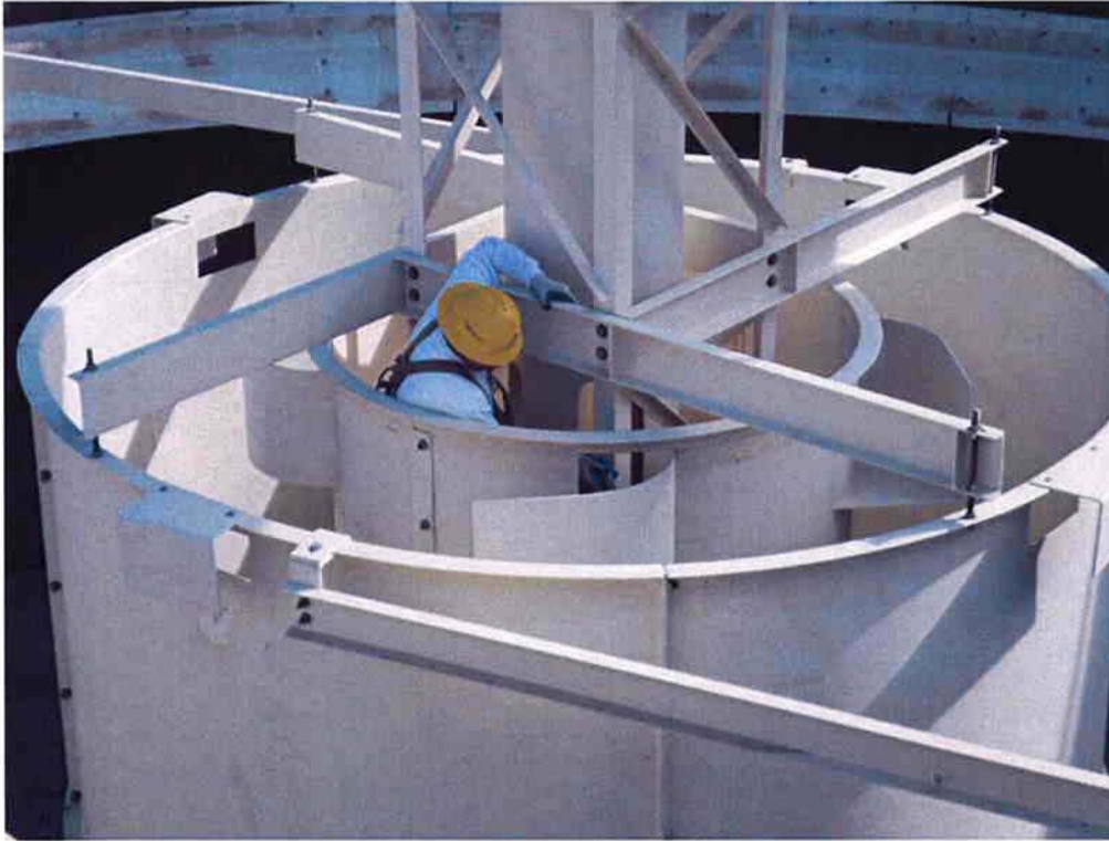
KNK Coating recoating where corrosion was removed on Clarifier #2 mechanism.
