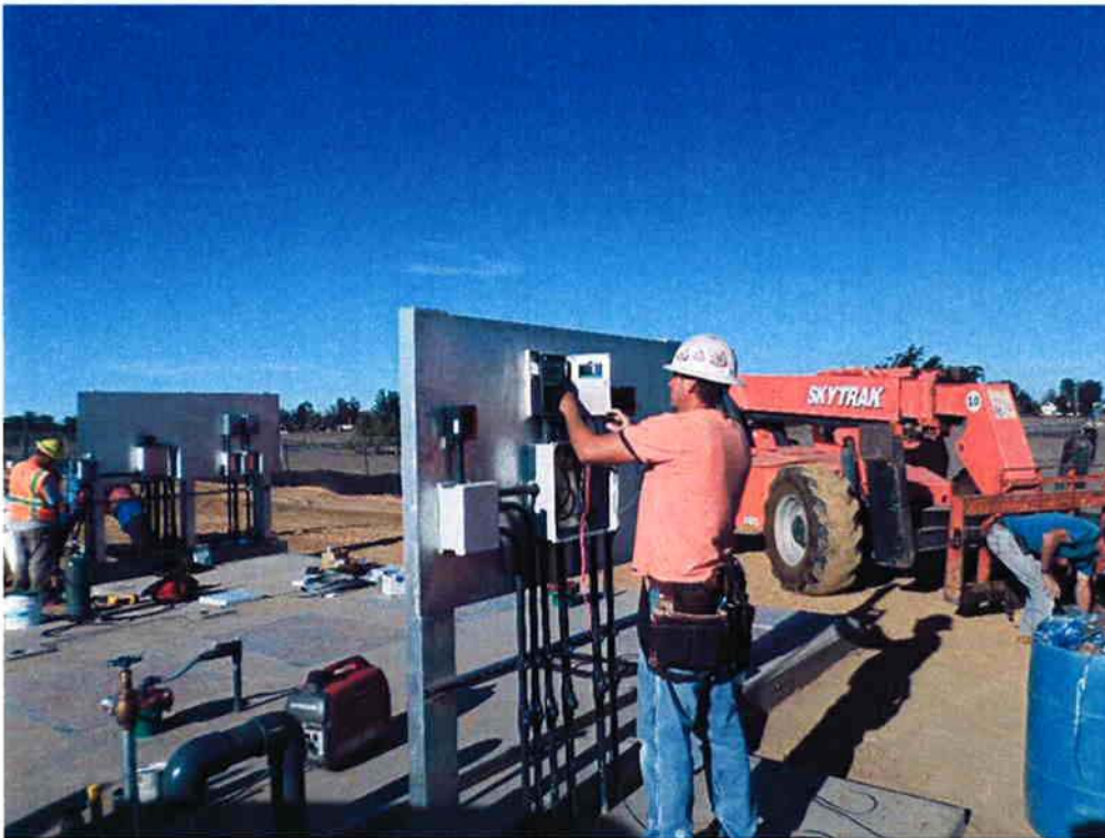
Bergelectric terminating level sensor at the Influent Pump Station.
