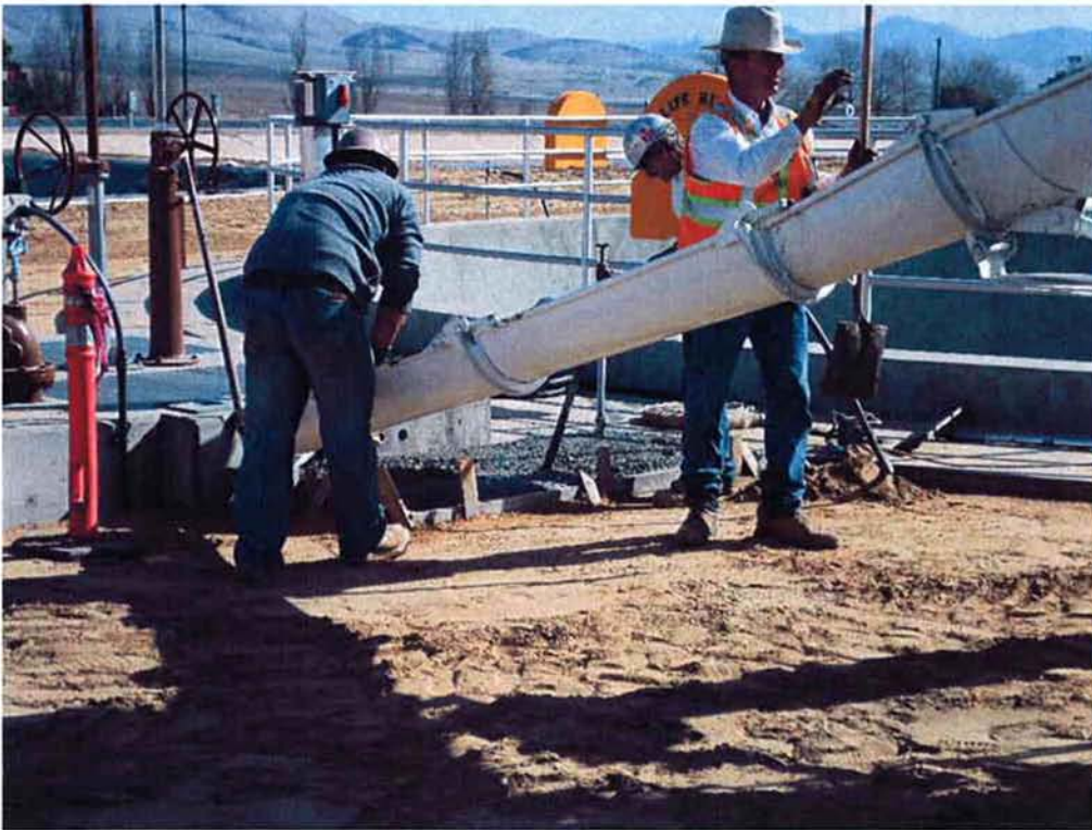
Cushman pouring concrete for hose bib pads.
