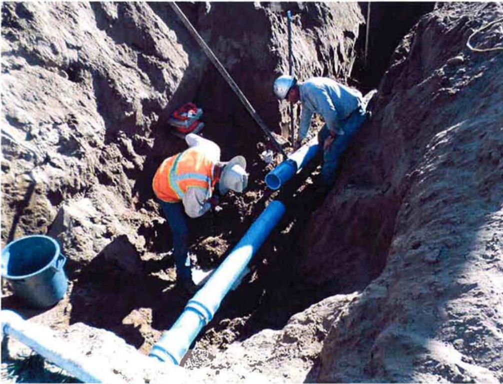
Cushman tying in the 6-inch water line.
