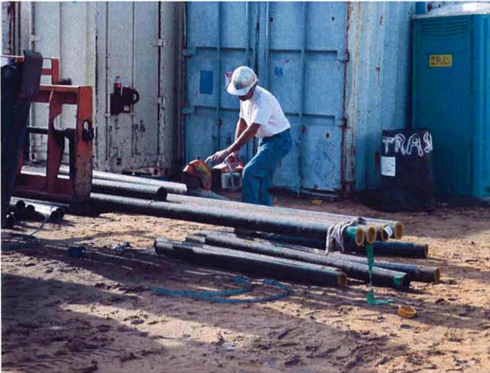
Cushman cutting pipe into bollards.
