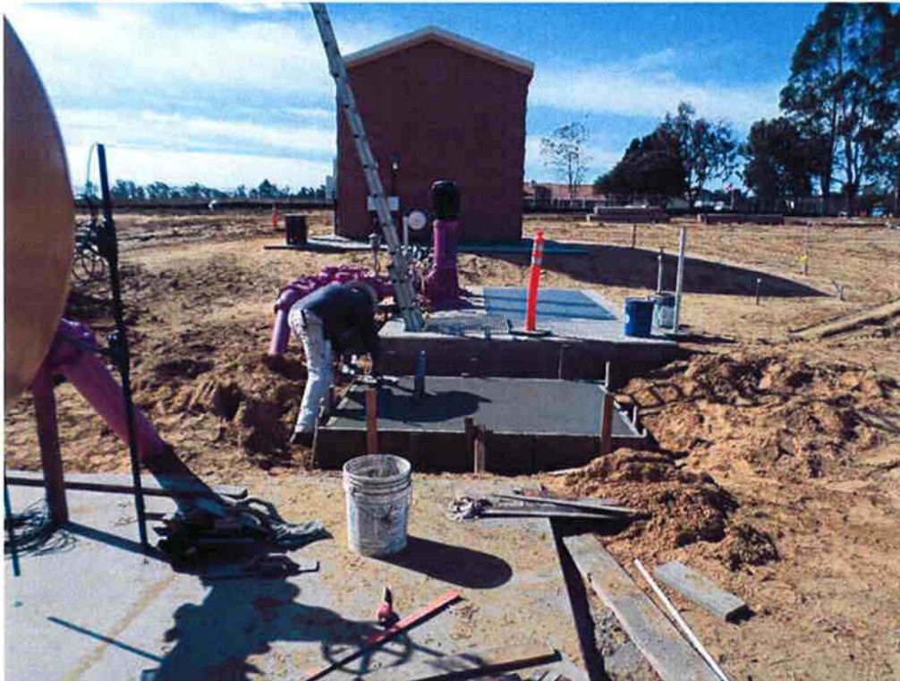
Cushman pouring concrete for the sampler pad and hose bib.
