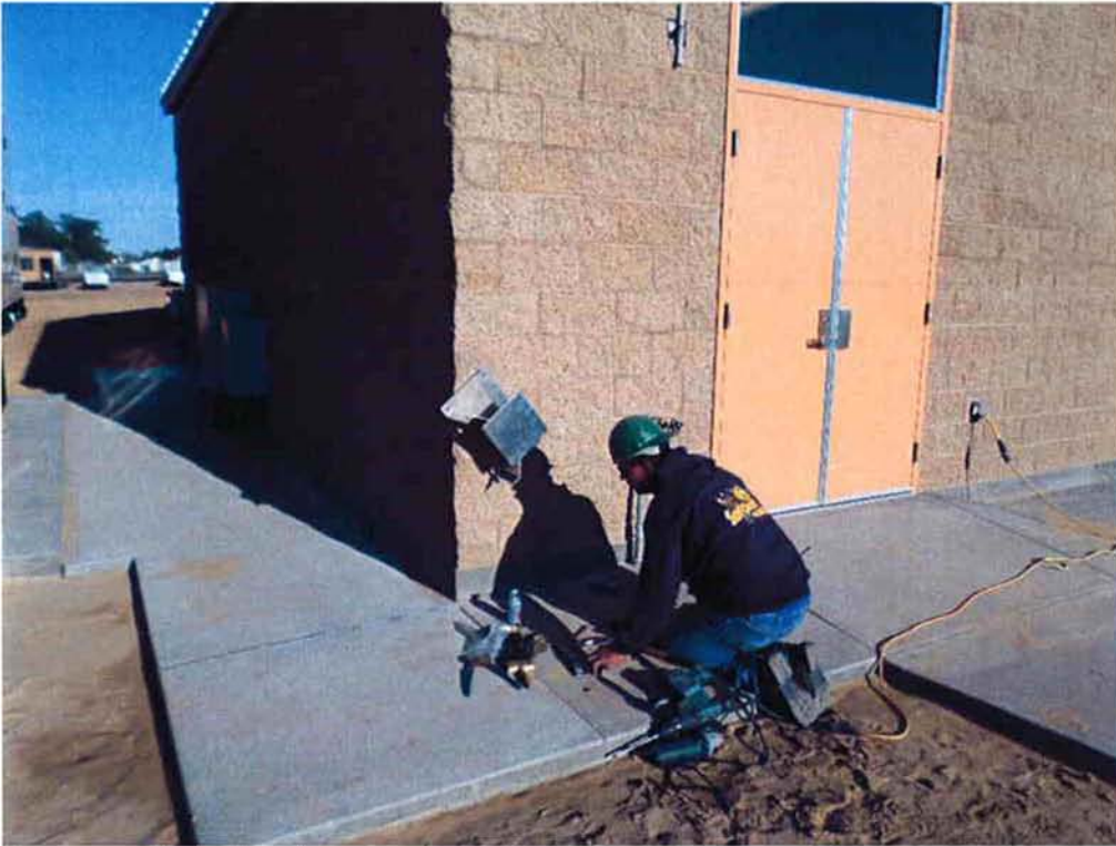
Cushman installing hose racks.
