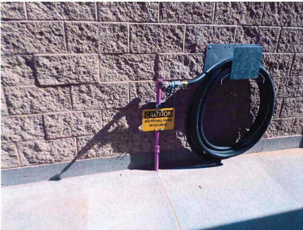
Non-potable water signs installed.
