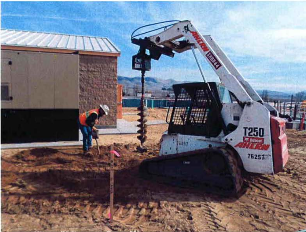
Cushman boring holes for bollard installation.
