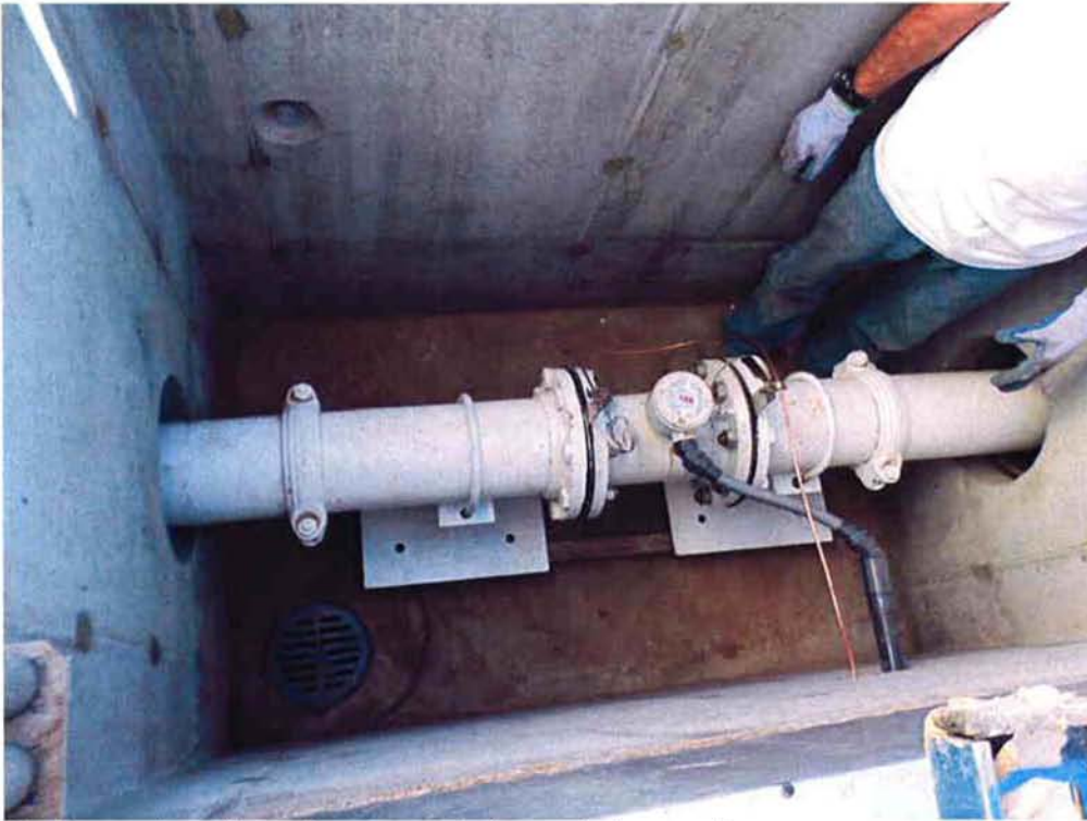
Cushman installing pipe supports in metering vault.
