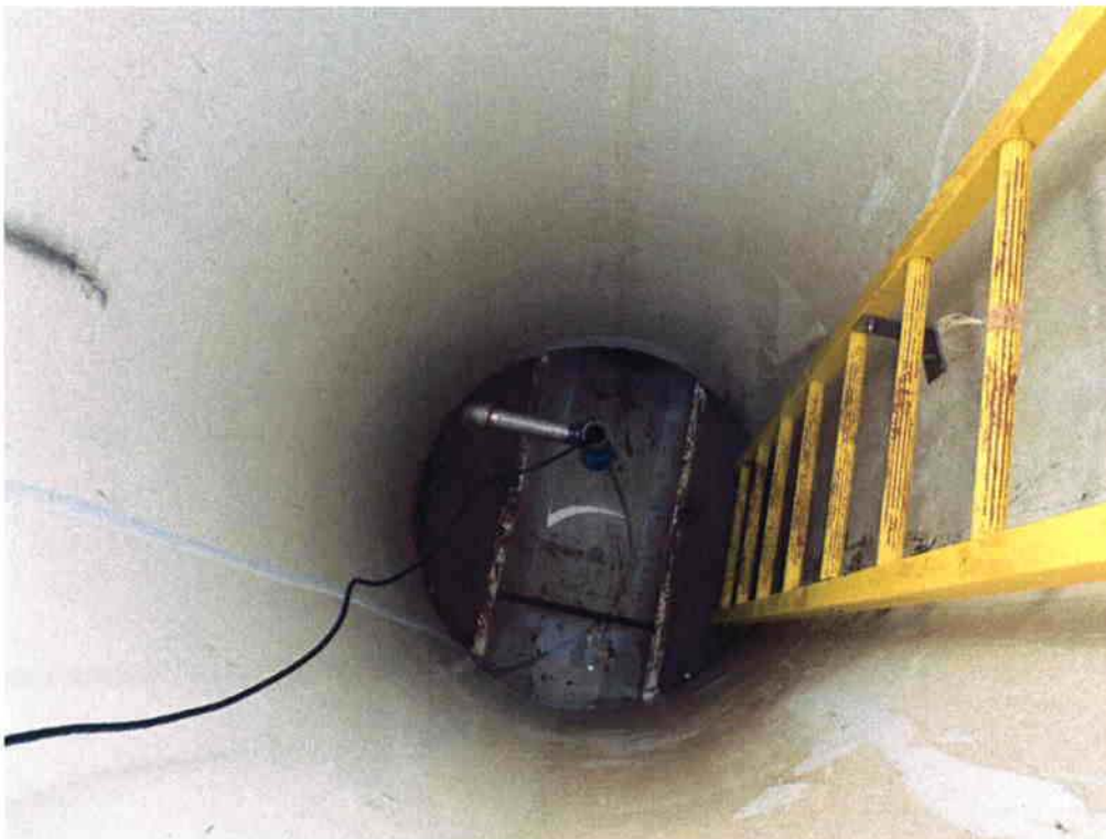
Installation of sensor in the flow metering manhole.
