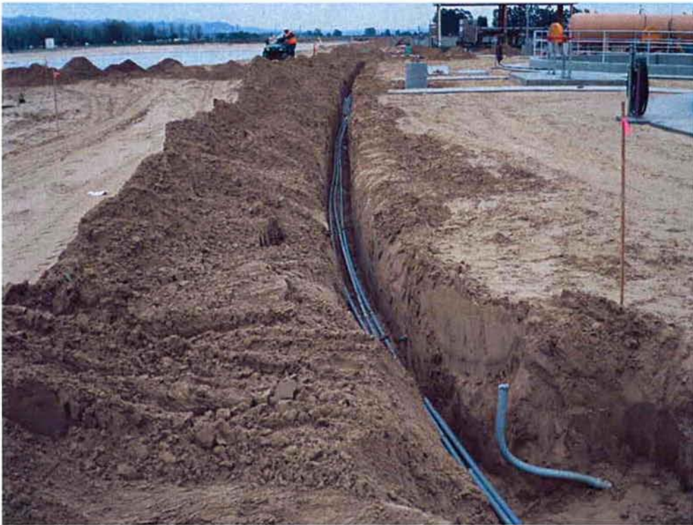
Bergelectric installing street light conduit.
