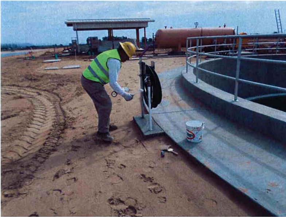
KNK Coating applying primer coat to non potable water piping.
