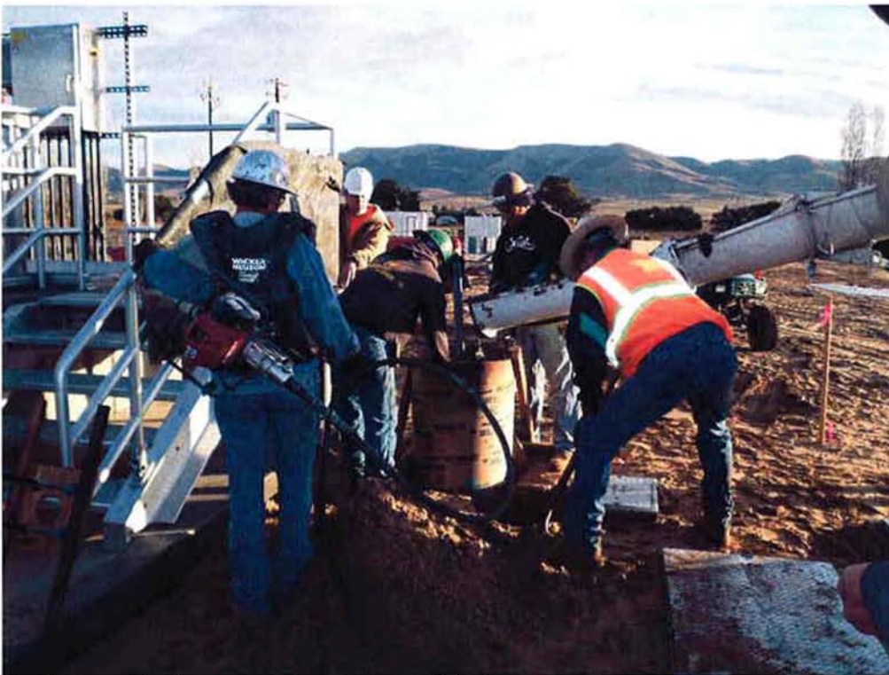
Cushman placing concrete at street light bases.
