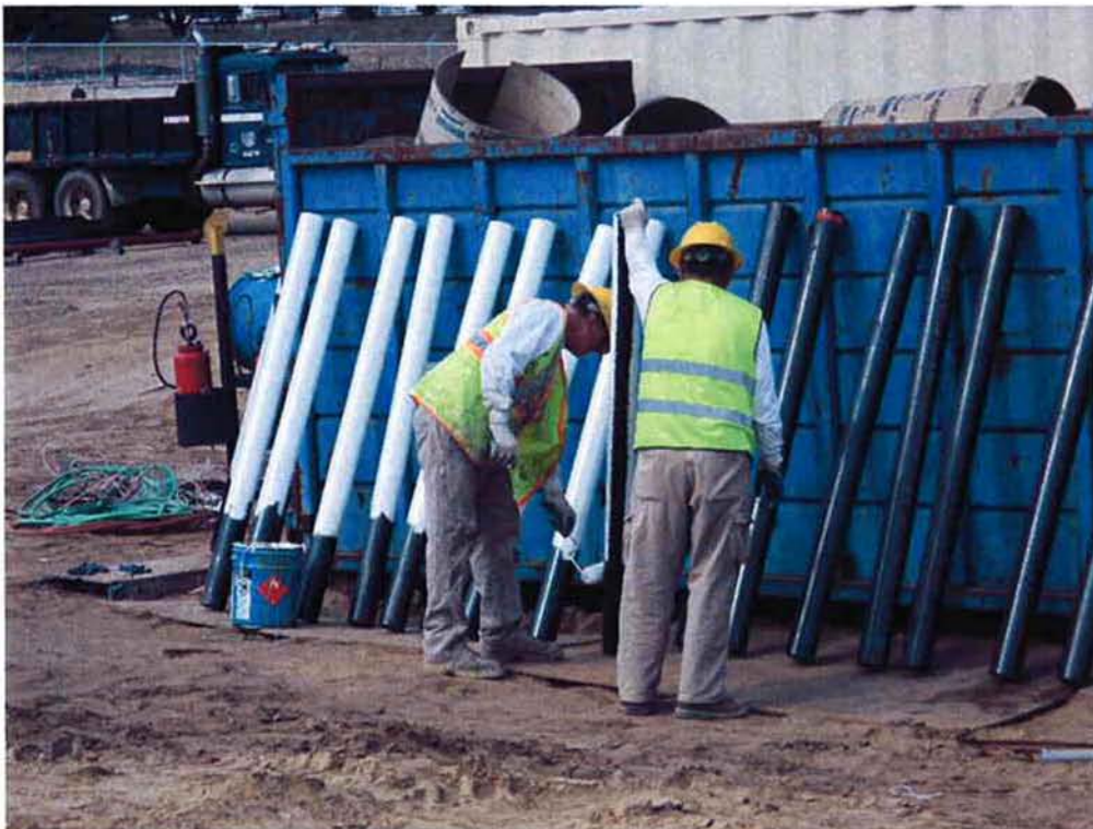
KNK Coating abrading the bollards and applying prime coat.
