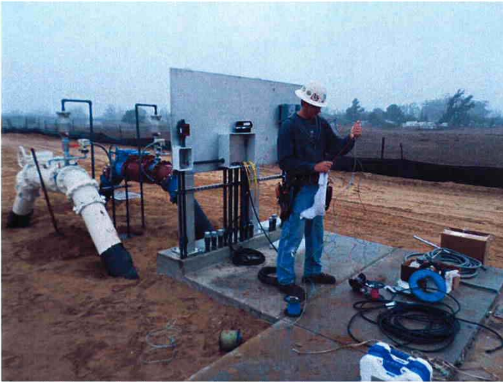
Bergelectric terminating wires at control panel.
