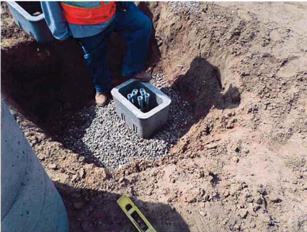
Bergelectric installing street light pull boxes.
