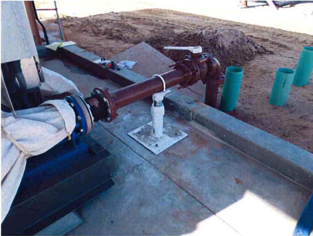
Cushman installing pipe support at WAS piping.
