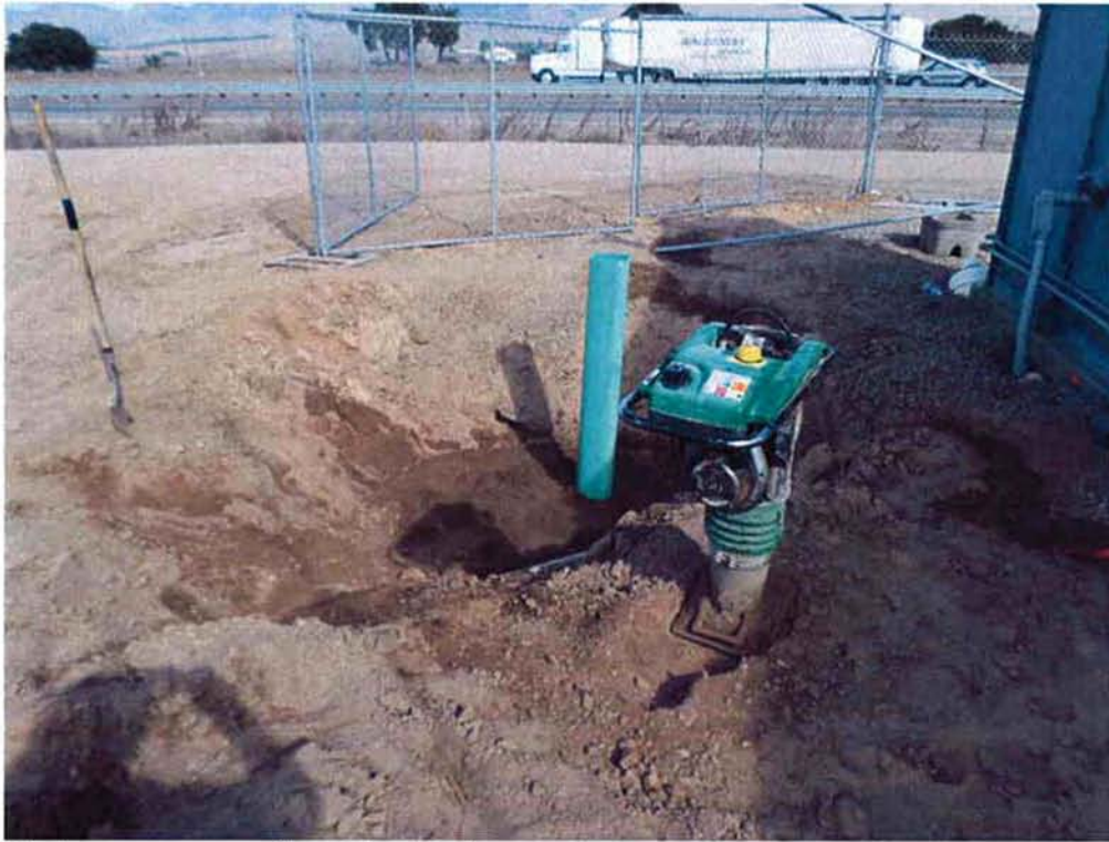
Cushman compacting 6-inch valve can.
