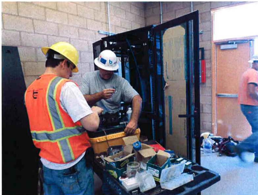
Cushman terminating the new fiber optic line.
