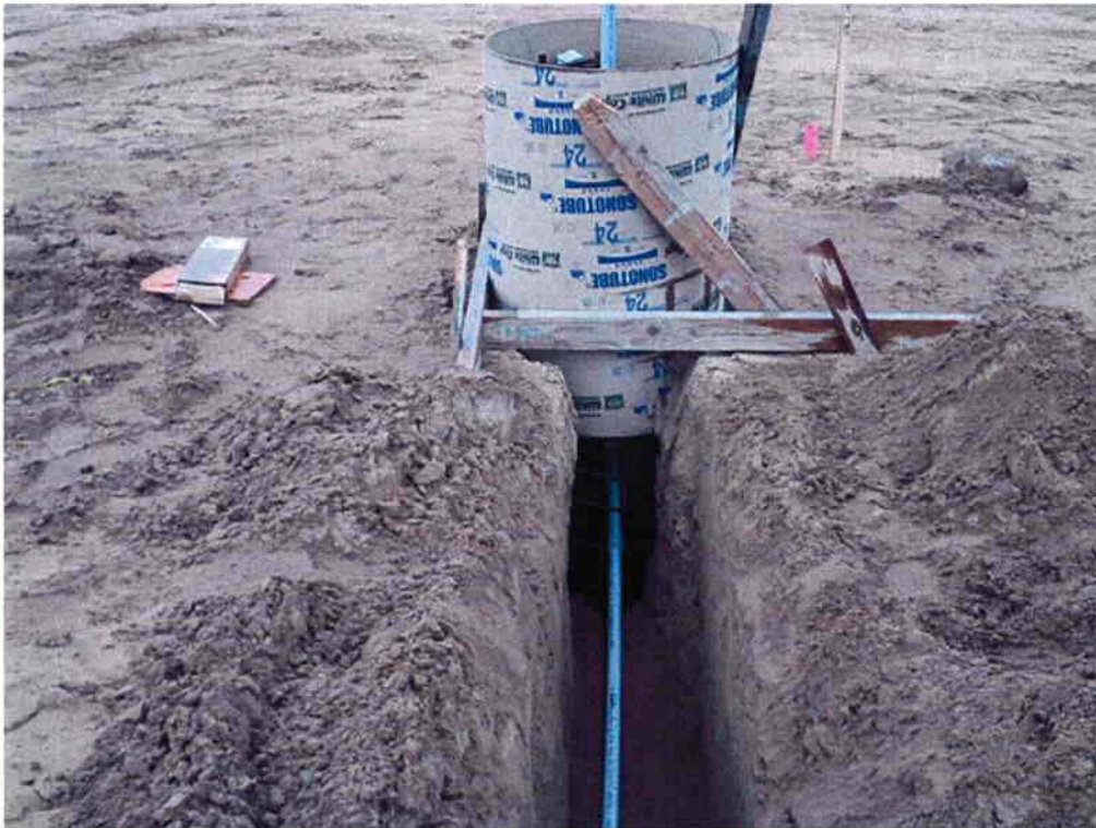
Bergelectric installing conduit to street light pole bases.
