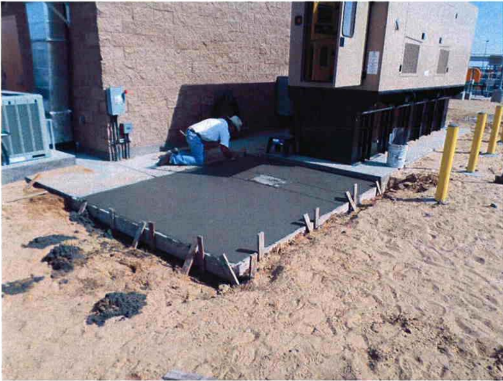
Cushman pouring slab for the aluminum stair landing at the emergency generator.
