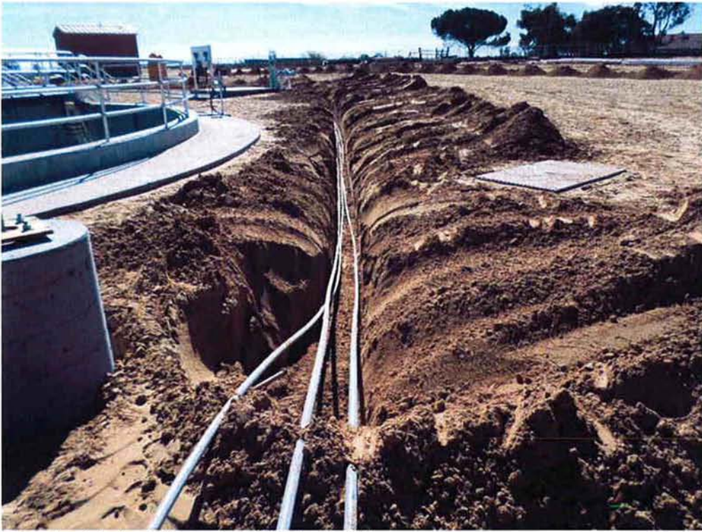
Bergelectric installing street light conduit.
