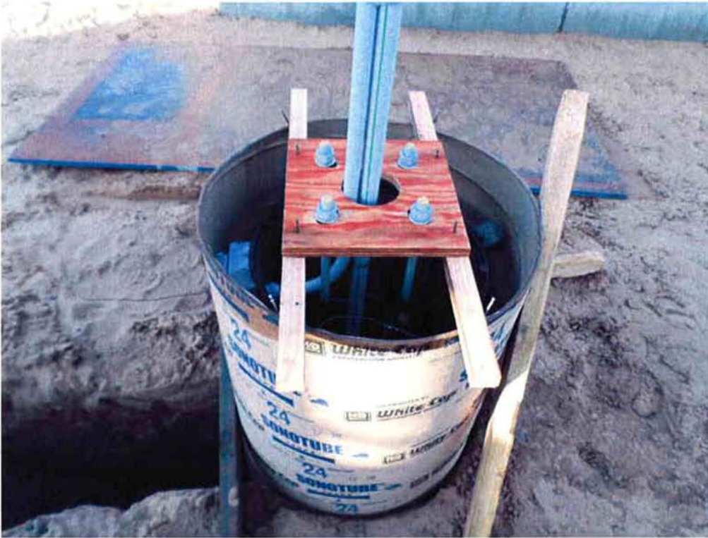
Street light base formed and ready for concrete.
