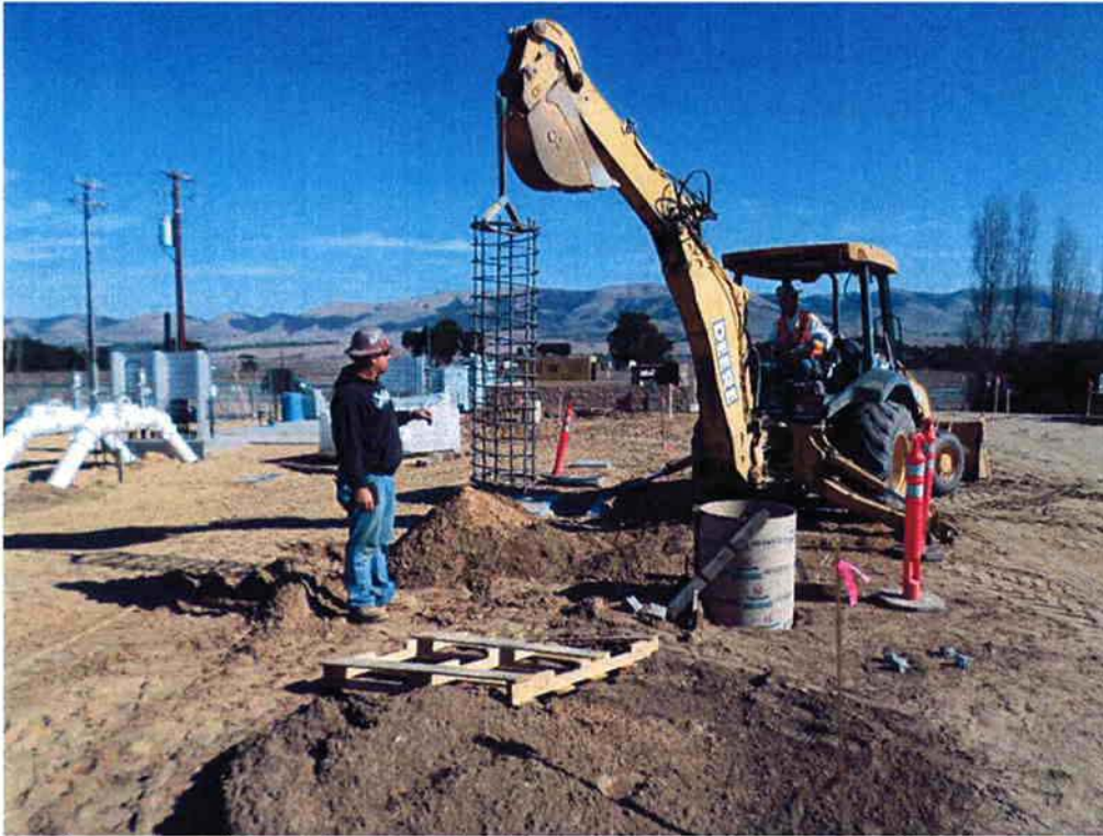
Cushman installing rebar cage inside sonotube for the street light bases.
