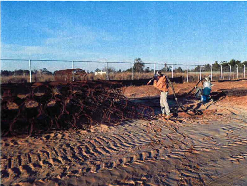
Cushman sandblasting rebar for street light bases.
