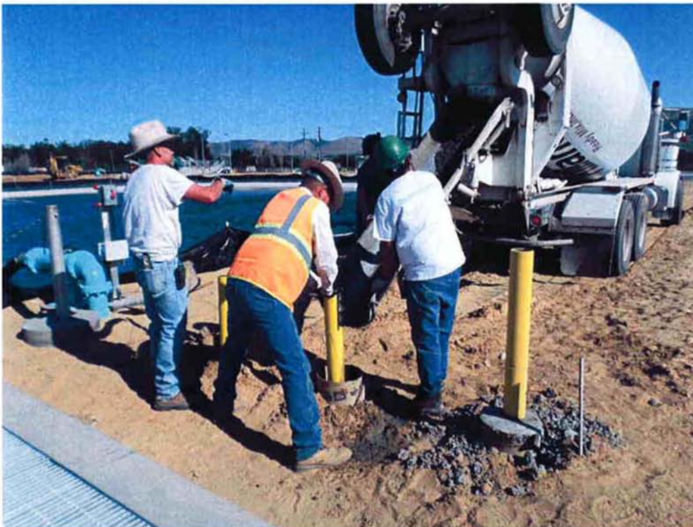
Cushman setting bollards and pouring concrete for bases.
