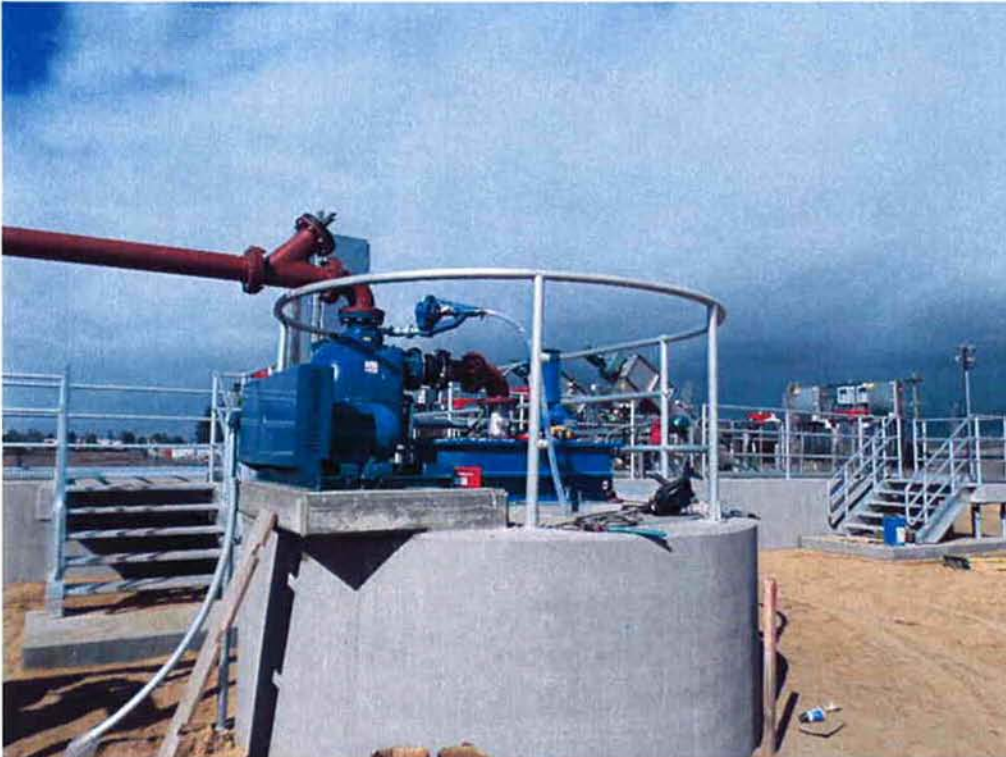
Cushman completing handrail installation at the headworks.
