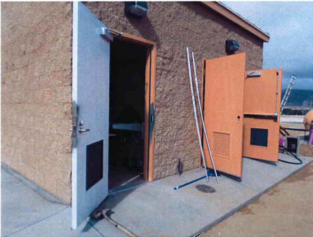
J & J Door installing door hardware at the Sodium Hypochlorite Storage Building.
