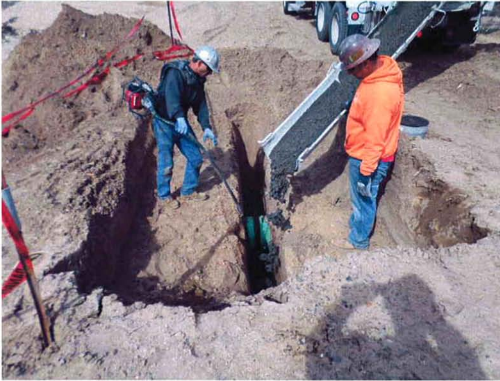
Cushman pouring concrete collar around pipe between Infiltration Ponds 1 & 2.
