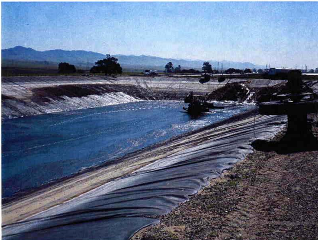
Cushman removing sludge from Influent Pond #3.
