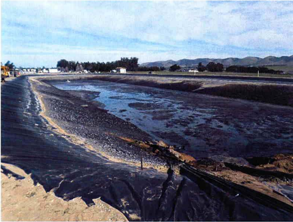
Cushman pumping sludge out of existing Influent Pond #3.
