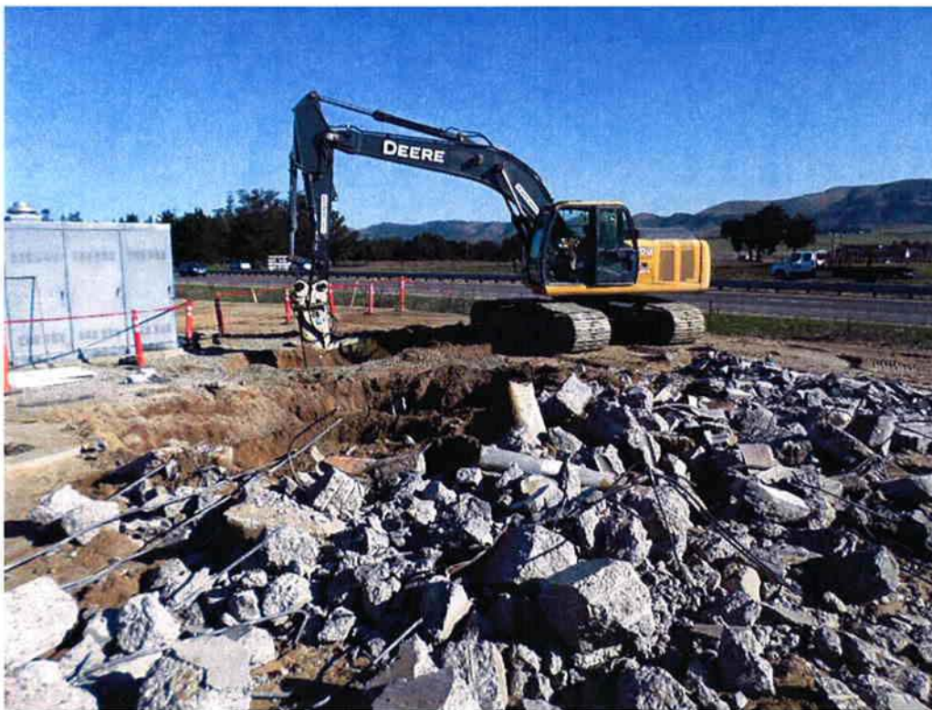
Cushman performing demolition at the existing wet well and manhole.
