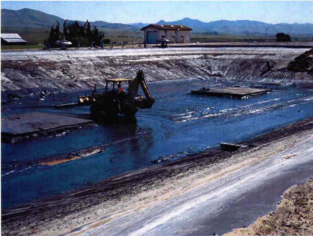
Cushman pushing and pumping sludge out of Influent Pond #2.
