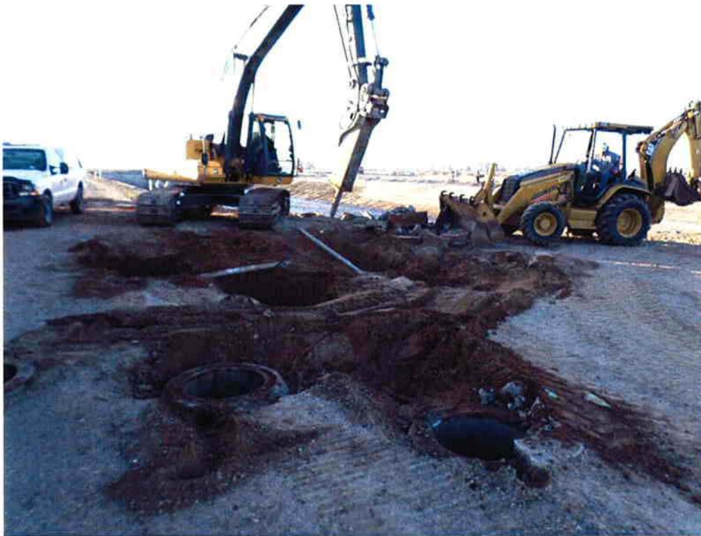
Cushman performing demolition of existing manholes.
