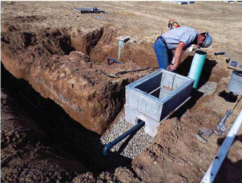
Cushman installing a pressure reducer on the 2-inch potable waterline.
