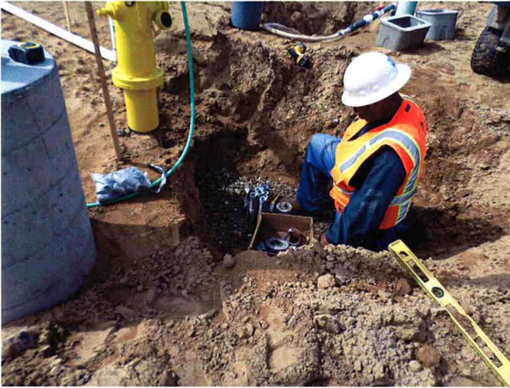
Bergelectric installing street light pull boxes.
