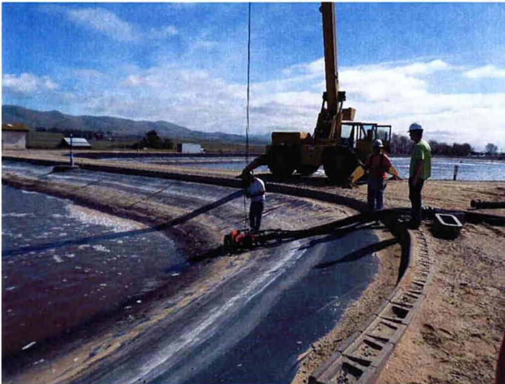
Cushman setting up pumps to pump sludge out of Influent Pond 2.
