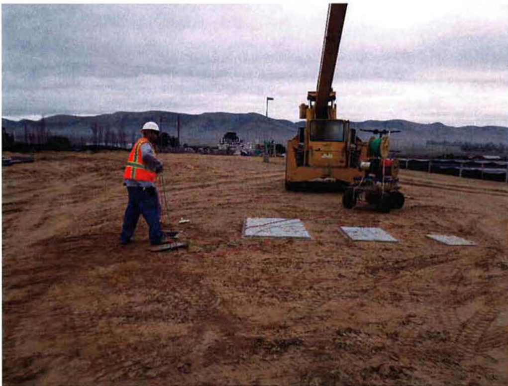
Bergelectric pulling wire for street lights.
