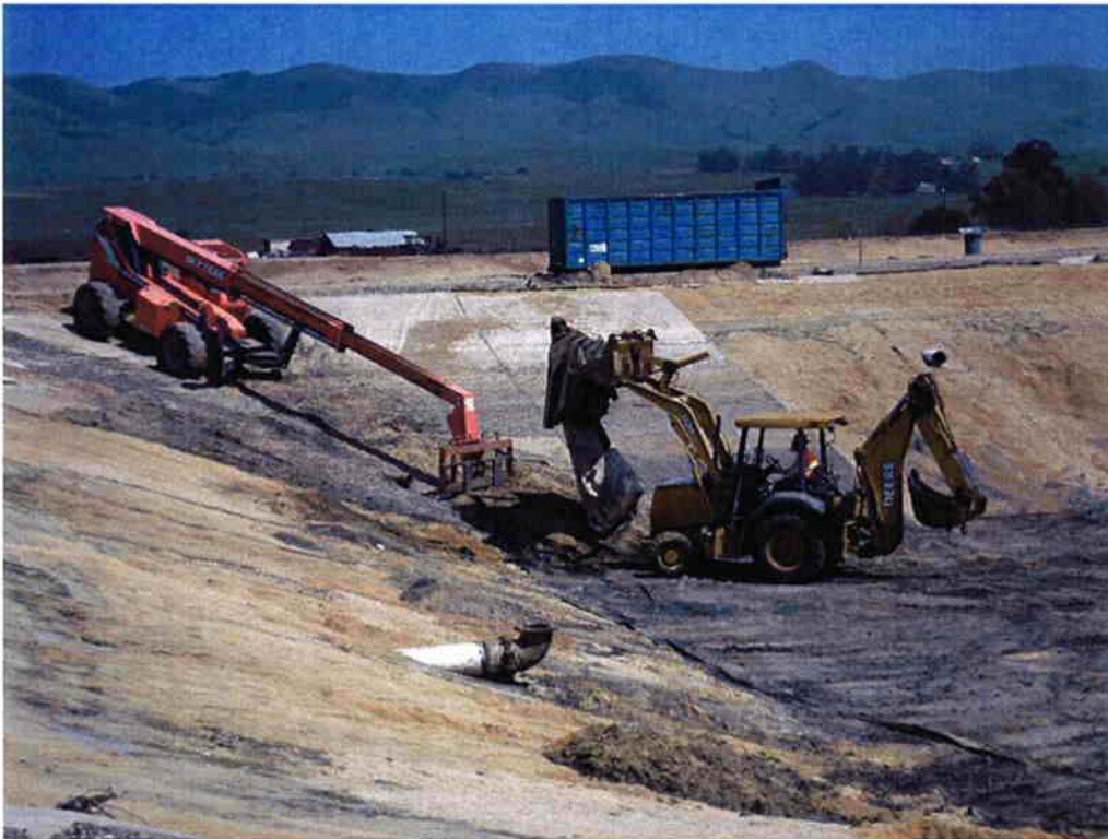
Cushman removing liner from Influent Pond #4.
