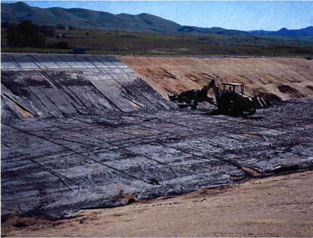
Cushman removing liner from Influent Pond #3.
