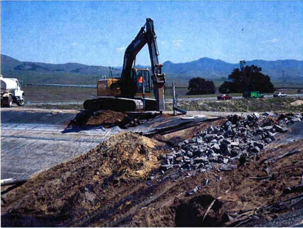
Cushman performing demolition of concrete structures at existing Influent Ponds.
