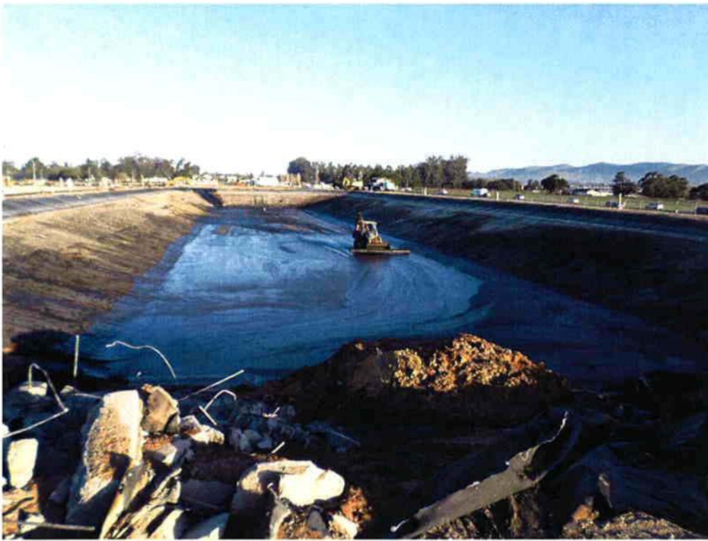
Cushman pushing sludge to pump in Influent Pond #3.
