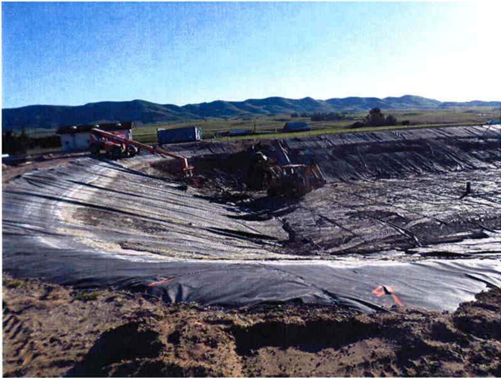
Cushman starting removal of the liner in Influent Pond #3.
