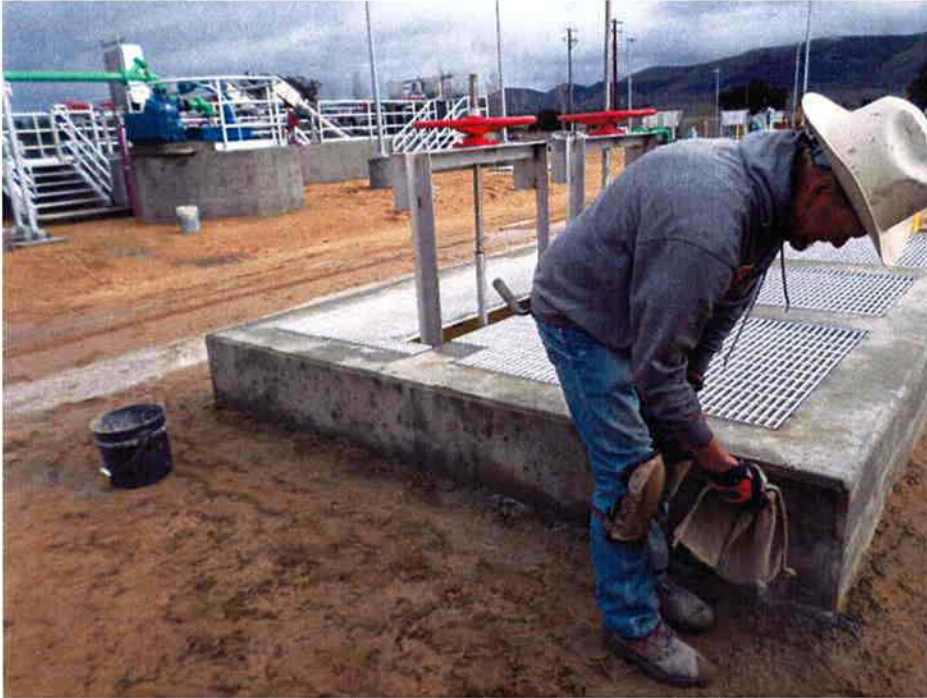
Cushman patching concrete and performing punch list items.
