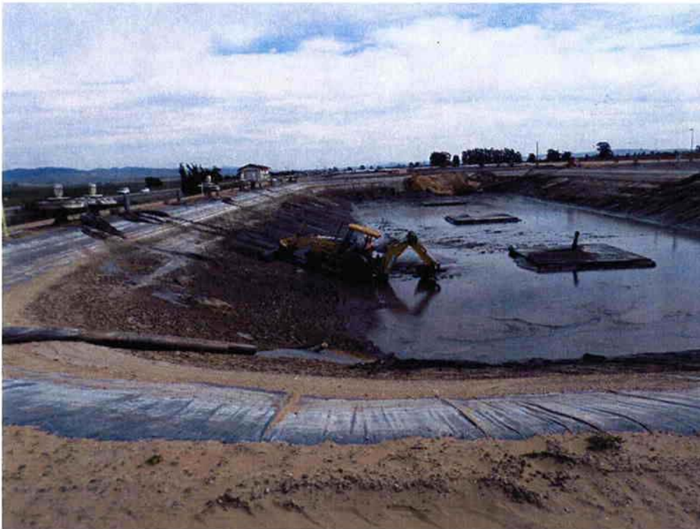
Cushman removing sludge from Influent Pond #2.
