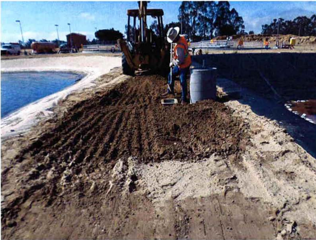
Cushman compacting around pull boxes for street lights.
