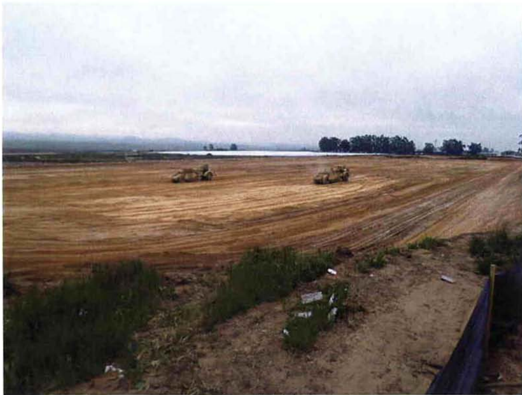
Switzer continuing work on Ponds 9 & 10 in Area F.
