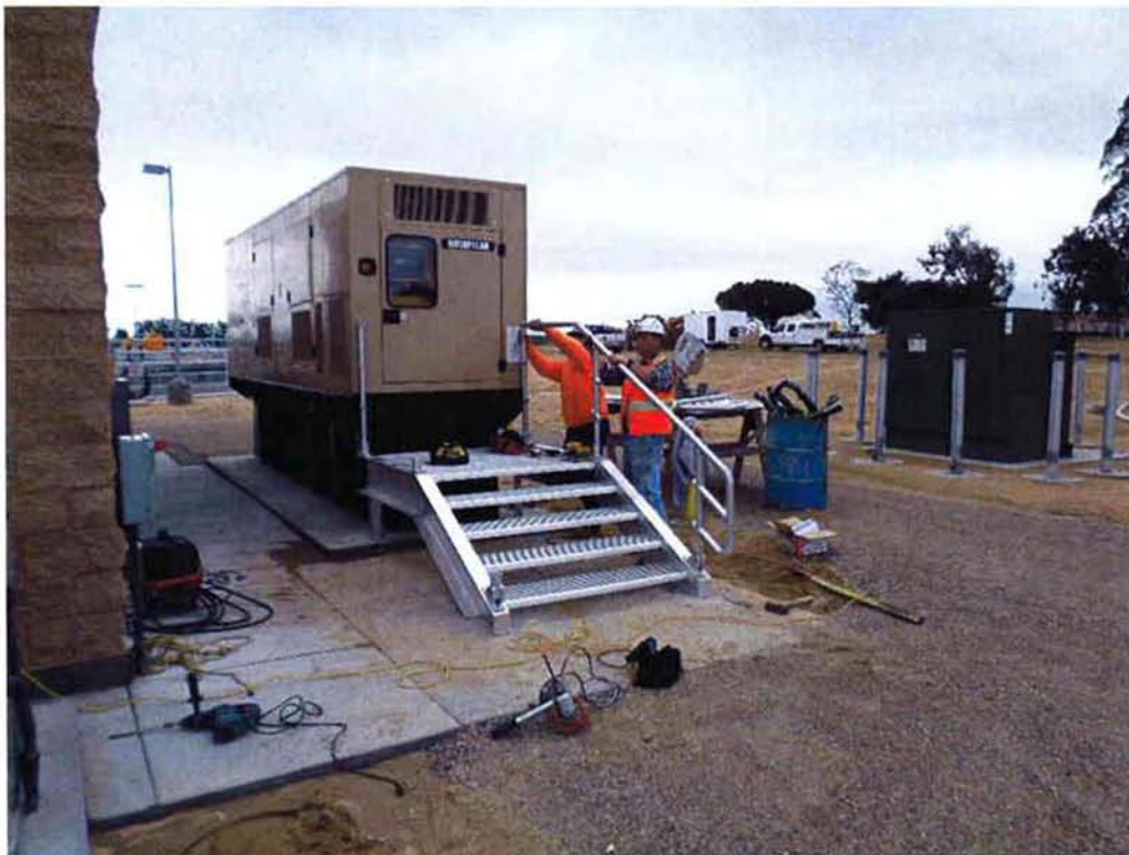
Cushman installing aluminum stairs and deck to access new emergency generator.
