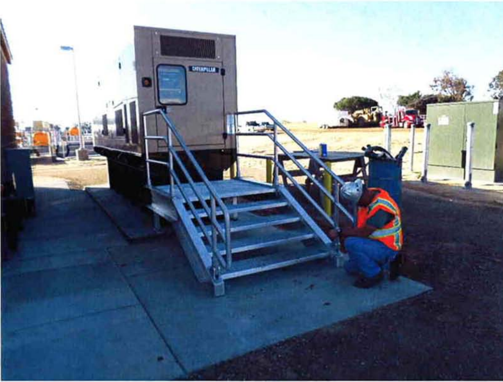
Cushman installing handrail at stairs for new emergency generator.
