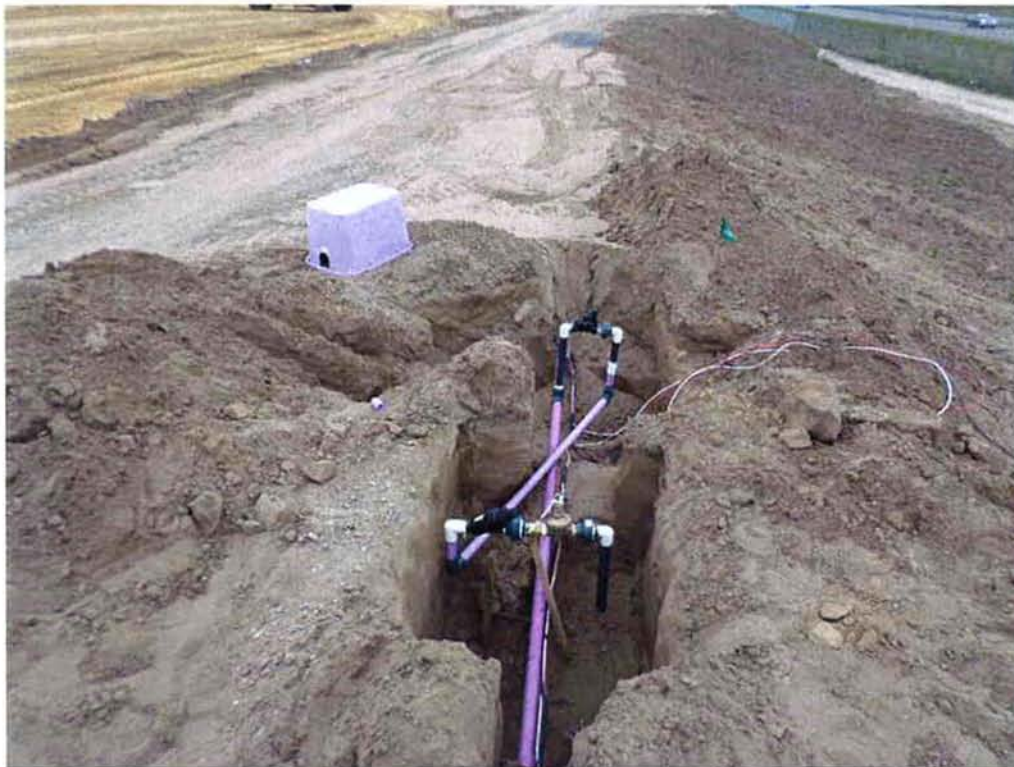
Installing piping for landscaping.
