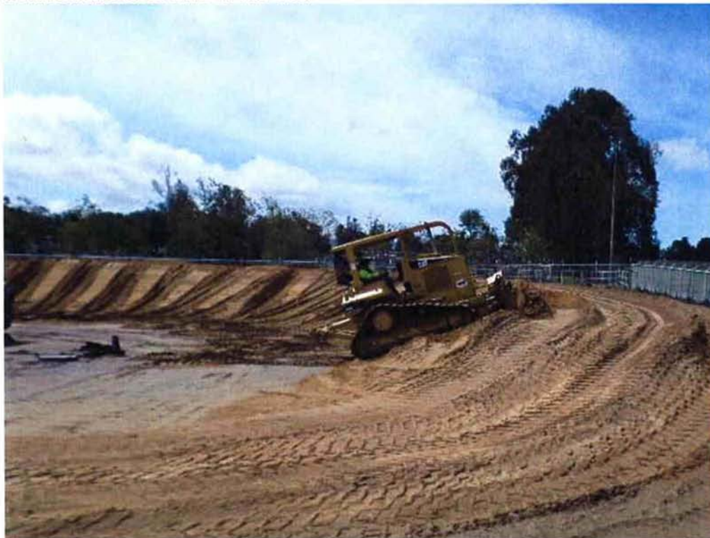
Switzer shaping berm on the west side of the site.
