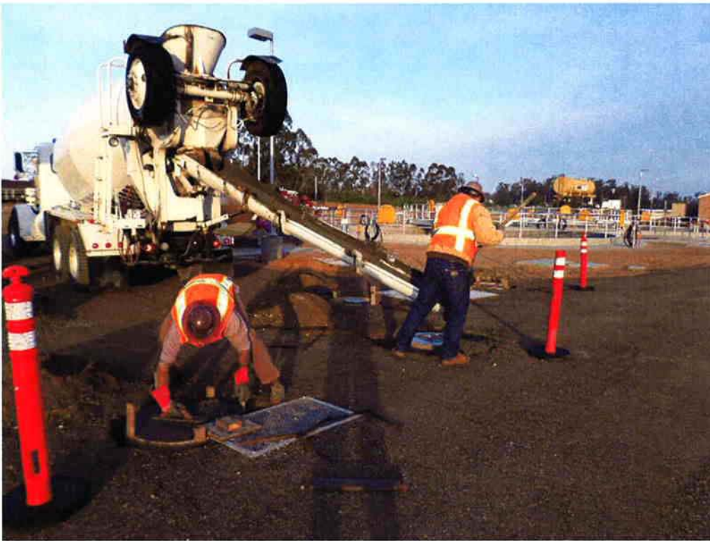
Cushman pouring concrete collars around valves.
