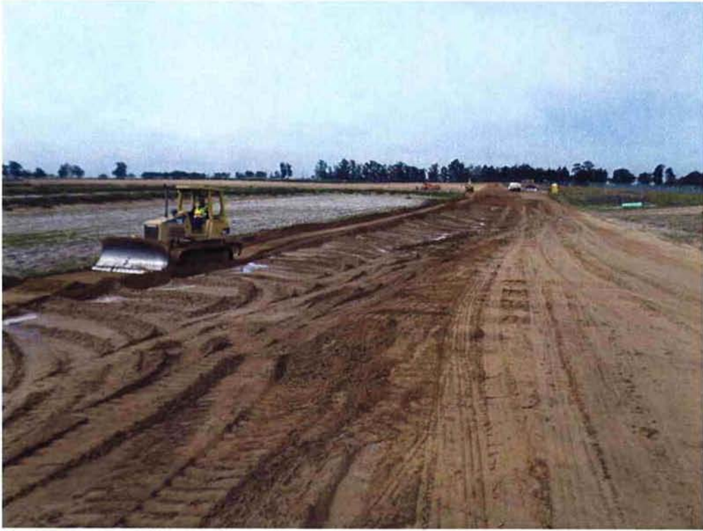
Cushman backfilling and compacting over new 24-inch SE pipe to Ponds 9 & 10.
