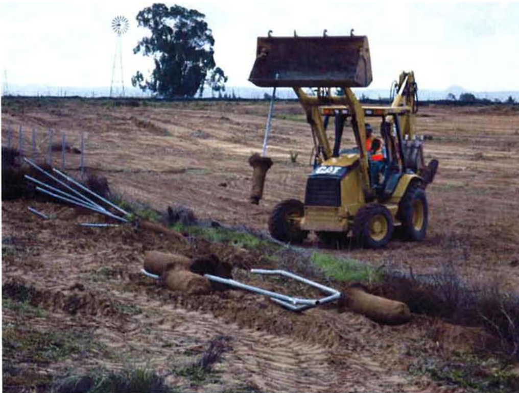
Cushman removing existing fence around Area F.
