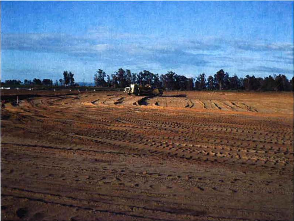
Switzer excavating Ponds 9 & 10 in Area F.
