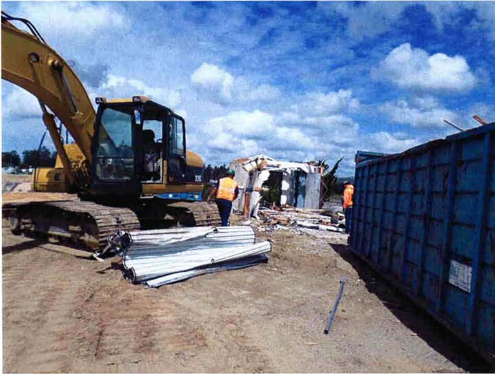
Demolition of existing blower building.
