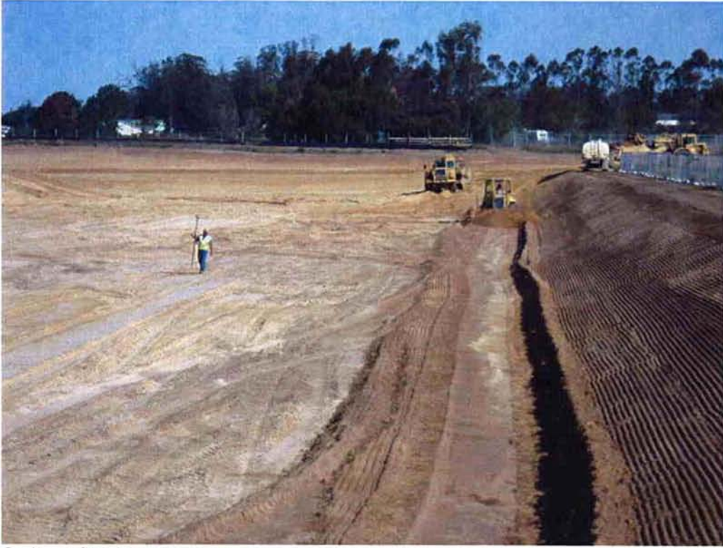
Switzer finishing the bottom of Ponds 9 & 10 and checking grade.
