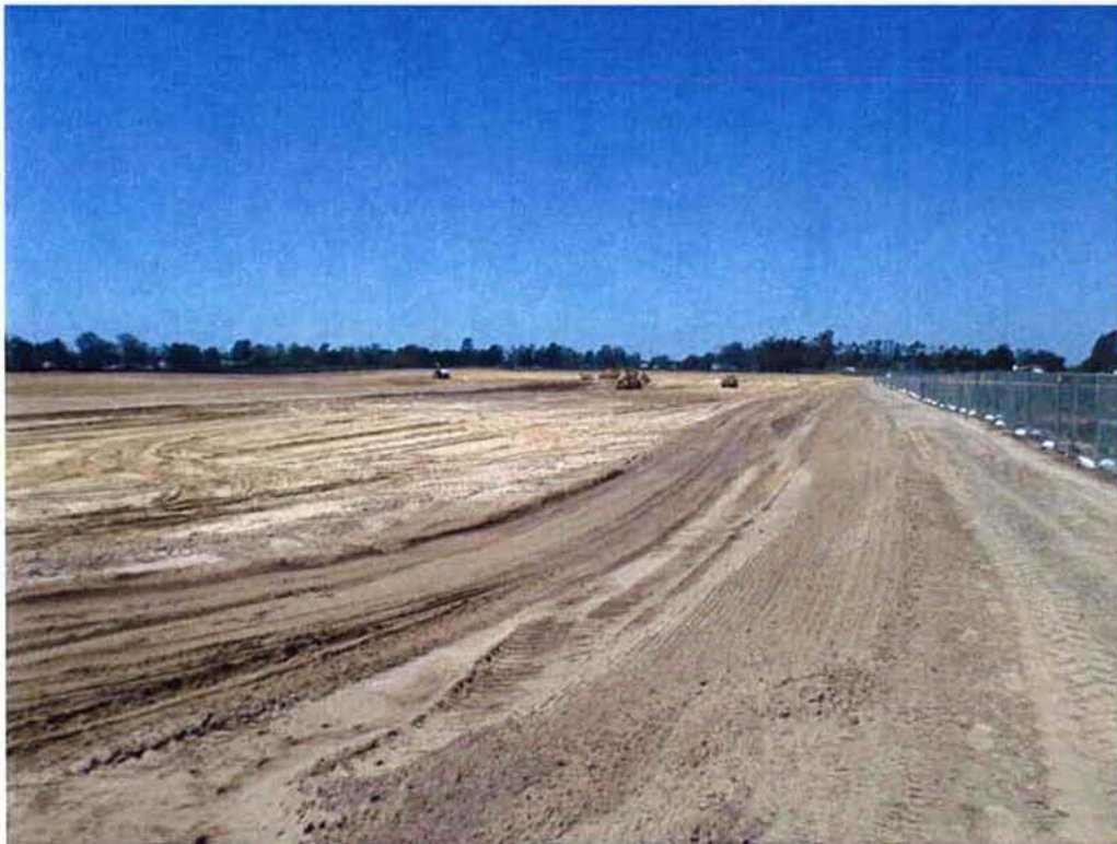
Switzer continuing to excavate in Area F to build Ponds 9 & 10.
