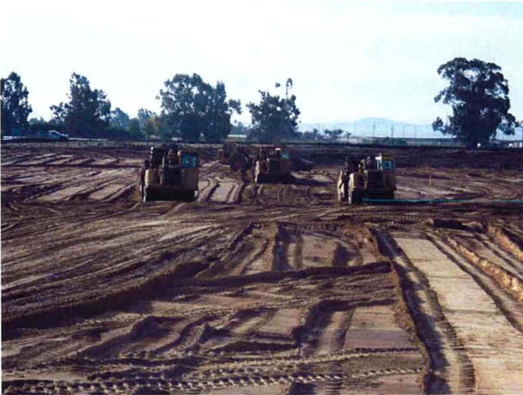
Switzer excavating material from Area F to build Ponds 9 & 10.
