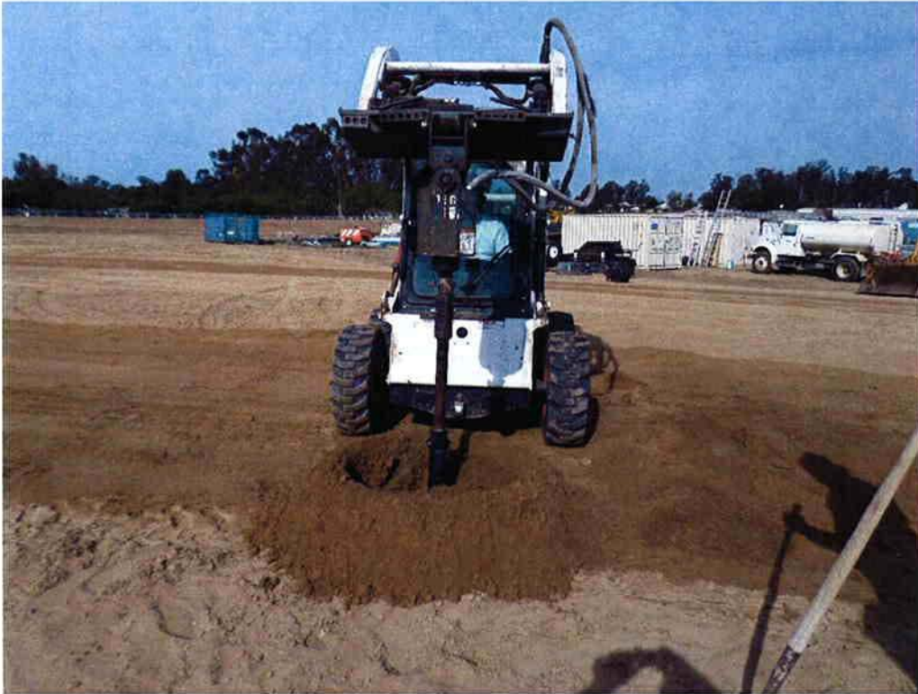
Cushman using auger to bore hole for remaining street light bases.
