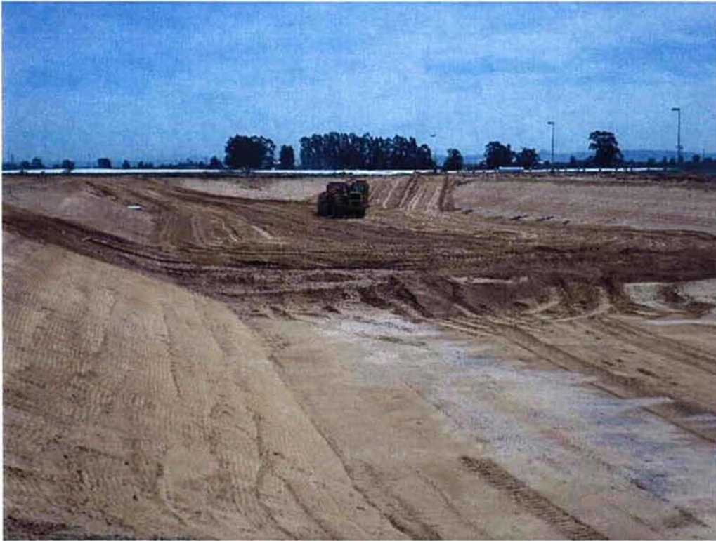
Switzer filling Pond 4 and creating berm for future Aeration Basin #2.
