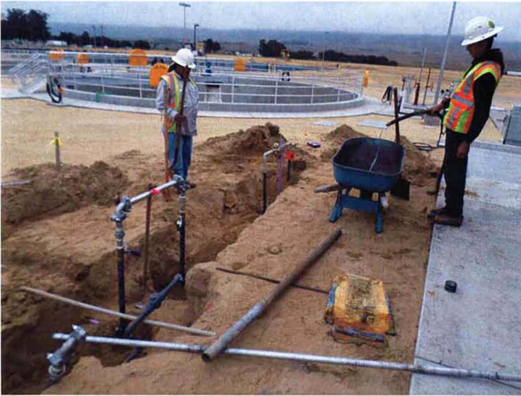
KCI Environmental installing back flow prevention assembly.
