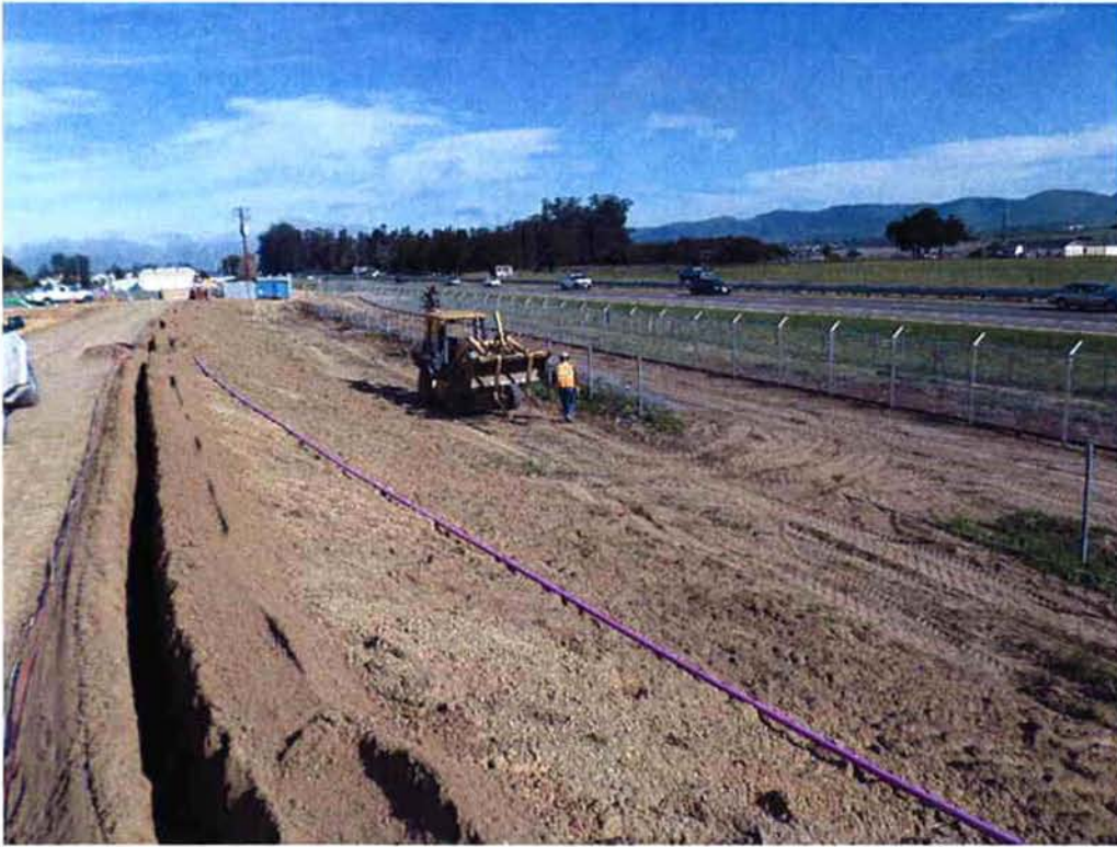
Cushman removing shrubs and existing chain link fence.
