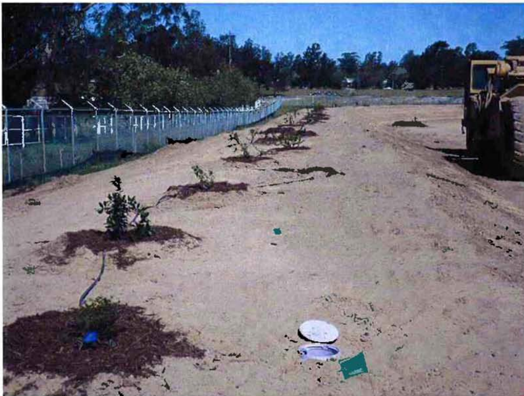
KCI Landscaping placing mulch around new plants on east berm.
