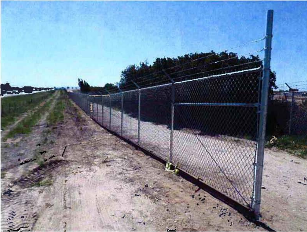
New fencing being installed along the Hwy 101 border.
