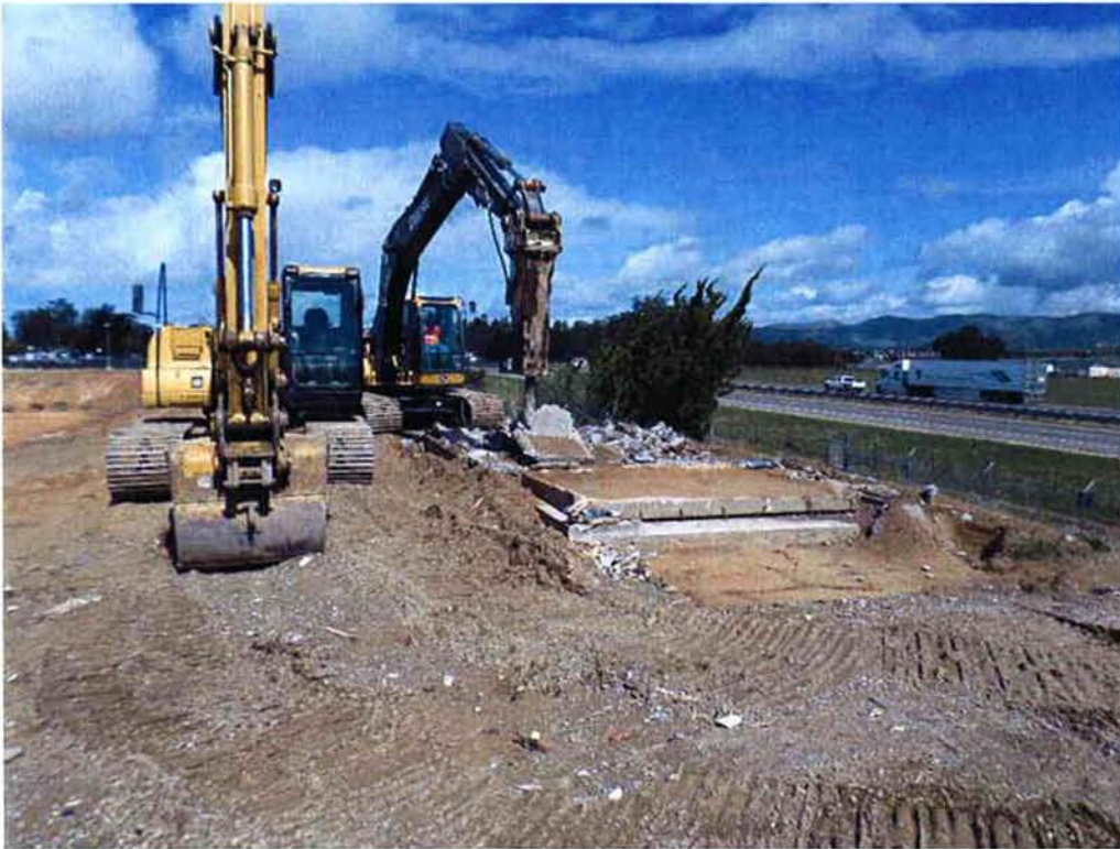
Cushman completing demolition of the existing building.
