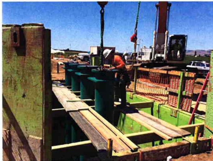
Pump Can Installation - Bottom
