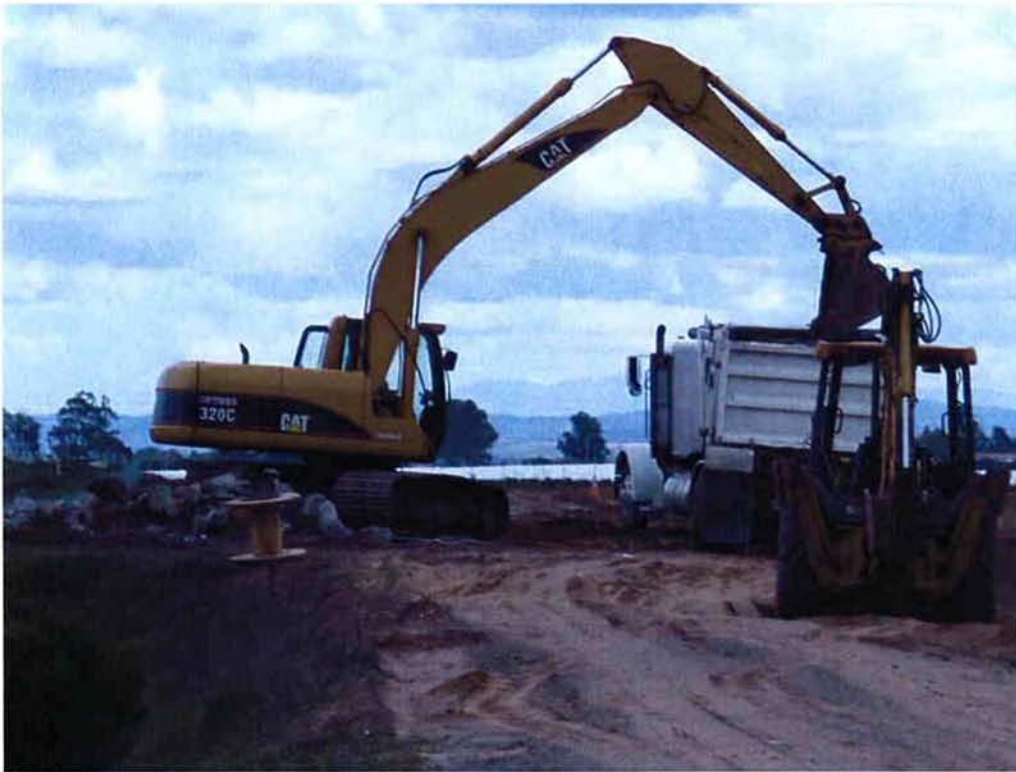
Cushman loading and hauling debris from existing building.
