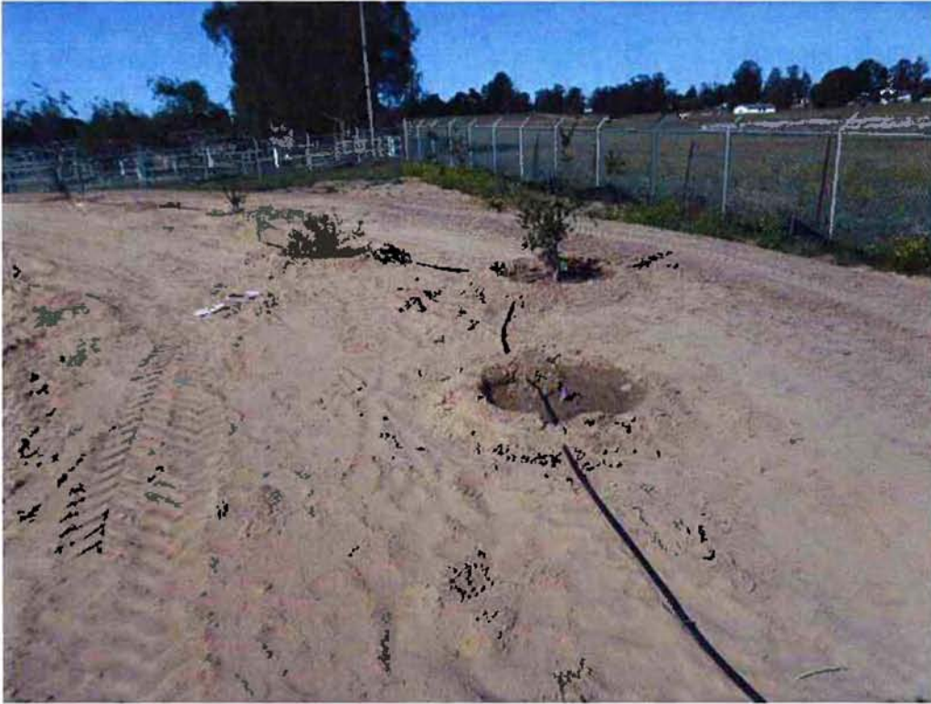
KCI Environmental installing irrigation lines to new plants.
