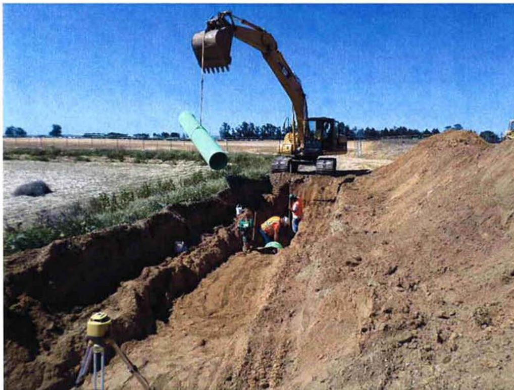
Cushman installing 24-inch SE piping to Ponds 9 & 10.
