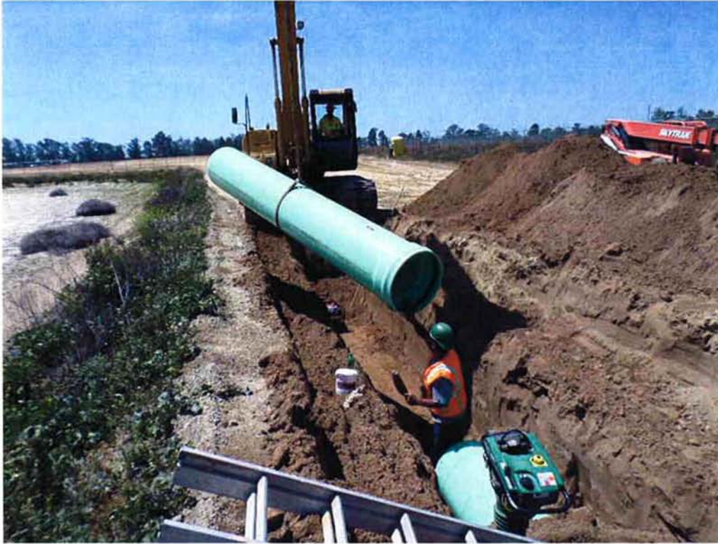
Cushman installing 24-inch SE piping to Ponds 9 & 10.
