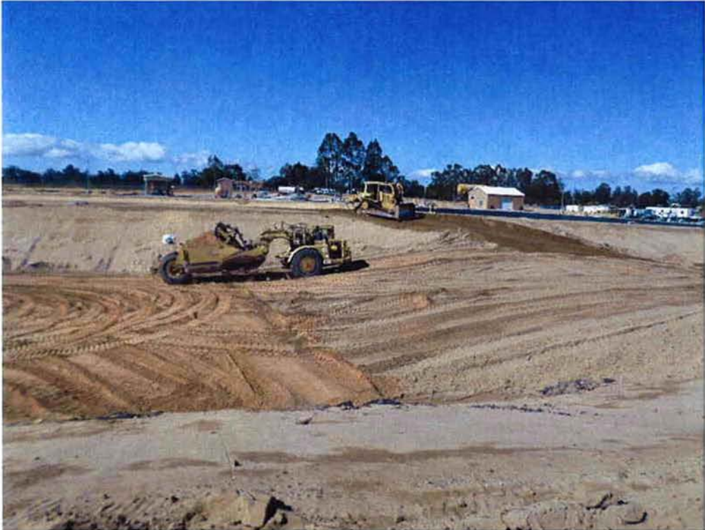
Switzer filling Ponds 2 & 3 with native material from Ponds 9 & 10.
