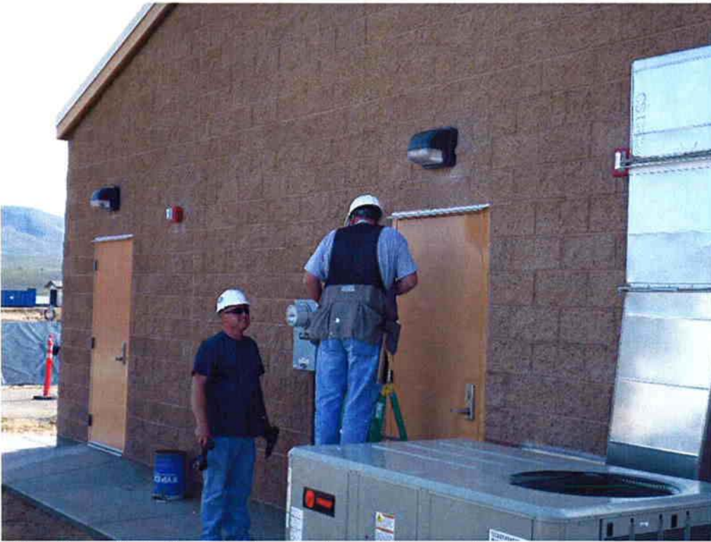
J N J Doors installing aluminum rain guards over doors.
