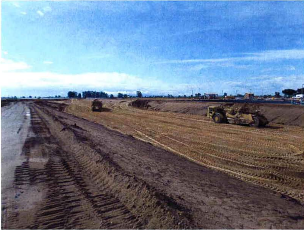
Switzer continuing to fill Ponds 2 & 3 with native material.
