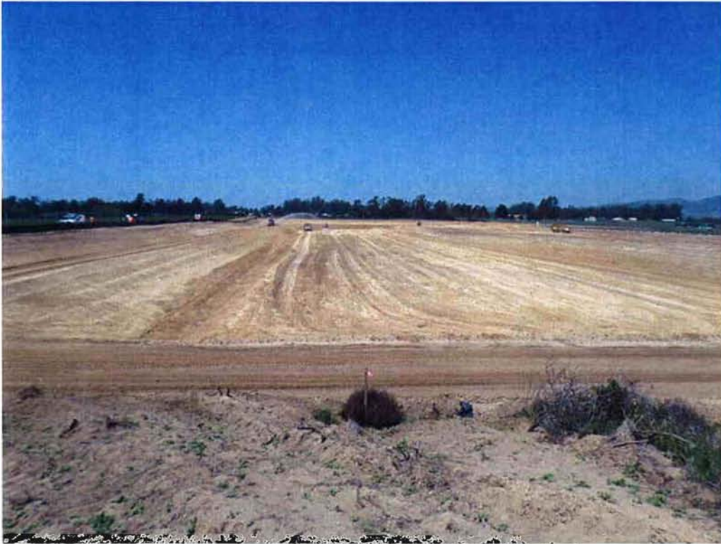
Switzer continuing to excavate material to build Ponds 9 & 10.
