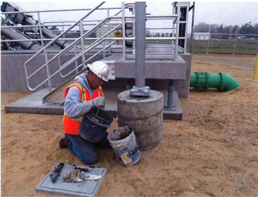
Cushman grouting street light bases.
