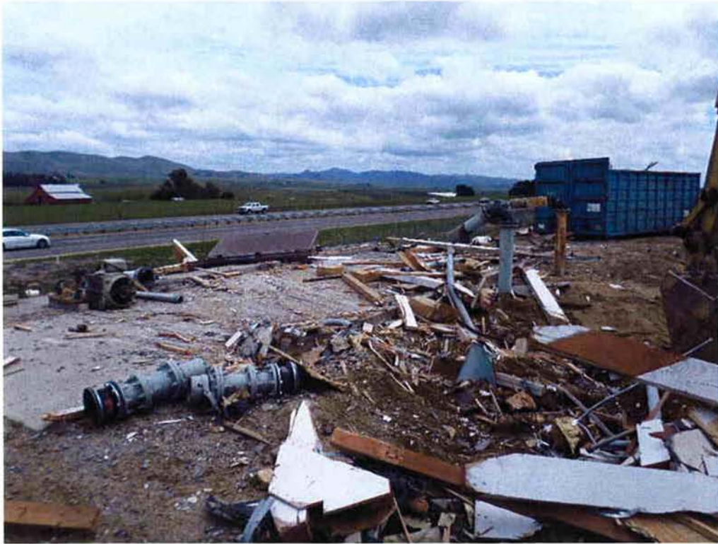
Demolition of existing blower building.
