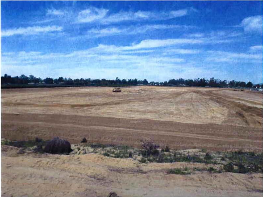
Switzer excavating Area F for Ponds 9 & 10.
