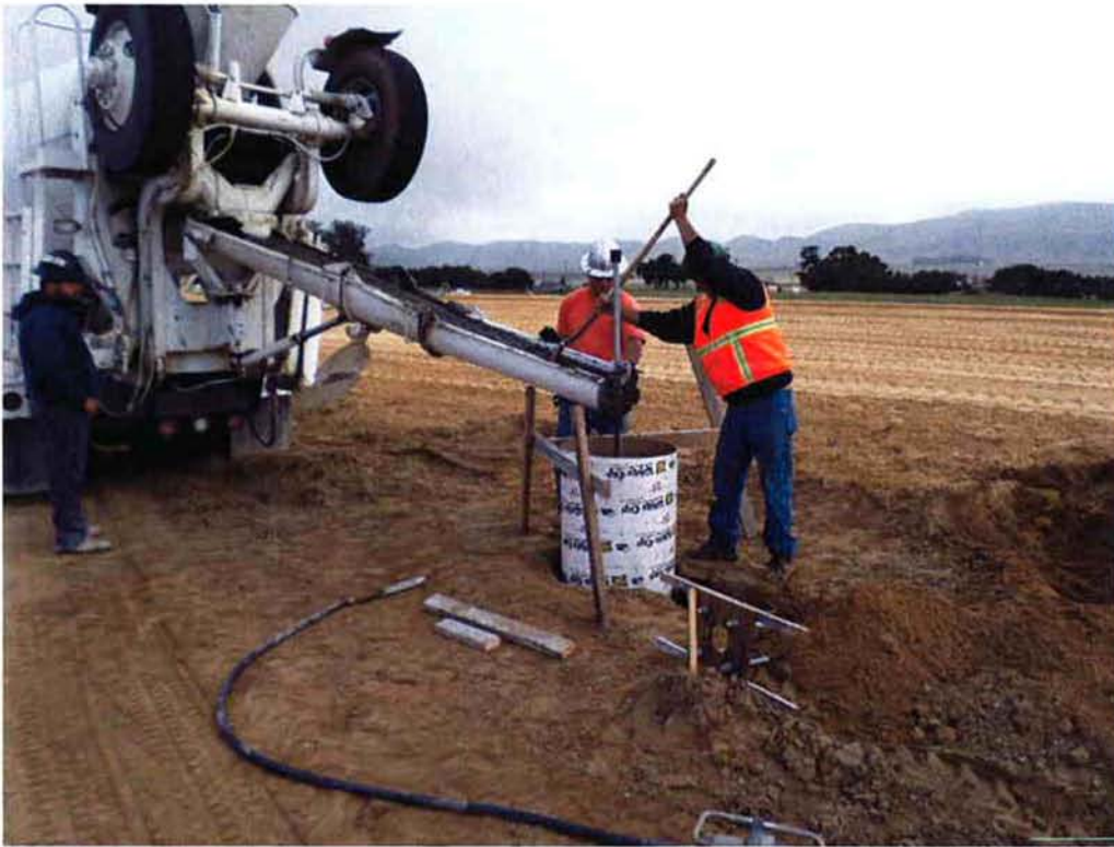
Cushman pouring bases for remaining street lights.
