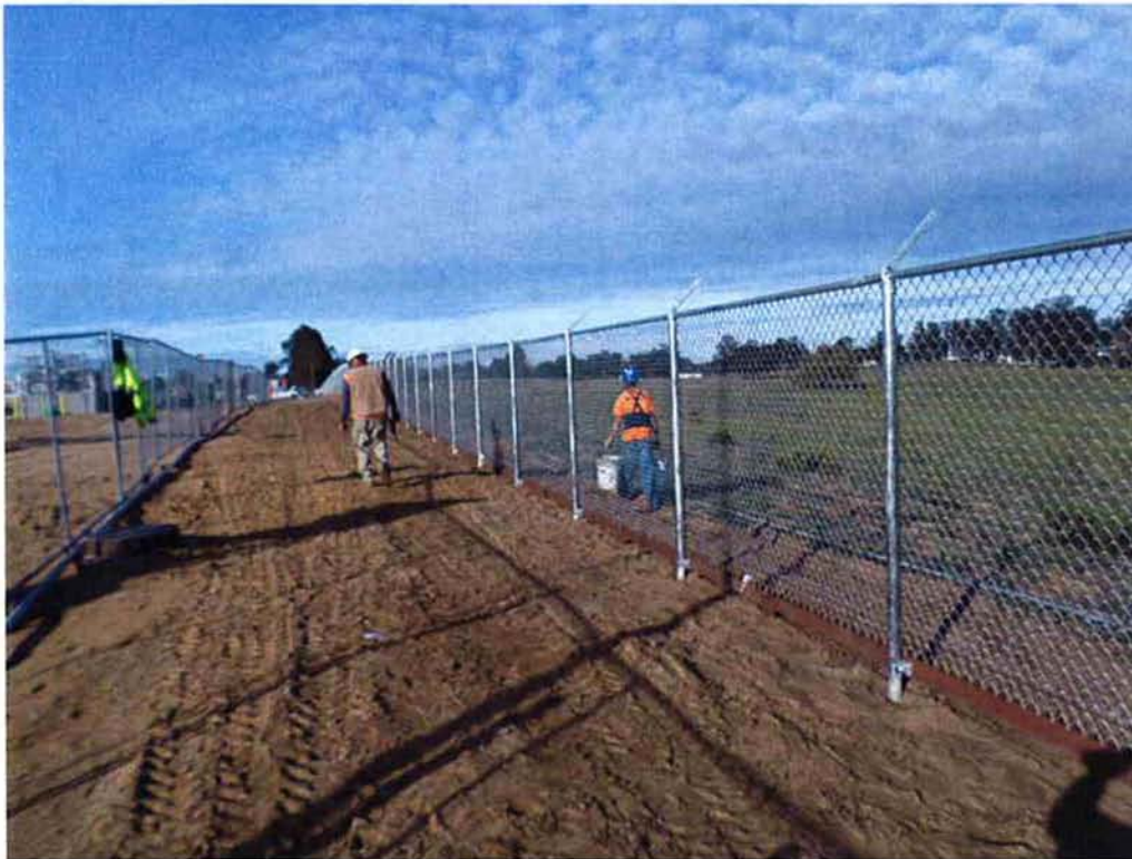
Fencing on the north side of the WWTF installed.
