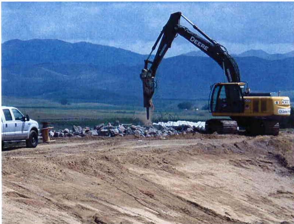
Cushman breaking up slab from existing building.
