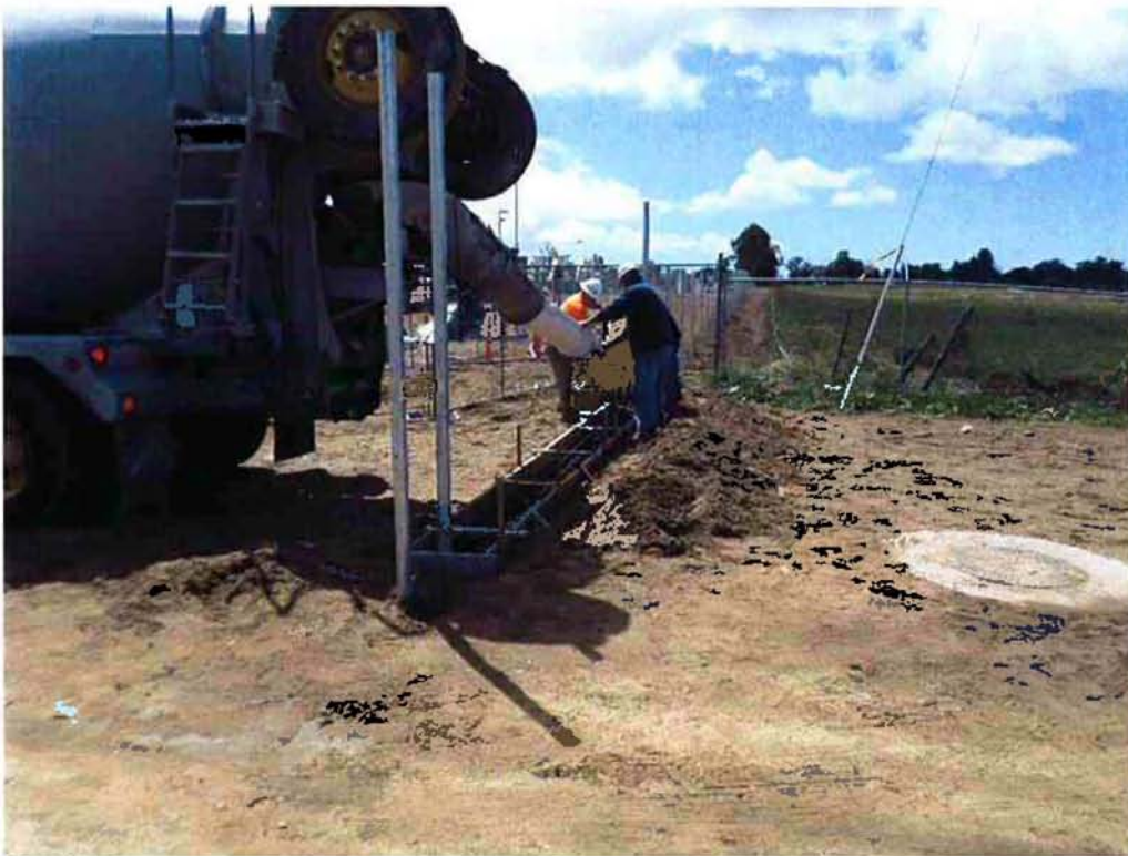
Cushman pouring concrete channel for new electric gate at site entrance.
