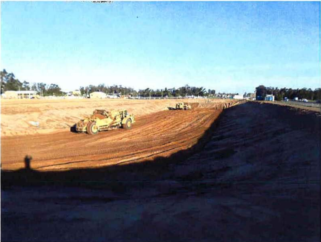
Switzer filling existing Ponds 2 & 3 with native material from construction of Ponds 9 & 10.
