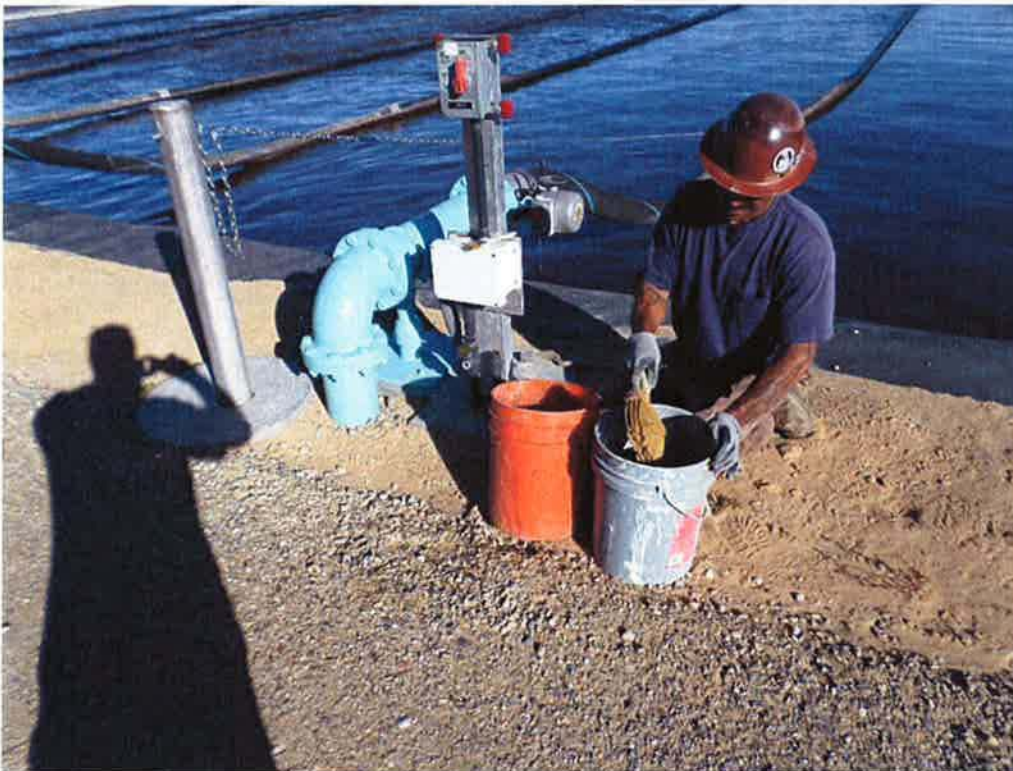
Cushman dry-packing electric stand at motorized valves for Aeration Basin #1.
