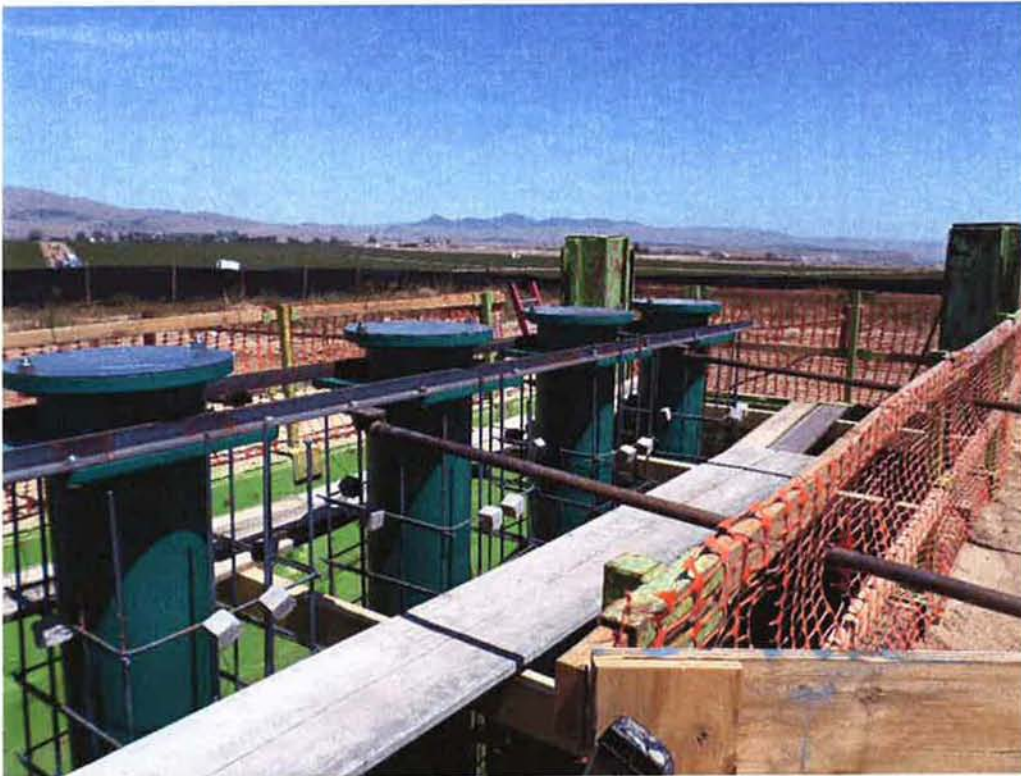
Spiess installing stabilizing structure/bracing to the tops of the pump cans.
