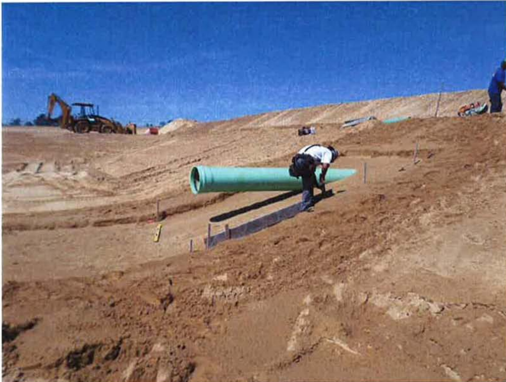
Cushman forming splash pads at new Ponds 9 & 10.
