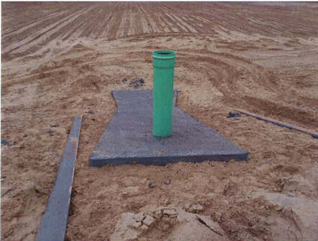
Completed concrete discharge pad after forms are removed.
