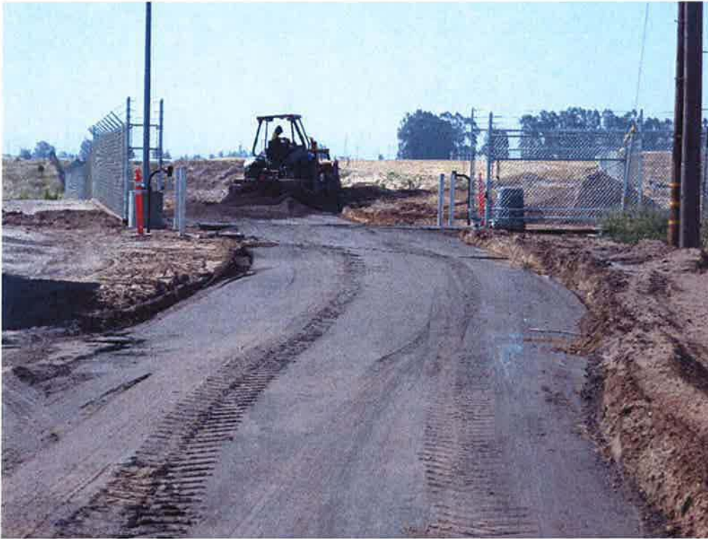
Switzer placing aggregate base for new road at site entry.
