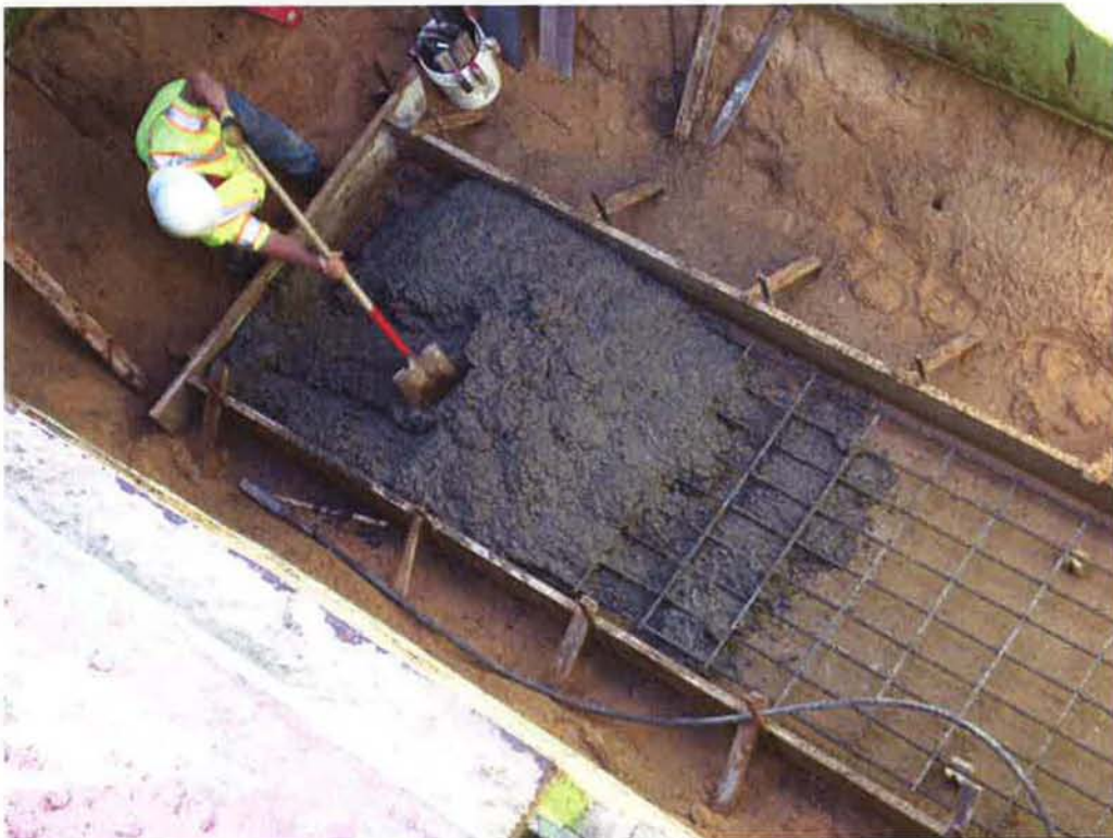
Spiess pouring concrete slab to set pump cans on top of.
