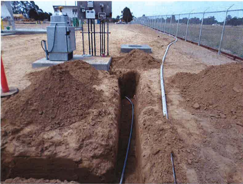
KCI Environmental installing conduit to landscaping controller.
