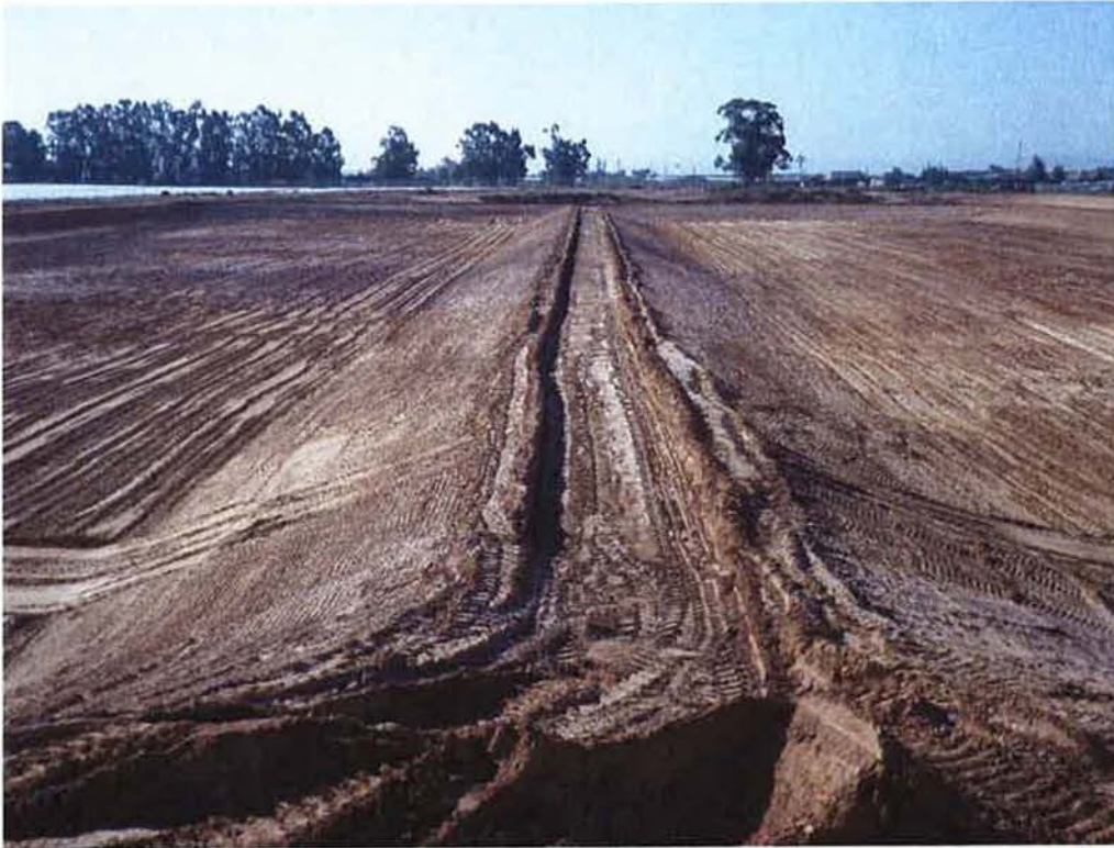
Switzer cutting new road between Ponds 9 & 10 to subgrade.
