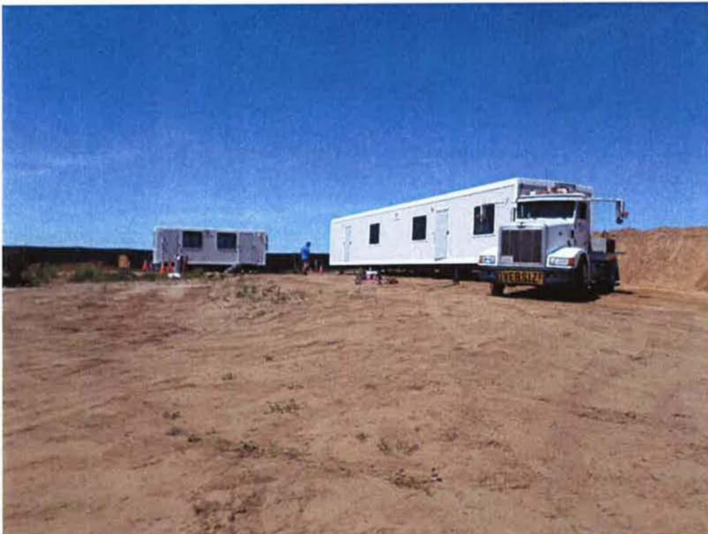
Jobsite trailers arriving on site.
