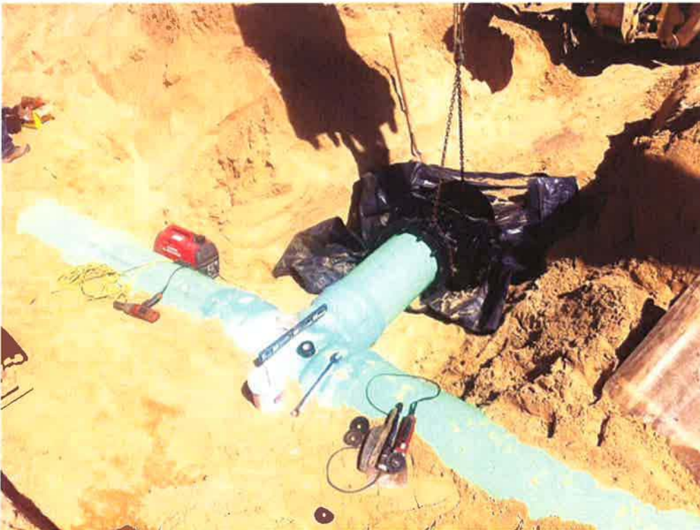
Cushman installing 18-inch plug valve off 24-inch SE line at Pond 9.
