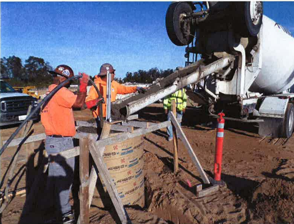
Cushman pouring the new SCADA tower base.
