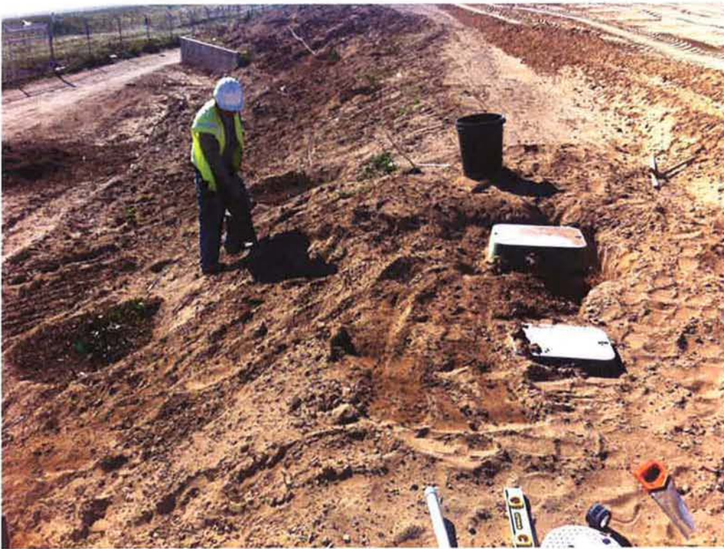
KIC Environmental installing new valve boxes on berm along Hwy 101.
