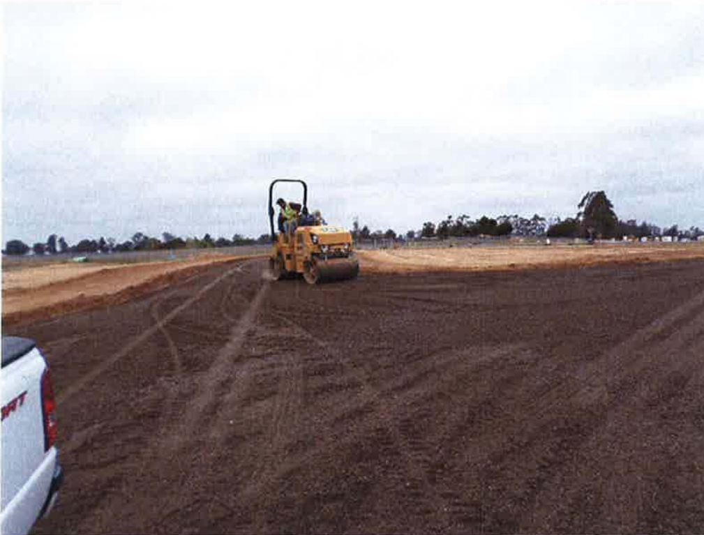
Switzer Excavating compacting aggregate base material for new site roads.
