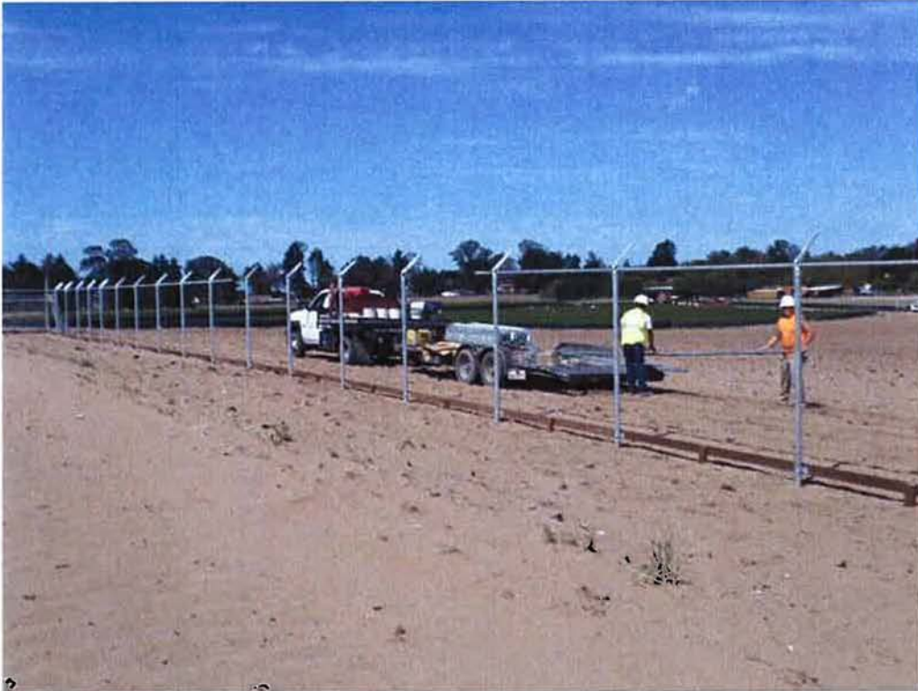
Cushman's fencing subcontractor, Valley Fencing, completing new fencing around Ponds 9 & 10.
