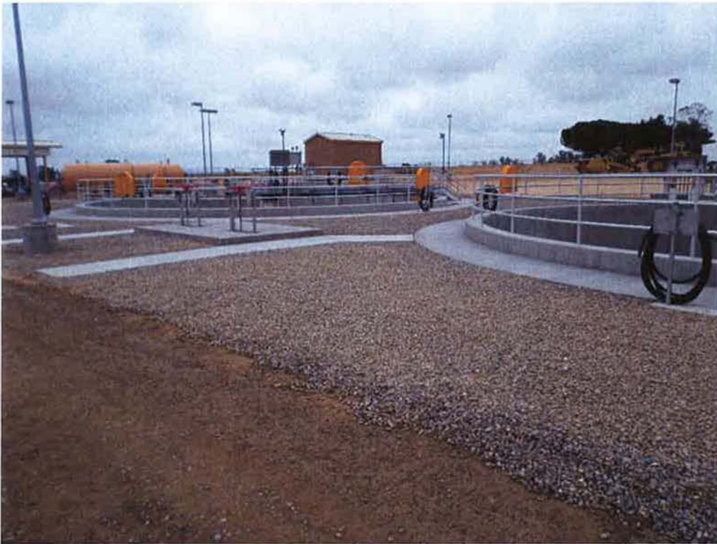
3/4-inch rock around the clarifiers.
