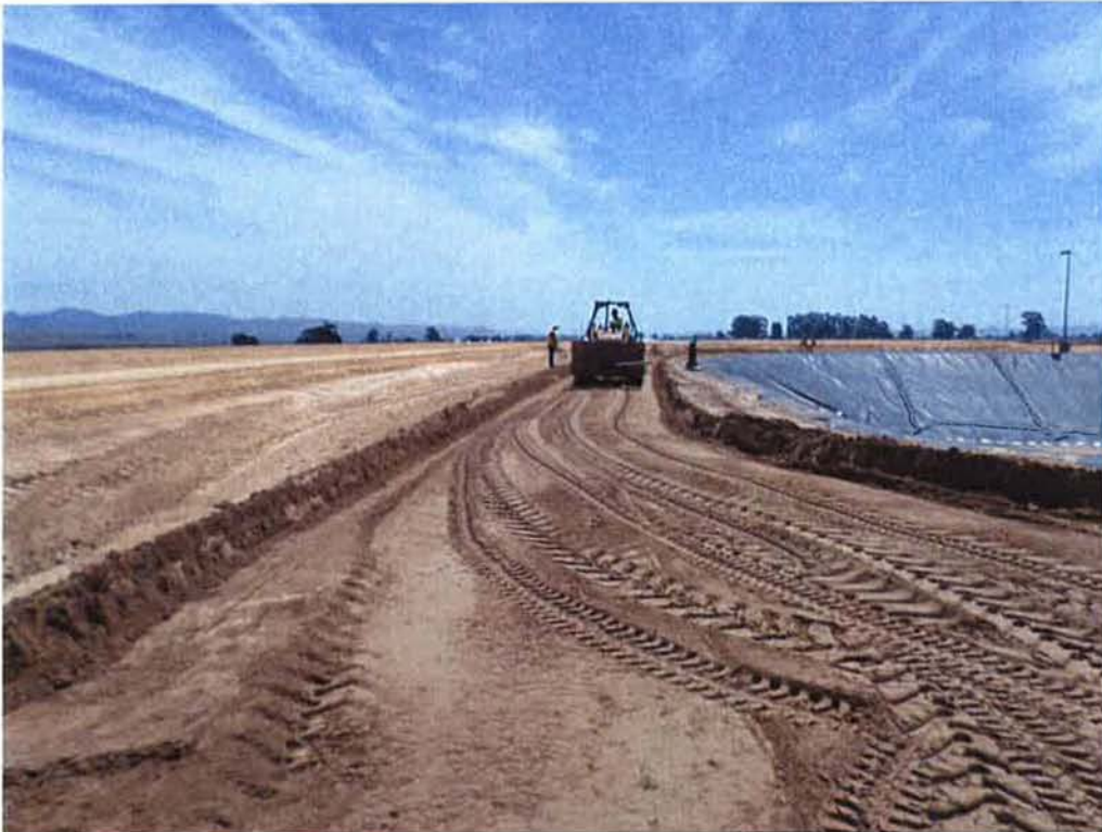
Mark Switzer Excavating cutting new site roads to subgrade.
