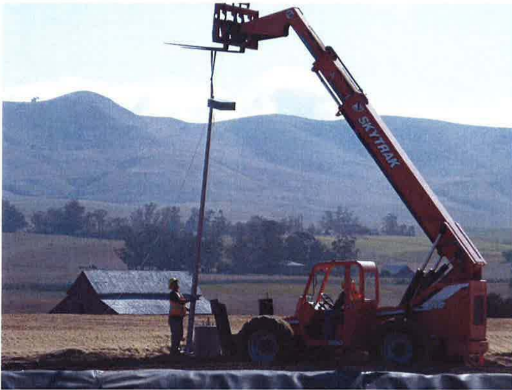
Cushman and Bergelectric setting light posts.
