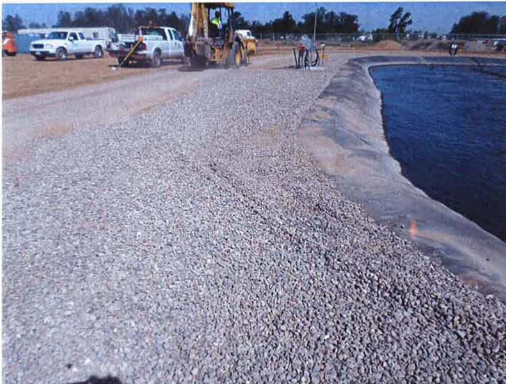
\frac{3}{4} -inch rock placed around Aeration Basin #1.
