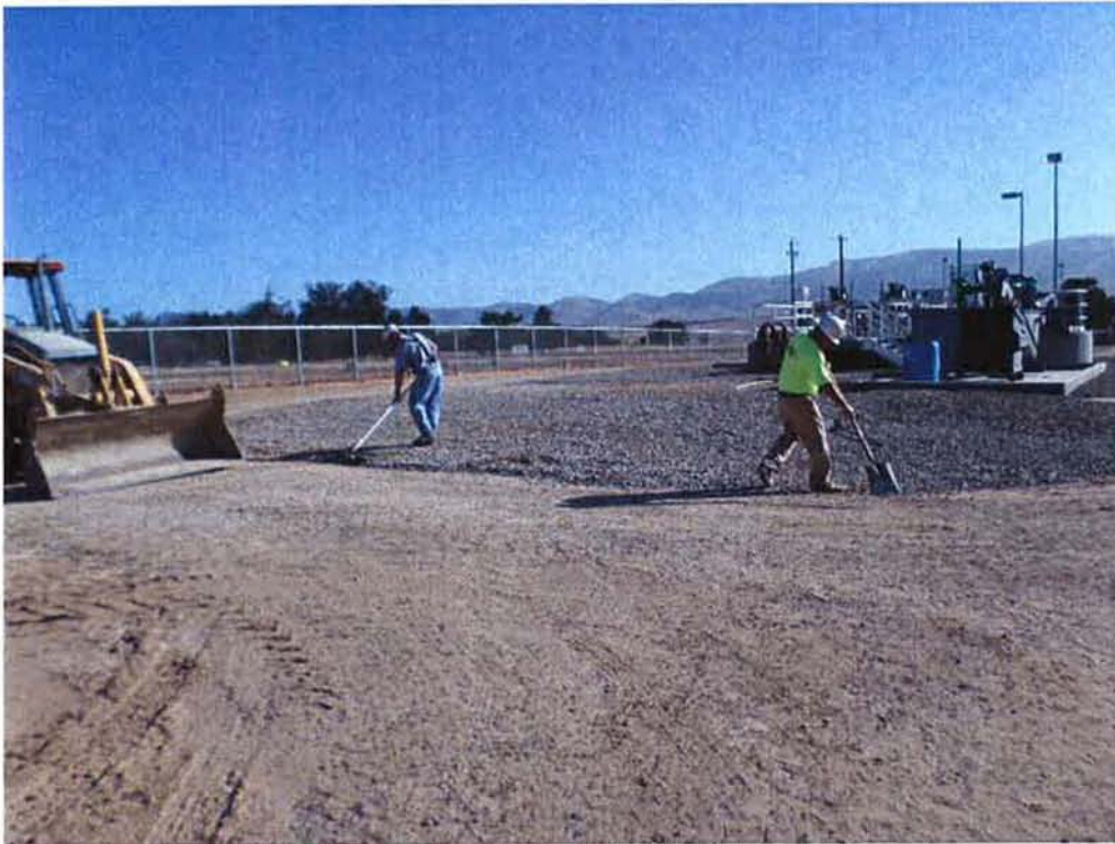
Cushman spreading \frac{3}{4} -inch rock around the Headworks.
