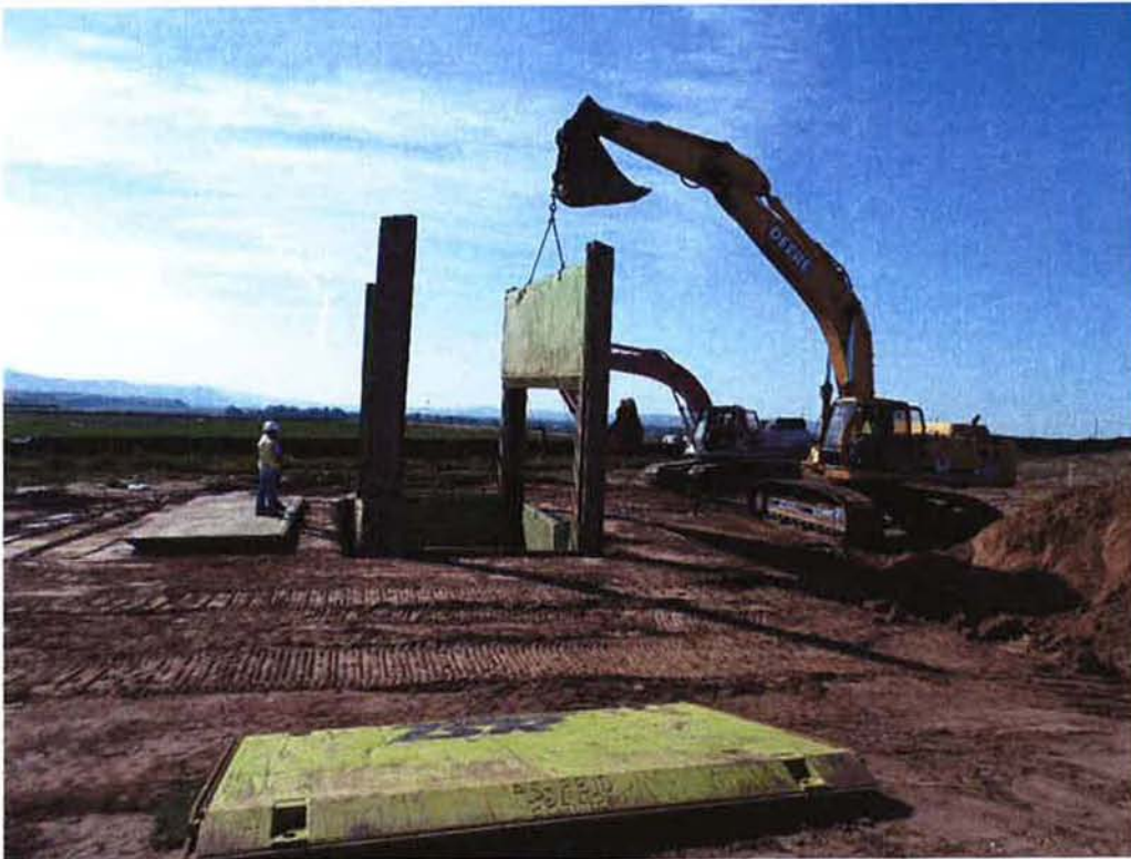
Spiess excavating and installing shoring for pump cans.
