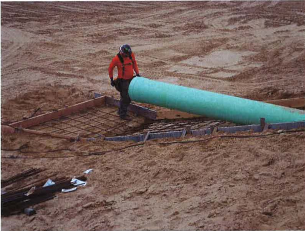
CMC tying reinforcing at concrete discharge pads in Ponds 9 & 10.
