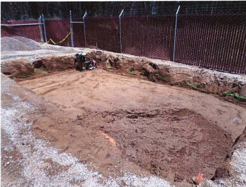
Spies over excavating and compacting for slab under the chemical building.
