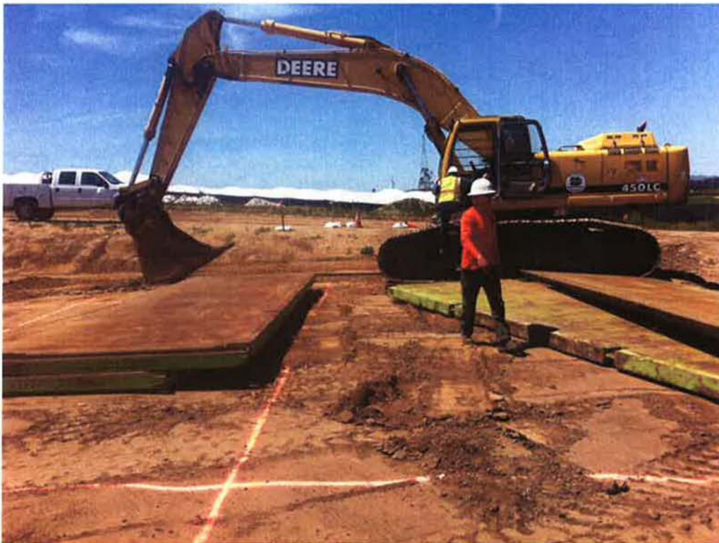
Layout for pump can excavation and shoring staged.
