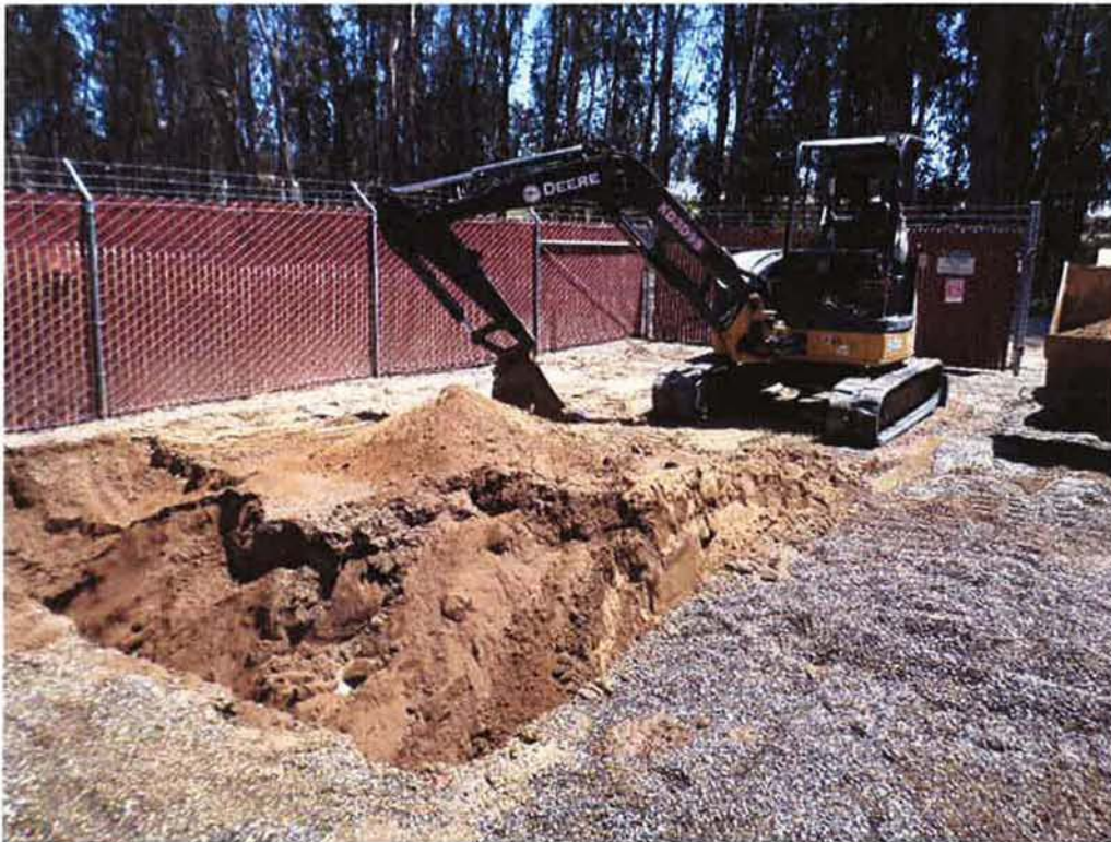
Spiess excavating for slab under the chemical building.
