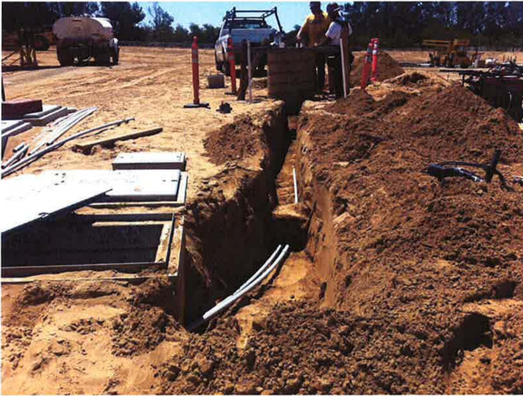
Cushman forming the base for the new SCADA tower.
