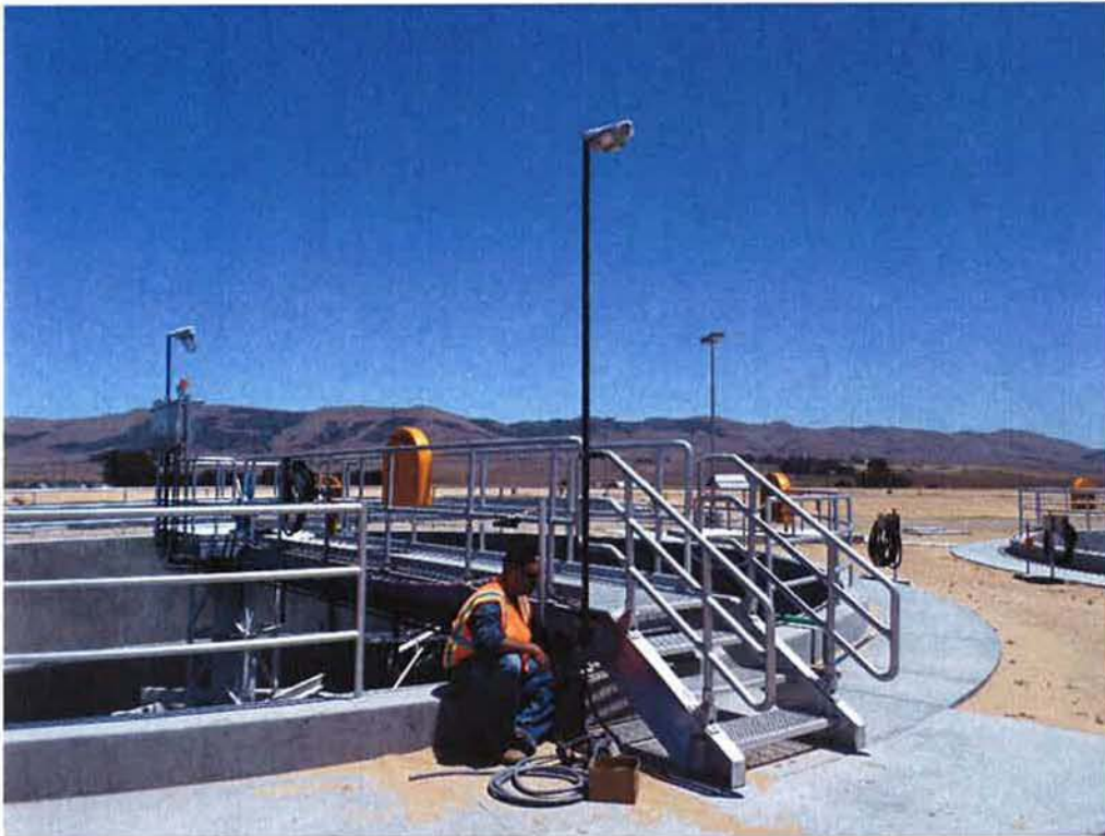
Bergelectric installing lights at clarifier stairs.
