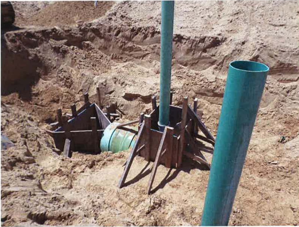
Forming thrust block at cleanout.
