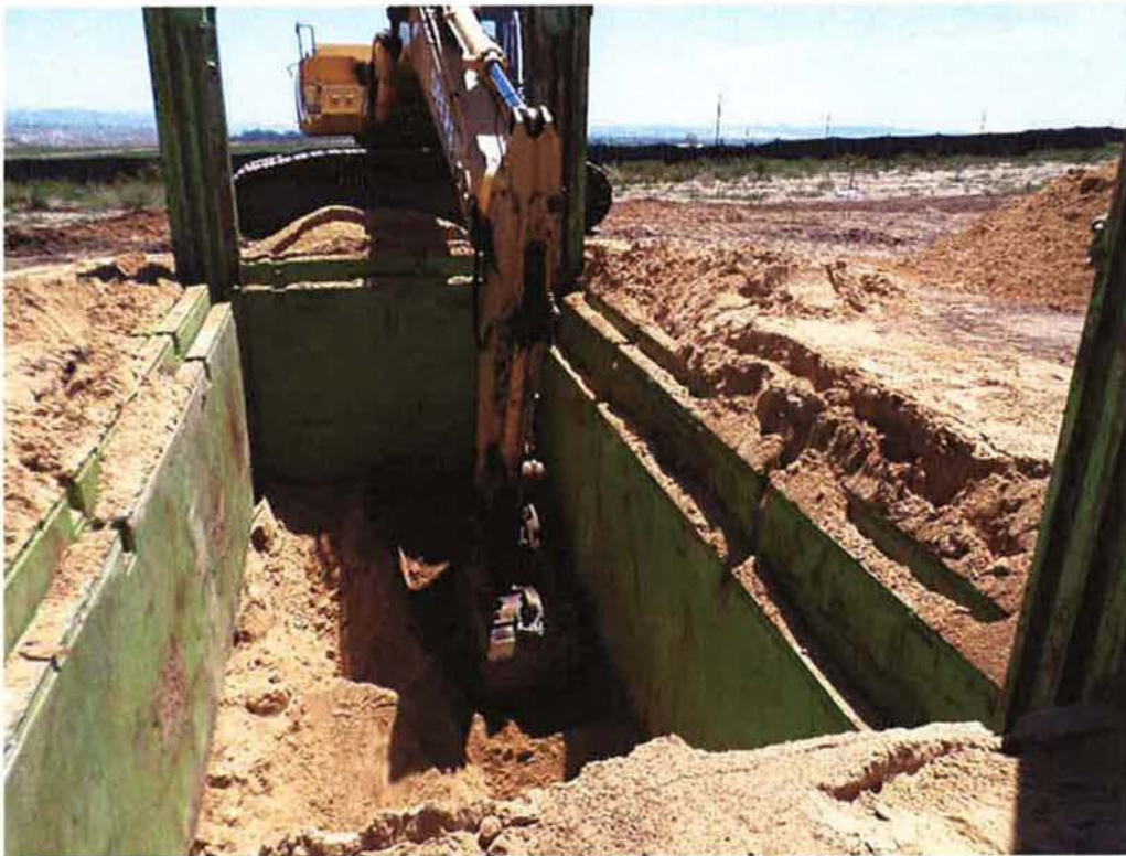
Spiess excavating inside shoring for pump can installation.
