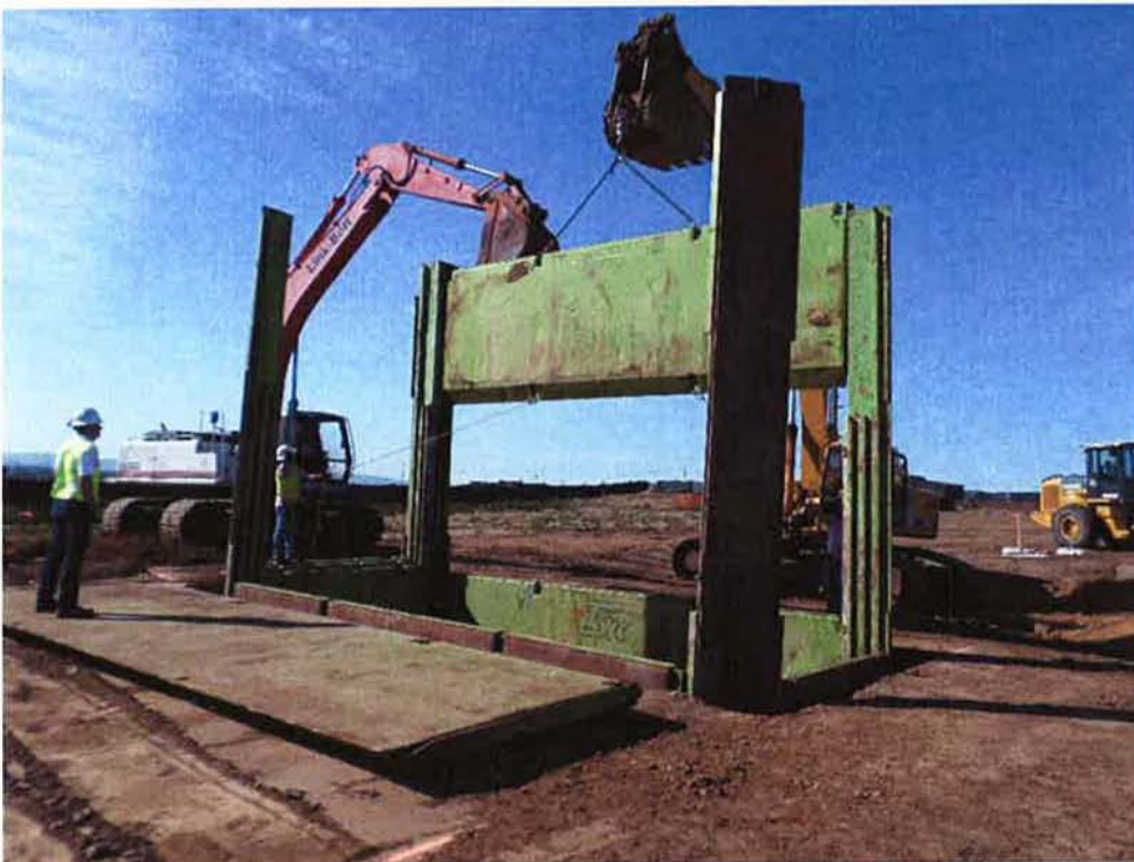
Spiess excavating and installing shoring for pump cans.
