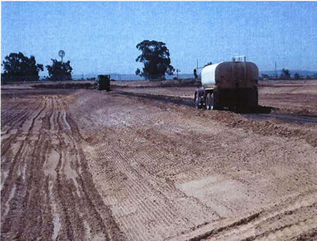
Switzer watering down aggregate base on road between Ponds 9 & 10.
