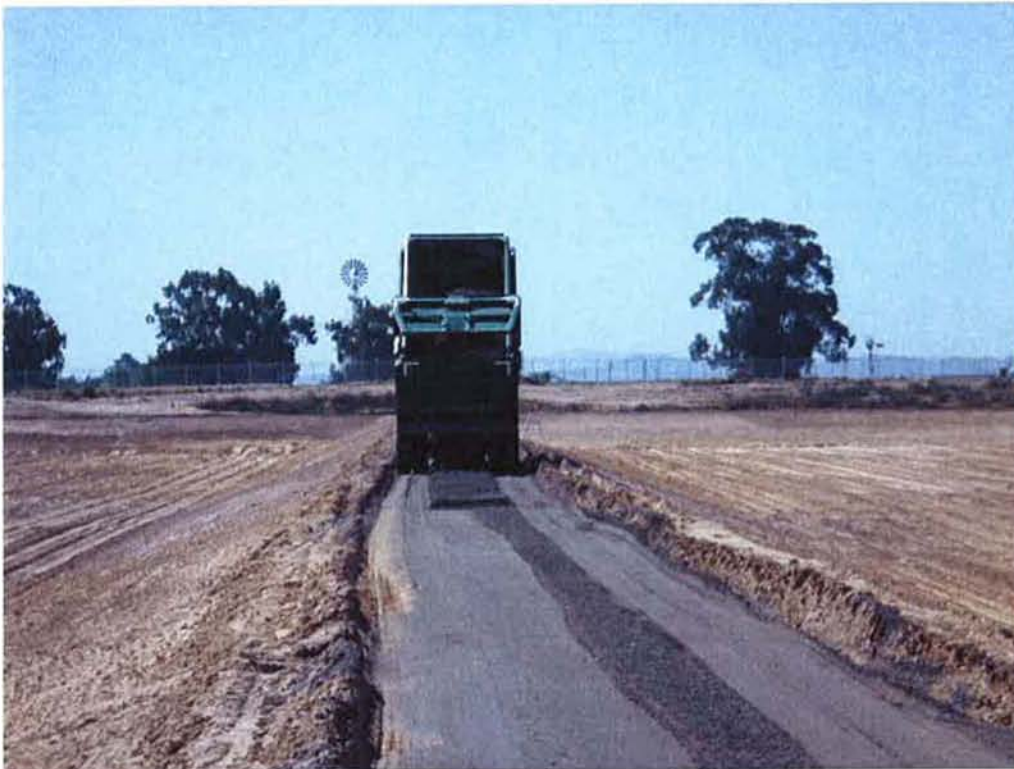
Aggregate base being delivered to road between Ponds 9 & 10.
