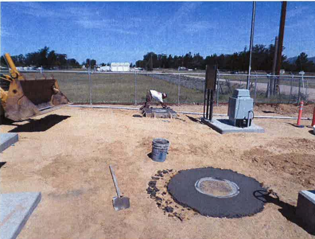
Cushman pouring manhole collars.
