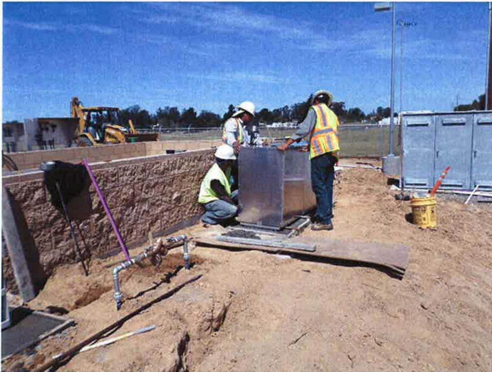
KCI Environmental installing cover over landscaping irrigation manifold.
