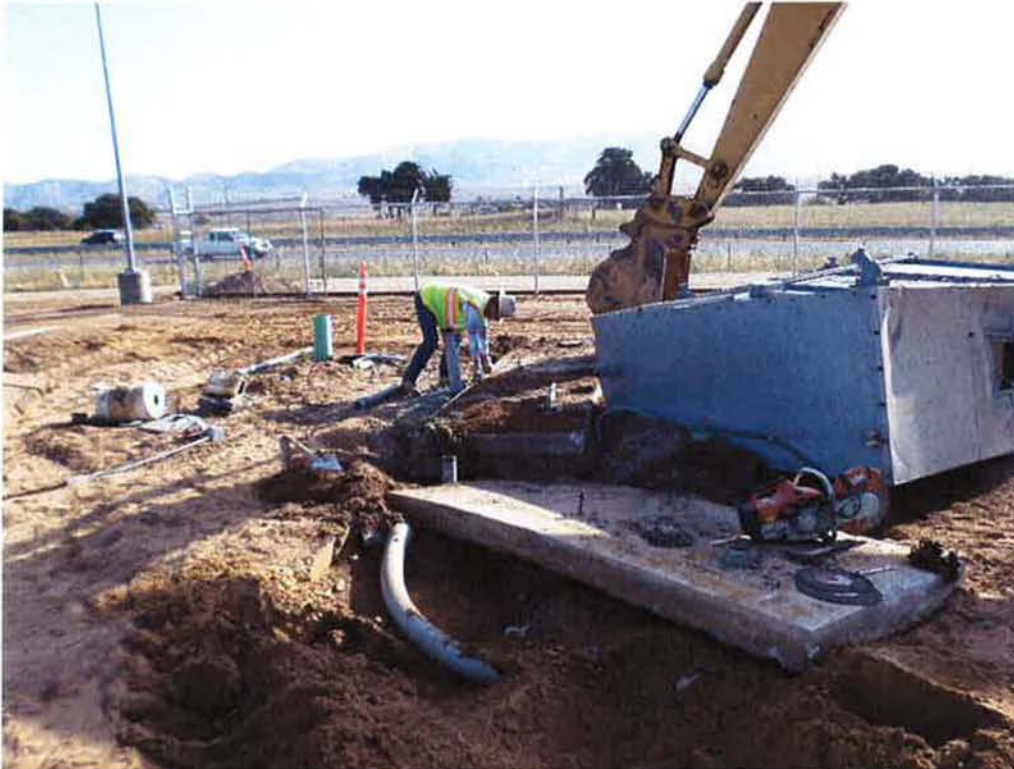
Cushman demolishing existing MCC panel and concrete slab at site entrance.
