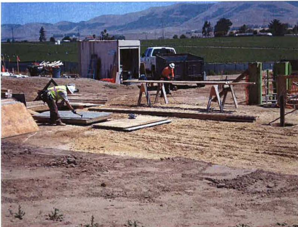
Spiess constructing forms for pump can encasements.
