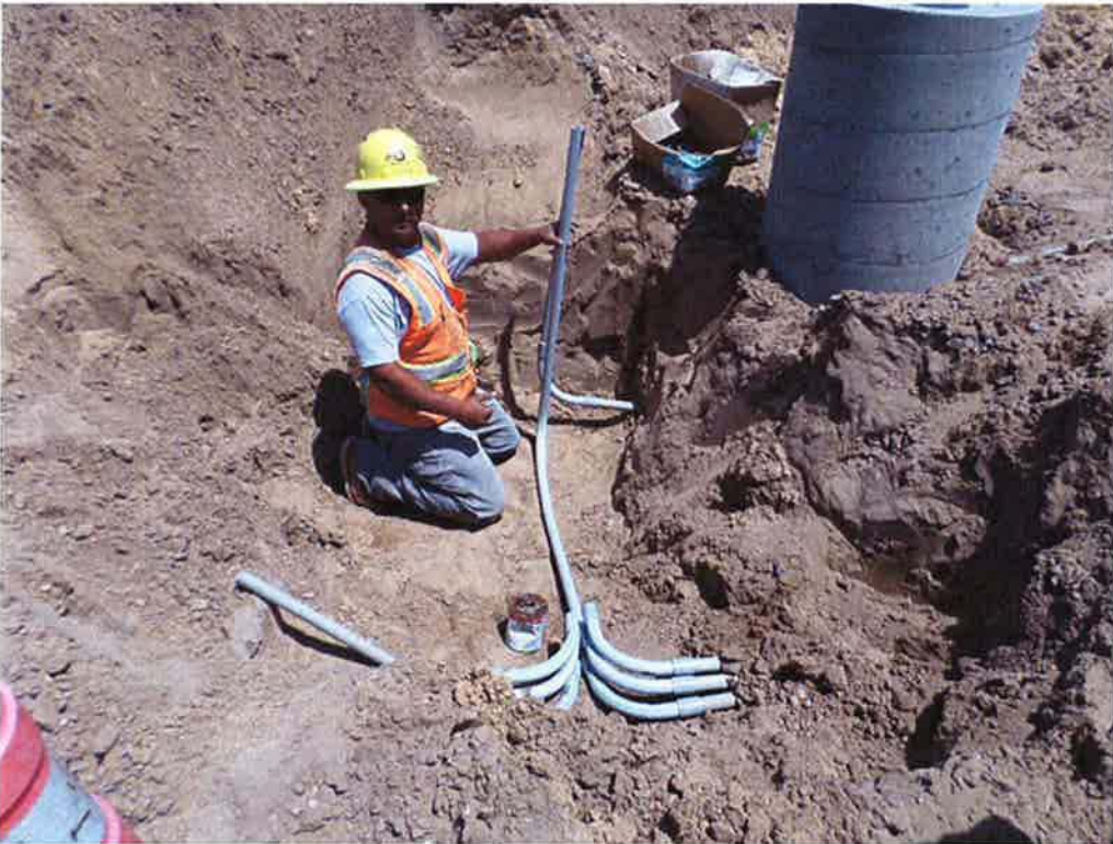
Bergelectric installing conduit to remaining street lights.
