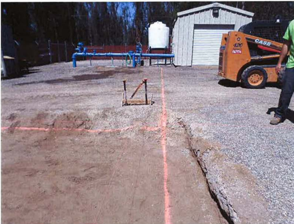
Laying out pipe trenches.
