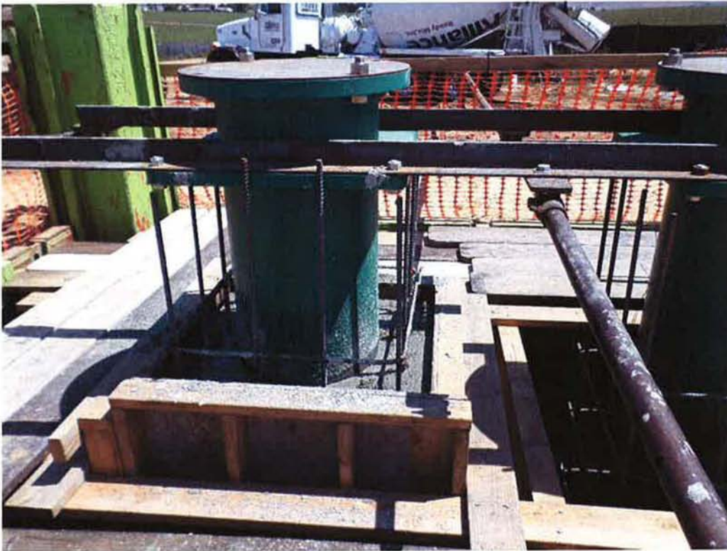
Concrete pour for first two pump can encasements completed.
