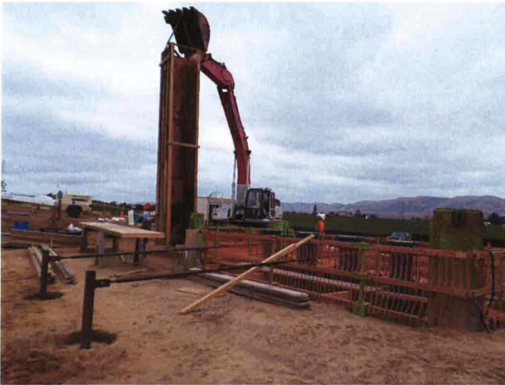
Spiess installing pump can encasement forms.
