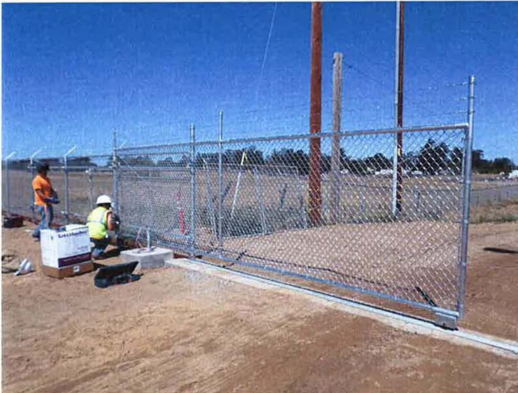
Valley Fencing installing new sliding and automated gate to site entry.
