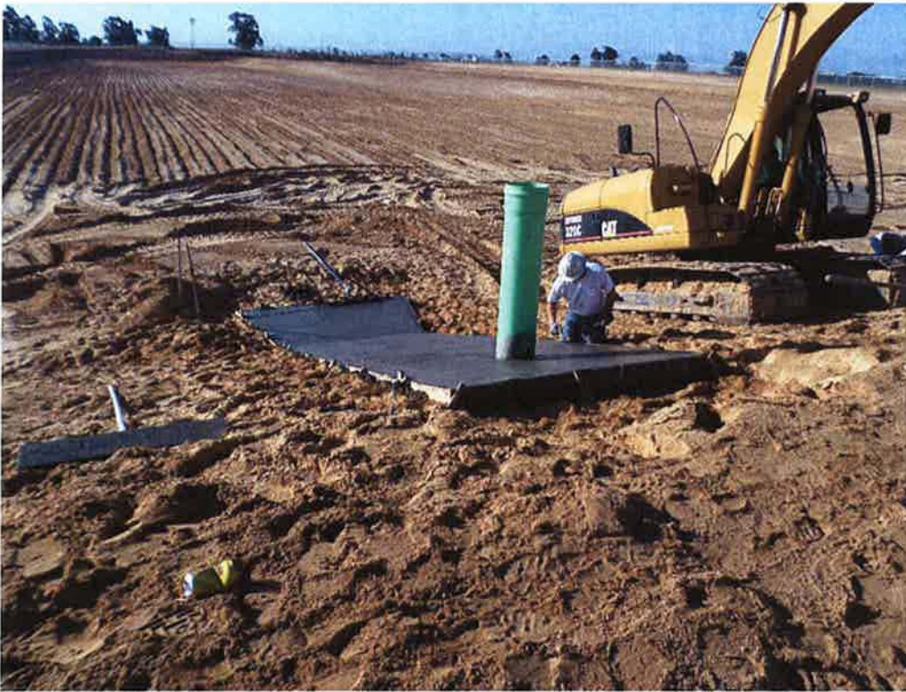
Cushman finishing concrete discharge pads at Ponds 9 & 10.
