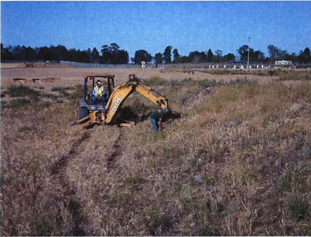
Cushman removing existing barbed wire fencing along DWR easement.
