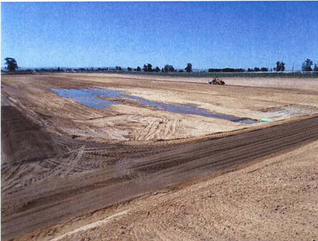
Effluent being discharged into new Pond 10.
