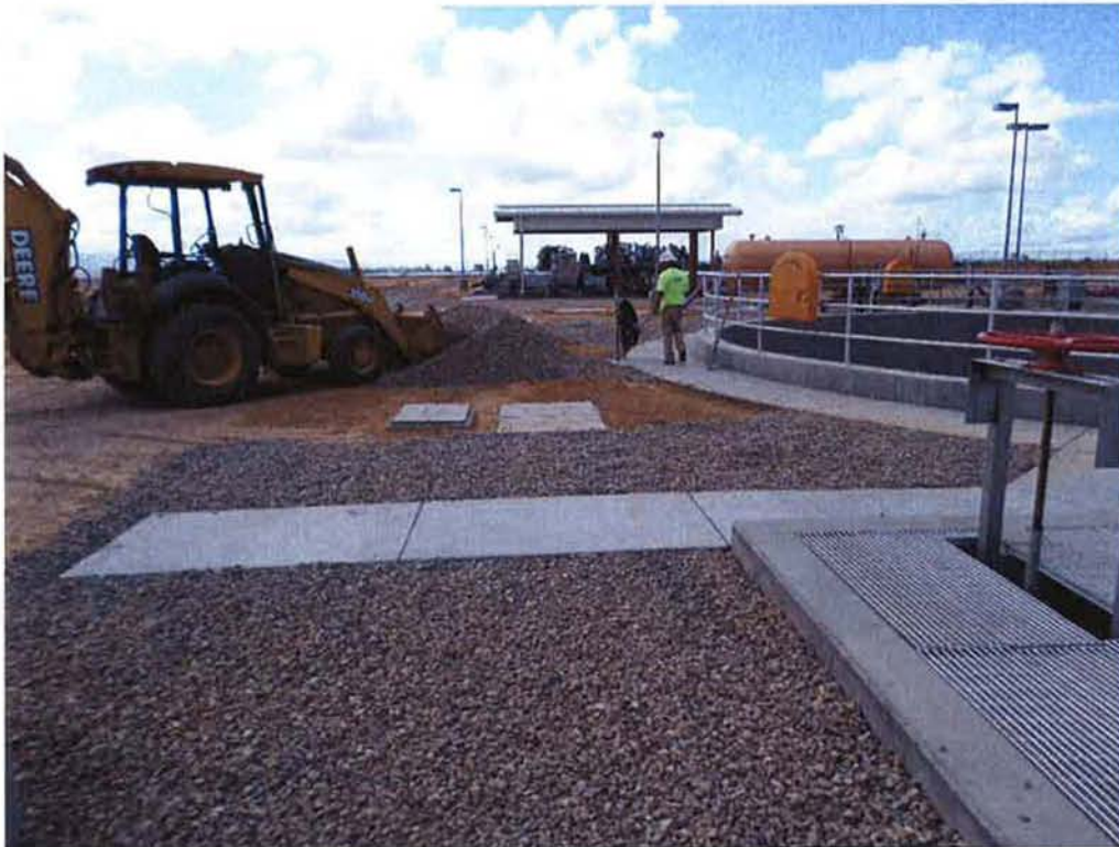
Spreading \frac{3}{4} -inch rock around the clarifiers.
