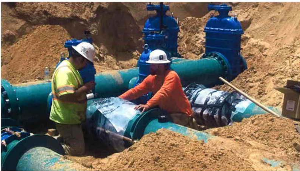
Spiess wrapping joints with wax tape and plastic on suction pipe.
