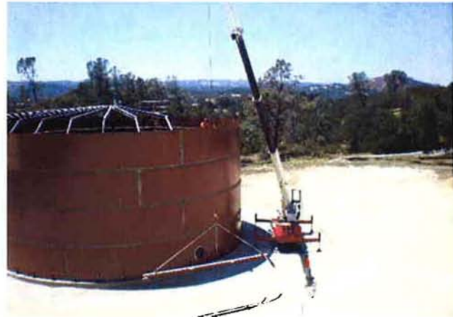
Figure ES-4. Nacimiento Water Project, Rocky Canyon Water Storage Tank Construction (2008)
