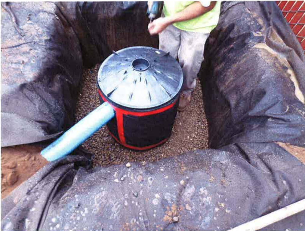
Spiess installing the drywell at Sundale.
