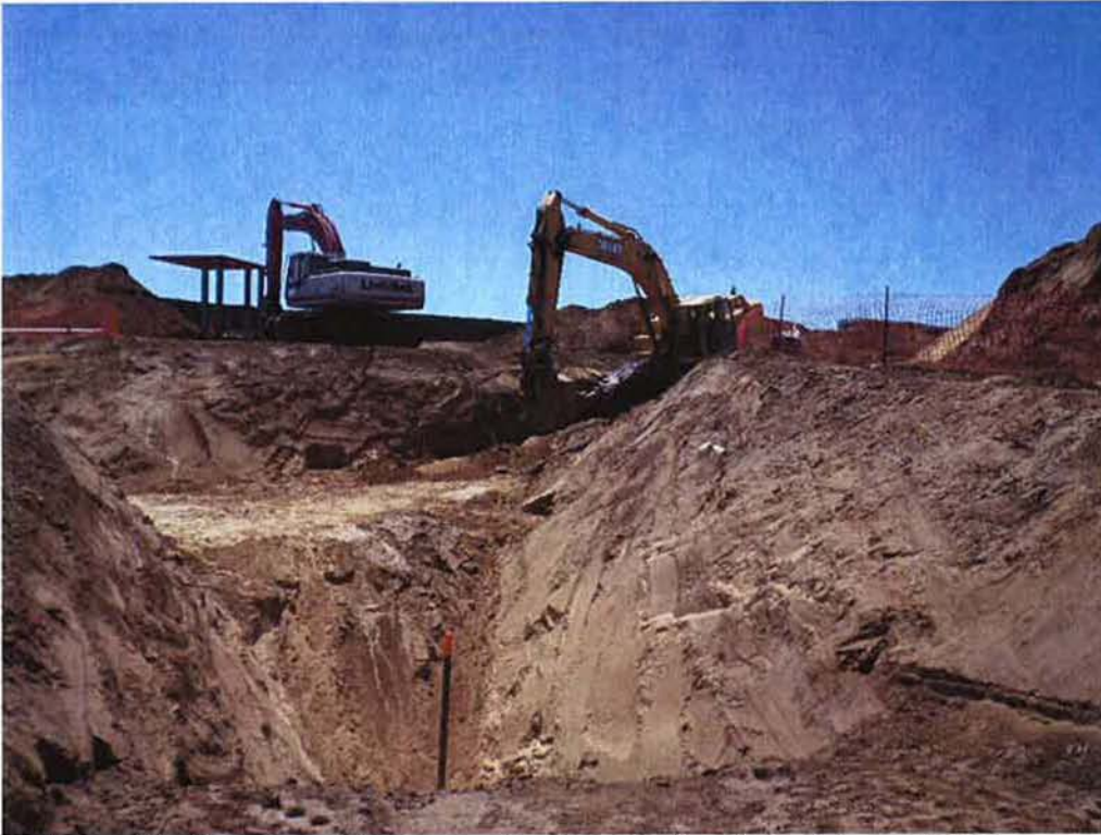
Spiess widening ramp into excavation for pipeline from future HDPE connection.
