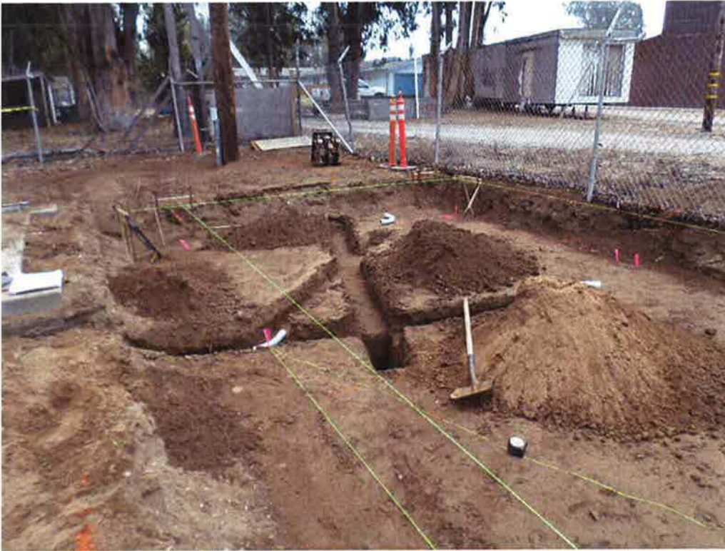
Trenching for underslab piping.
