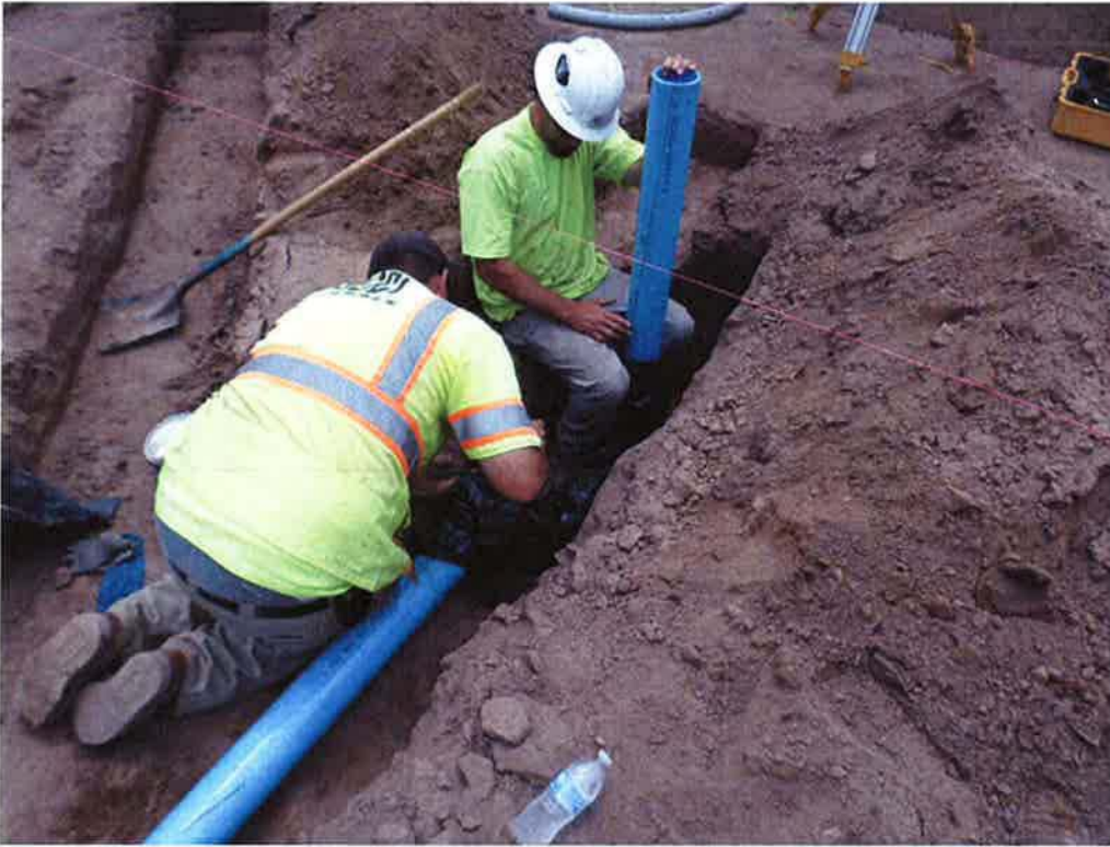
Spiess installing 4-inch drain line.
