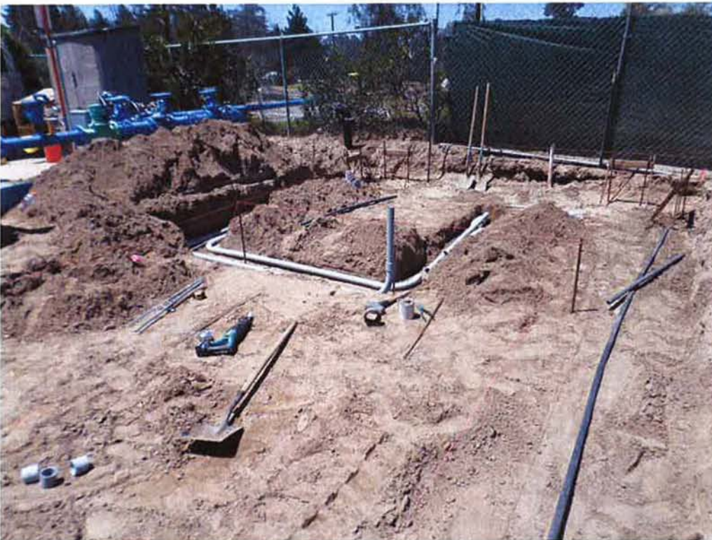
Spieß installing underslab piping.
