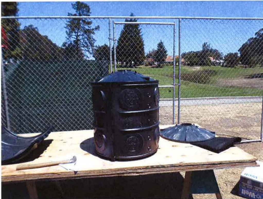
Assembling the drywell.
