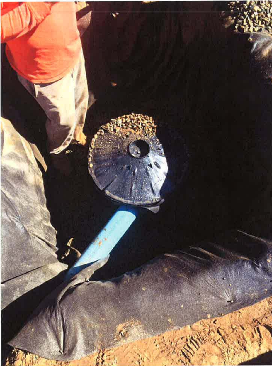
Spiess installing the drywell.
