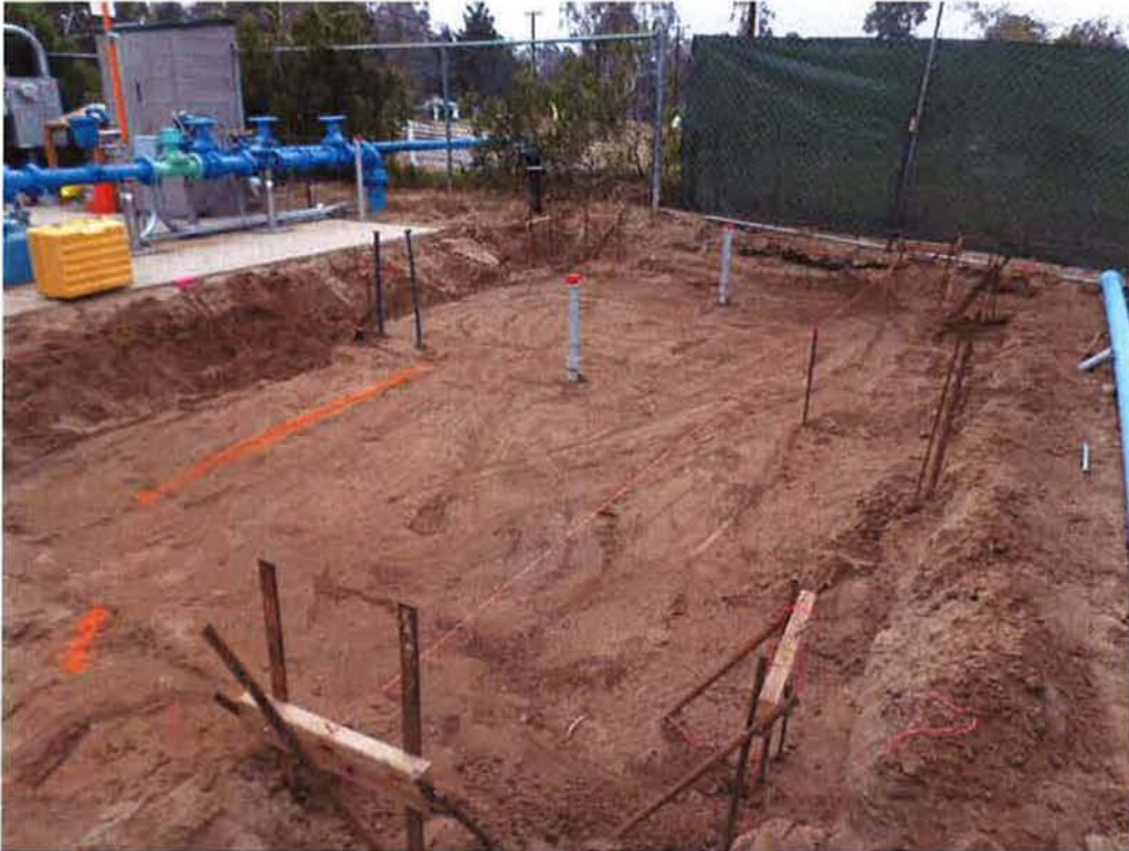
Spiess laying out the foundation and installing underslab conduit and waterlines.
