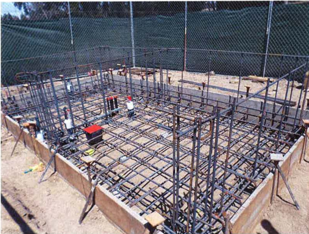
Reinforcing installed for chemical building slab.
