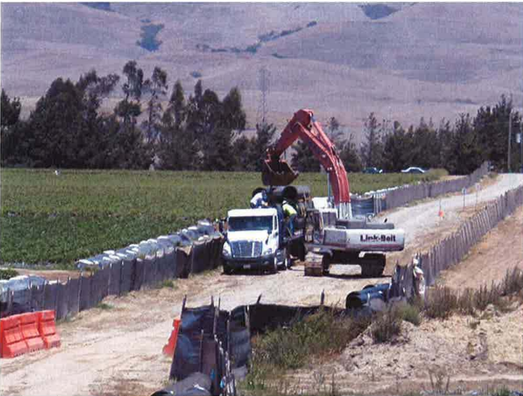
Spiess staging 24-inch DIP along access road for future installation.
