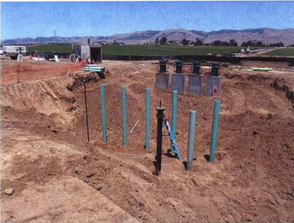
Spiess installing valve can risers on inlet manifold.
