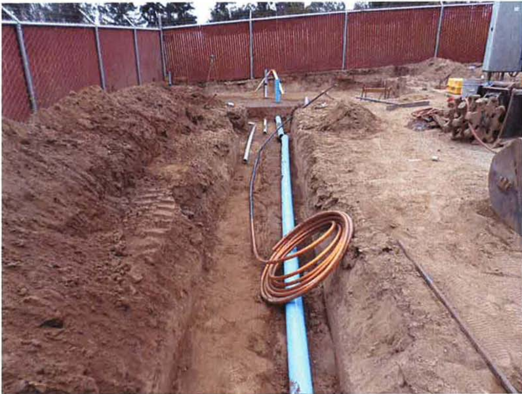
Installing site piping.
