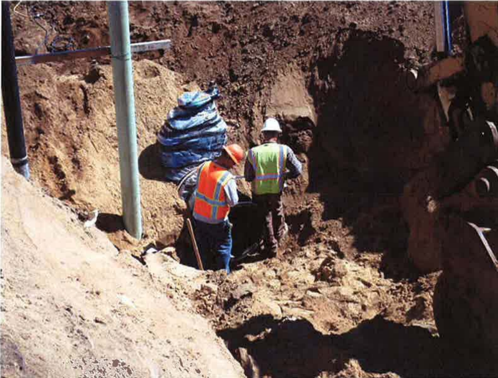
Spieß installing flange adapter on 24-inch DIP.
