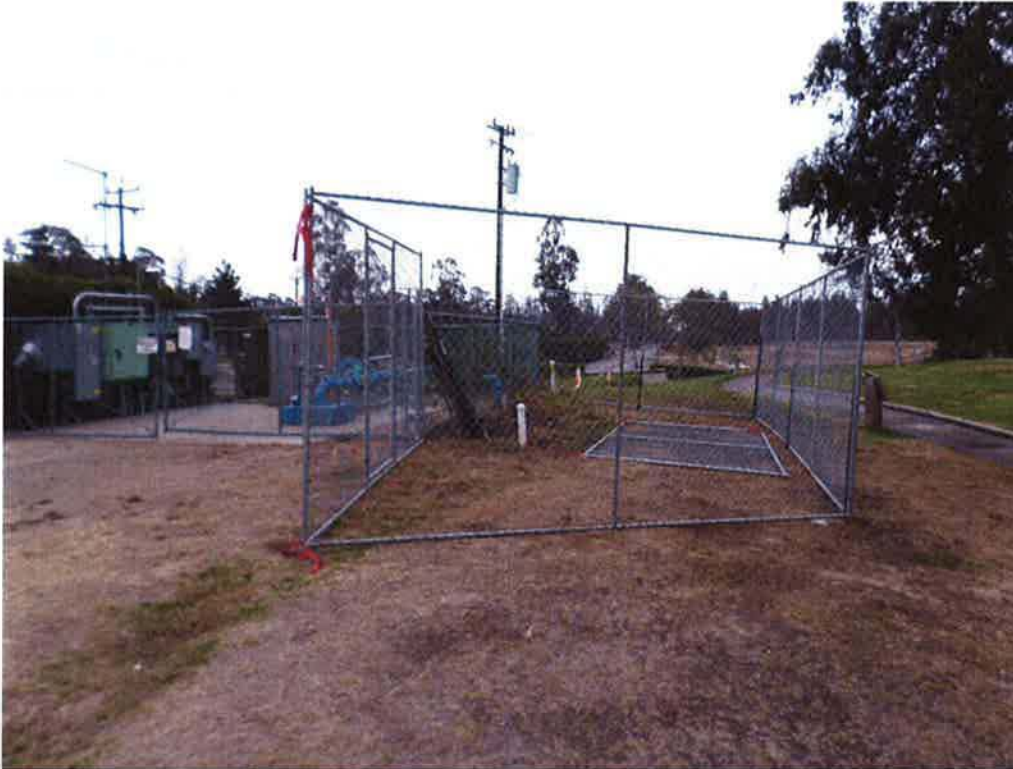
Installing temporary fencing to expand site.
