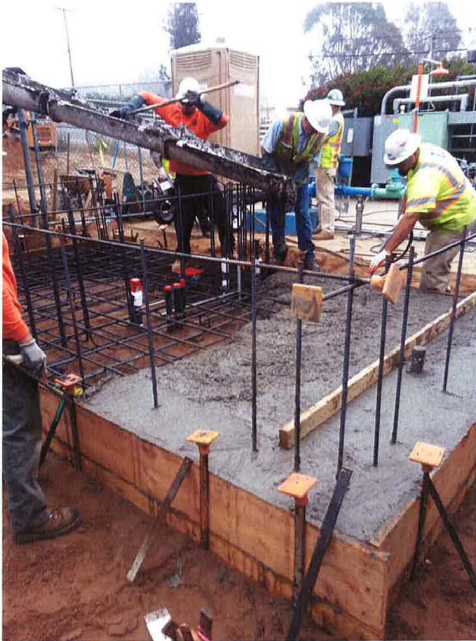
Spiess pouring the chemical building slab.
