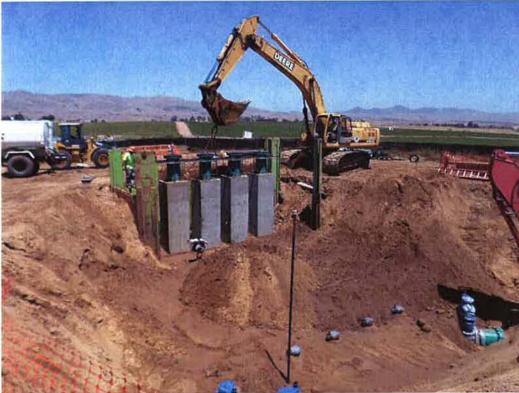
Spiess removing shoring plates at pump cans.
