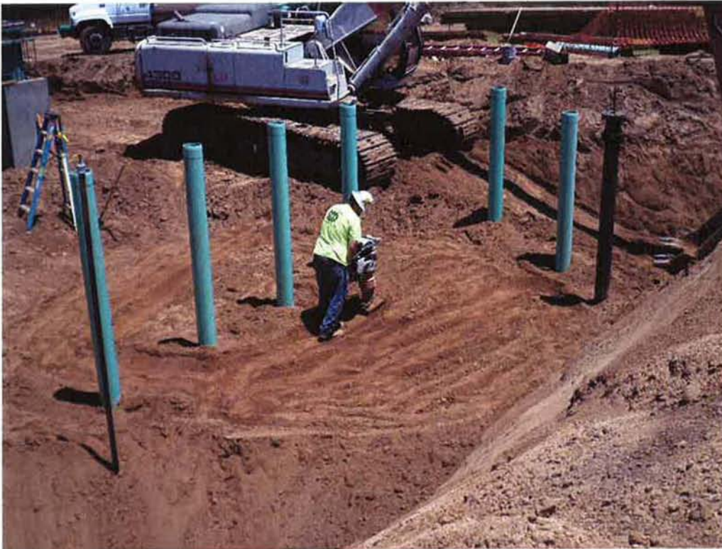
Spieess compacting around the valve can risers.
