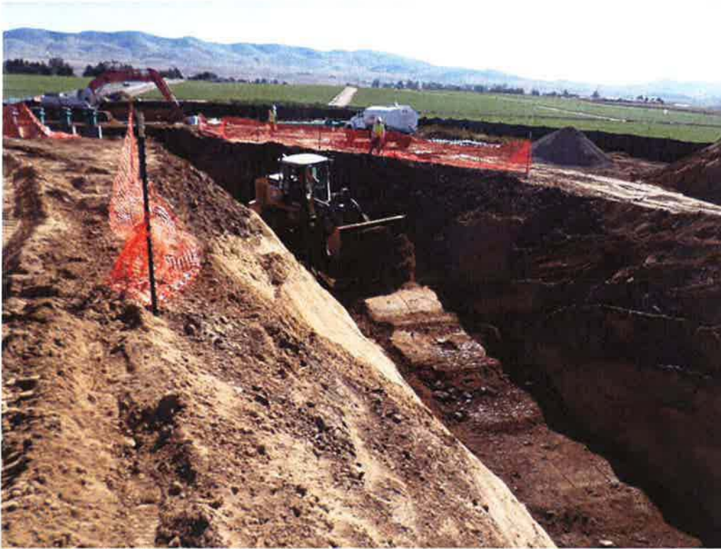
Spiess backfilling over 24-inch DIP.
