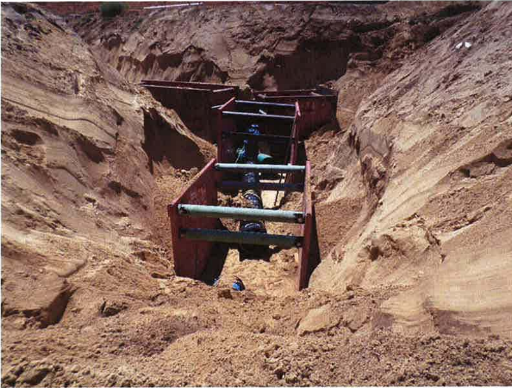
Spieß installing the 24-inch DIP around the pig launcher.
