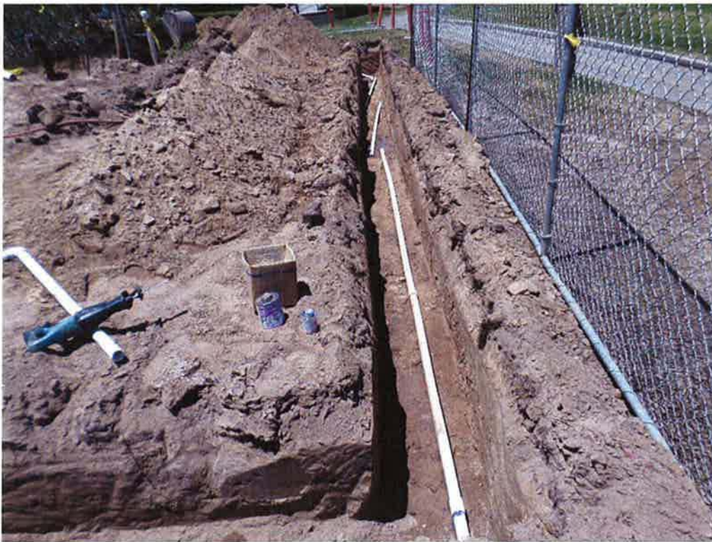
Spieß relocating 1-1/2-inch irrigation line.
