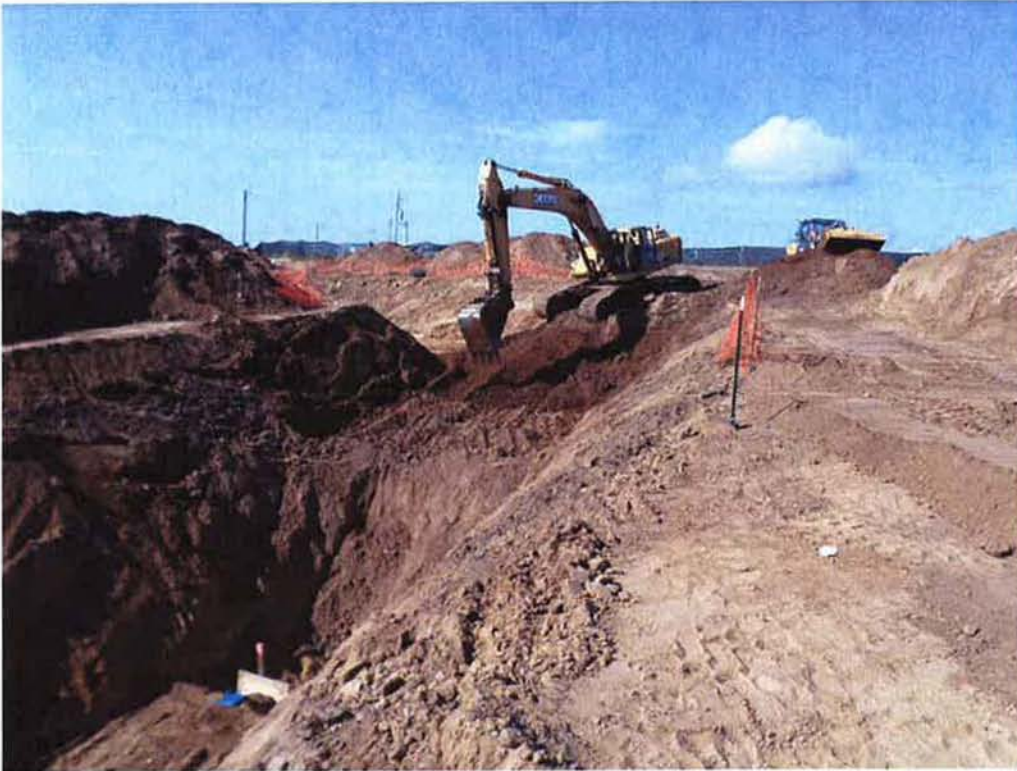
Spiess excavating for 24-inch DIP between pump station and BP #1 connection.
