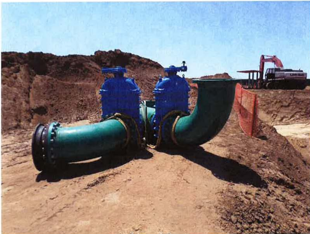
Pig outlet assembled and ready to set into place.
