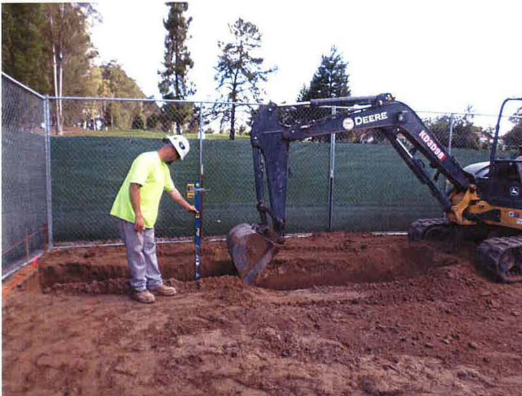
Spiess over excavating for the chemical building slab.
