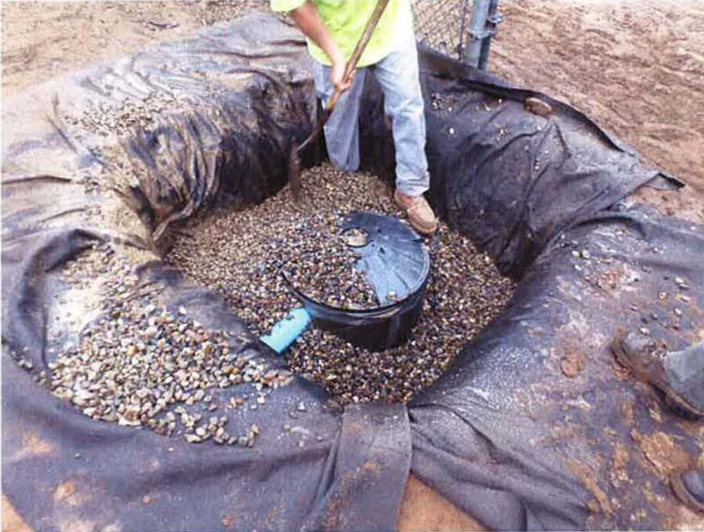
Spiess installing drywell at Via Concha.
