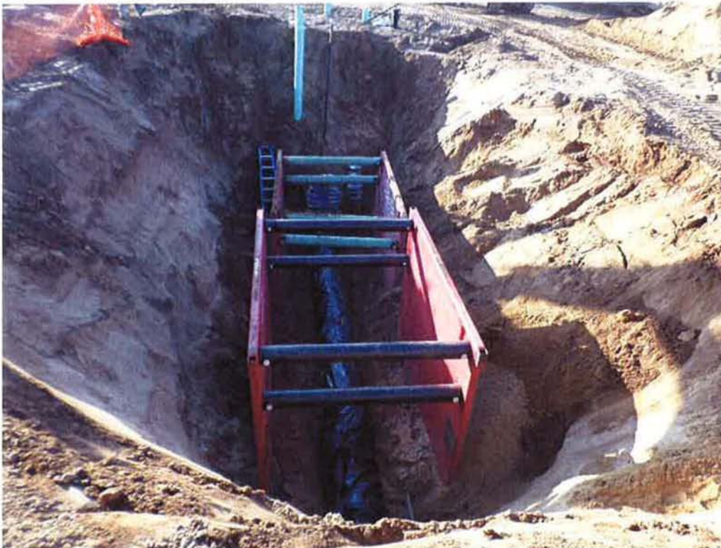
Spiess installing pipe extension to future tank outlet piping.
