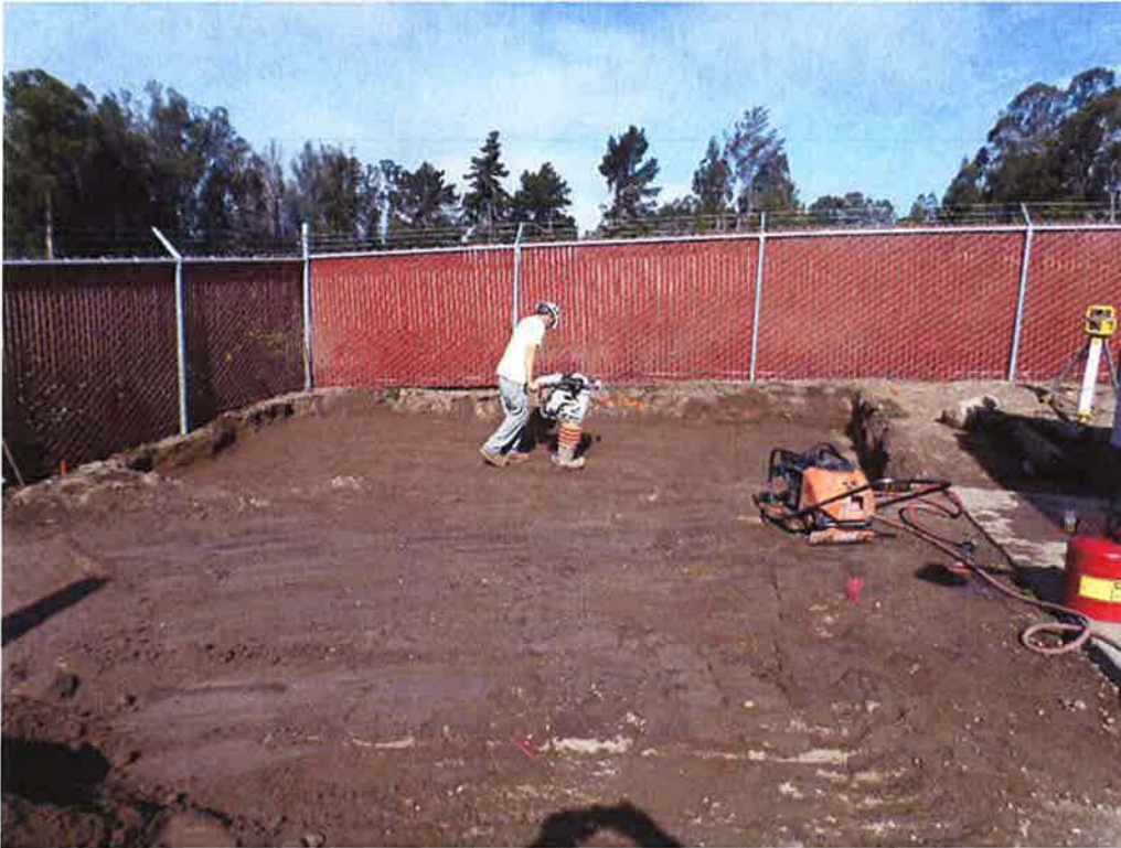
Spiess excavating and compacting subgrade for chemical building slab.
