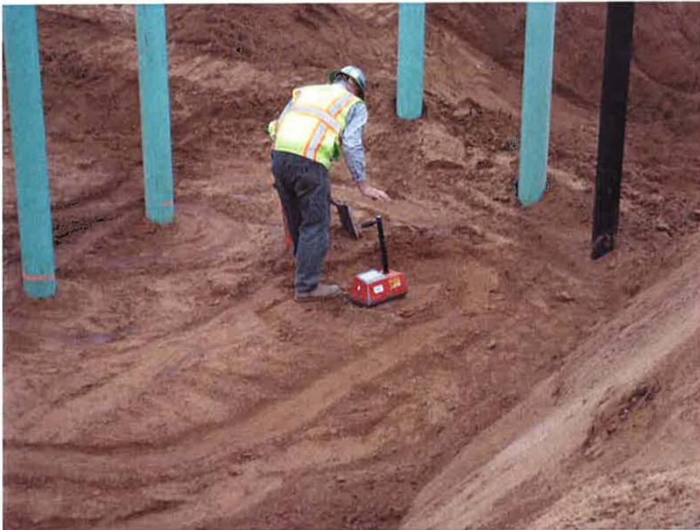
Fugro testing compaction.
