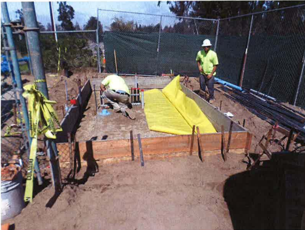
Spiess installing underslab vapor barrier.
