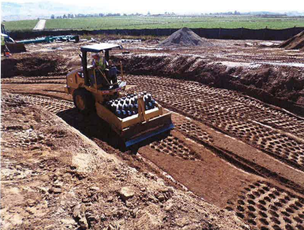
Spiess compacting over 24-inch DIP.
