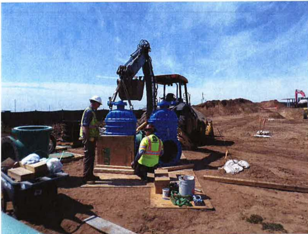
Spieß bolting up 24-inch valves.
