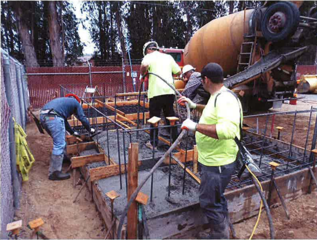
Spiess placing concrete for chemical building slab.
