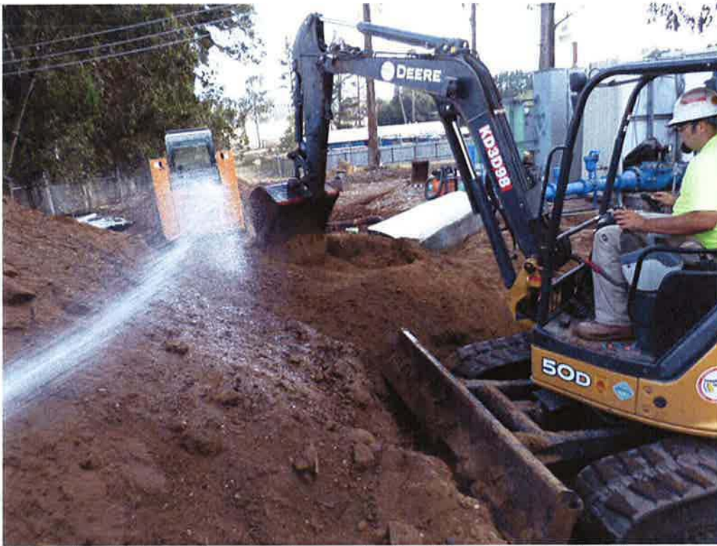
Spies backfilling and compacting under the future chemical building slab.
