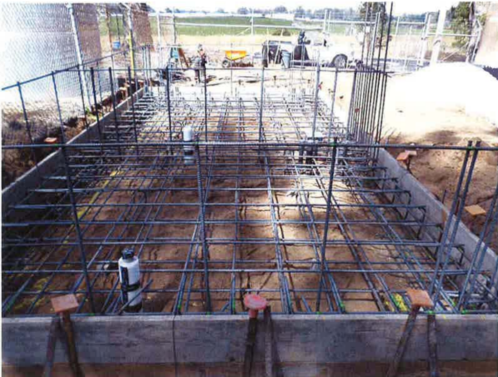
Chemical pad reinforcing installed by Vista Steel.
