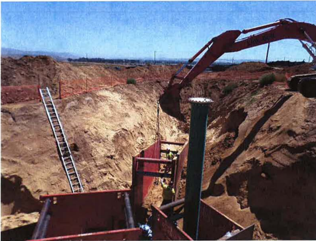
Spiess removing shoring around the pig launch and riser.
