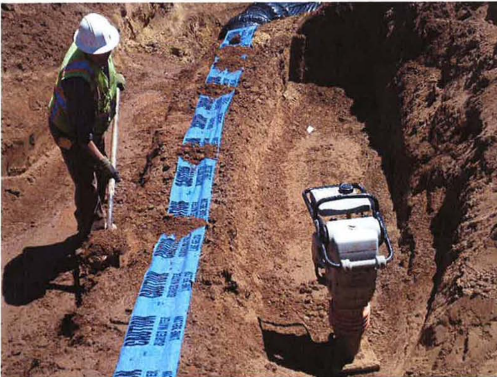
Spiess installing marker tape over 24-inch DIP during backfill.
