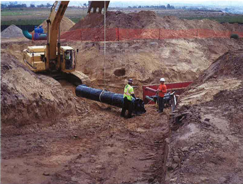
Spiess installing the 24-inch DIP.
