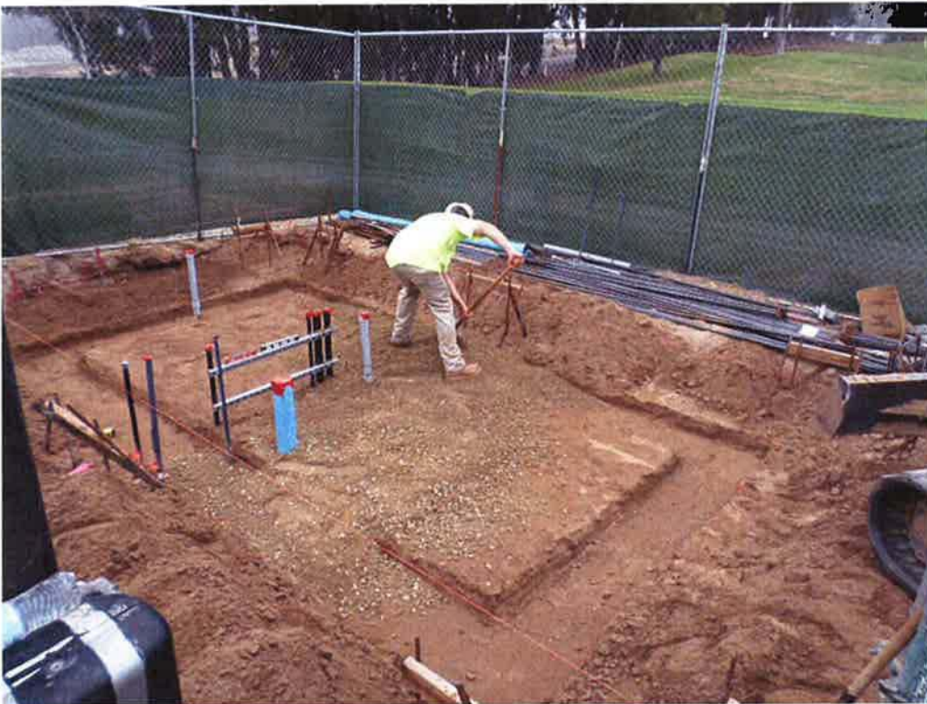
Spiess preparing the foundation base for the chemical building slab.
