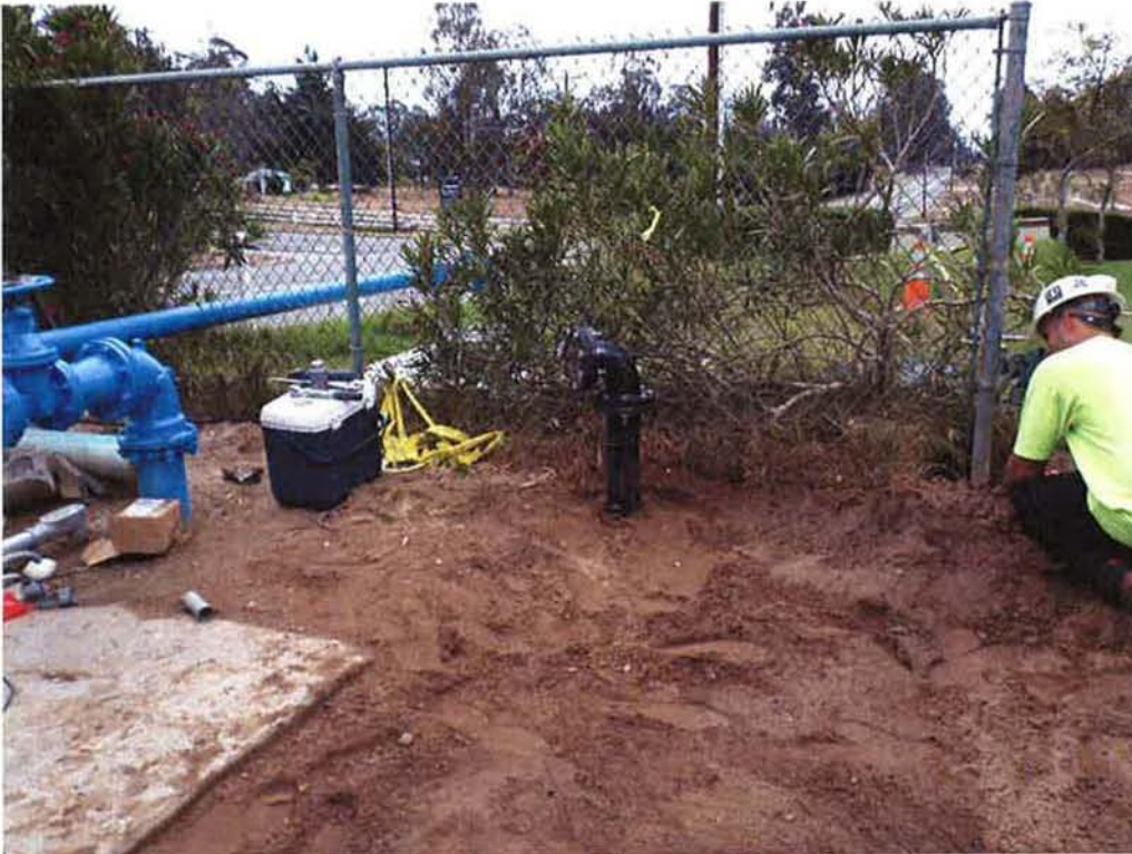
Relocated 4-inch riser.
