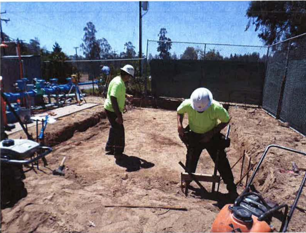
Spieß laying out the chemical building slab.
