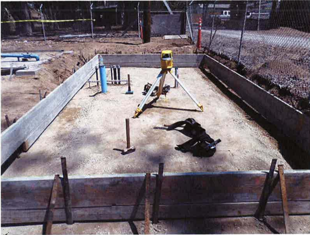
Forming the chemical building slab foundation.
