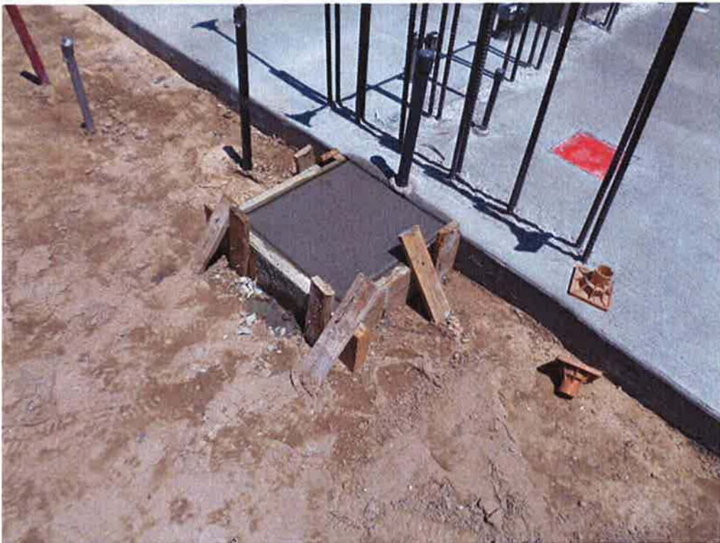
Eyewash station pad installed.
