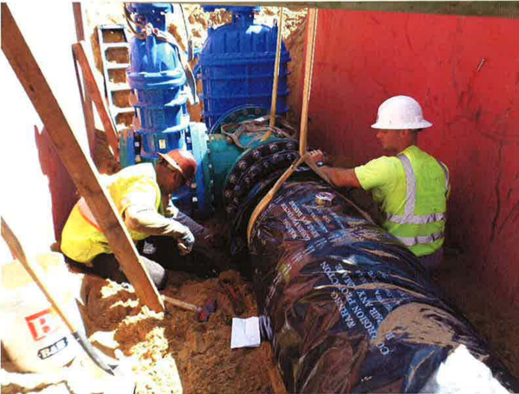
Spieß connection the 24-inch DIP to the "tee".
