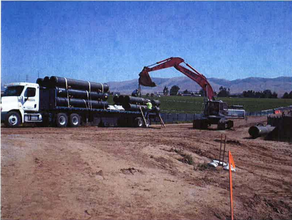
Spiess taking delivery of 24-inch DIP.
