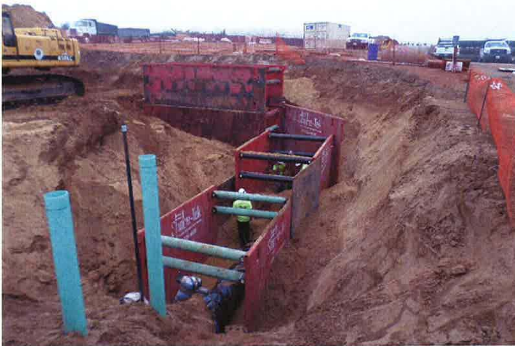
Spiess installing pipe extension to future tank outlet piping.
