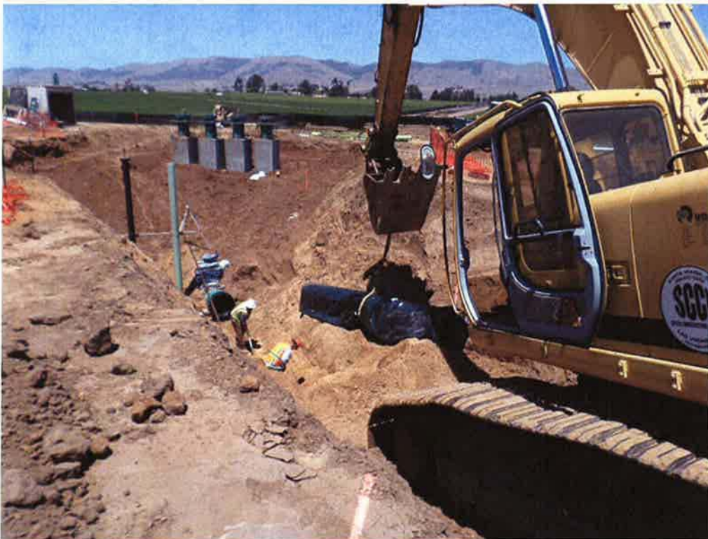
Spieß installing 24-inch DIP from pump station inlet manifold toward the BP #1 connection.
