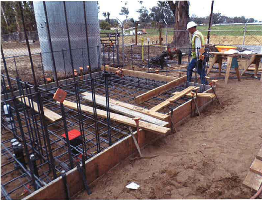
Spiess forming equipment pads on top of chemical building slab.
