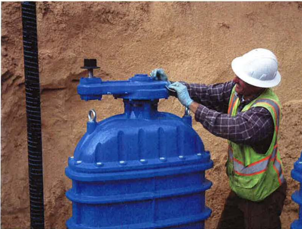
Spiess abrading valve in preparation for coating touch-up before backfill.
