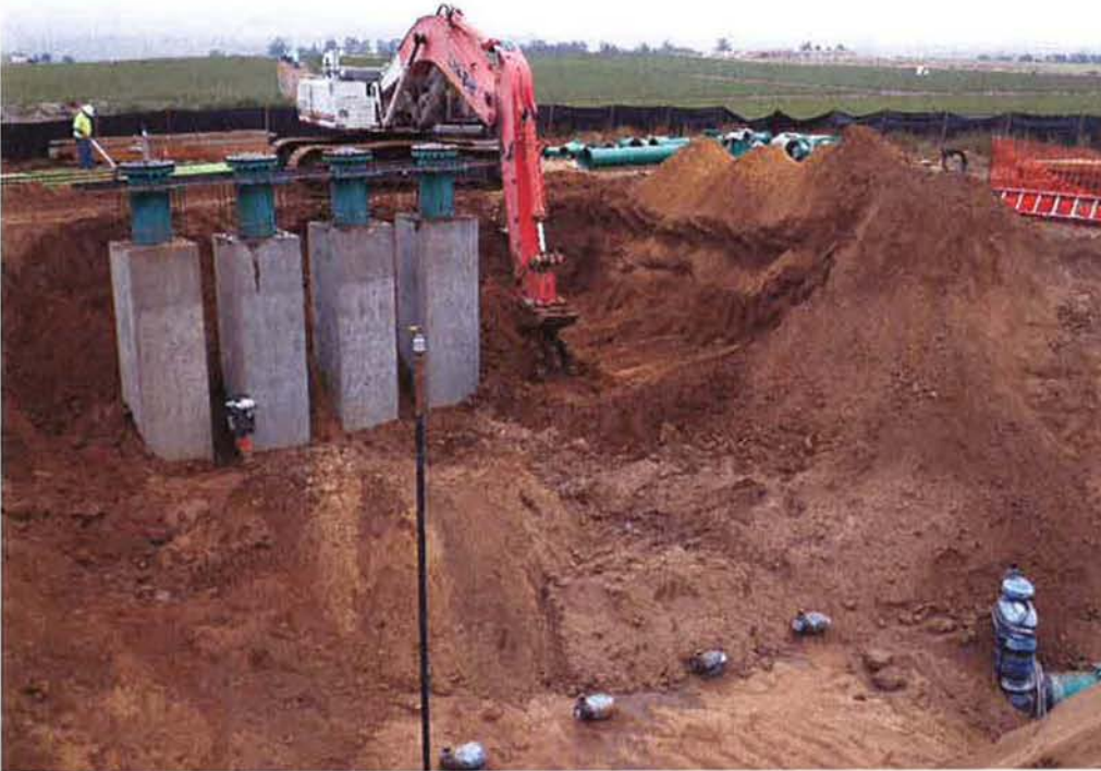
Spiess continuing backfill around the pump cans.
