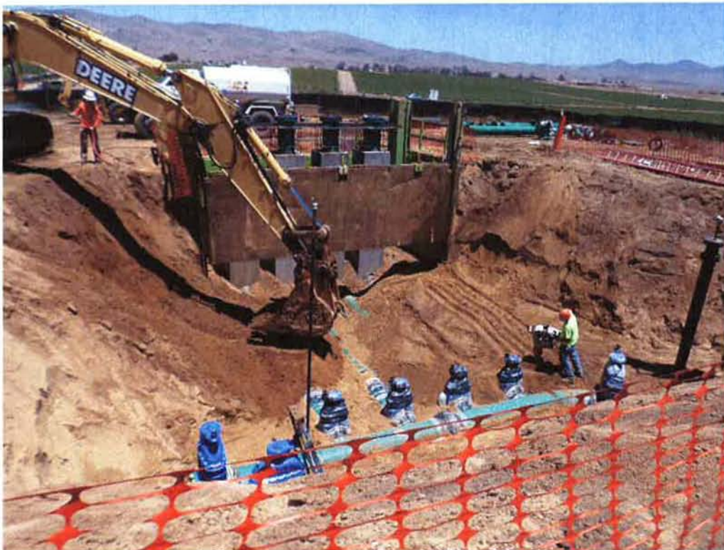
Spiess continuing backfill and compaction over inlet piping.
