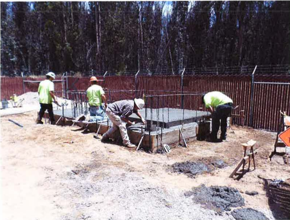
Spiess finishing concrete at chemical building slab.
