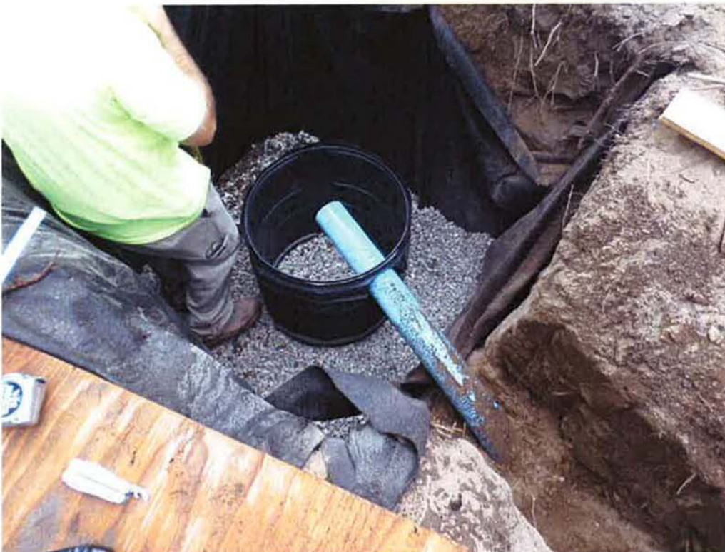
Spiess installing drywell.
