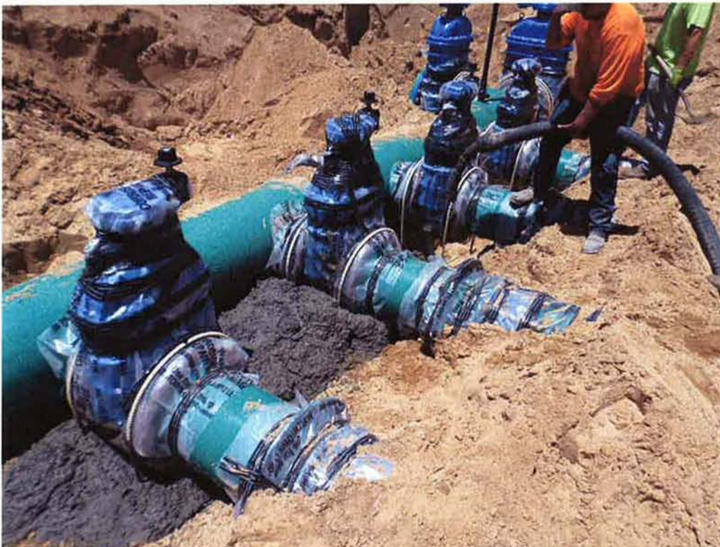
Pouring concrete valve anchors on inlet piping.
