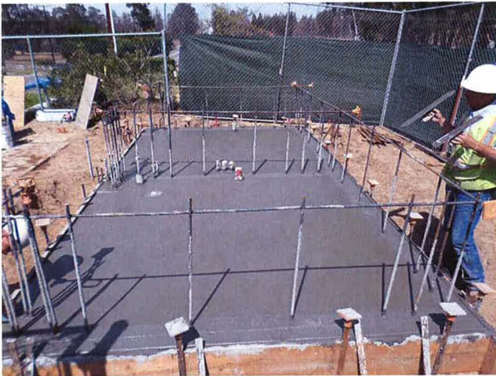
Spieß finishing the chemical building slab.
