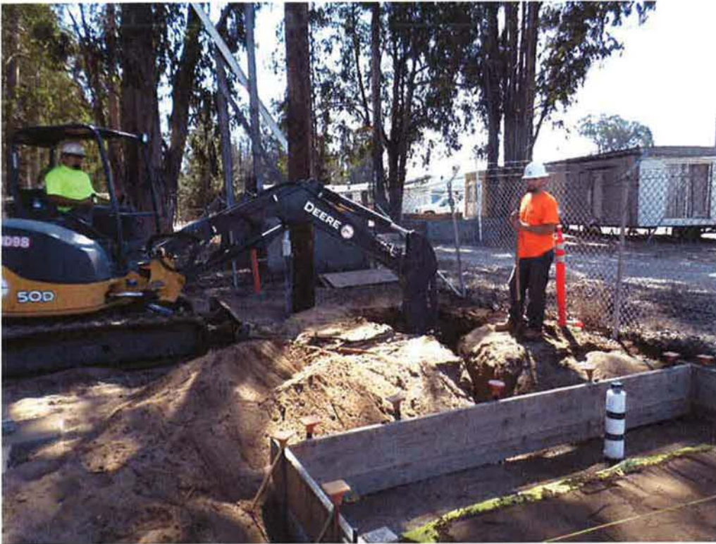
Spiess excavating for drywell.
