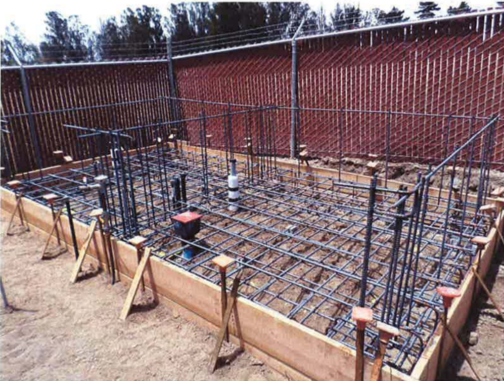
Spiess subcontractor Vista Steel installing reinforcing for chemical building slab.
