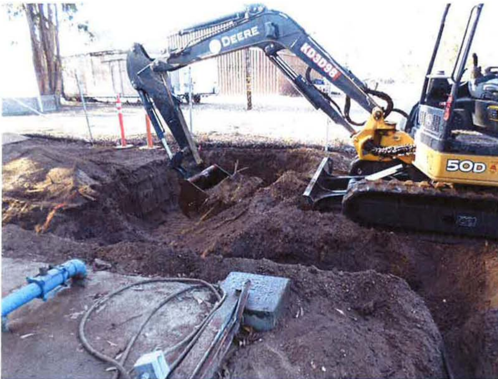
Spiess over excavating native material under the future chemical building slab.
