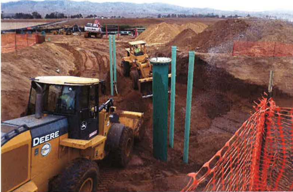
Spiess backfilling around installed valve can risers.
