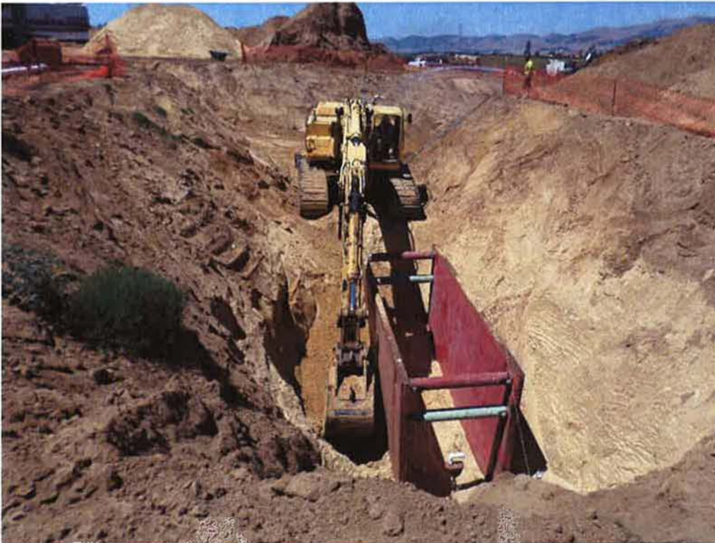
Spiess installing shoring at future connection point to HDPE pipeline.
