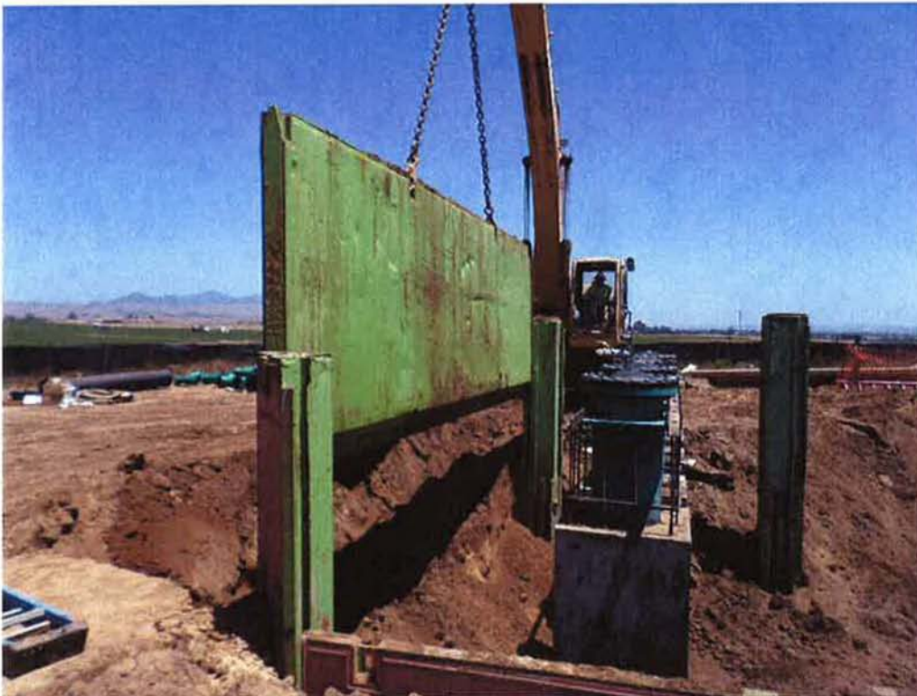
Removing shoring from around the pump cans.
