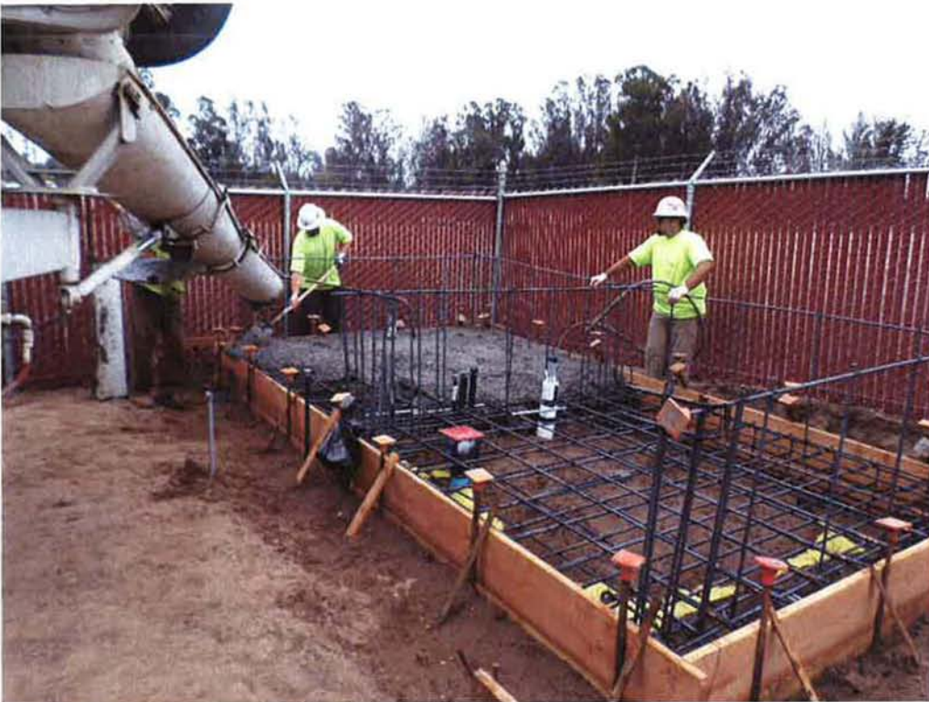
Spiess pouring chemical building slab.
