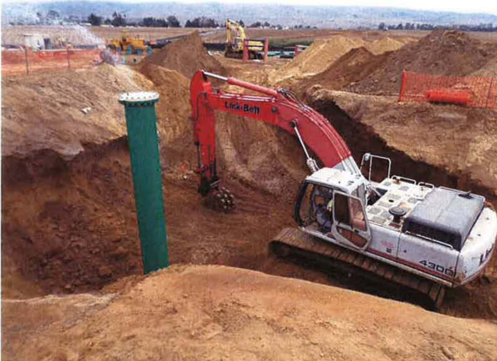
Spiess backfilling and compacting the 24-inch DIP pipe.
