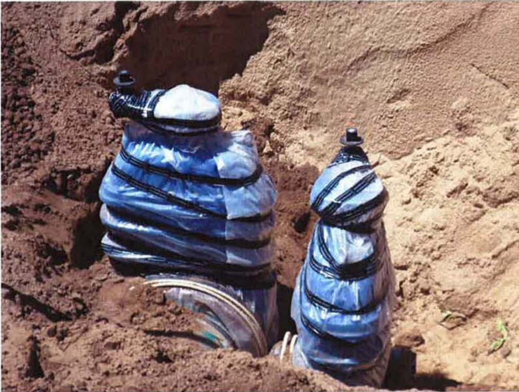
Spiess wrapping valves with plastic before backfilling.
