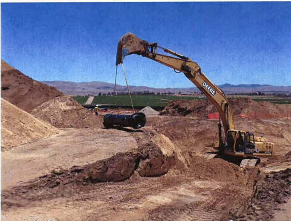
Spiess installing 24-inch DIP.
