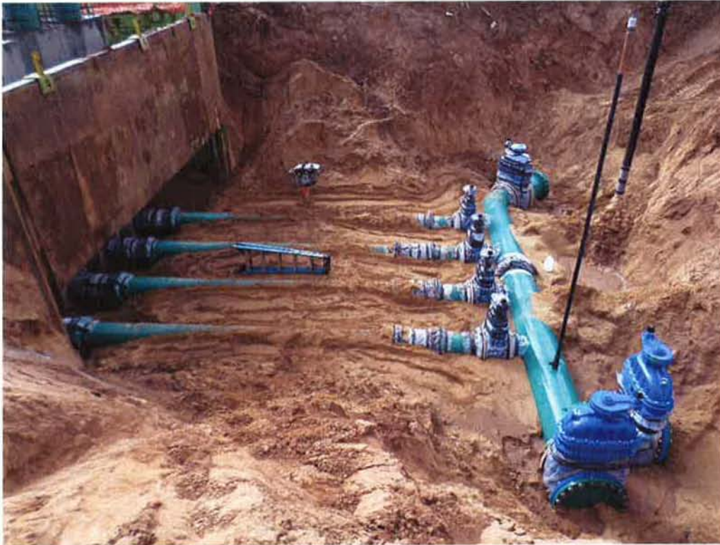
Spiess compacting around inlet piping and manifold during backfill.
