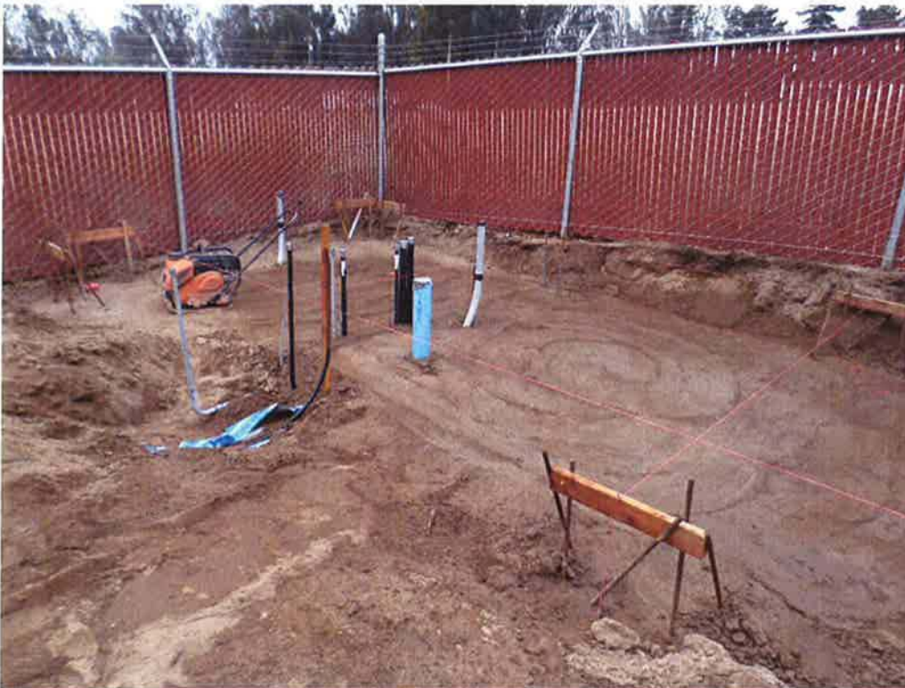
Compacting pipe trenches under future chemical building slab.
