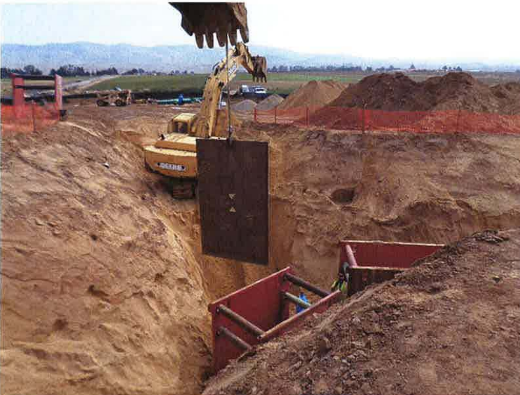
Spiess adjusting shoring at pig launcher location on 24-inch DIP.
