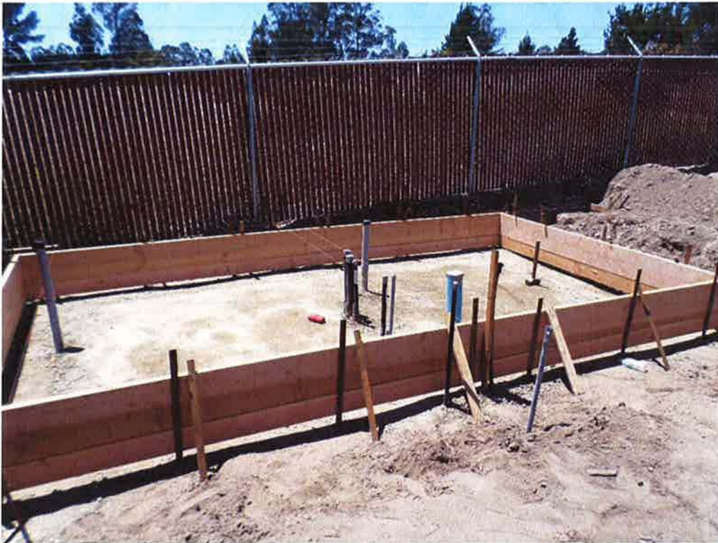
Spiess forming chemical building slab.
