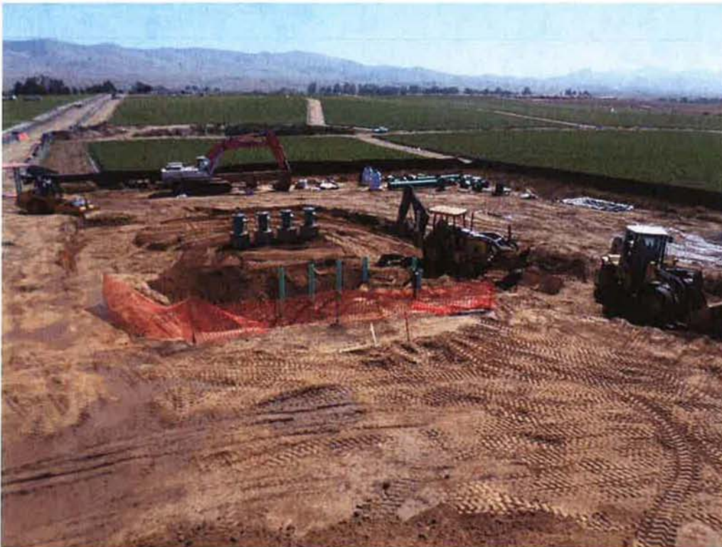
Spiess backfilling around the pump station pump cans and valve risers.
