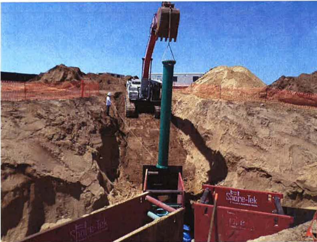
Spiess setting the pig launcher riser.
