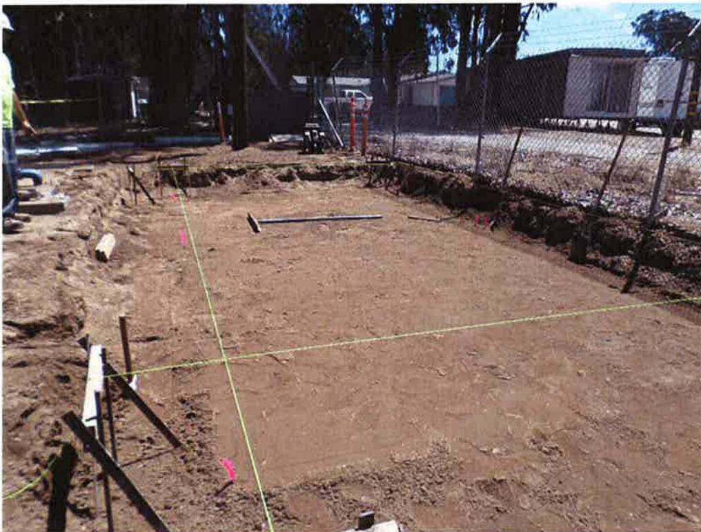
Laying out the chemical building slab foundation.
