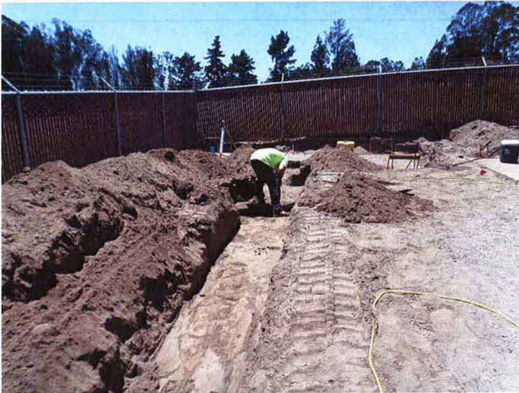
Spies trenching for site piping.
