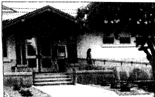
Visitors leave the new Nipomo Community Services District offices at 148 S. Wilson.
