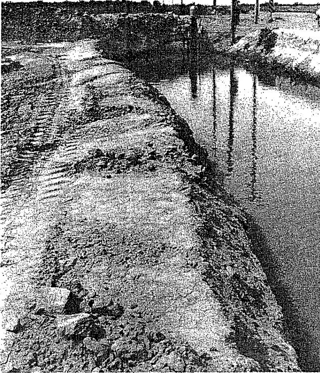
Surface-irrigation return system with sump and pump, which returns the collected tailwater to the field.
