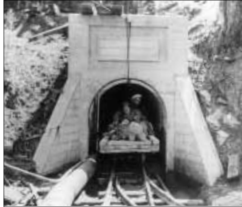
Construction in progress on Mission Tunnel, completed in 1912
