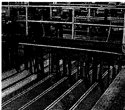
AquaDiamond® backwash assembly and laterals.
