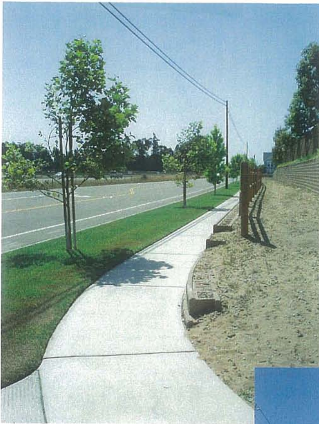
Photo 7: South Frontage Road looking South along Pipeline Route
