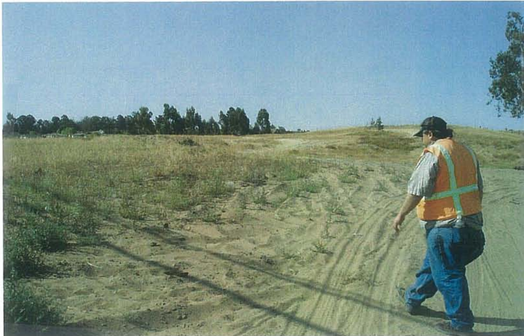
Photo 10: Graded Parcel West of South Frontage Road near Site SLO-808
