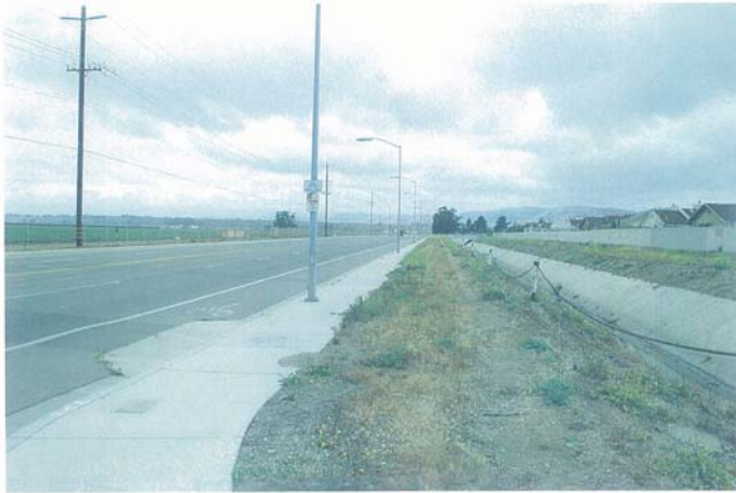
Photo 1: Blosser Road near West Taylor Street along Pipeline Route
