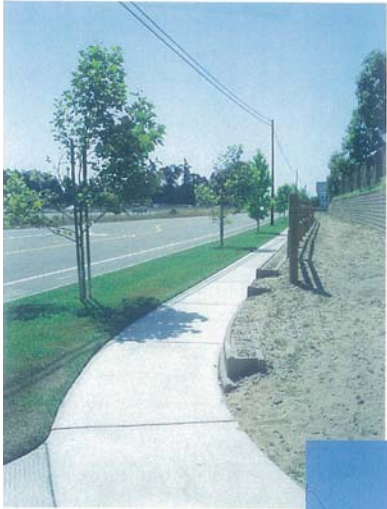
Photo 7: South Frontage Road looking South along Pipeline Route
