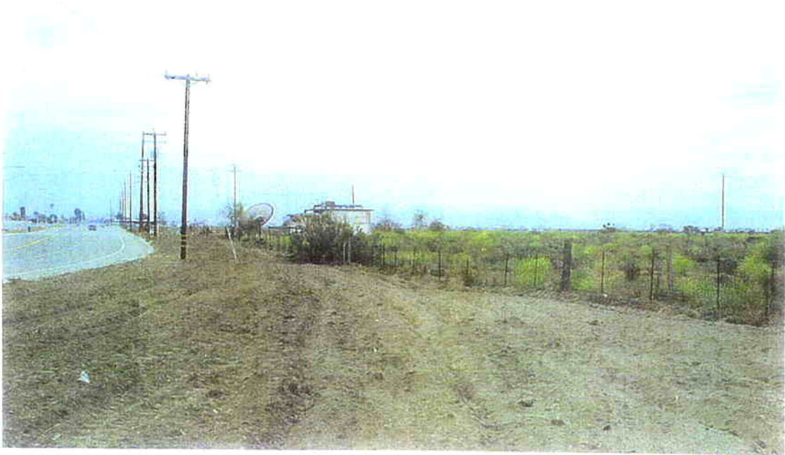
Photo 4: Blosser Road looking South Pump Station No. 1, Site 2
