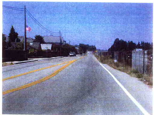
Southland Street and South Frontage Road
