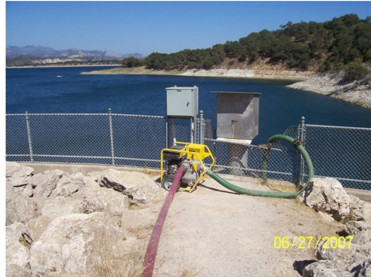
Cachuma Reservoir / Water Level Gauge (Shaft Encoder)
