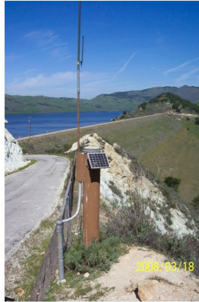
Twitchell Repeater & Reservoir
