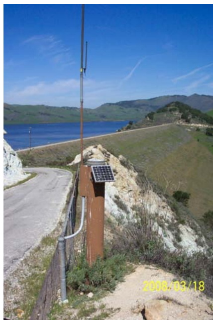
Figures 75 & 76 – Twitchell Reservoir & Dam
