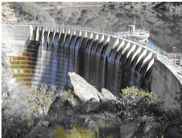
Figure 73 – Juncal Dam & Spillway
