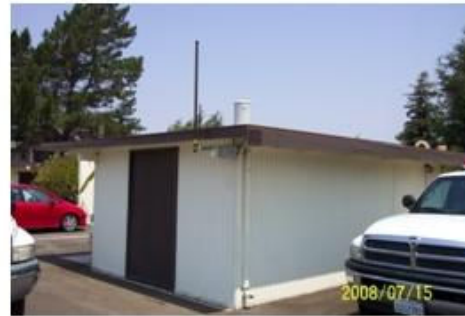
ALERT 0.01" Rooftop Install (Buellton Fire)
