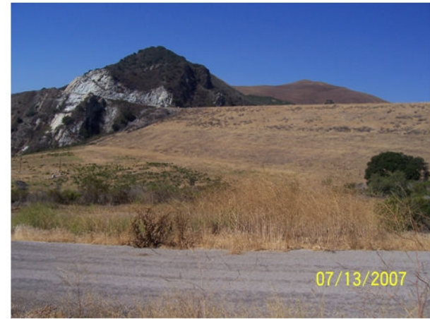
Twitchell Earth-Filled Dam
