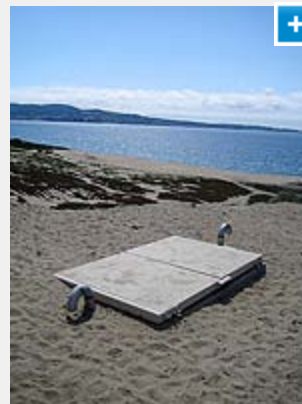
The plant uses reverse osmosis (RO) process to desalinate brackish seawater.
