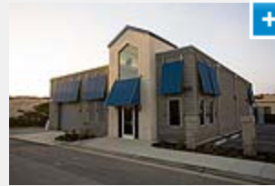
Sand City Coastal Desalination Plant is California's first full-scale seawater desalination facility.
