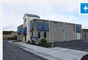
The $11.9m plant became operational in April 2010.
